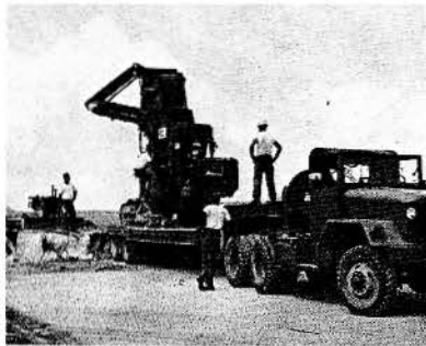
CRAWLER EQUIPMENT IS MOVED EARLY
