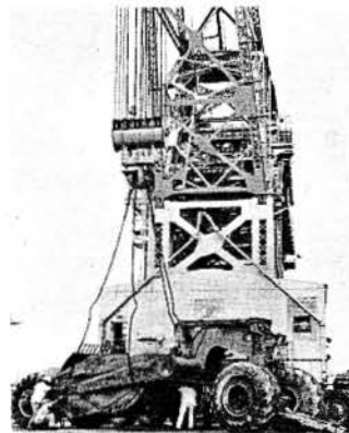
HEAVY EQUIPMENT IS HOISTED BY CRANE
