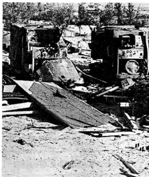
FIGURE 88 SABOTAGE OF PROJECT MATERIAL
