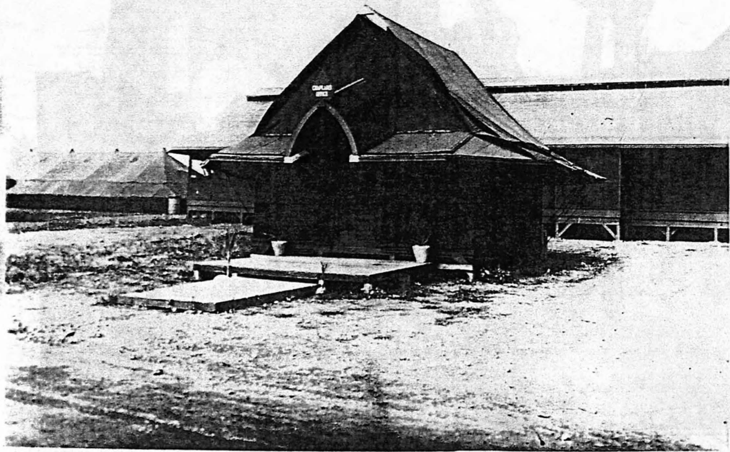
194 "We built an office for (Chaplain) Toomey. Then we built a Chapel." The Chapel is seen in background right. Ace of Spades above 1st roof. Photo-NAVFAC-P.H.
