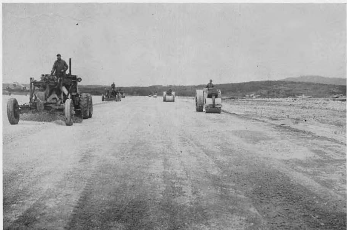
ROLLING AND GRADING
