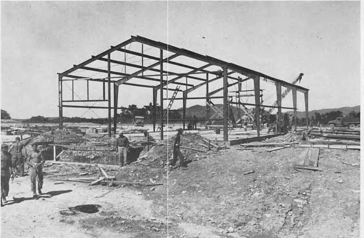
A BUTLER BUILDING
