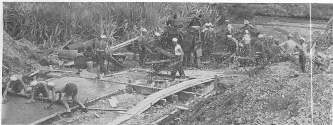
FOUNDATION FOR AIR RAID SHELTER
