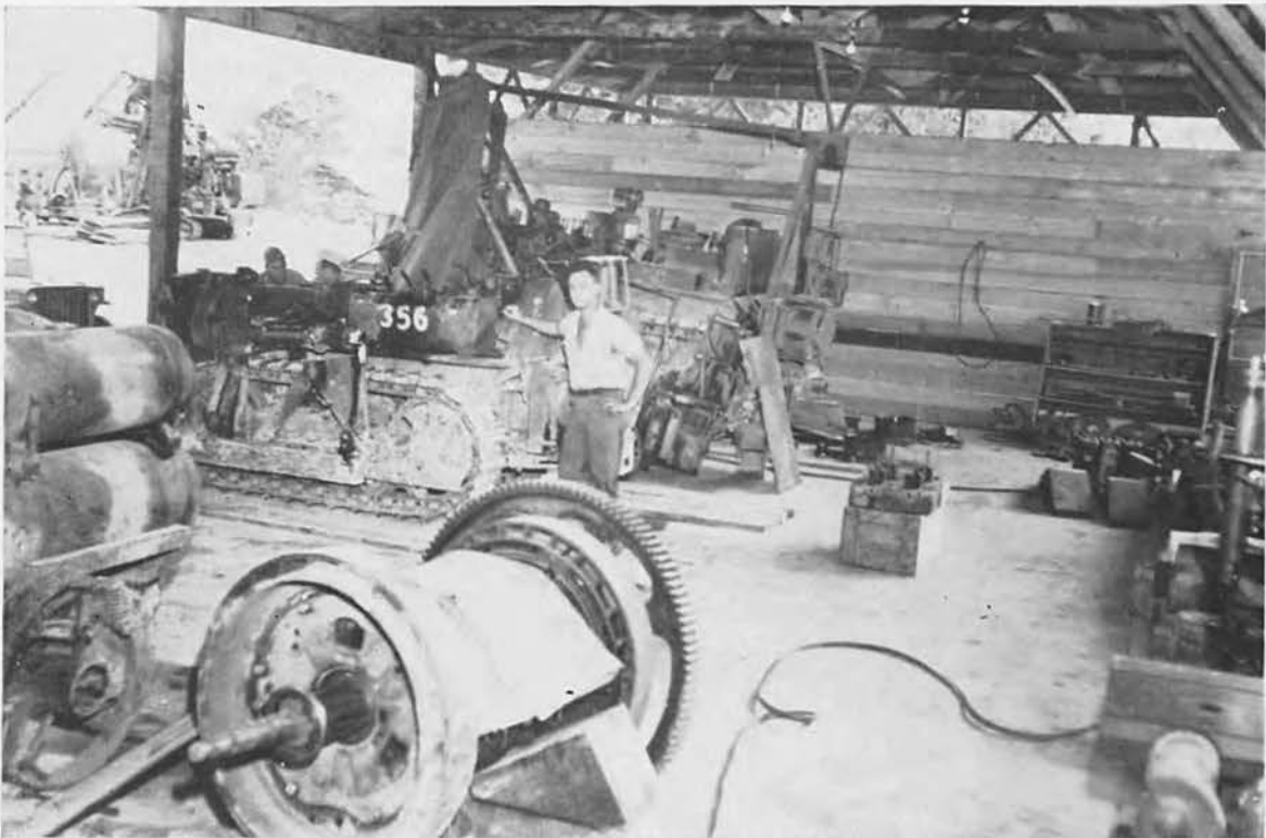
HEAVY EQUIPMENT REPAIRS
