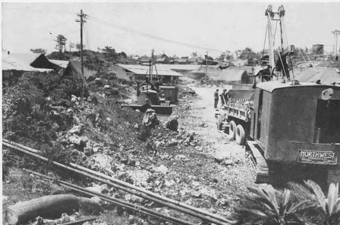
GRADING FOR MESS HALL
