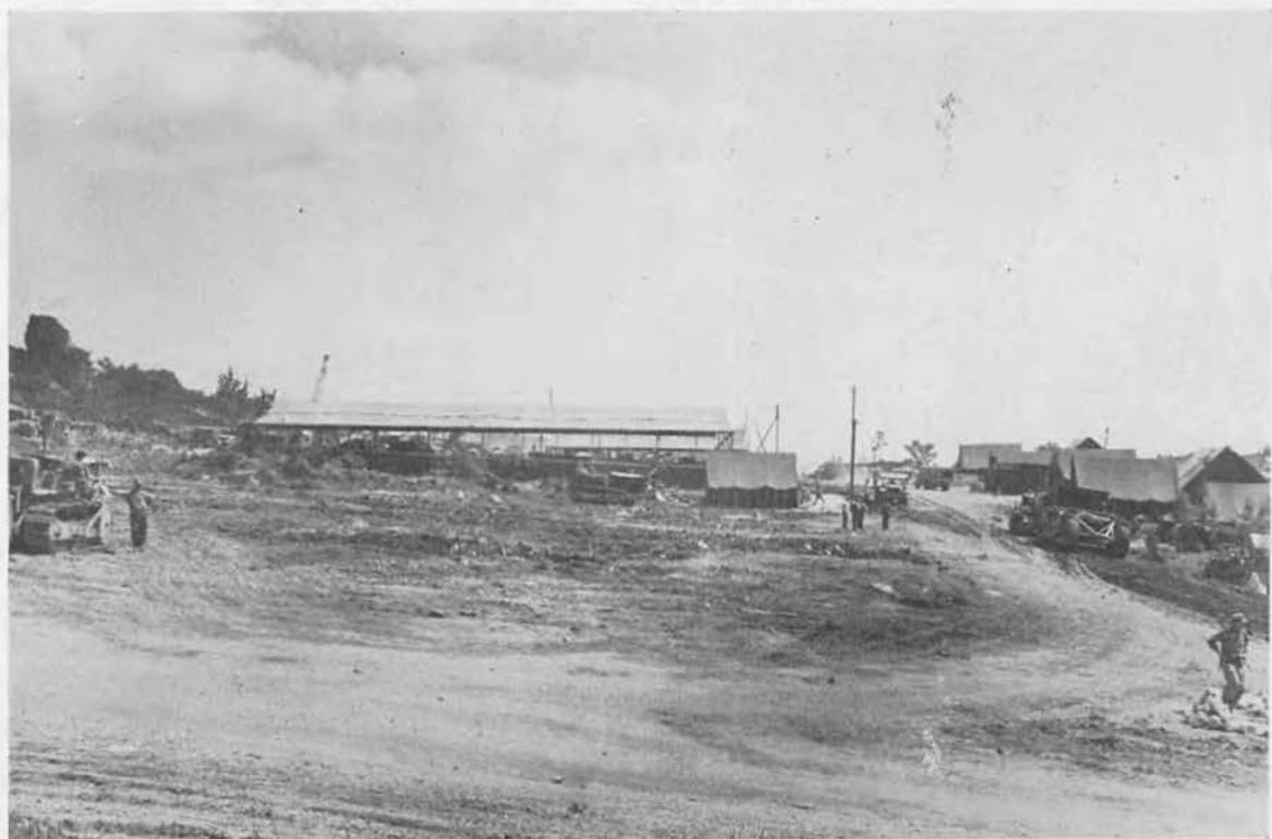
CONSTRUCTION OF PERMANENT CAMP
