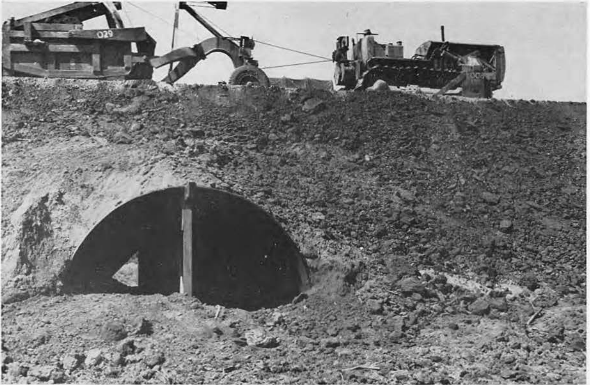
FINISHED CULVERT
