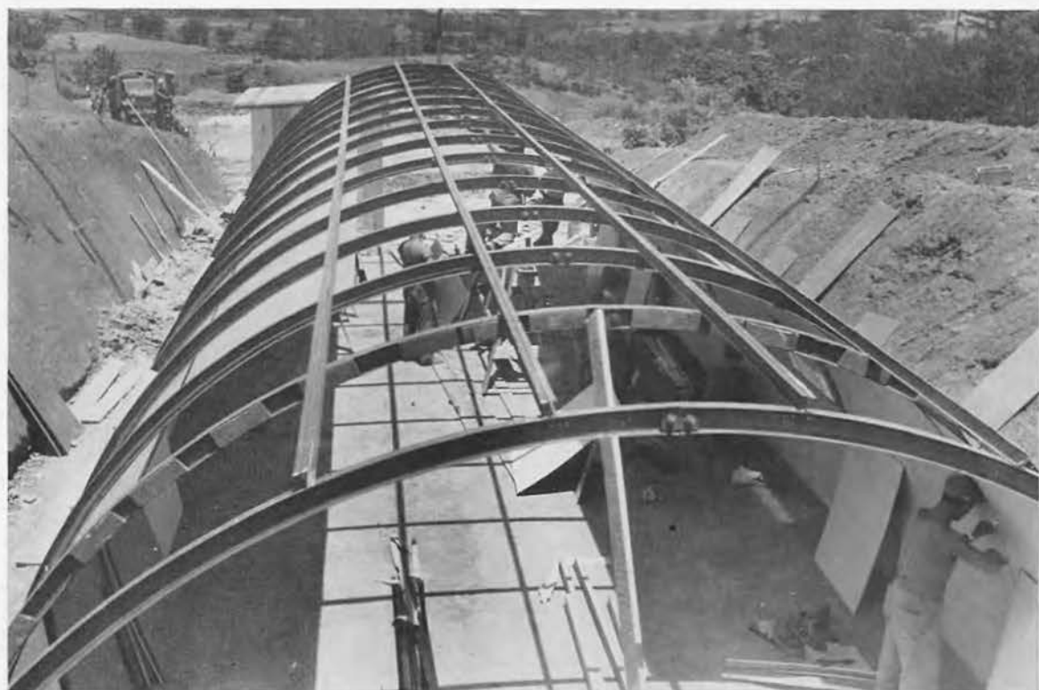
CHINA TELEPHONE EXCHANGE
