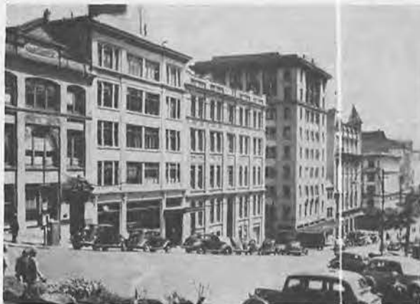
TOP OF QUEEN STREET
