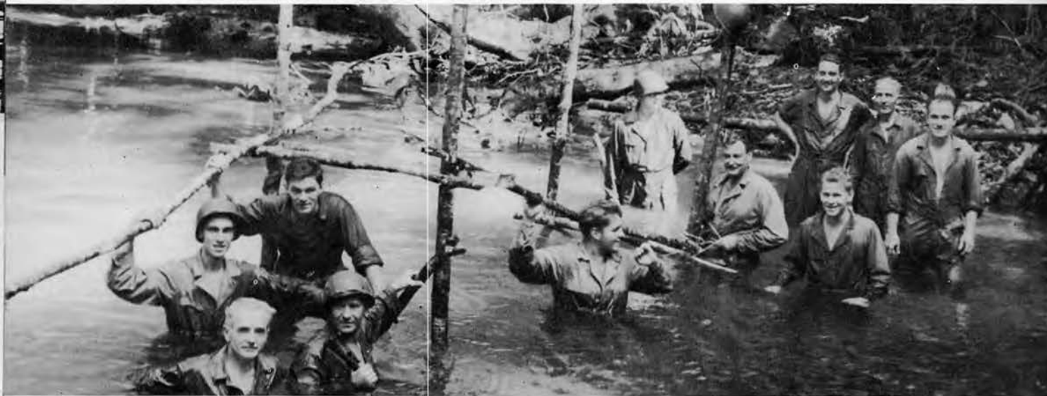
▼ The Commandos build a Foot Bridge
