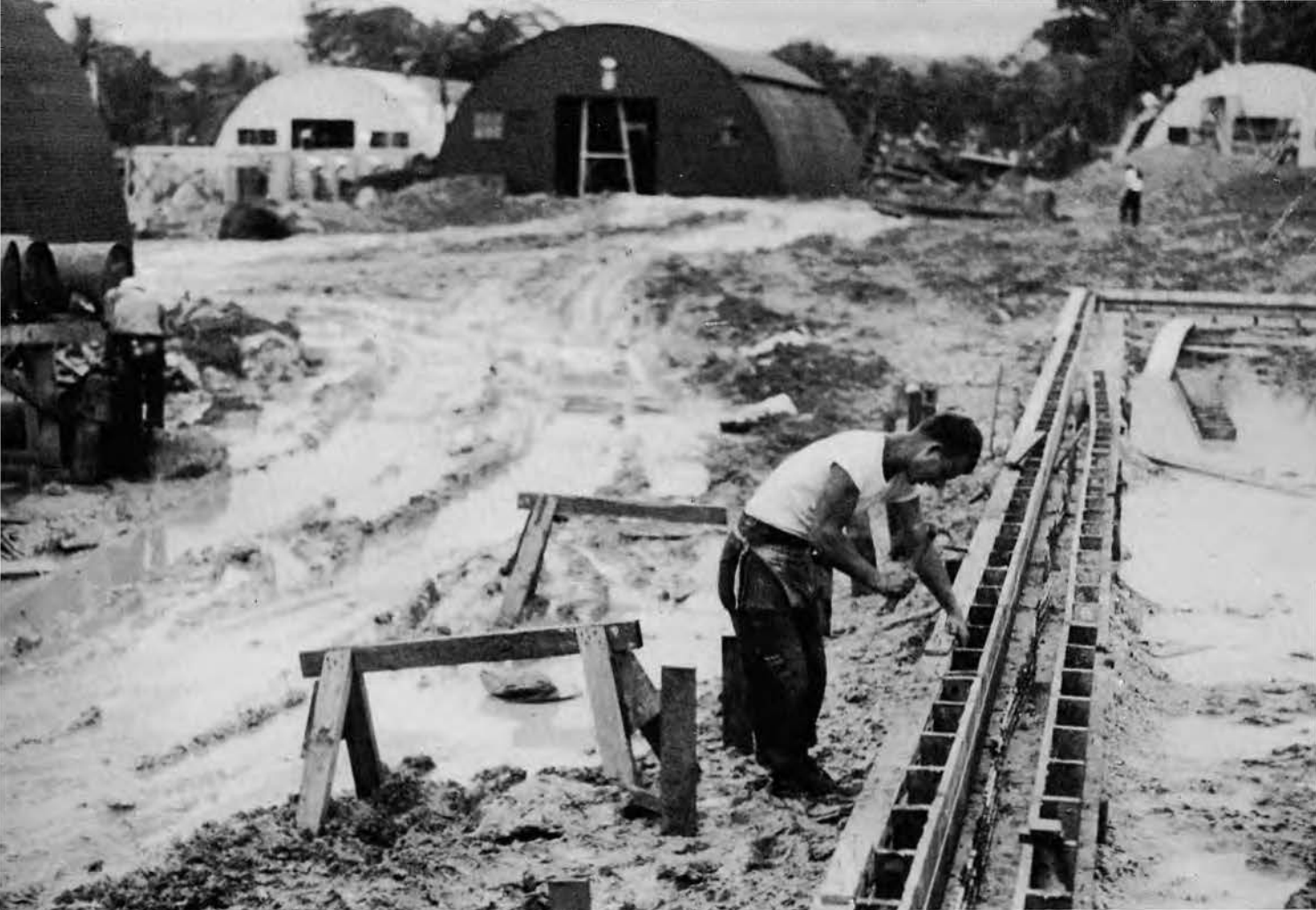
▲ Aligning Footing Forms
