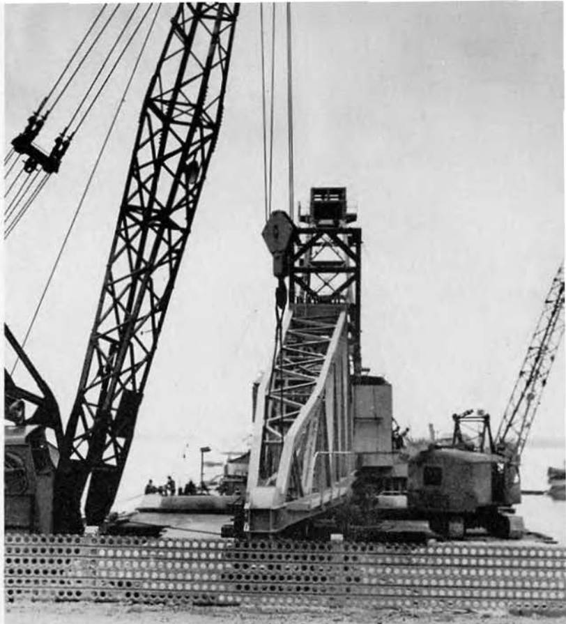
Rigging the Boom
