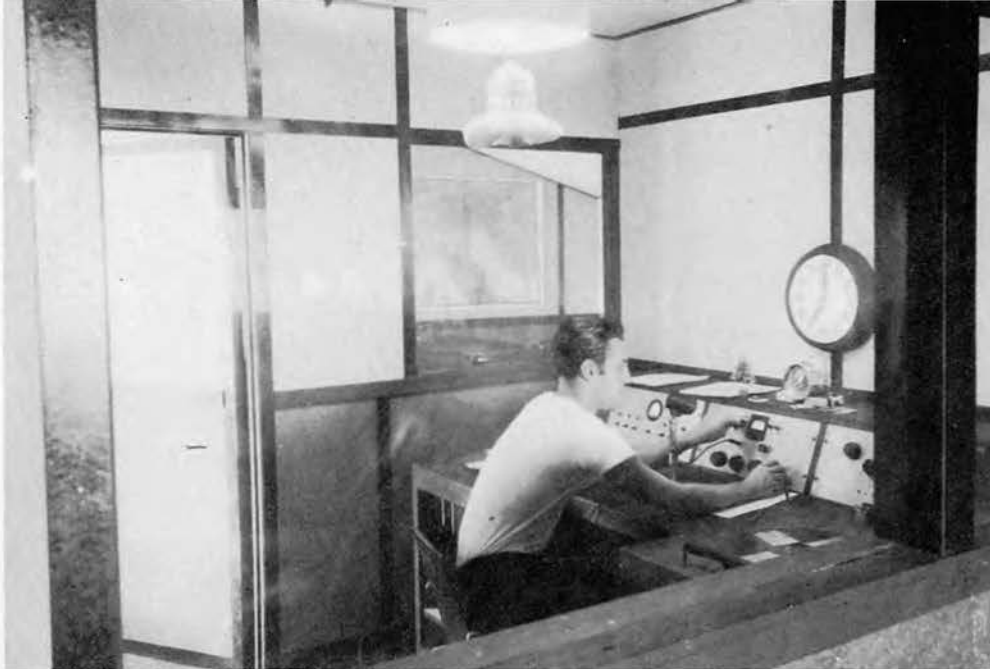
Broadcasting Room, Base Radio Station
