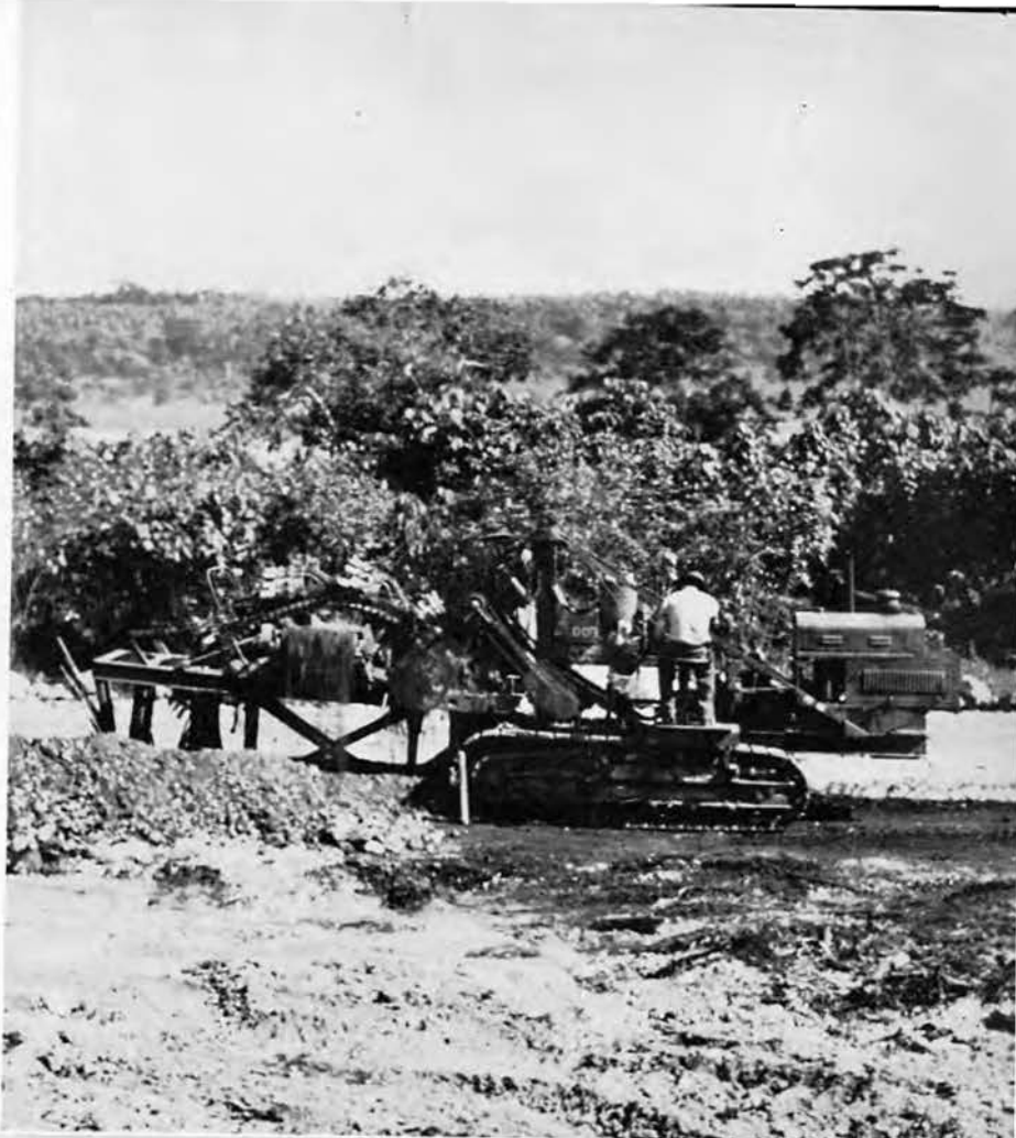
Ditch Digger churning Pipe Trenches . . .
