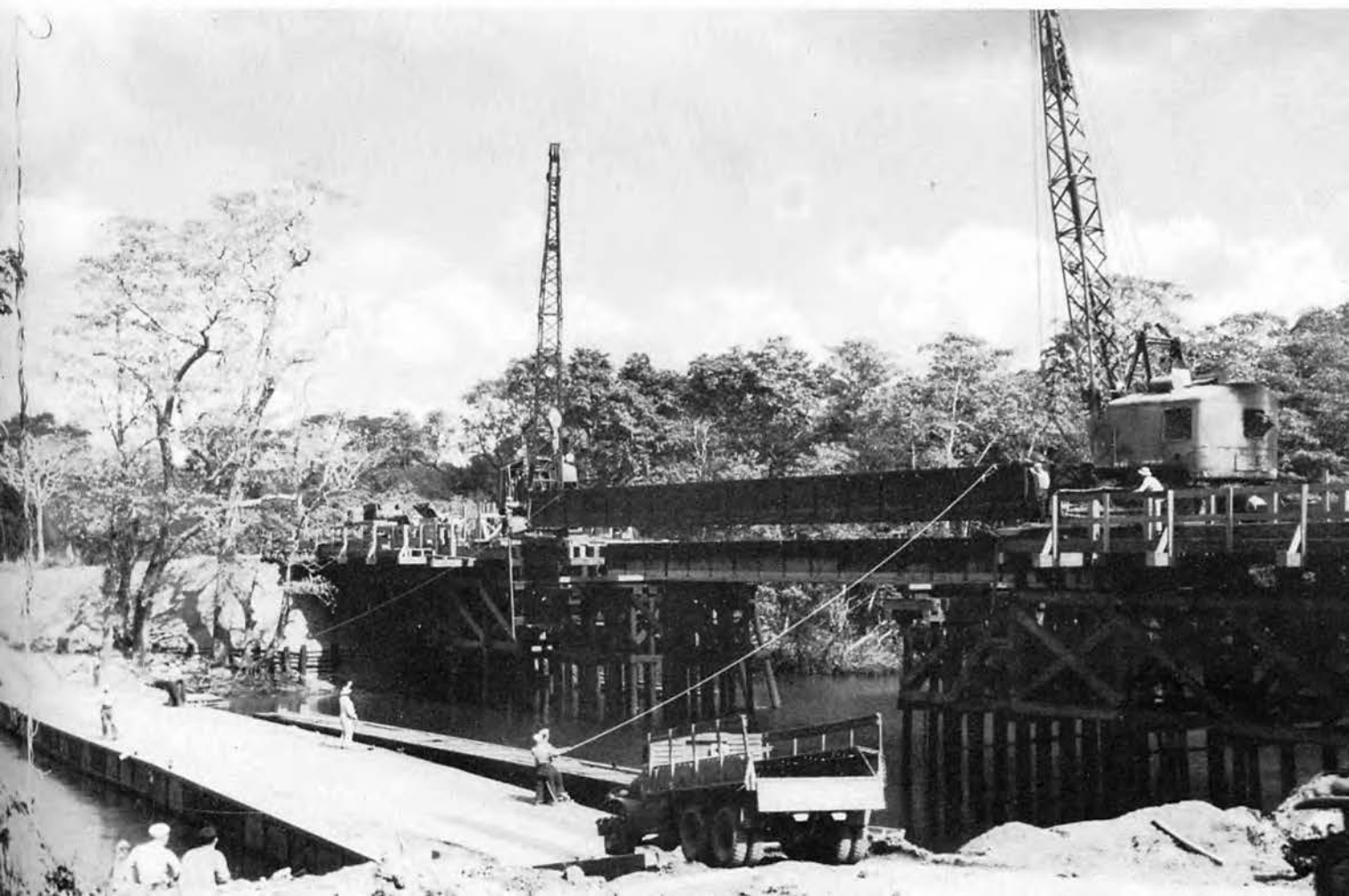
The Sarakata Bridge was built by the 57th and 44th Battalions. These pictures show the placement of the Pontoon Strings
