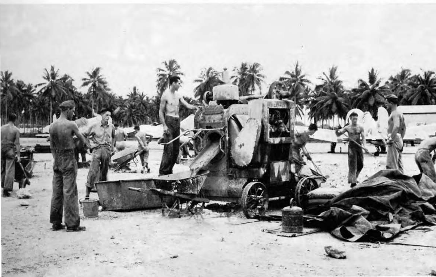
▼ Concrete Crews poured foundations for Hangars
