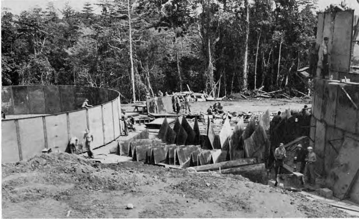
Progress shots of Water Tank construction
