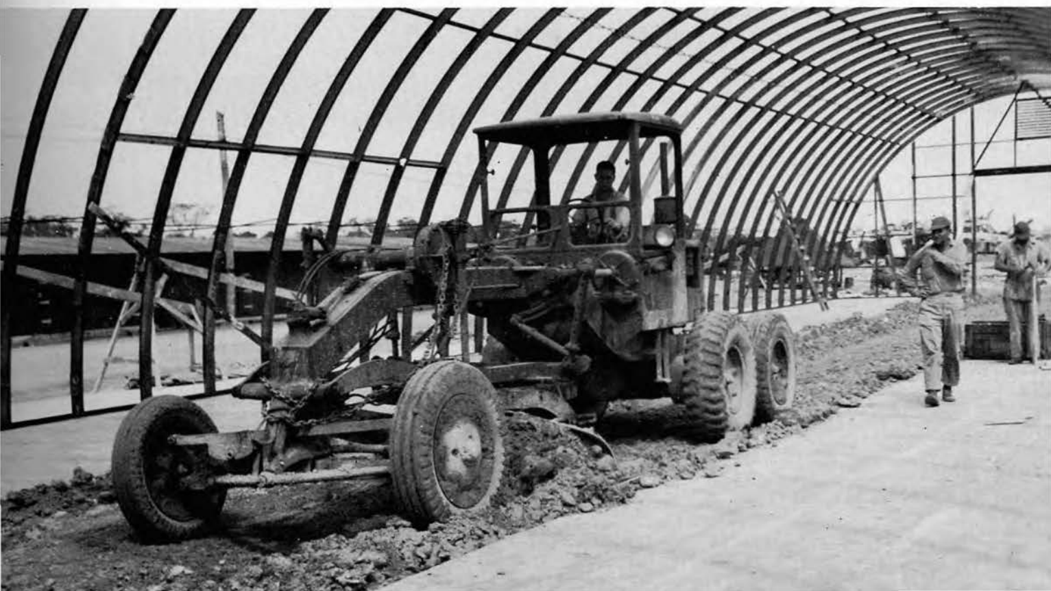
▼ Grading in the Spud Locker
