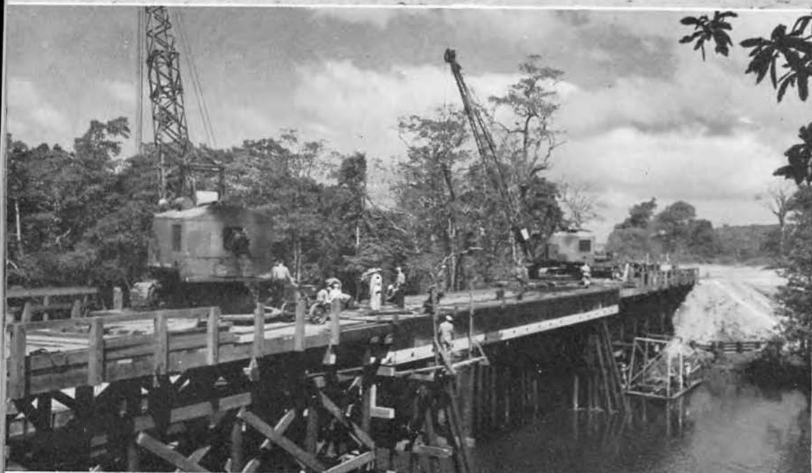
Temporary Pontoon Bridges were rapidly constructed
