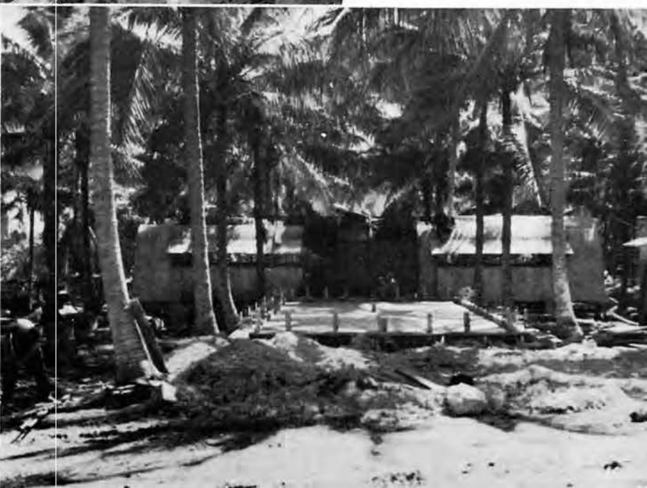
Mess Hall under construction
