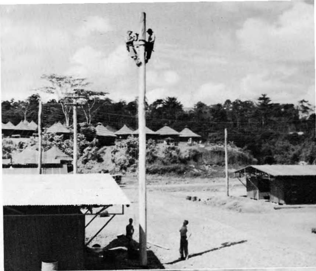
Installing power lines to Reefers
