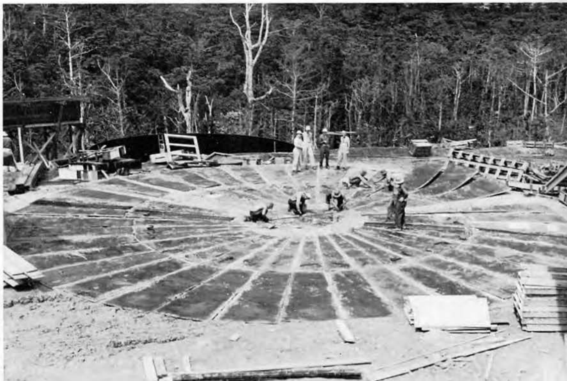
Deck Layout for Water Storage Tank
