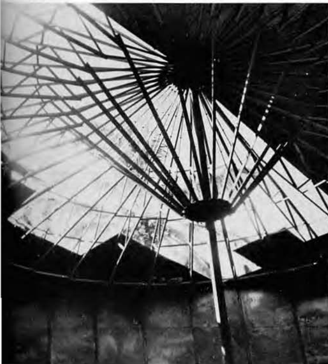
Setting Rafters for the Roof Plates
