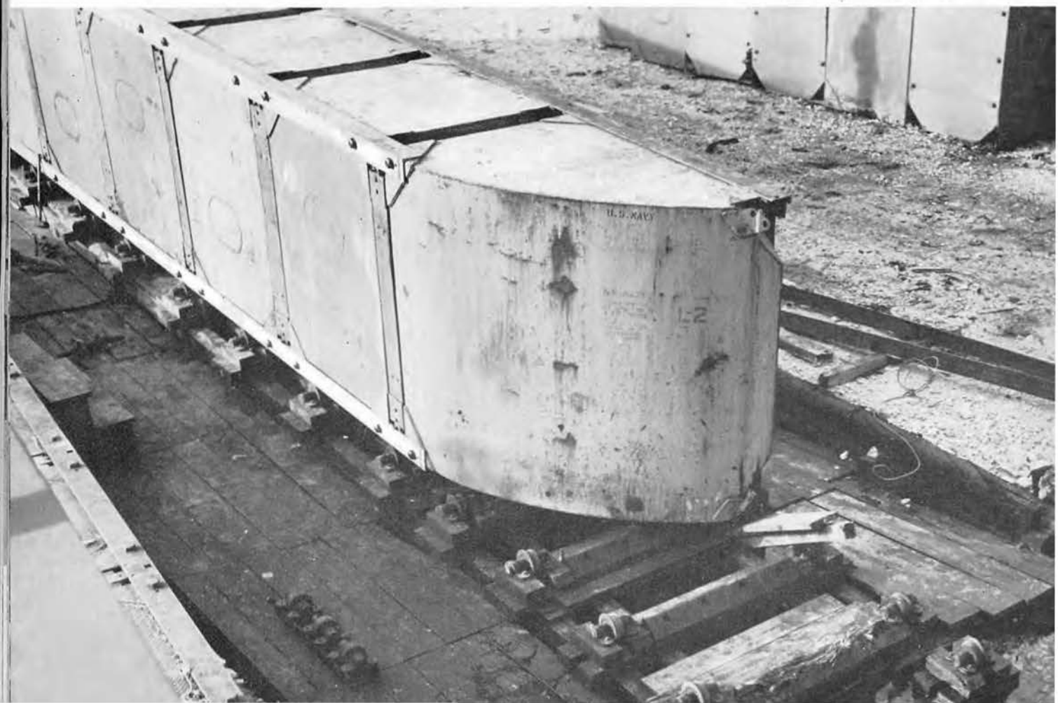
▼ Assembled string ready for launching
