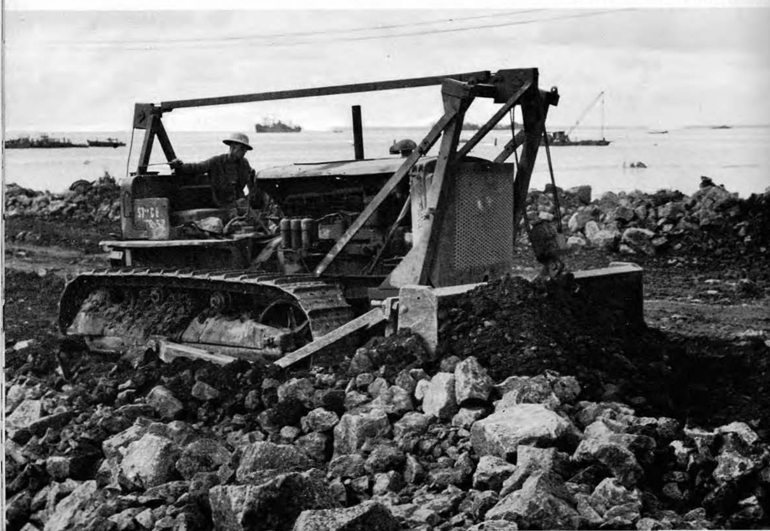
▼ Bulldozer cutting Victory Highway
