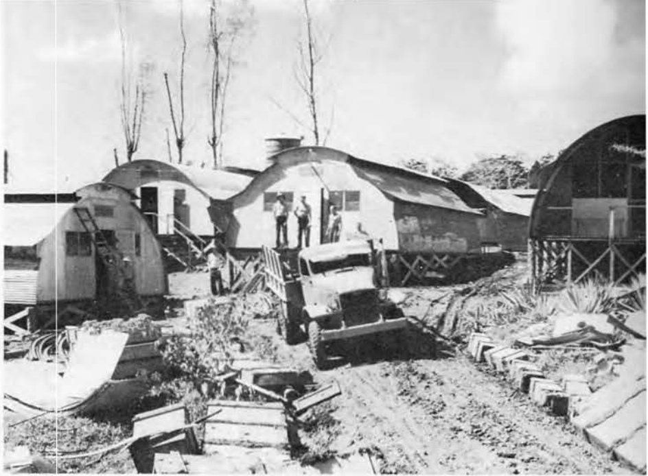
Base Dispensary under construction
