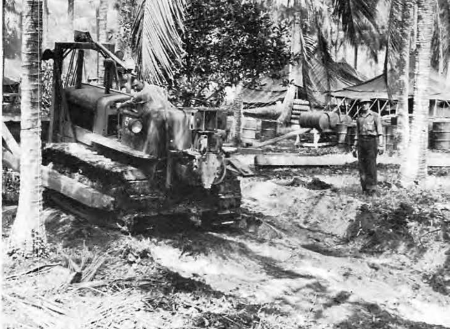
Excavating for Grease Rack
