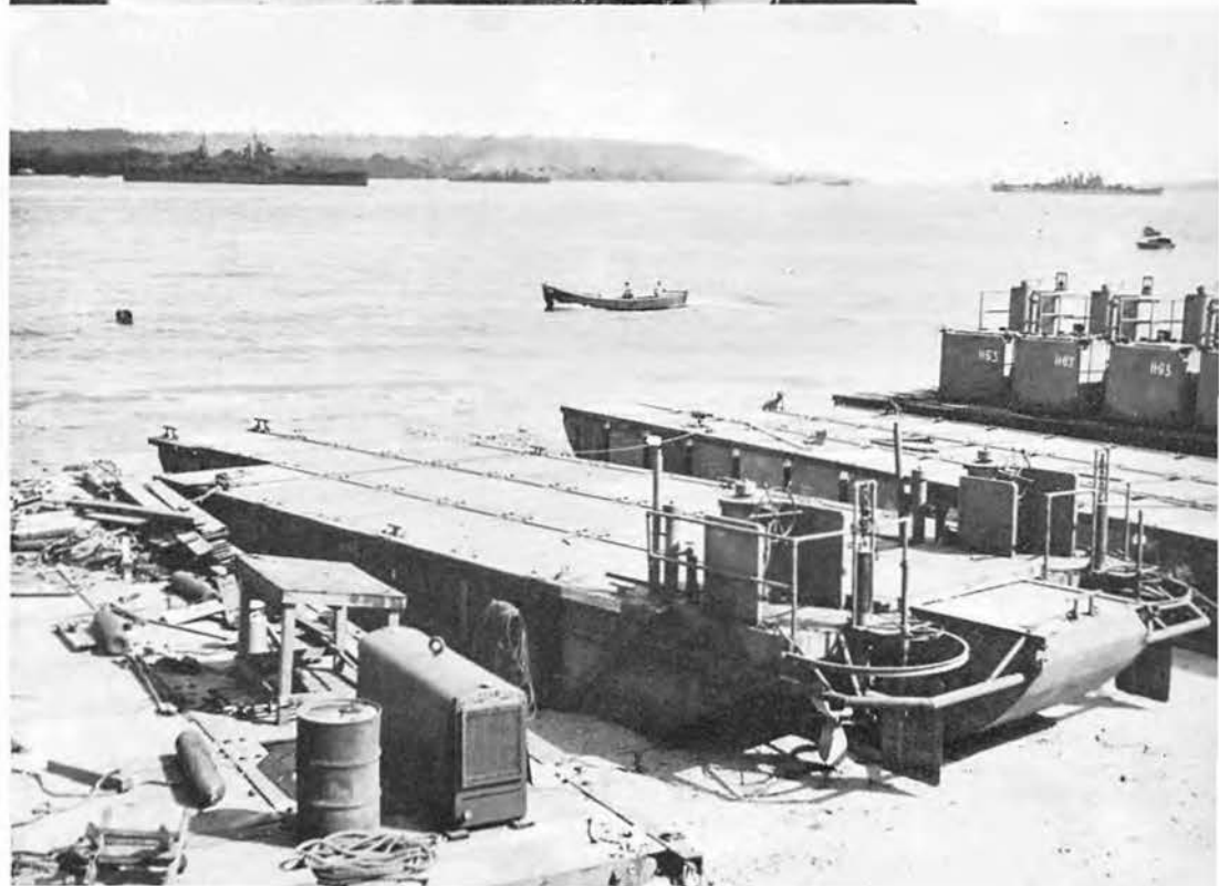
and final Barge Assembly
