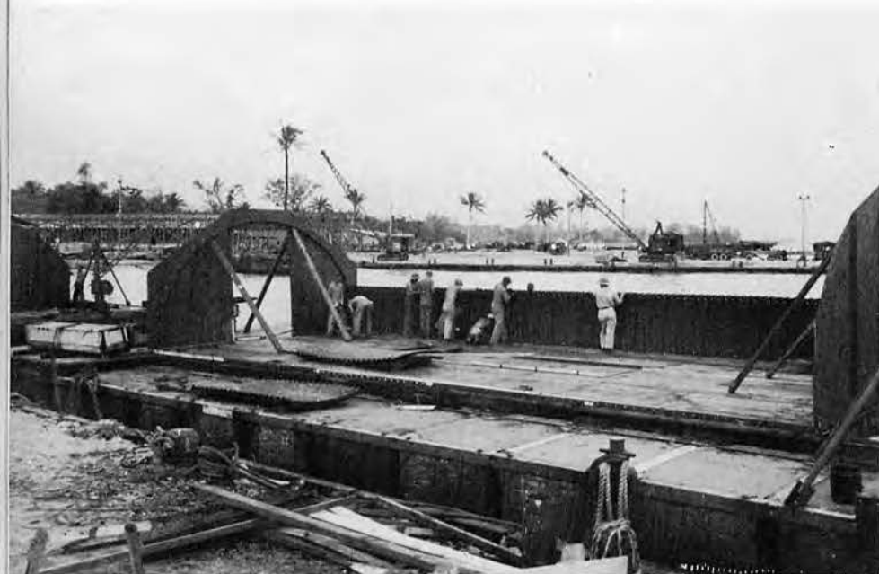
Setting the steel
