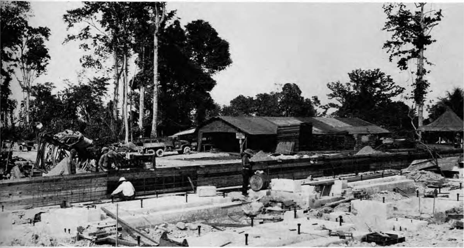
▲ 52 yards of concrete were poured in each of these Generator Footings
