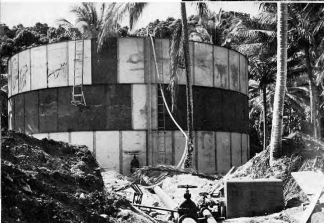
Valve and Pump installation
