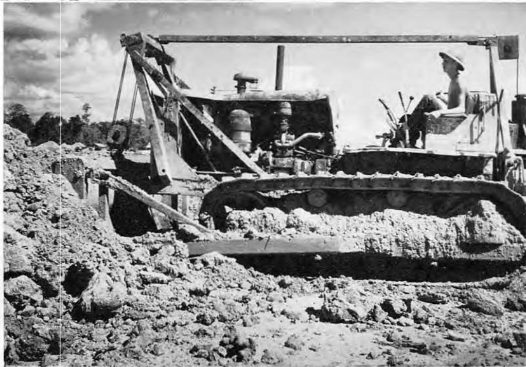
Bulldozer at work on beach road
