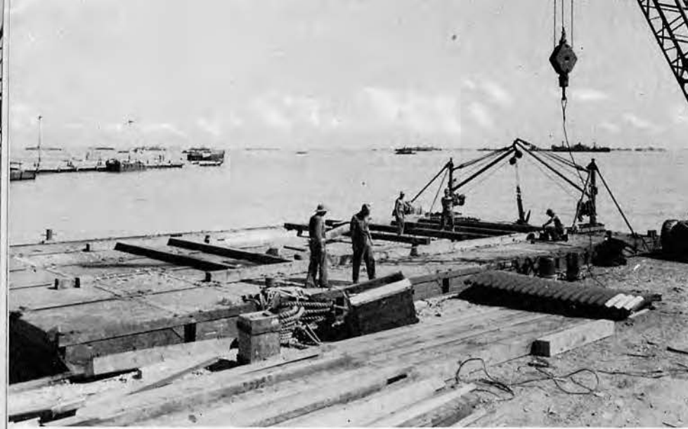
Pontoon Barge with timber for Magazine Foundations
