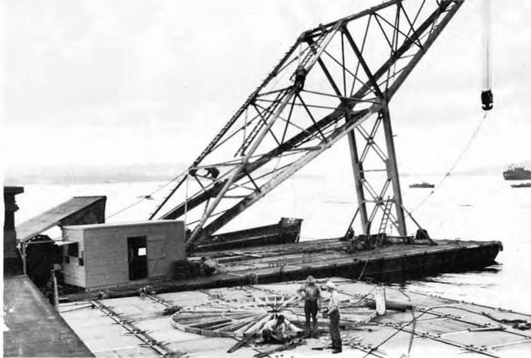
Pontoons were also used for Floating Stiff-legged Cranes and . . .
