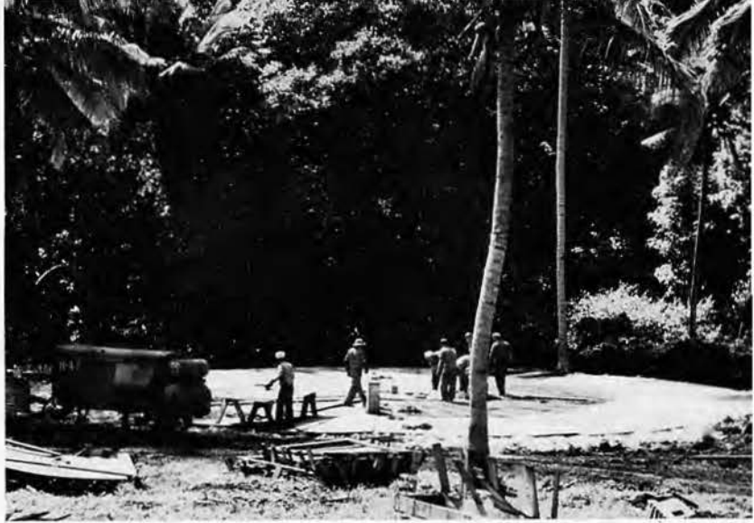
Laying the Deck
