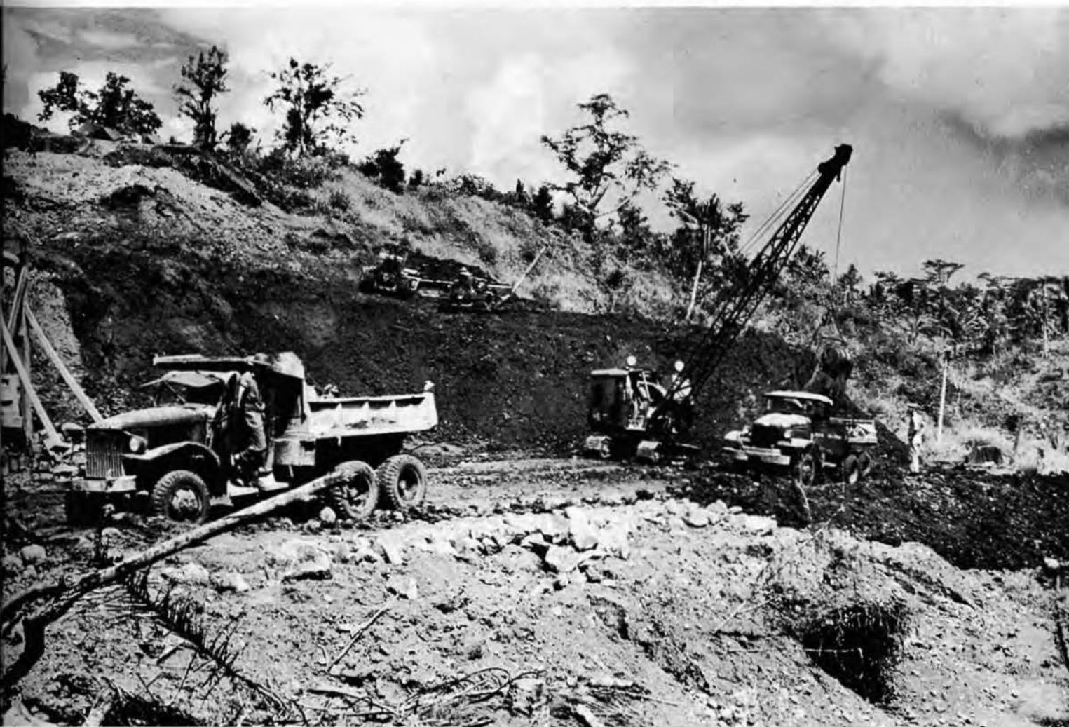
▼ Dragline loading rock for transportation to Crusher
