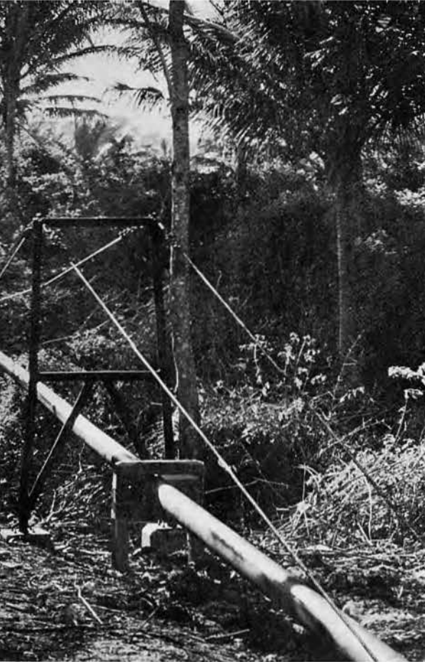
d supported across ravines by Suspension Bridges
