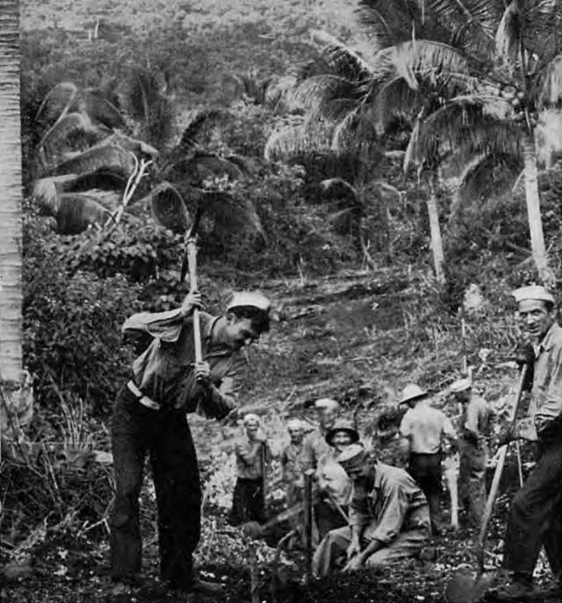
Pipe Ditching - by hand
