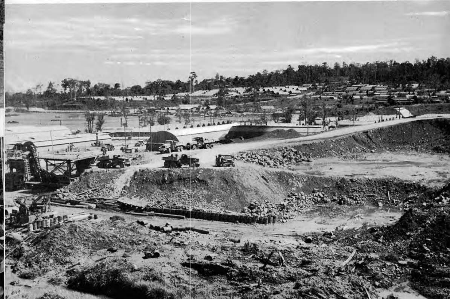
▼ General view of Quarry and Crusher
