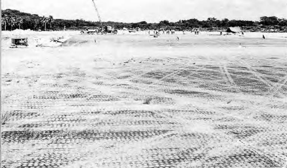
Finishing a Plane Parking Area
