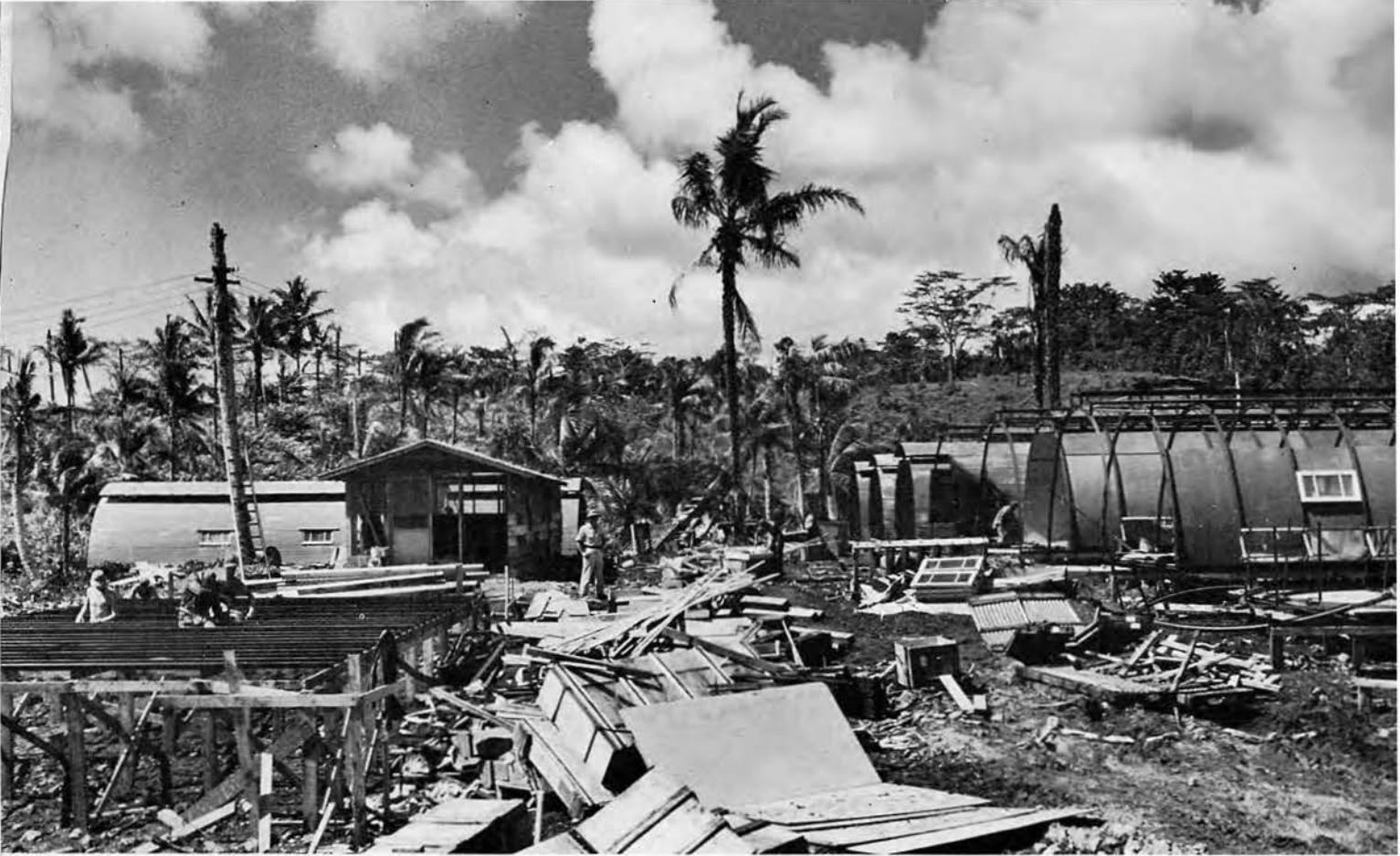
▲ Personnel Living Quarters under construction
