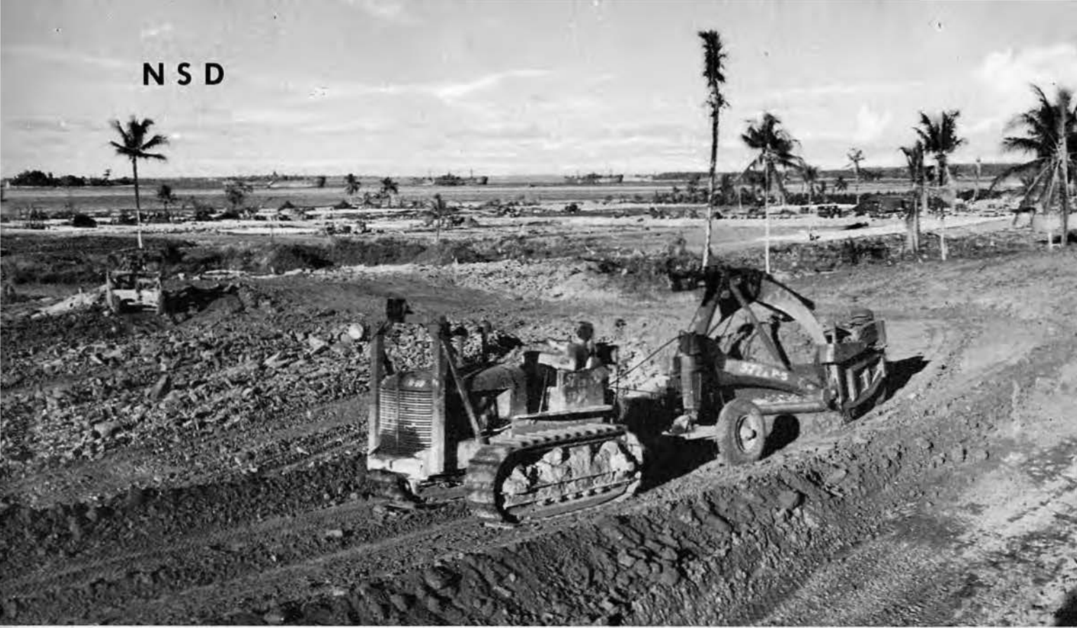
▲ Carryall discharging coral fill for NSD Warehouses
