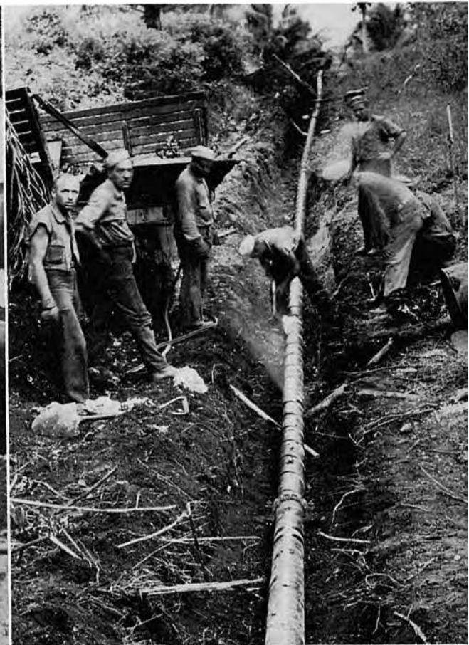
... was rapidly laid ...
