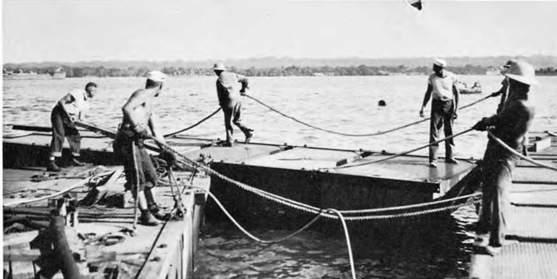
Maneuvering pontoons into position . . .
