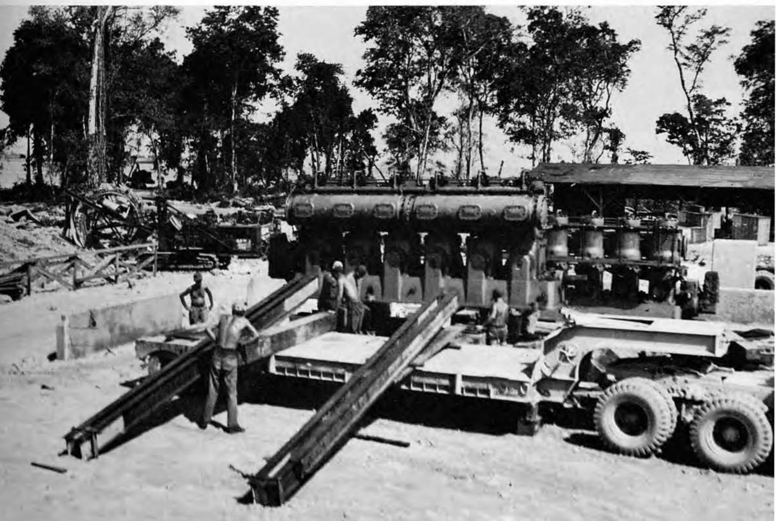
▼ Installing the Generators
