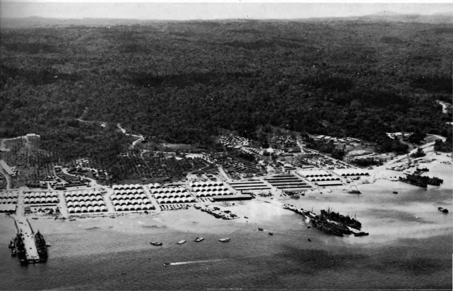
▼ Aerial view of NSD Area
