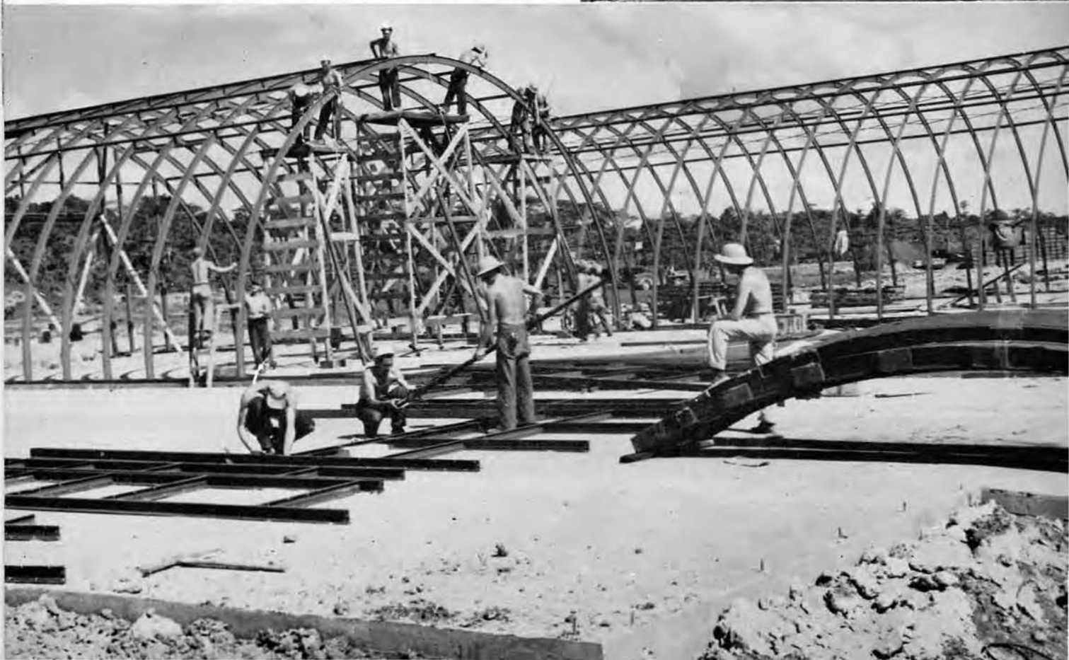
Erecting Ribs and assembling Bulkhead
