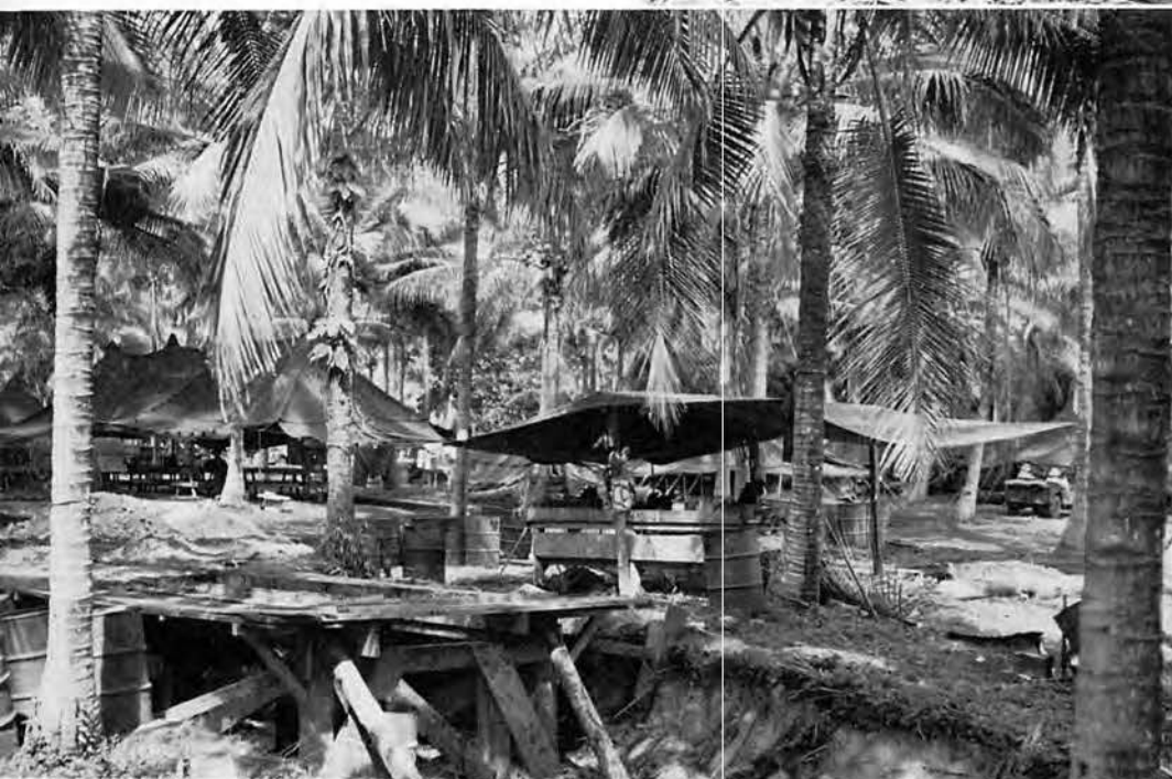
Completed Improved Grease Rack - Temporary Mess Hall at left rear
