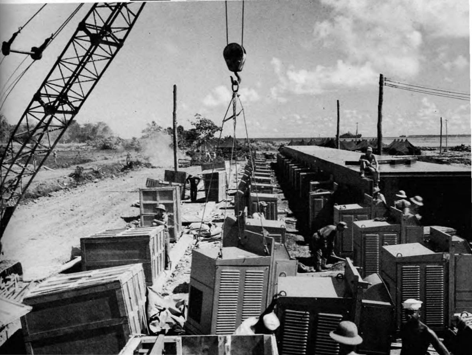
300,000 cubic feet of Refrigeration being installed
