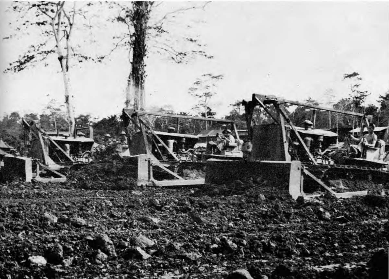
▼ Rough grading the Open Storage Area
