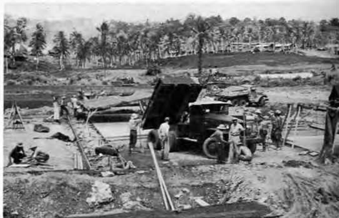
Pouring concrete deck for 40'x100' Warehouse
