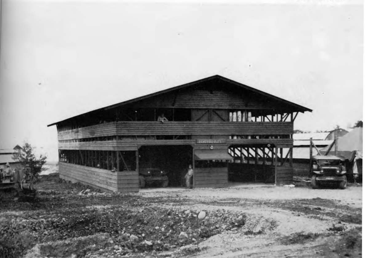
▼ NAB Fire Station
