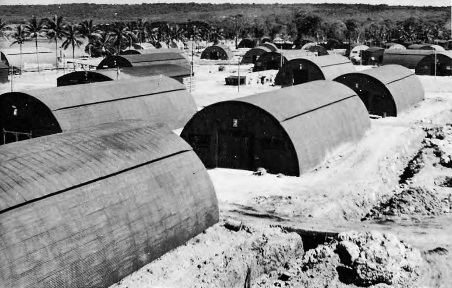
▲ Completed Quonset Warehouse . . .
