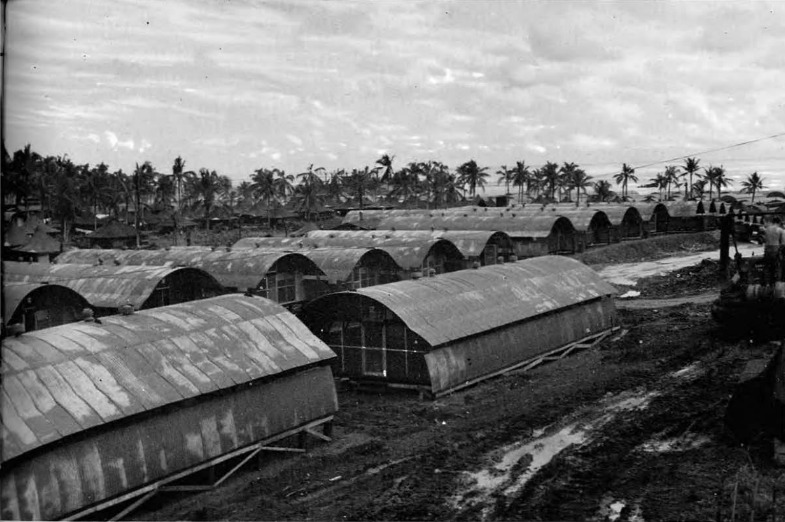
▲ Completed Personnel Camp Area
