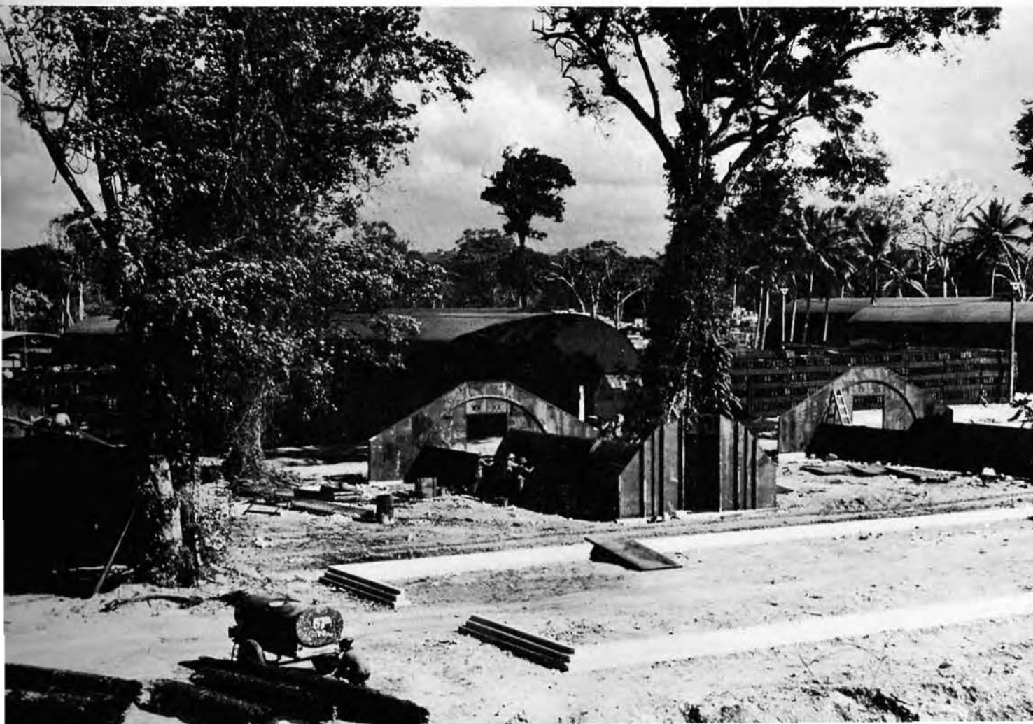
▼ . . . and Ammunition Magazines partially complete
