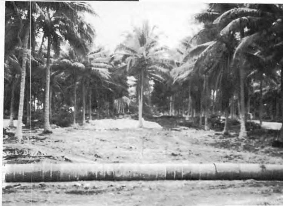
... Culverts made from discarded oil barrels
