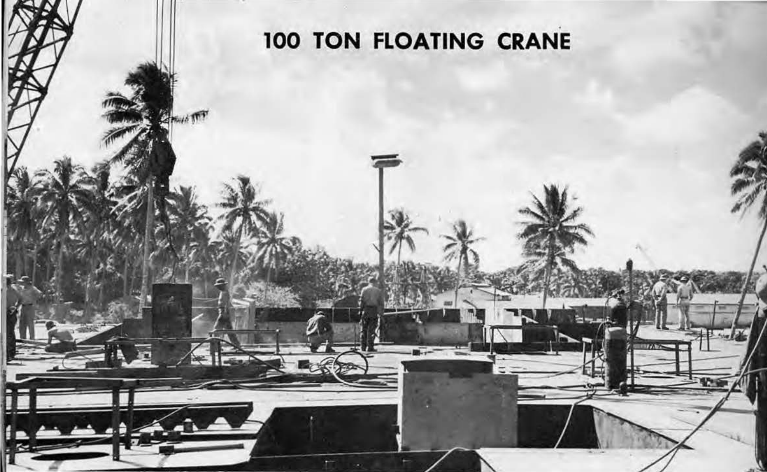
▲ Laying the Deck Plates
