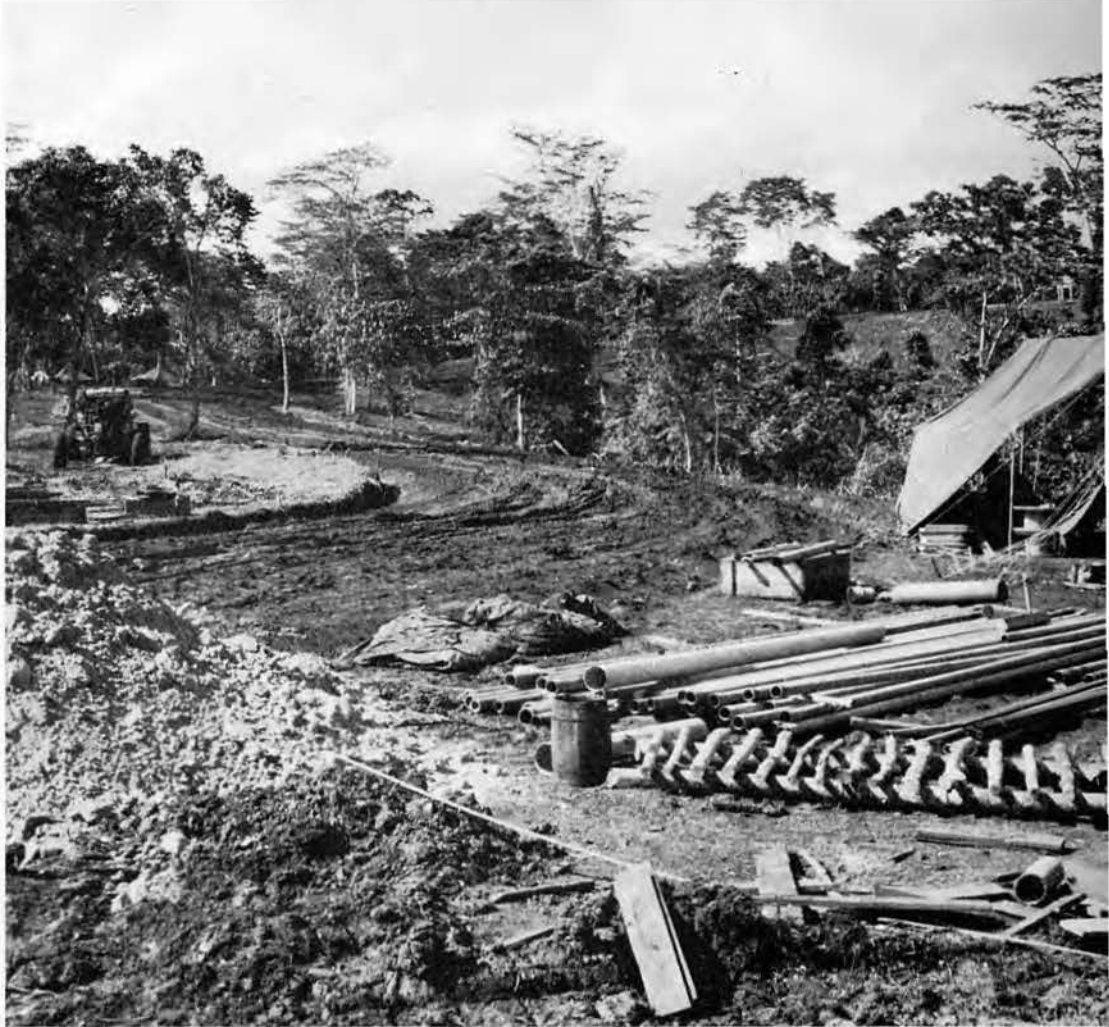
Constructing road through our permanent Camp
