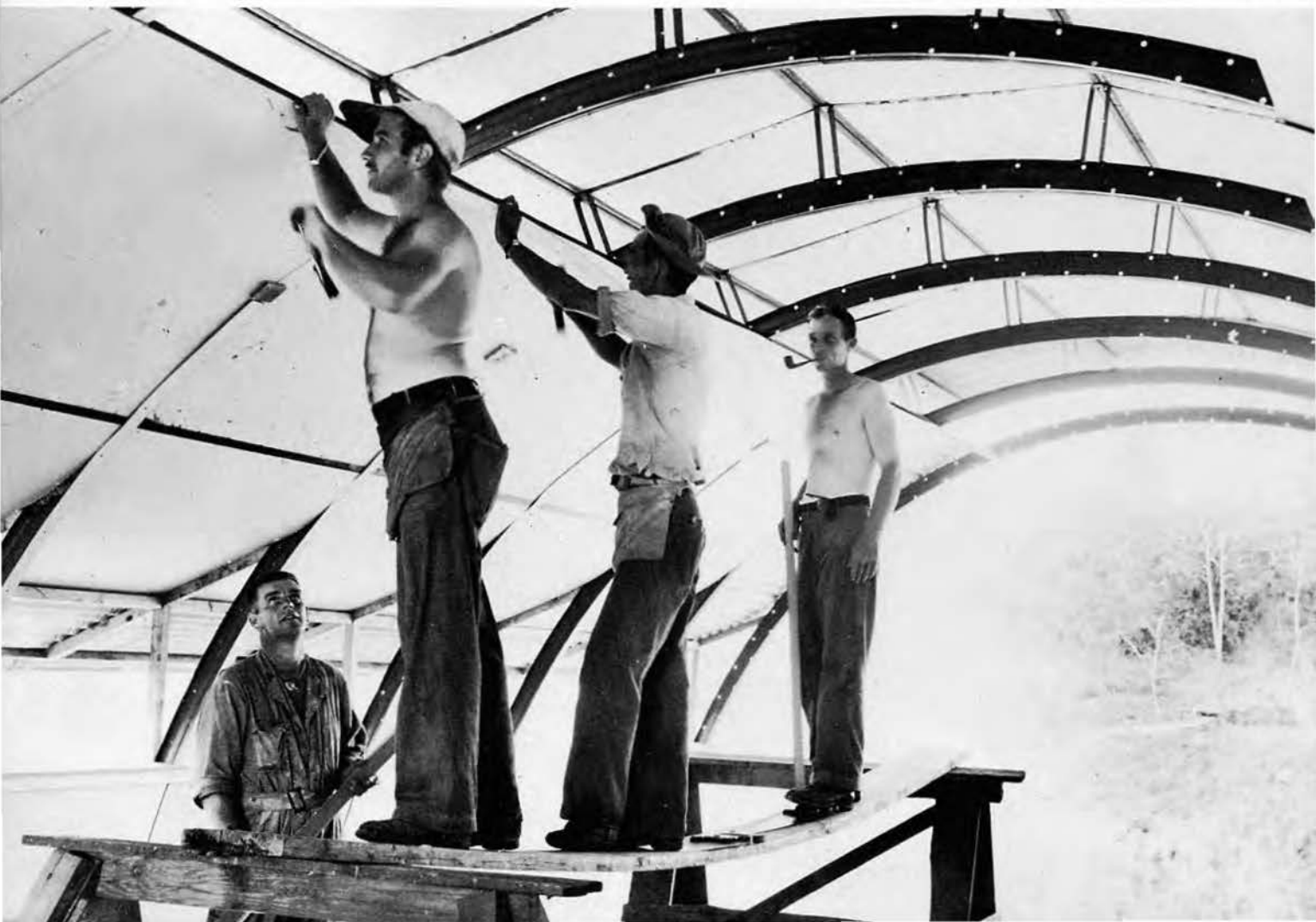
▼ Finishing interior of 20'x48' Quonset Hut
