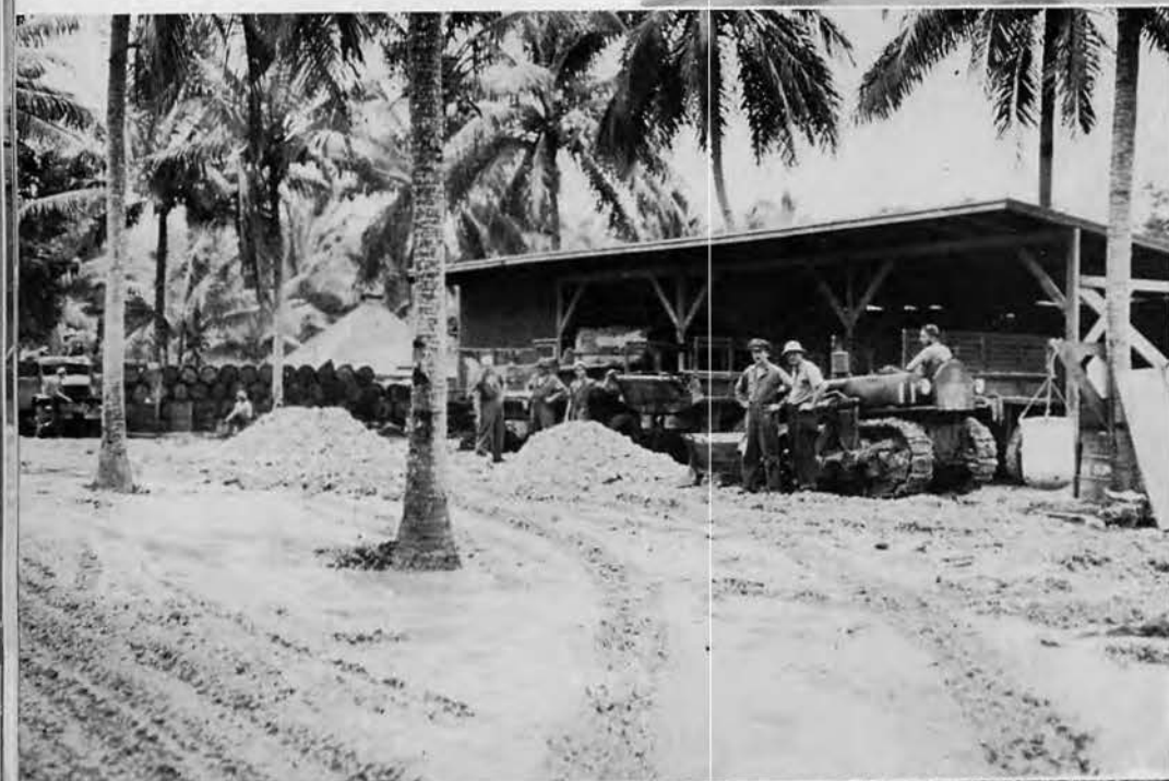
Coral Surfacing Heavy Equipment Area
