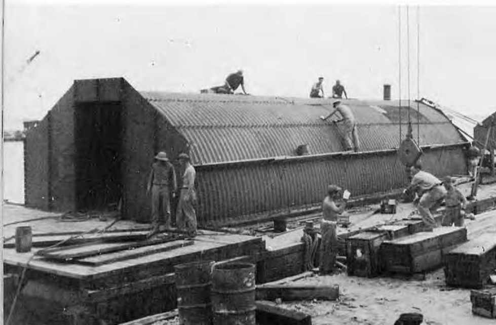
Caulking the joints
