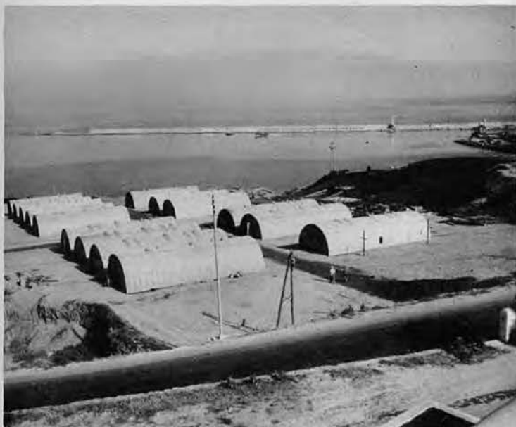
Quonset Camp, Mostaganem
