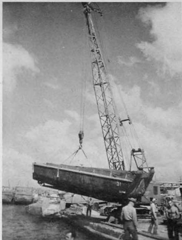
Damaged Landing Craft
