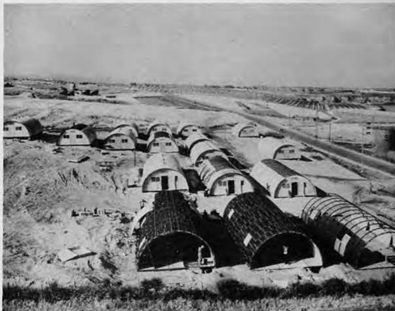
Hospital Unit, Mostaganem
