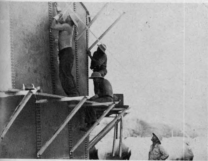
Building a 3,000-bbl. Tank Barge at Karouba. Barge Was Used to Haul Gasoline to Sicily.
