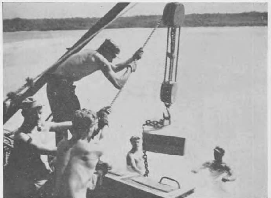
Laying anchors for submerged pipe line. Lundy, CM1c, smoking pipe; Steve Kusiak, SF2c, on right. Others: 25th NCB.
