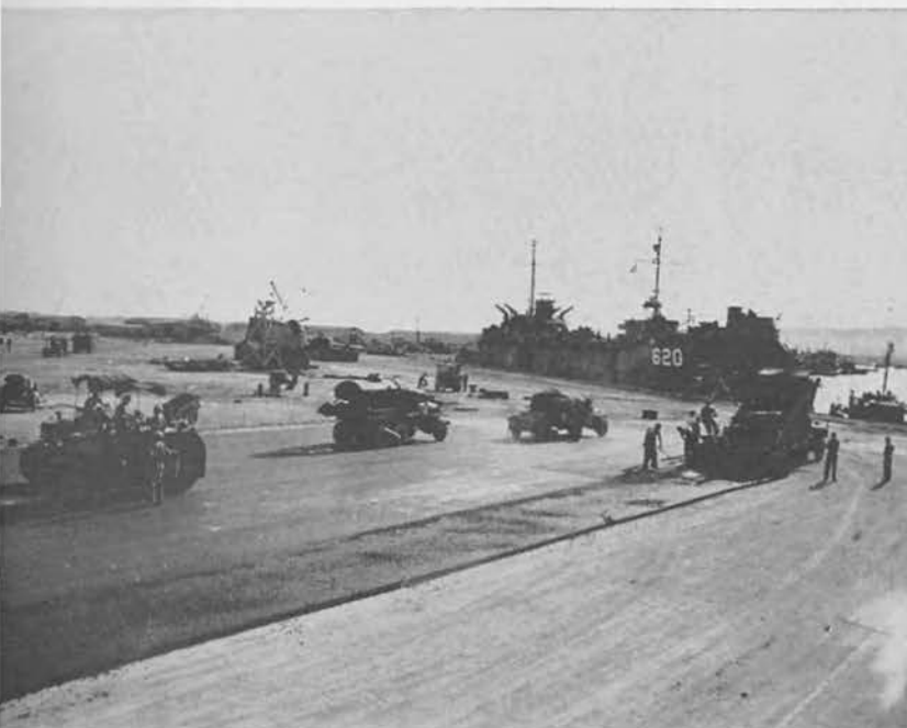
Paving a 100 foot strip at the docks.
