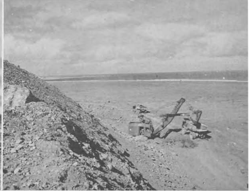
Shovel at work on the Seawall Cut.
