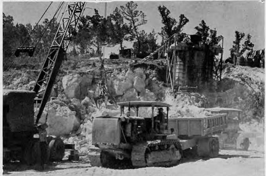
An Athey wagon gets its load of rock as this hill is cut back in order to widen the main road from Gate No. 1.
