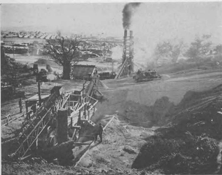
View of Crusher and Asphalt Plant in operation.
