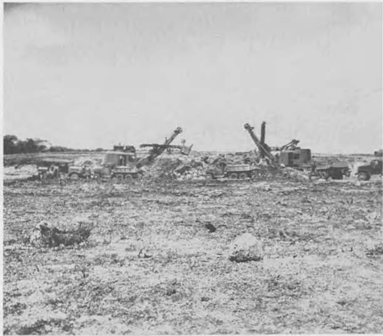
A 2½ cu. yd. and a 1½ cu. yd. shovel at work in hard coral formation after blasting, N. W. Field.
