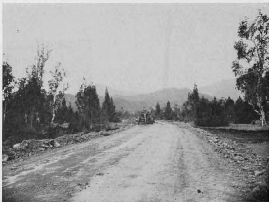
Road construction, Camp Kaiser.
