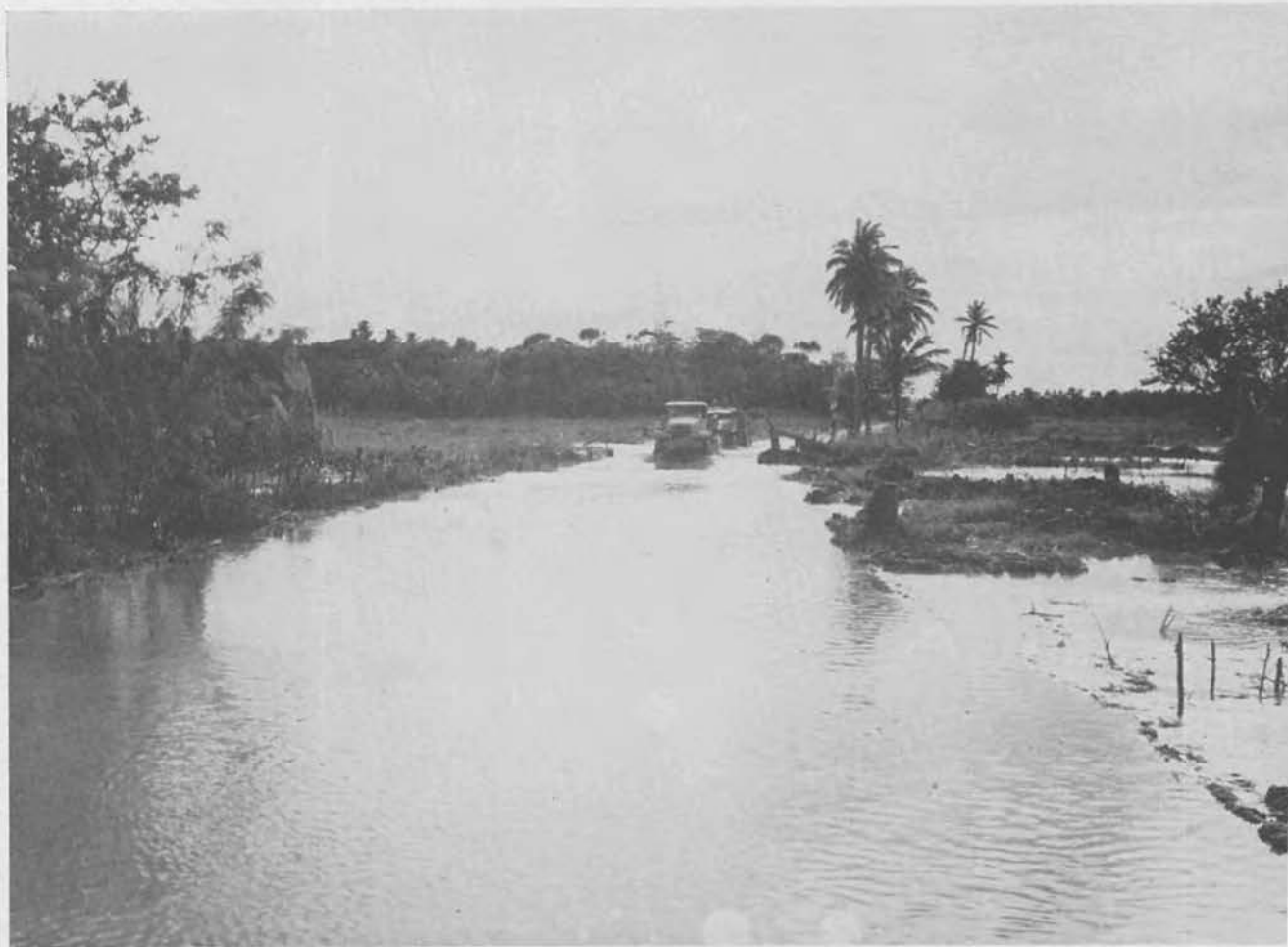
Old Sumay-Piti Road under water near site of present Fleet Laundry.
