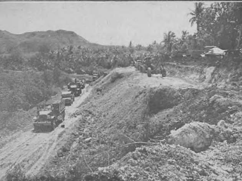
Early construction on the Sumay-Piti road. Note the handling of traffic.
