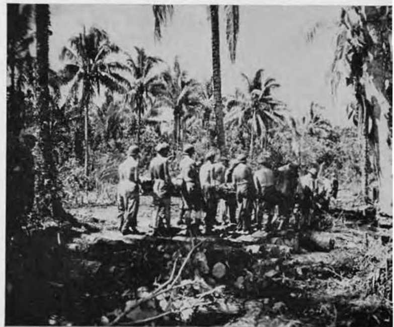
Placing corduroy for roadbed on Piva Trail
