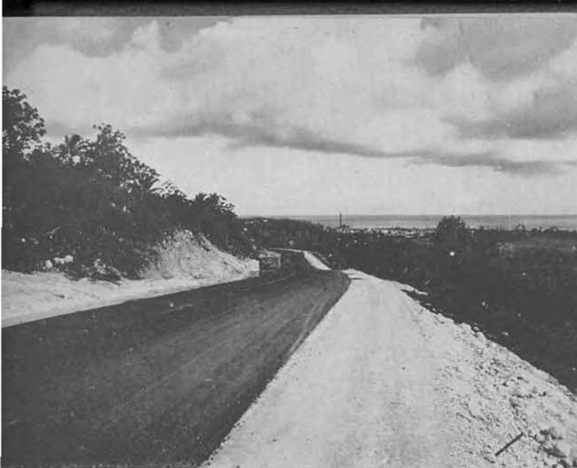
Three-lane pavement on the Cross Island Road above Agana.
