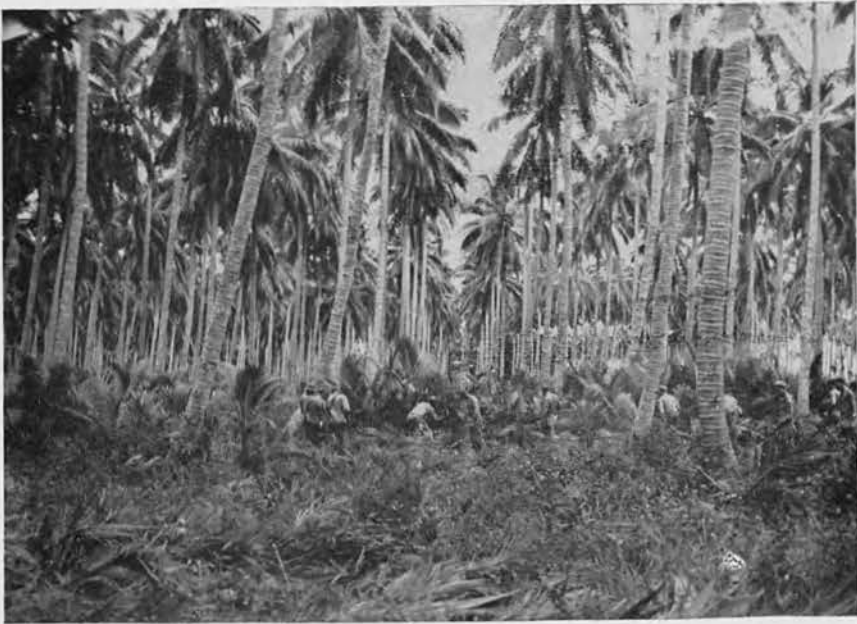
Clearing prior to grading for highway extension.
