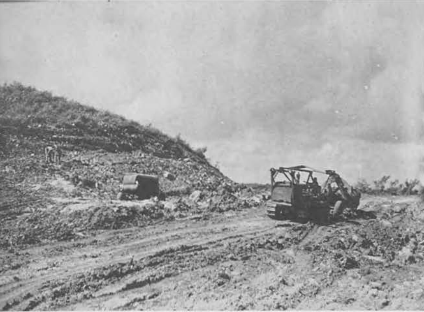
Initial grading operations on the Seawall Cut. approximately 150,000 cu. yds. of excavation was removed.
