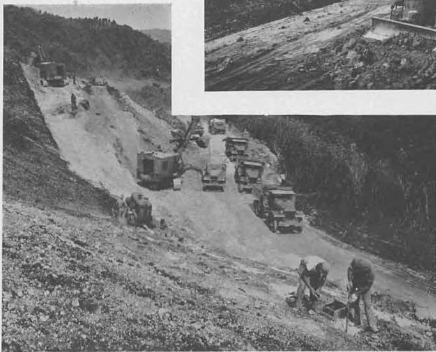
Above: Grading on the entrance road to the AROU Engine Test stands. Agat village is in the background.
