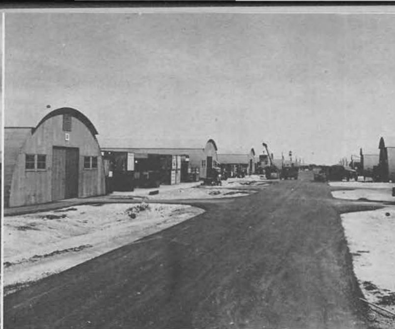
Pavement in ASD Warehouse area.
