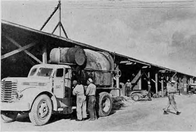
This building housed the various shops—machine shop, paint shop, sheet metal shop, carpenter shop and heavy equipment repair shop. In the foreground is a mixer truck getting a minor repair job outside the heavy equipment repair shop.
