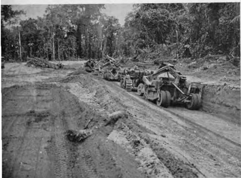
Road construction on Marine Drive.
