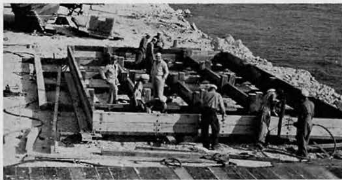
These unloading floats for seaplanes were built under the direction of Ensign Winkler and Chief Neumann of Company A.
