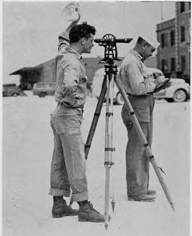
The survey parties were kept busy laying out roads, building sites, etc. J. M. Taft, CM2c is shown at the transit while J. D. Boyle, CM2c records the notes.
