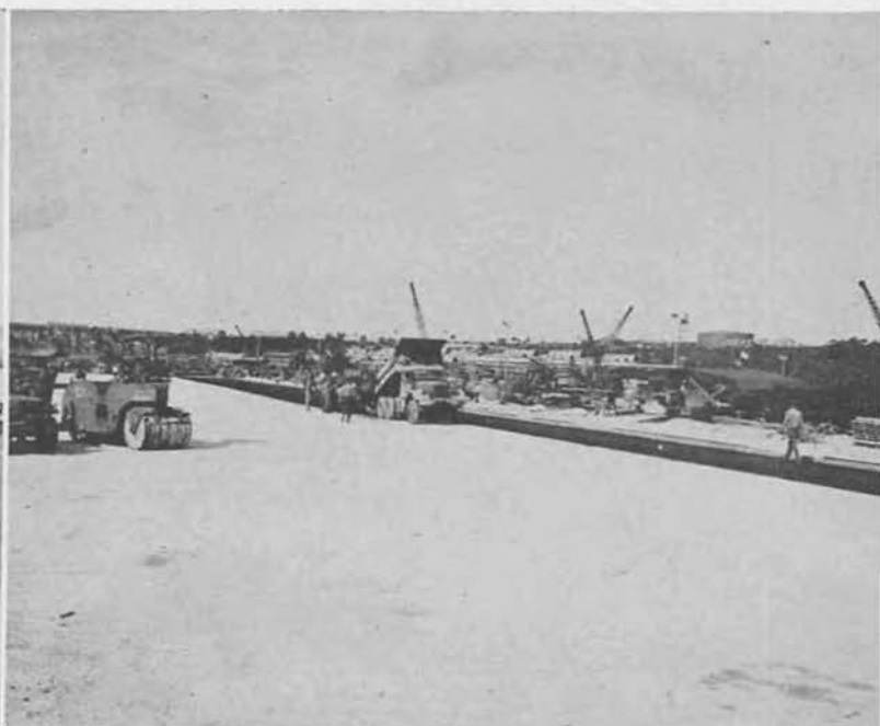
Asphalt pavement deck for Fleet Post Office, Apra Harbor.
