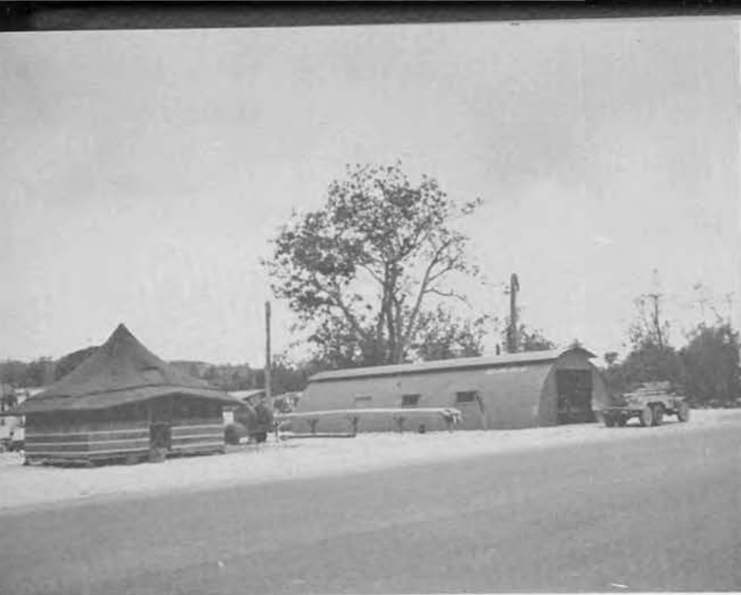
A typical fire station.
