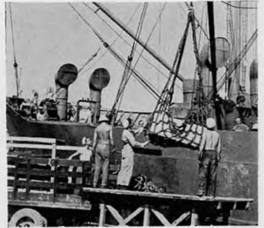
As soon as one truck was loaded and moved away to the warehouse another one moved into position and received its load.
