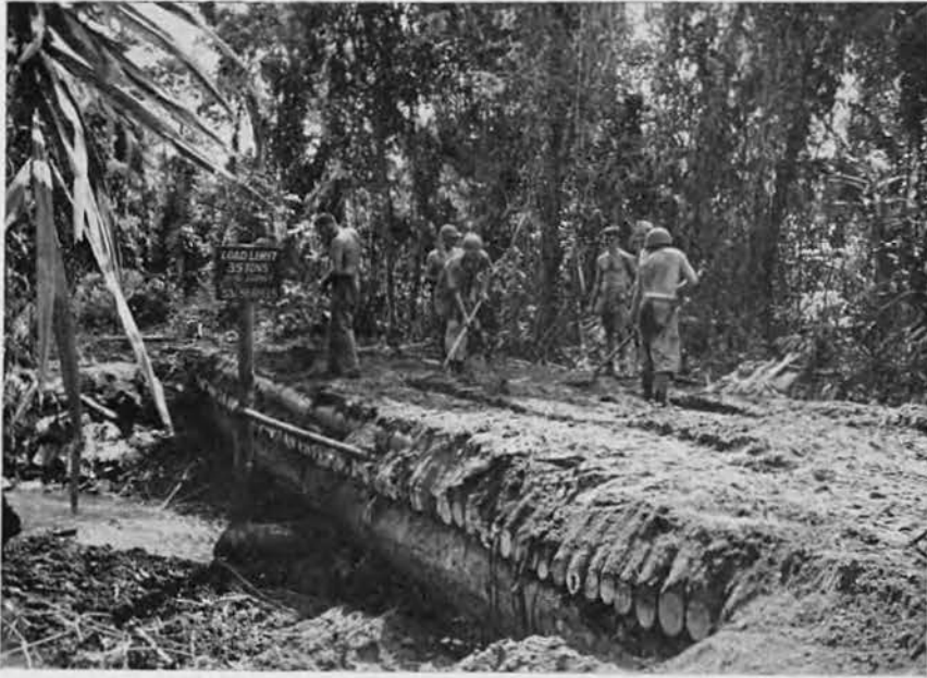
One of the first bridges nearing completion
