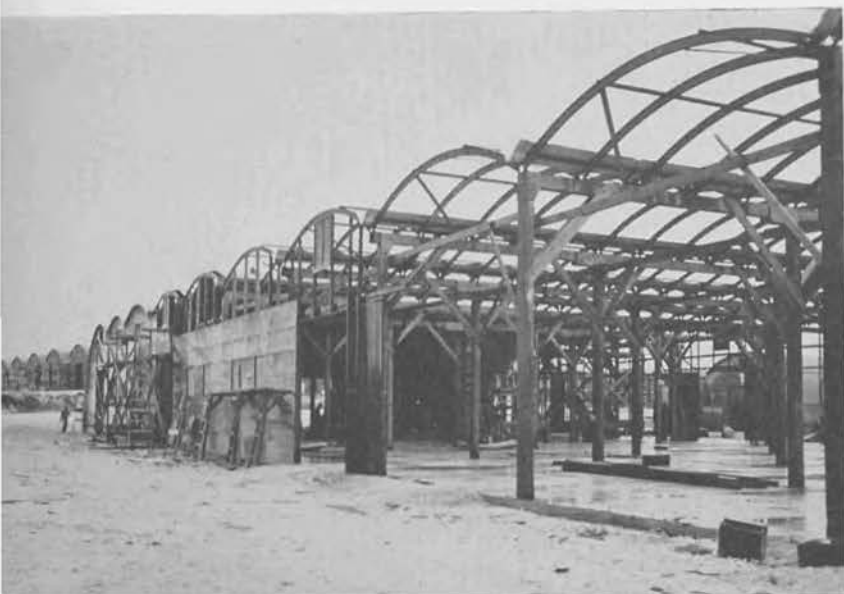
100x400 Mae West type warehouse under construction for SPDC.
