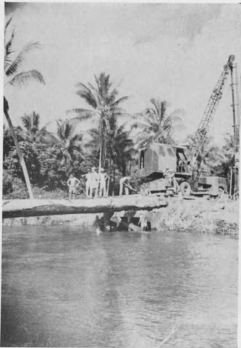
Native timber was used in these two steps of bridge construction.
