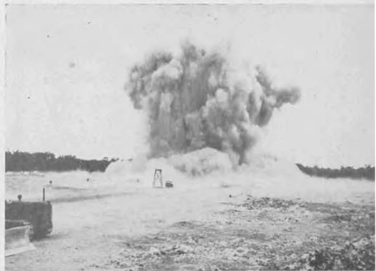
Below: Blasting charge goes off on rock cut N. W. Field.
