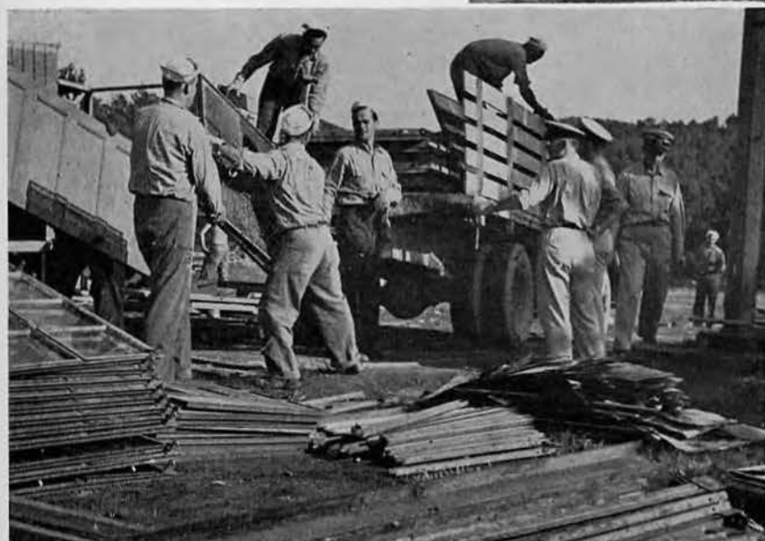
Windows, doors, walls, and all are loaded onto a truck and moved to a new location where they were again assembled into buildings.
