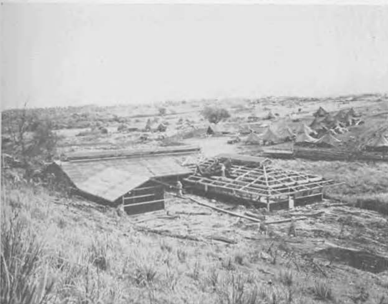
Bakery, Galley, and General Mess under construction.
