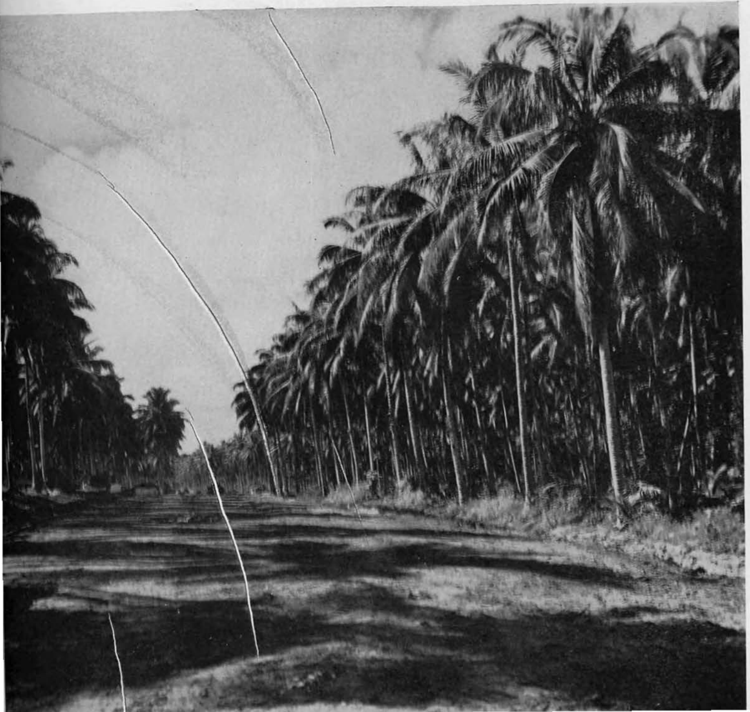
Completed section of road.
