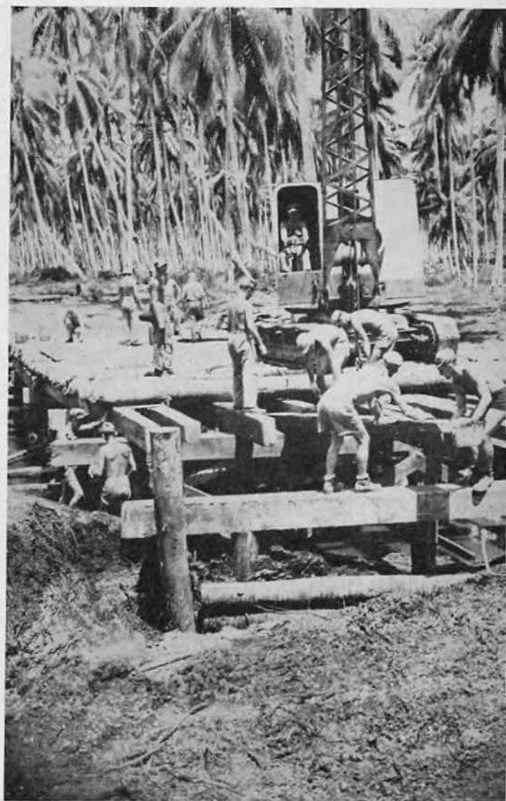
Native timber was used in these two steps of bridge construction.
