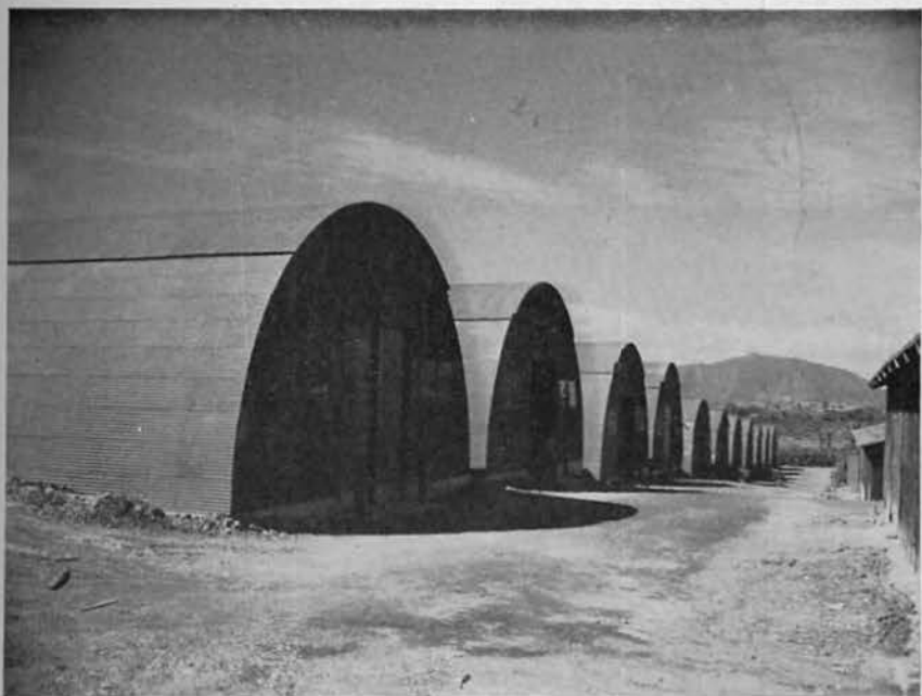
View of completed Quonsets, Engineer Warehouse, 1st Base Depot.
