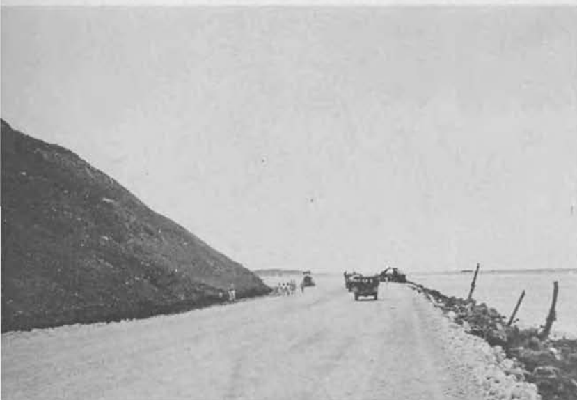
Finishing base course on Seawall Cut.
