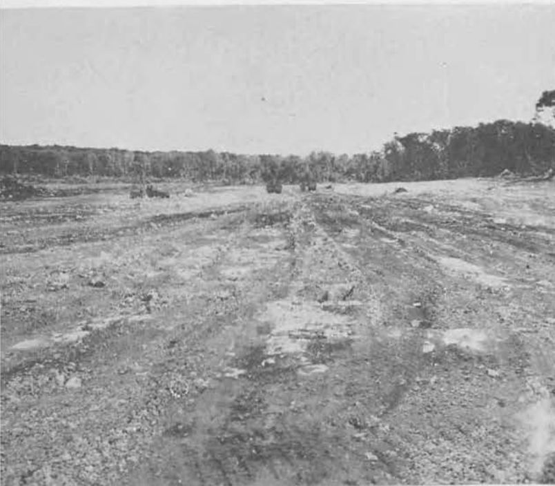
Preliminary grading with pans at N. W. Field.
