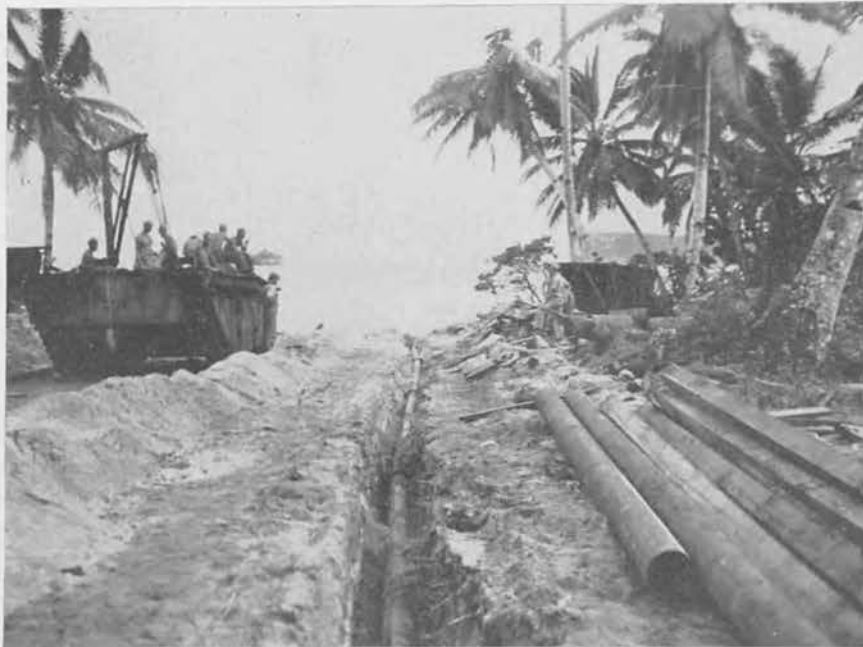
Installation of submarine pipe line from tank farm across reef to tanker discharge site. Approximately 1,500 lineal feet of pipe line lay on the reef.
