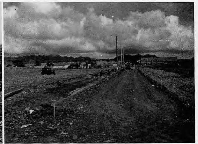
Access roads begin to criss-cross the area.
