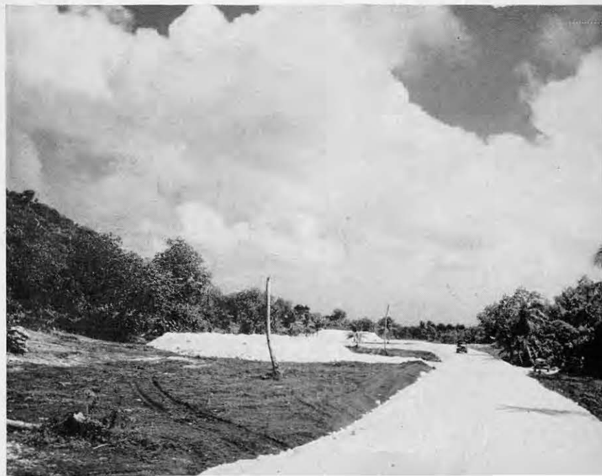
Below are two good examples of coral roads that were surfaced out of this pit. The crushed coral was also used in the making of concrete without it being necessary to use sand, and as a filler for macadam, in the building of the many miles of Macadam roads and airfield runways on the island.
