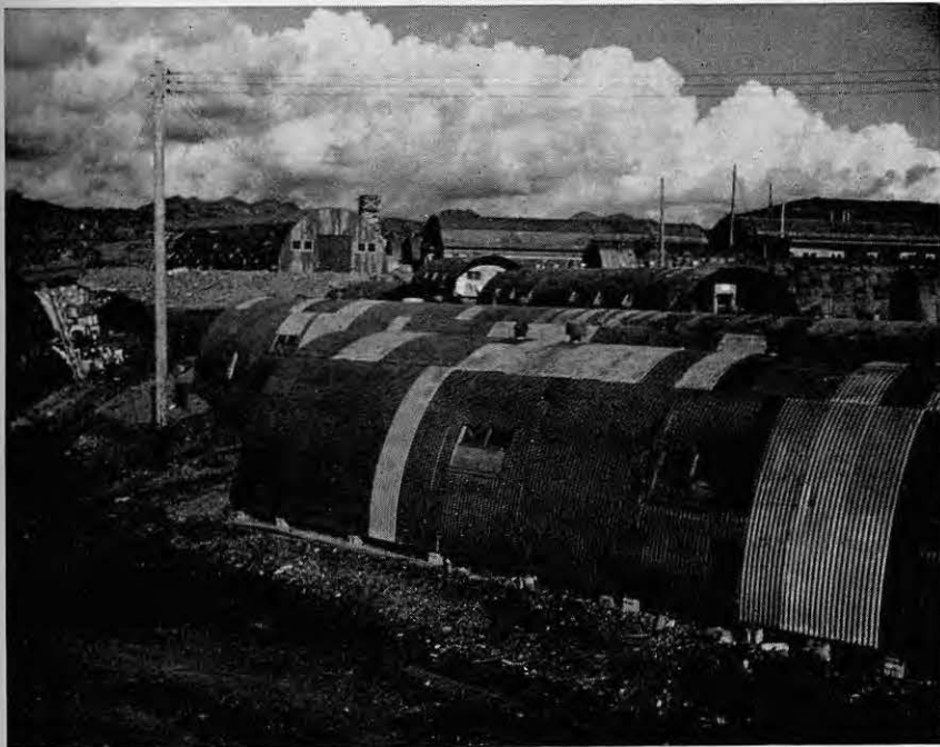
A completed section of our own area at the ridge.
