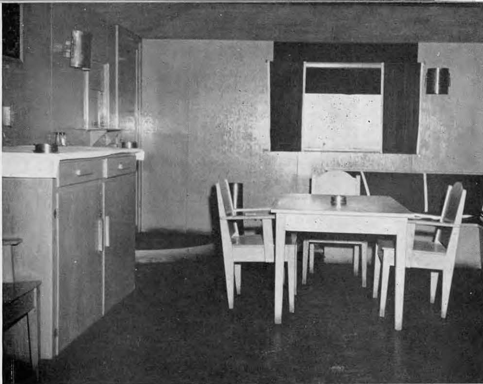
The Commander's dining room, an excellent exhibition of the skill of our finish-carpenters.
