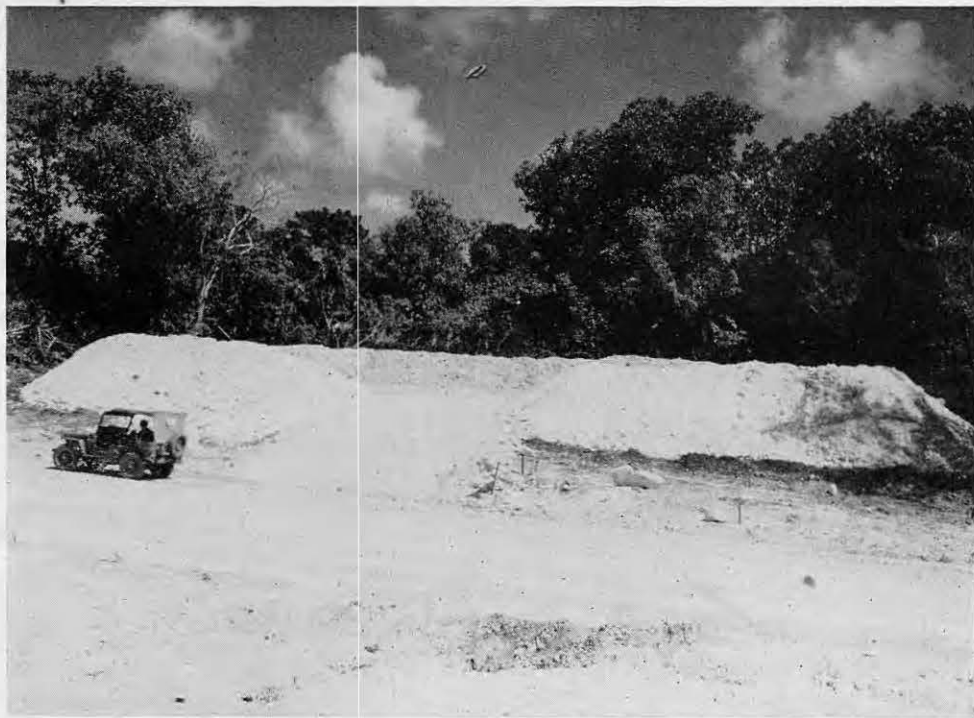
The revetments we prepared at N. A. D. for bomb storage.
