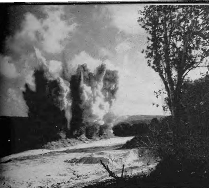
This is what four tons of powder looks like at the height of the explosion beginning the coral pit at N. A. D.
