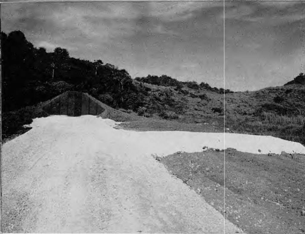
Here is the completed igloo, loaded with bad news for the Japs and covered with dirt to make it blend with the surrounding country.
