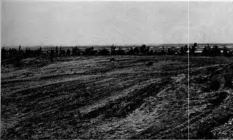
In a couple of weeks, the entire area looked like this—ready for grading and building.
