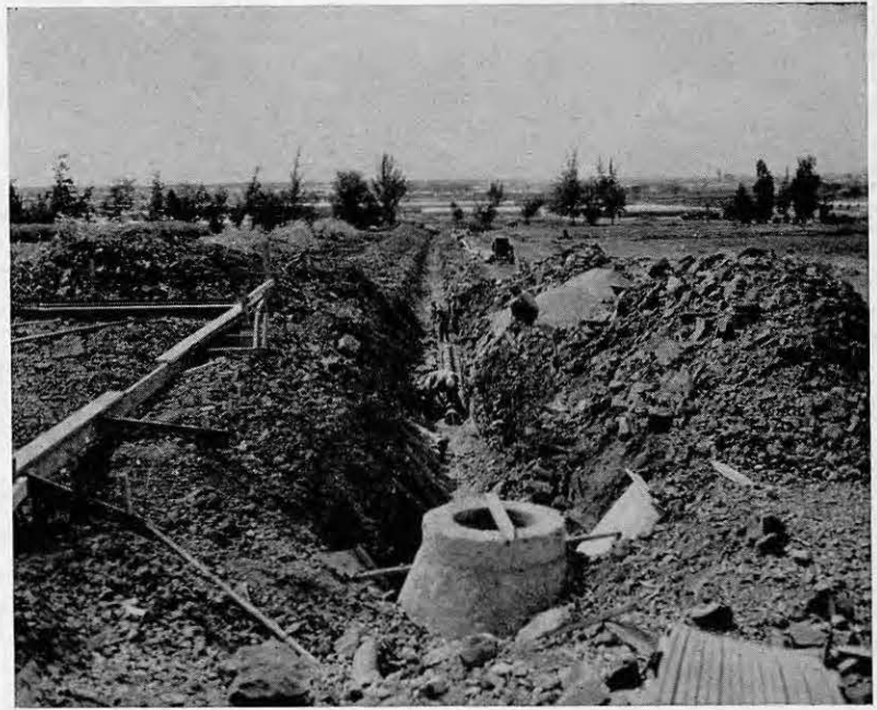
Putting in those concrete pipe sewer lines was rugged duty.
