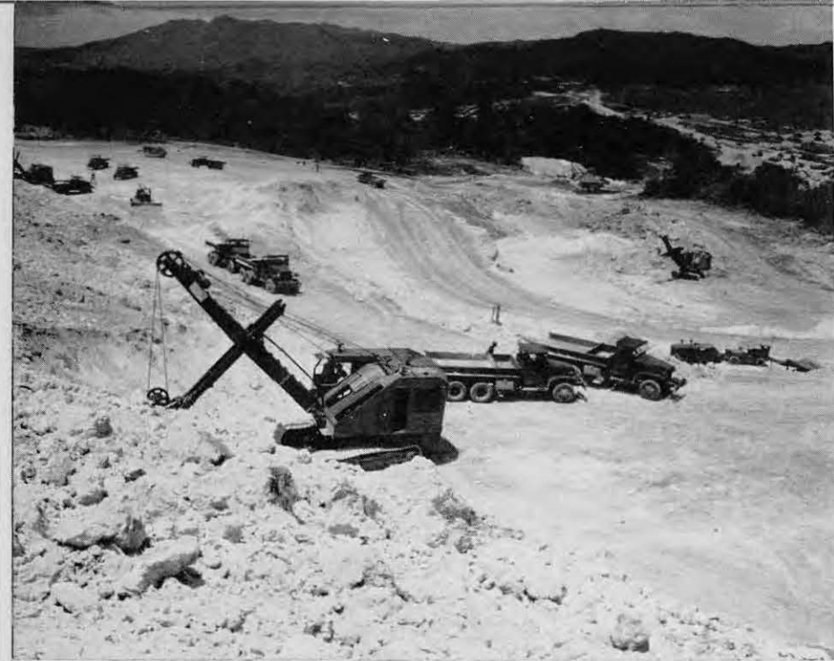
The existence of huge coral deposits on Guam provided us with an inexhaustible supply of road building material right on the job. Upper left shows our N. A. D. coral pit being worked and at the right is the coral crusher which made little ones out of the big ones.
