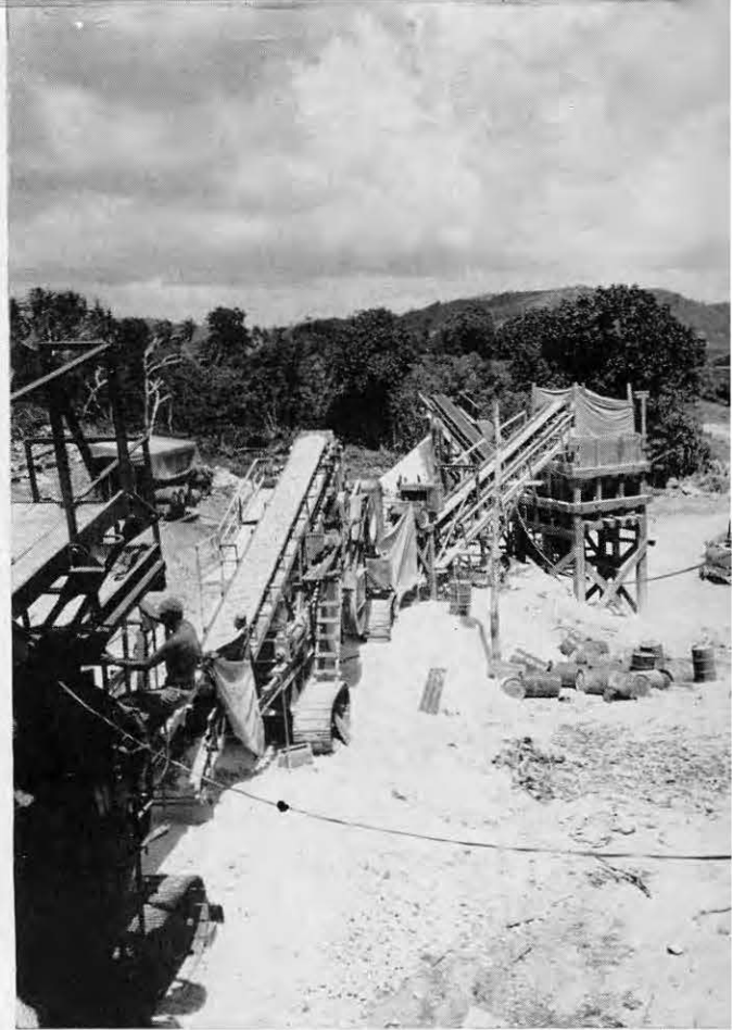
The existence of huge coral deposits on Guam provided us with an inexhaustible supply of road building material right on the job. Upper left shows our N. A. D. coral pit being worked and at the right is the coral crusher which made little ones out of the big ones.
