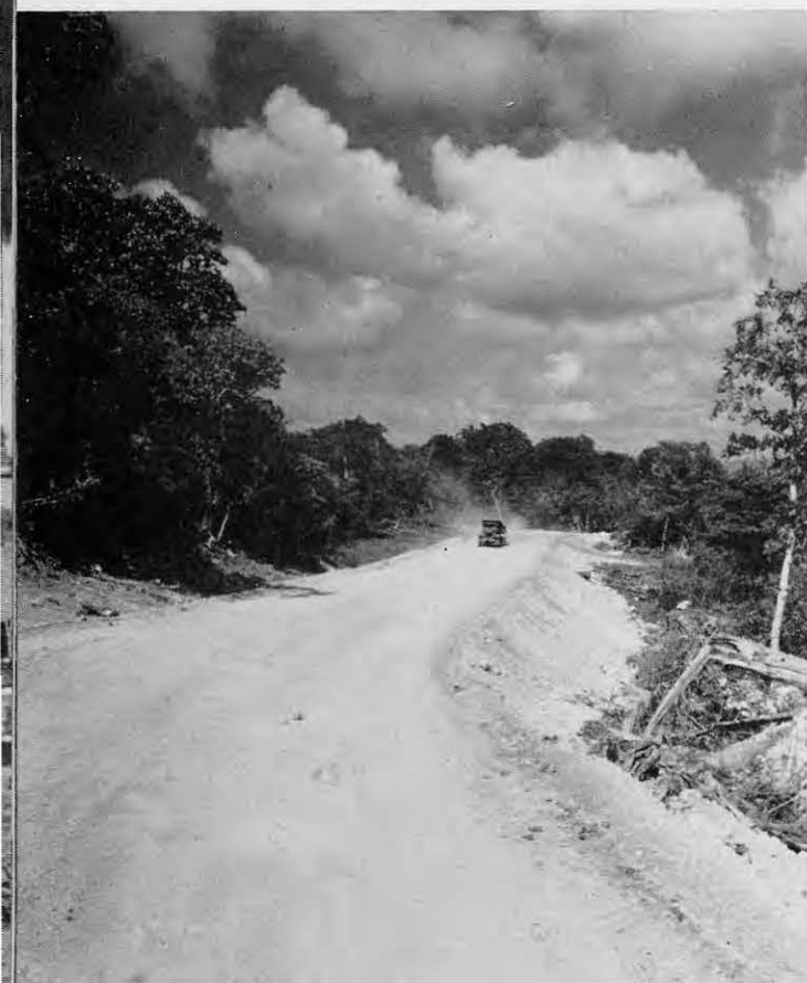
Below are two good examples of coral roads that were surfaced out of this pit. The crushed coral was also used in the making of concrete without it being necessary to use sand, and as a filler for macadam, in the building of the many miles of Macadam roads and airfield runways on the island.
