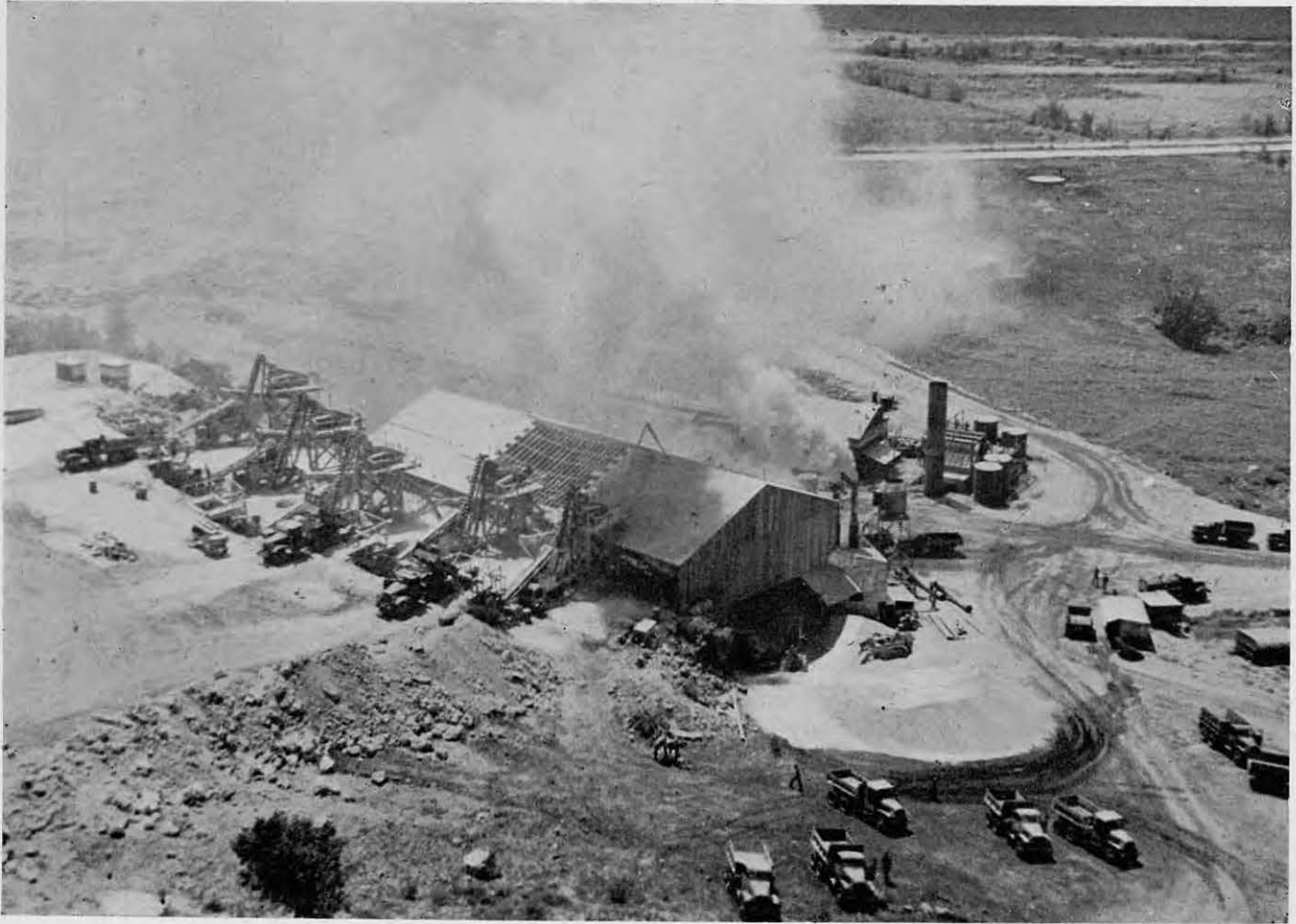
NORTH CRUSHER AND ASPHALT PLANT
