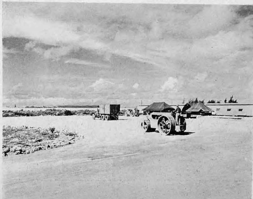
HIGH DENSITY COMPACTION
