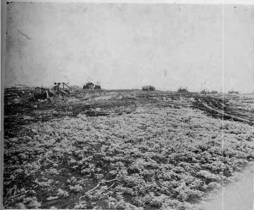
GRUBBING PRIOR TO EARTHWORK
