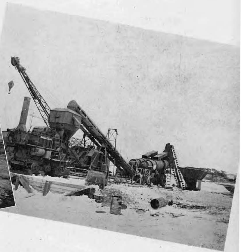
CONSTRUCTION OF STILL ANOTHER ASPHALT PLANT
