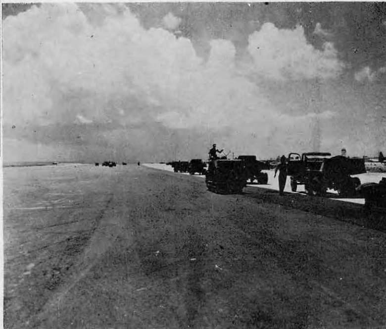
FINAL ASPHALT SURFACE
