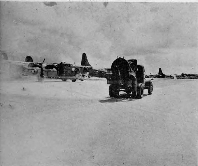
SURFACE CLEANING PROCESS PRIOR TO ASPHALTING
