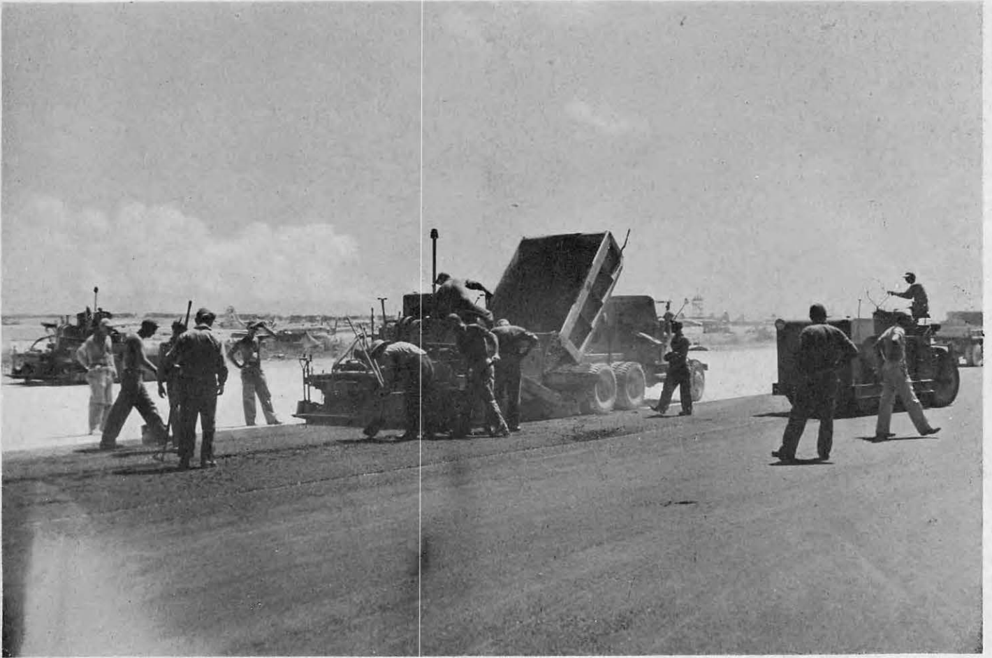
FINAL SURFACE—2 INCH ASPHALT MAT
