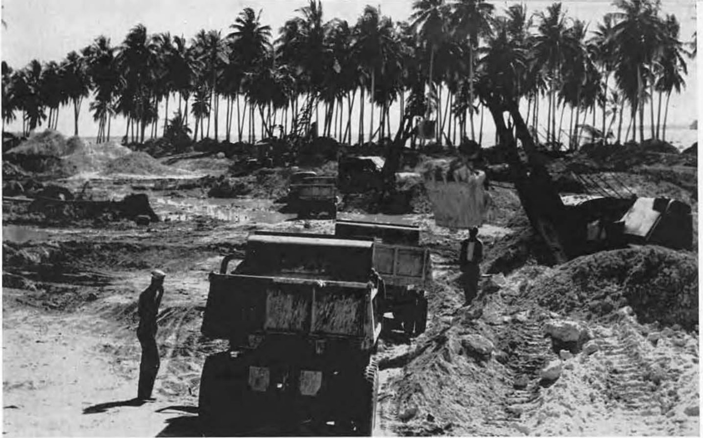
This is the Bougainville airstrip, in preparation.
