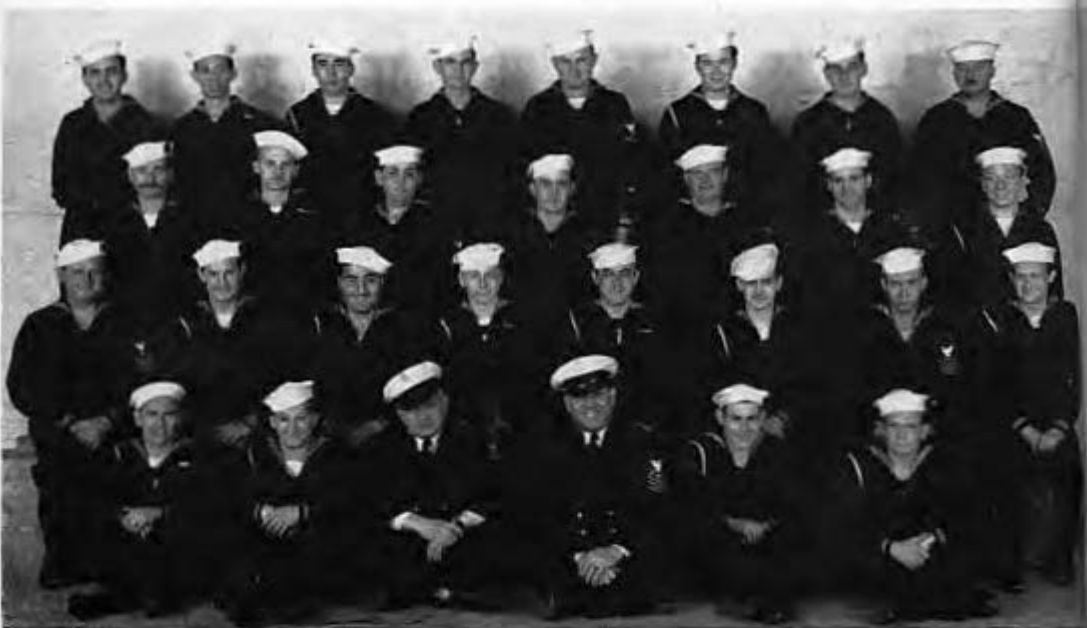
"B" Company, Platoon 5, of the 138th Naval Construction Battalion (Maintenance)
