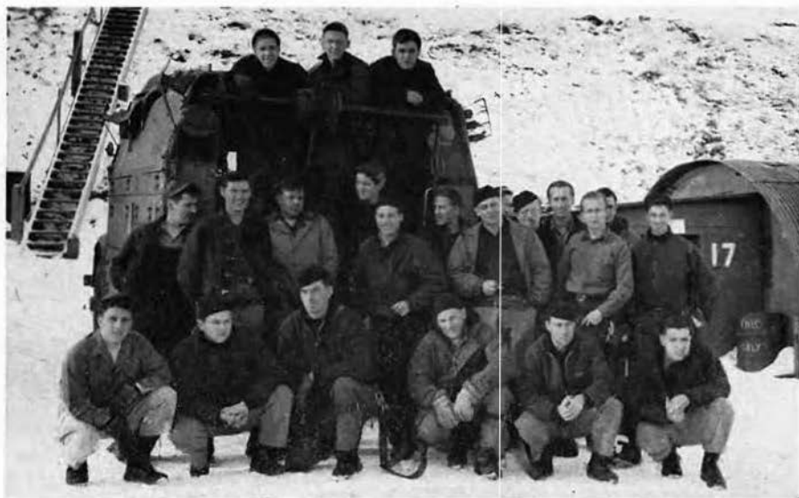
ELECTRICITY for lights, power and communications was a "must" or our base didn't function . . . it was up to our crews to keep utilities operating and they did it regardless of hours or weather.
