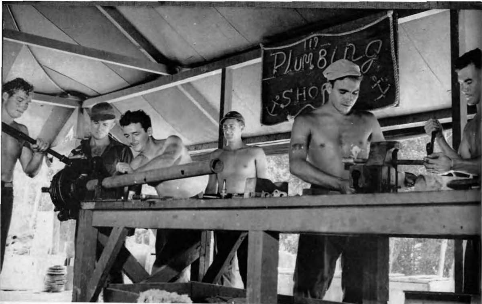
Threading pipe and making fittings before going out to major project.
