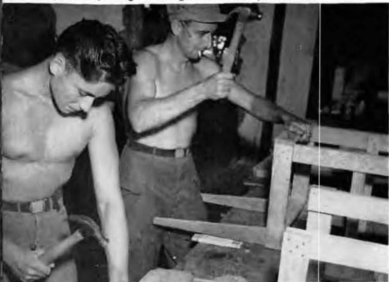
Carpenters putting finishing touches on prefabricated chairs.
