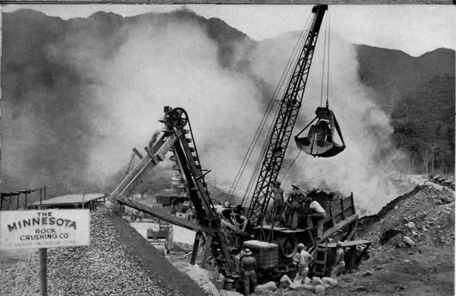
Crushing aggregate to be used in construction.
