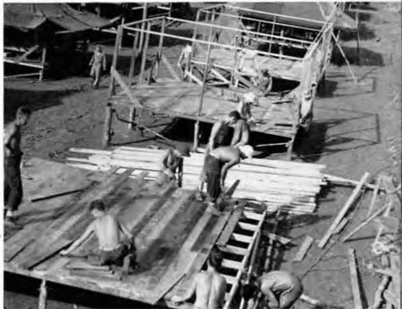
Building the enlisted men's quarters.
