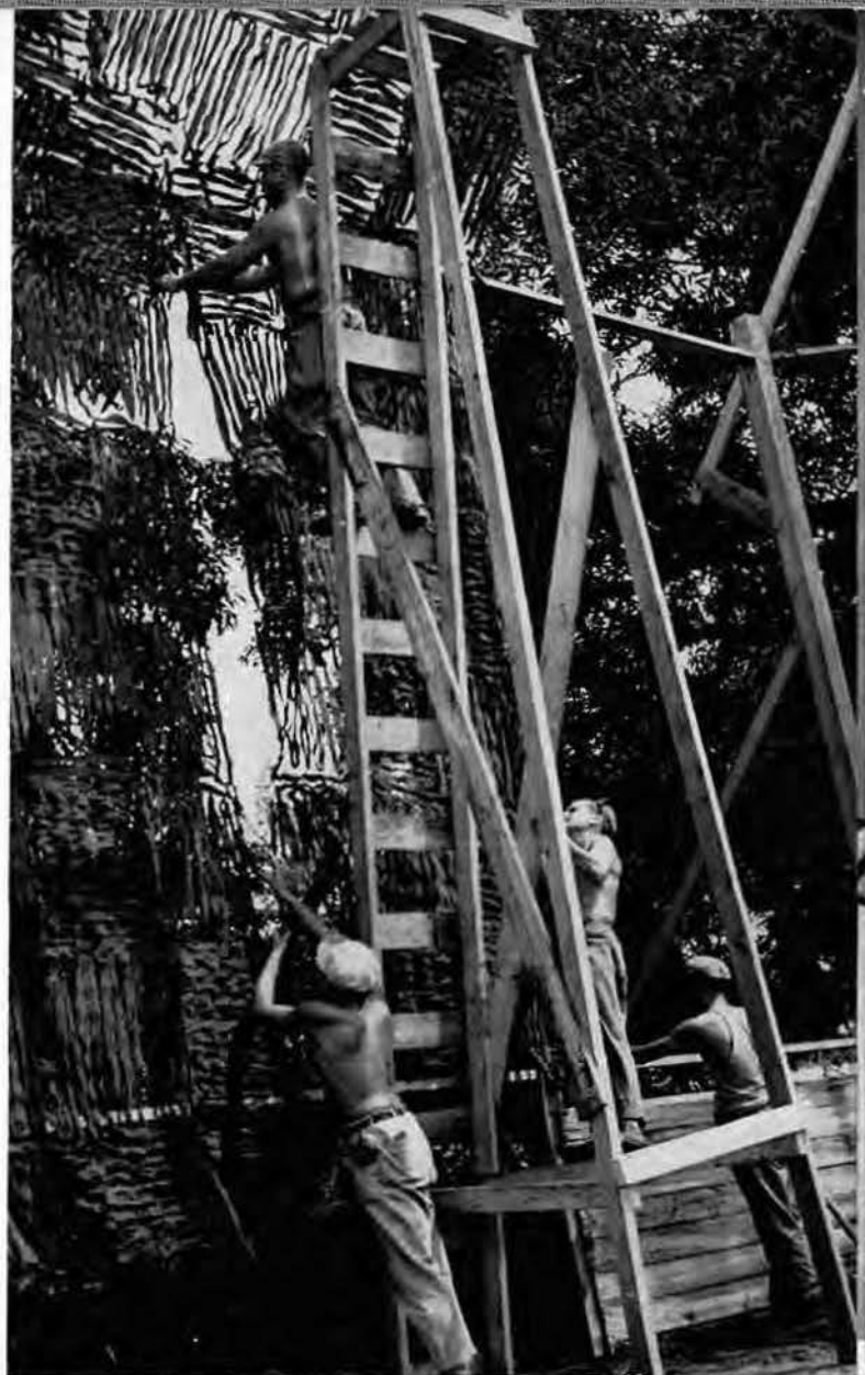
The camp maintenance gang building the back stop at "Mackey Field."
