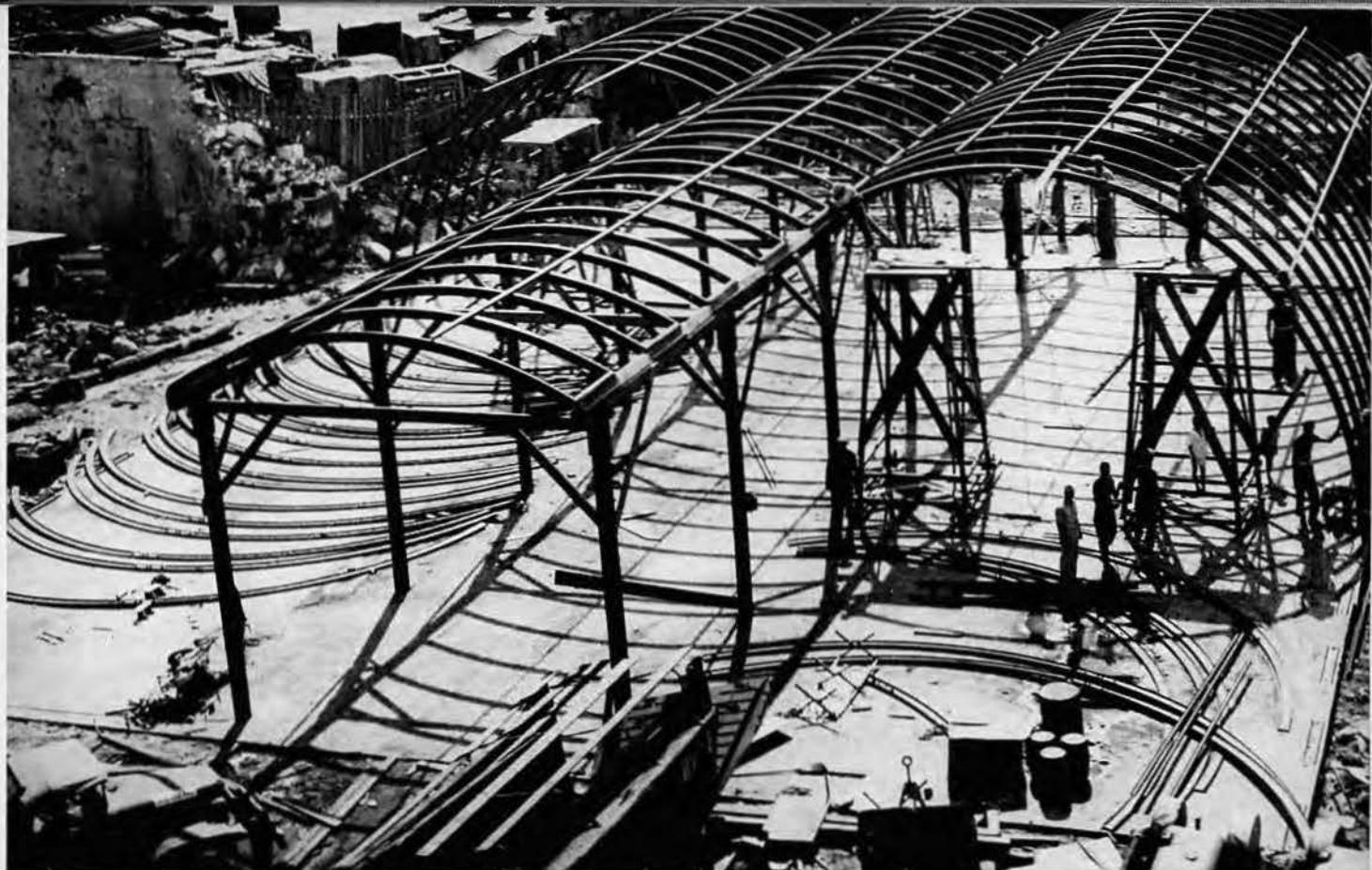
A multiple Quonset Hut warehouse under construction.
