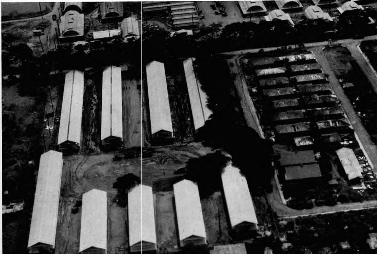
Double deck barracks for housing enlisted men at Philippine Sea Frontier.
