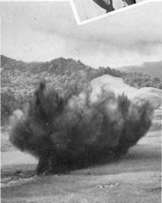
Blasting a ditch for malaria control
