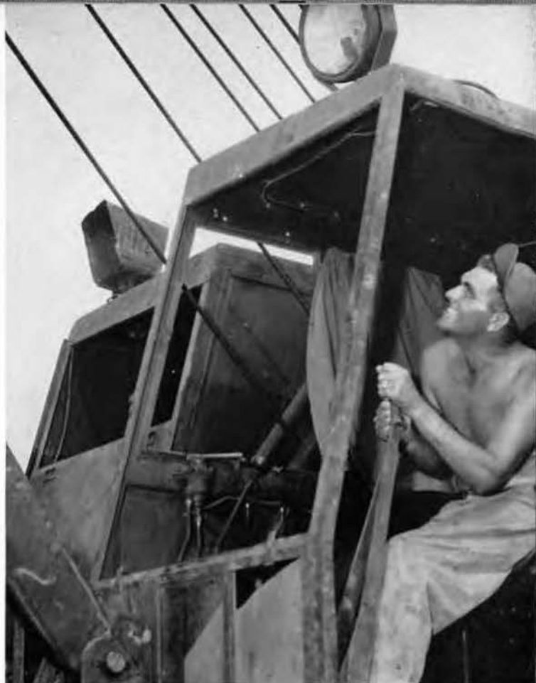
Making a lift and swinging the boom in the 7th Fleet Material Yard.
