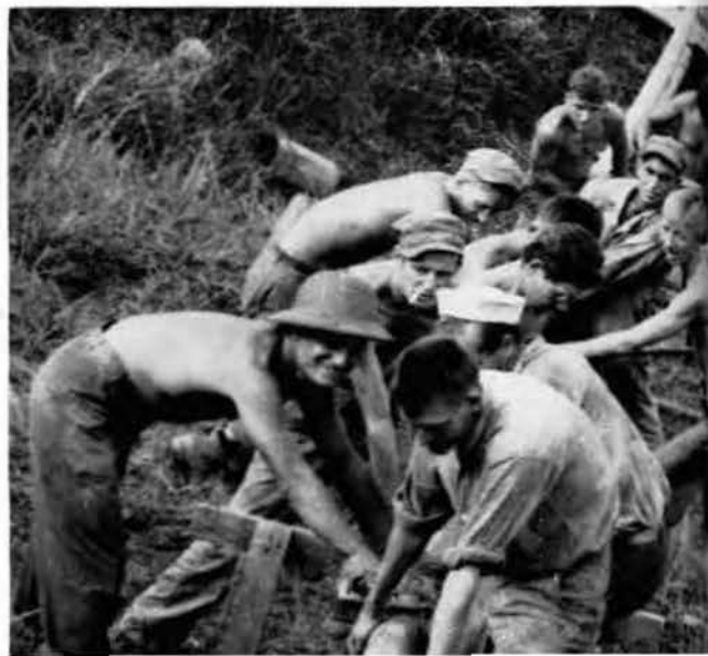
Laying the pipe lines for water.
