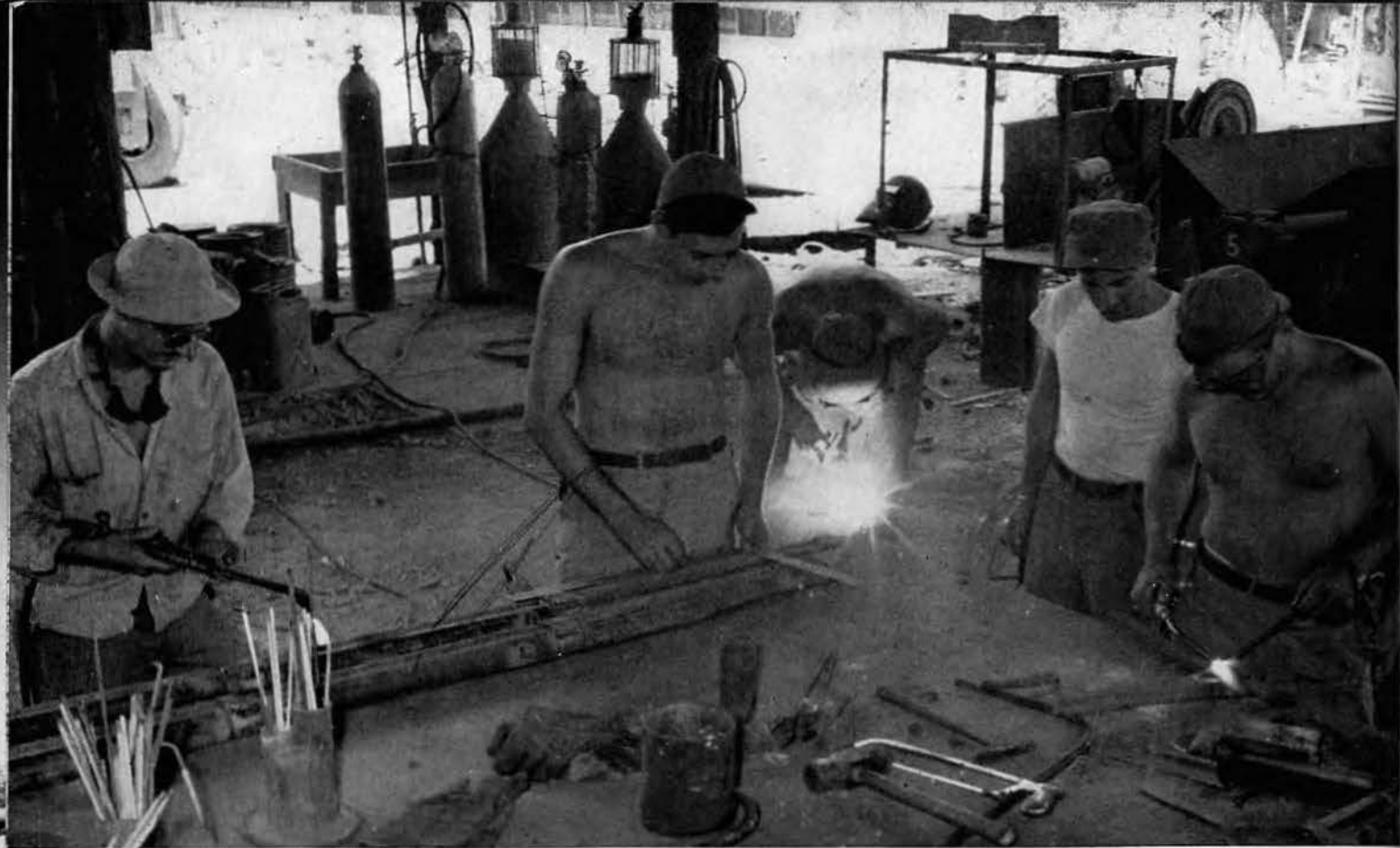
Men in welding shop rush work on shower room fittings.
