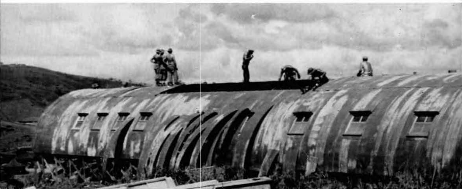
Another hut will soon be completed.
