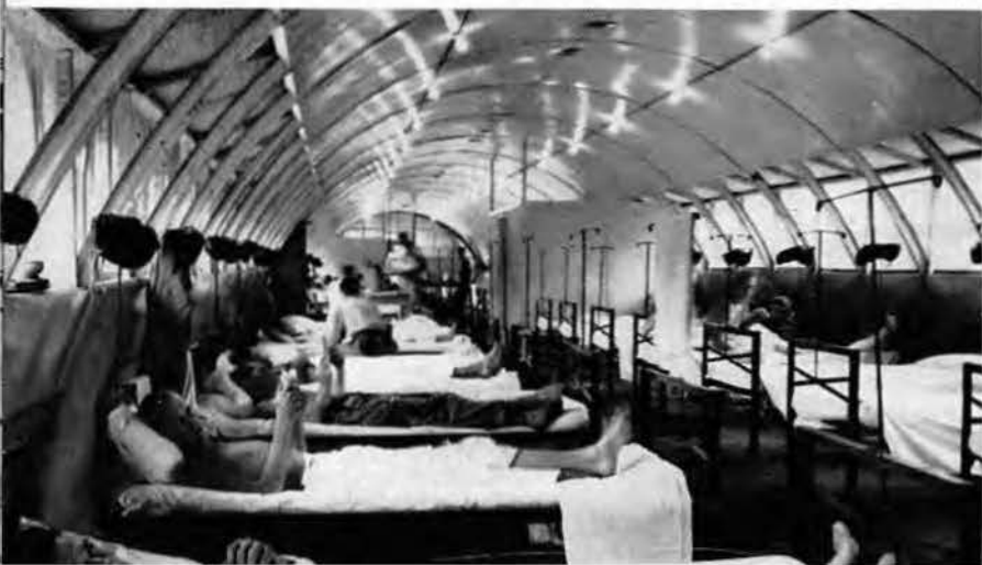
A wardroom in the new hospital addition.
