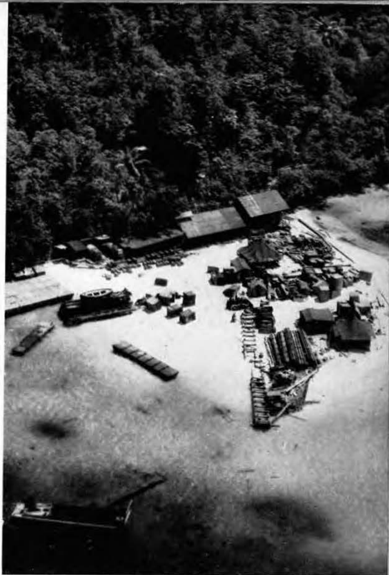
The galley and supply yard at the pontoon assembly site.
