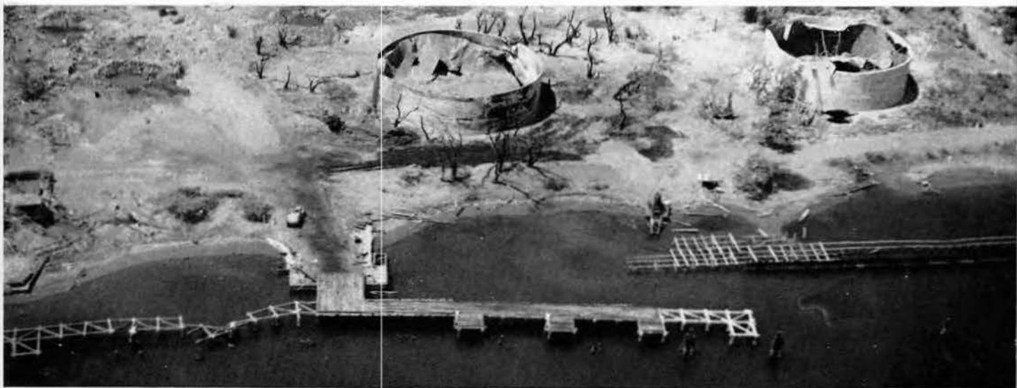
Wrecked docks and fuel tanks at Cavite.
