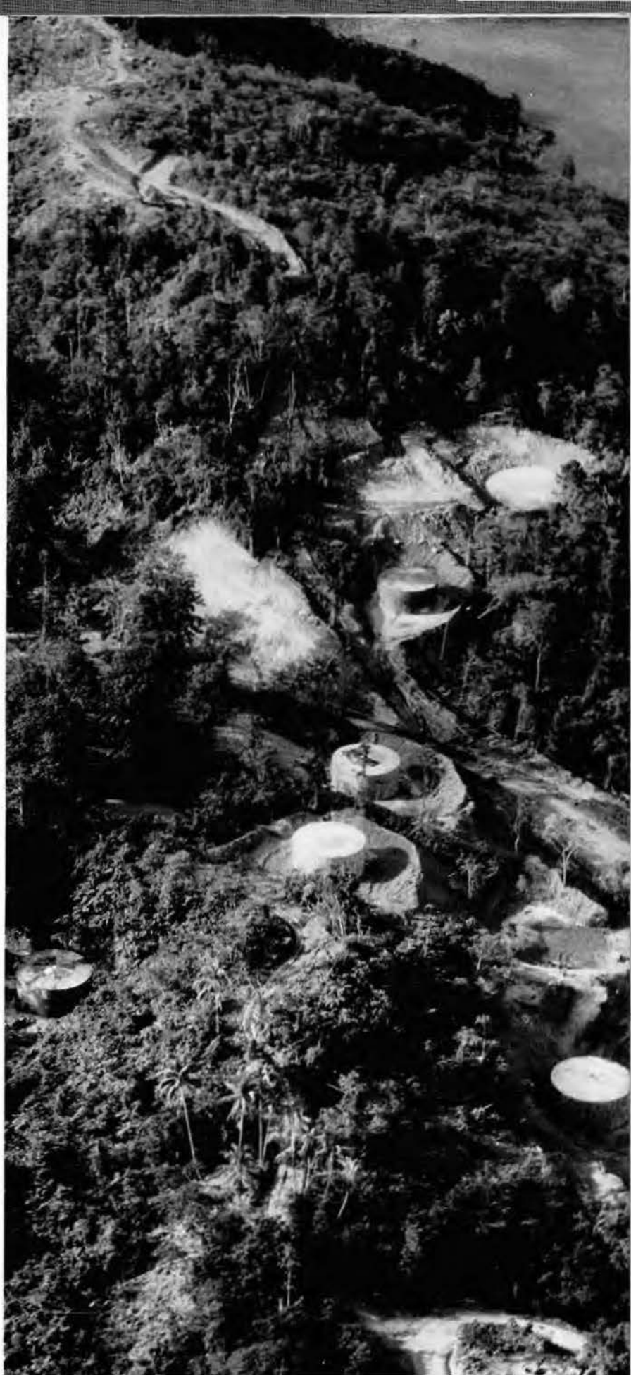
The Tank Farm — at Tanah Merah Bay.
