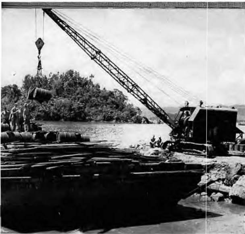
Fuel to run the equipment.
