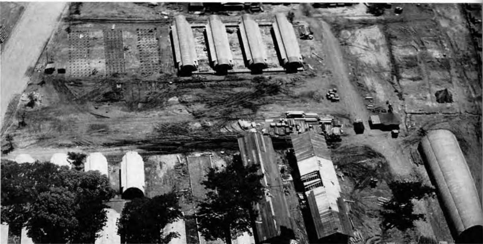
Facilities for Commander Naval Operating Base, Manila-Subic, under construction.
