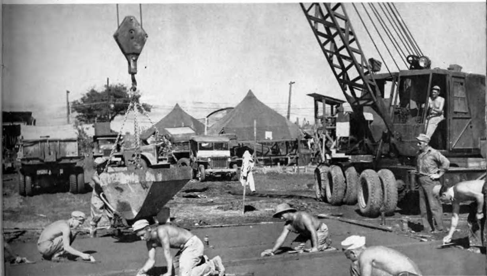
Chief Gier and crew finishing concrete.
