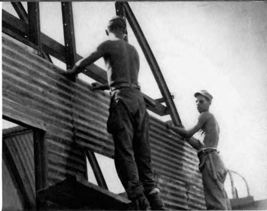
Putting the sheet iron on a large Quonset Hut.
