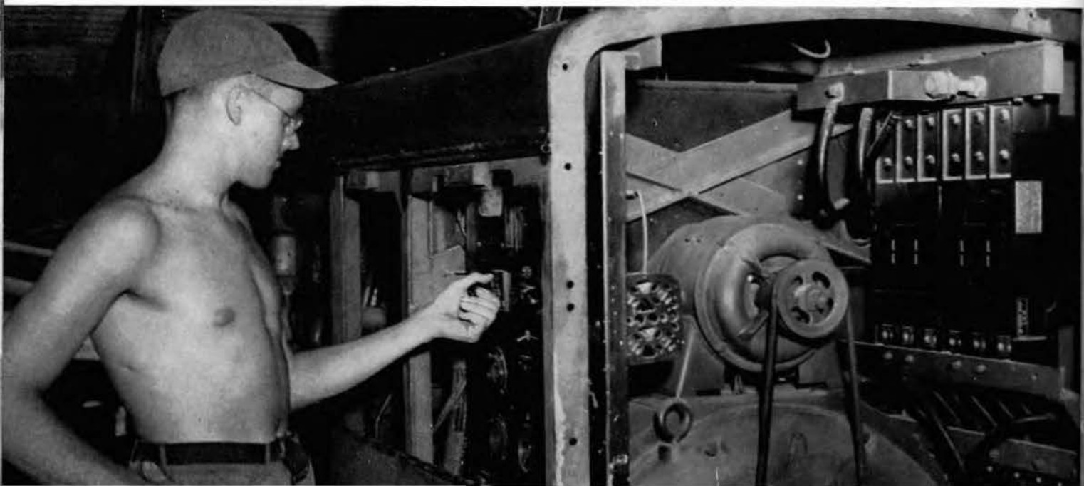
Checking the generators at the 29th Replacement Depot.
