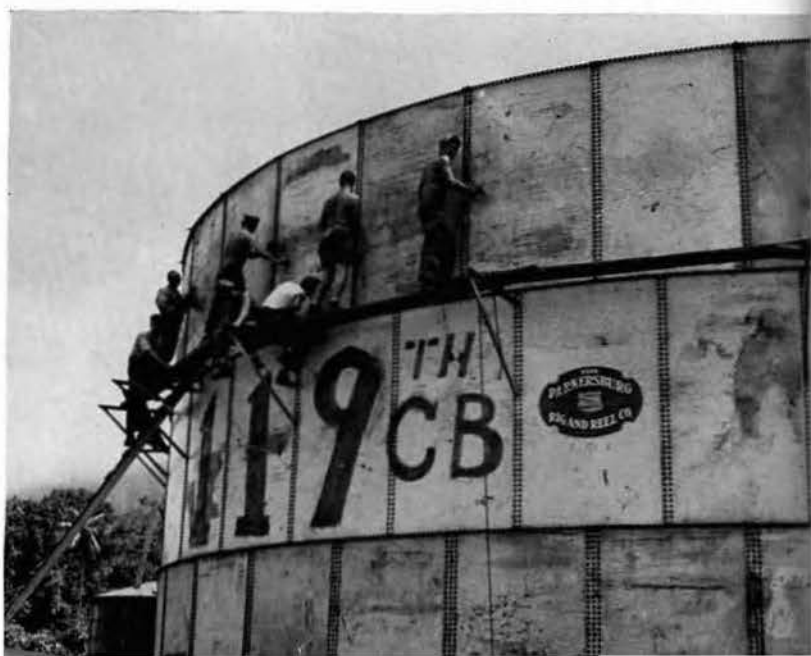
A final check on the bolts.
