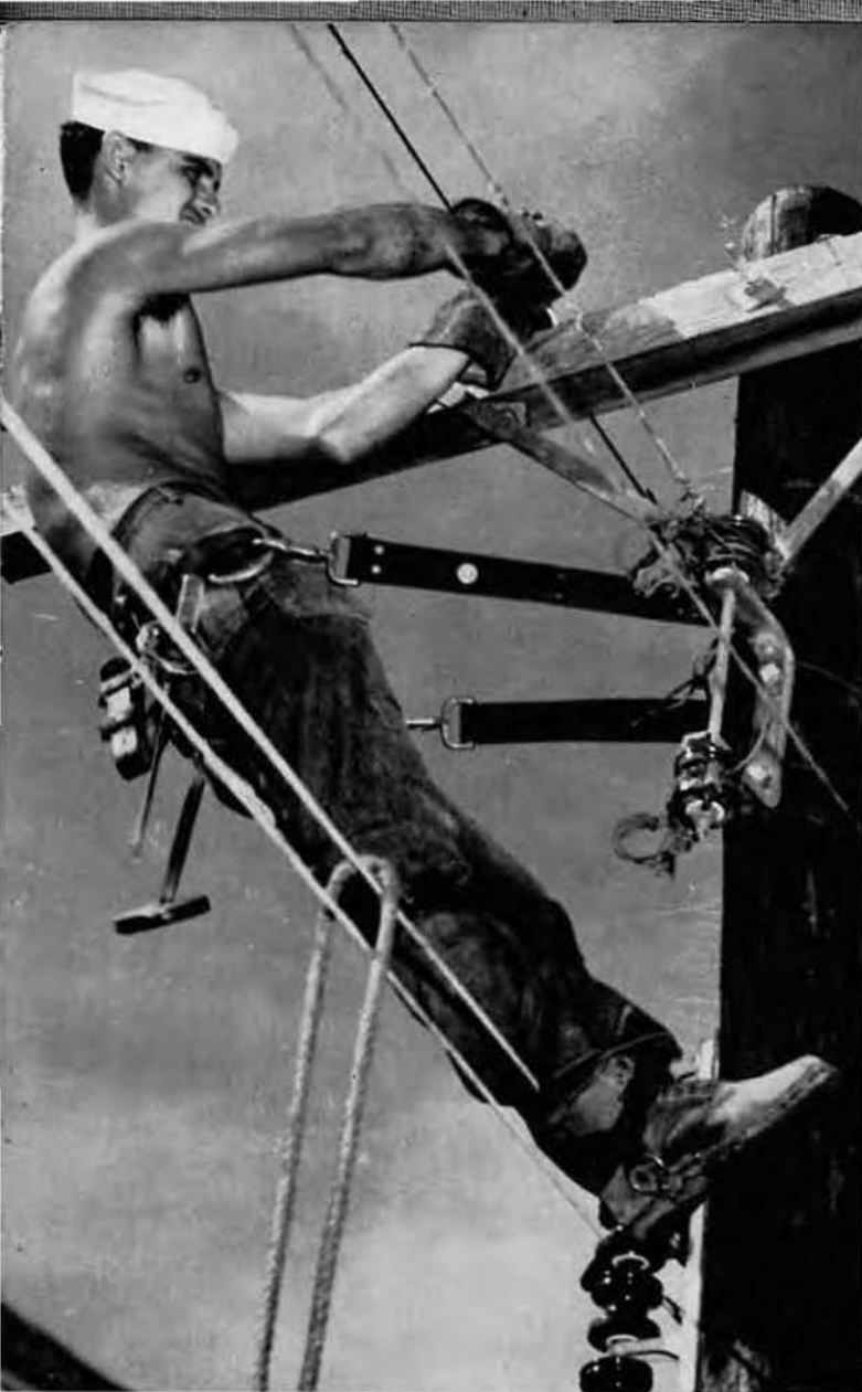
Installing Power and Communications.
