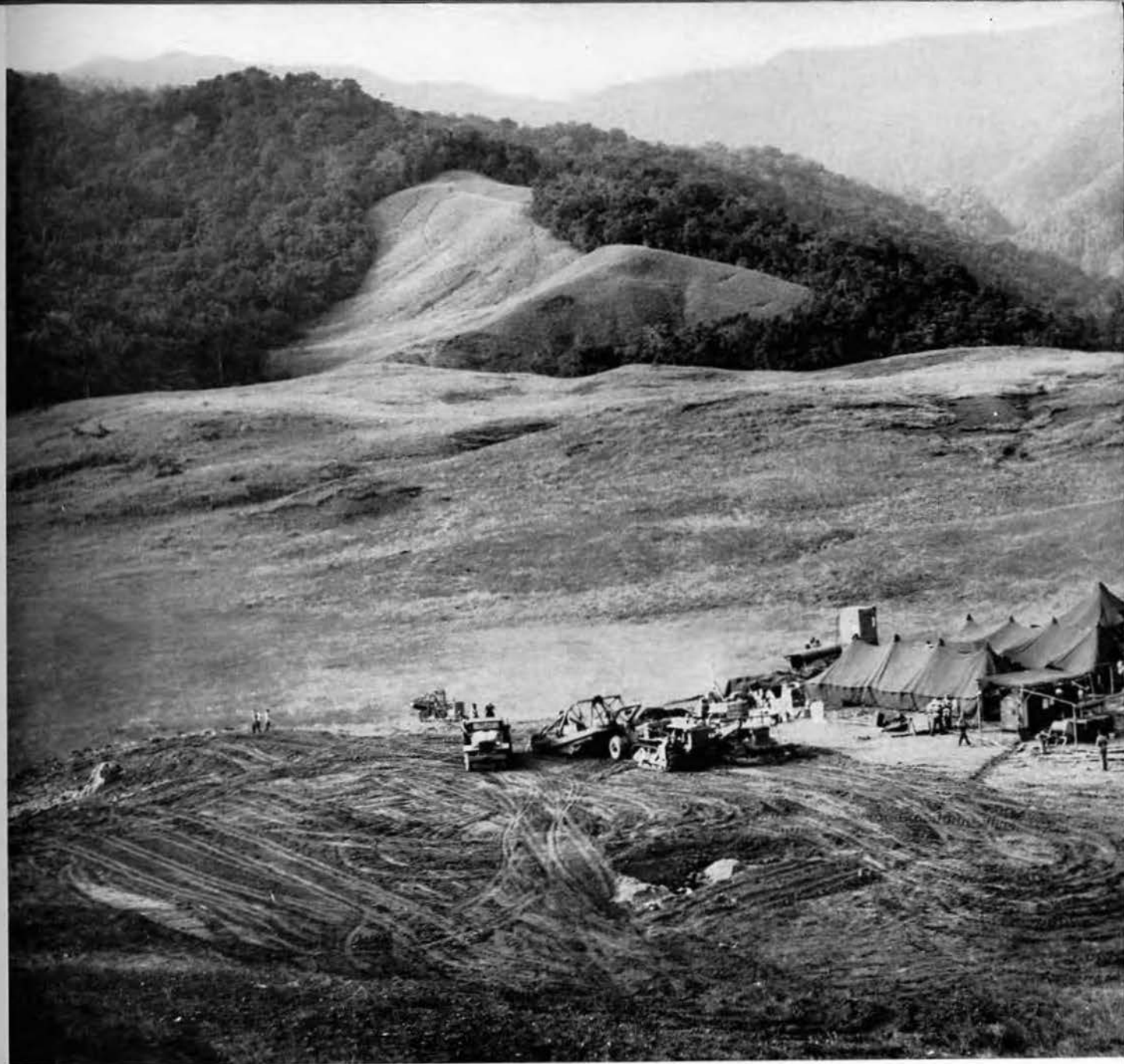
Breaking ground for the Lake Sentani camp.
