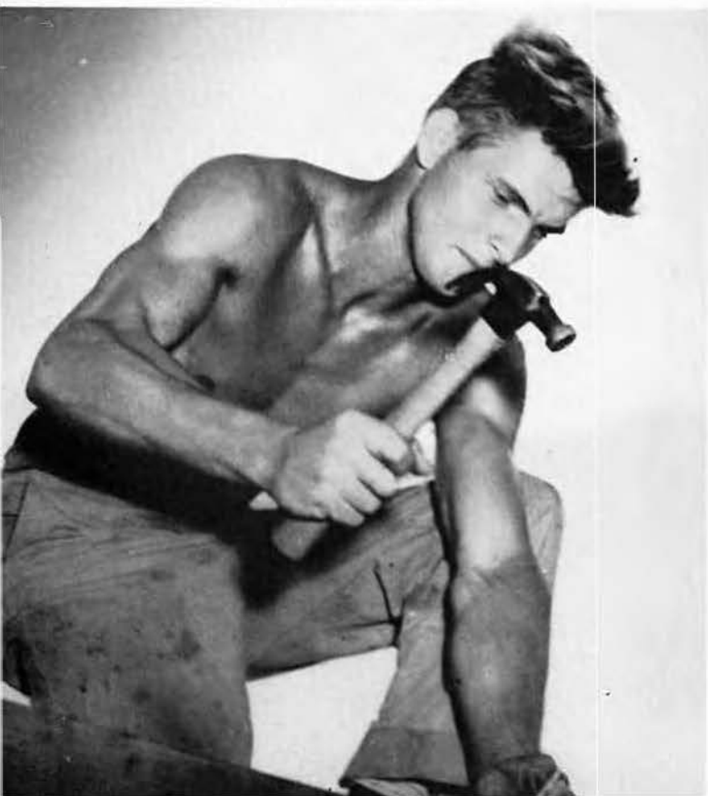
Woodrow Schelvan on construction work.
