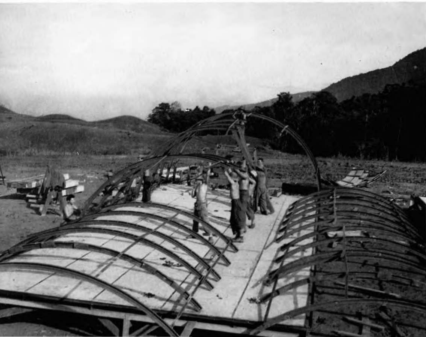
Raising the steel ribs for another Quonset Hut.
