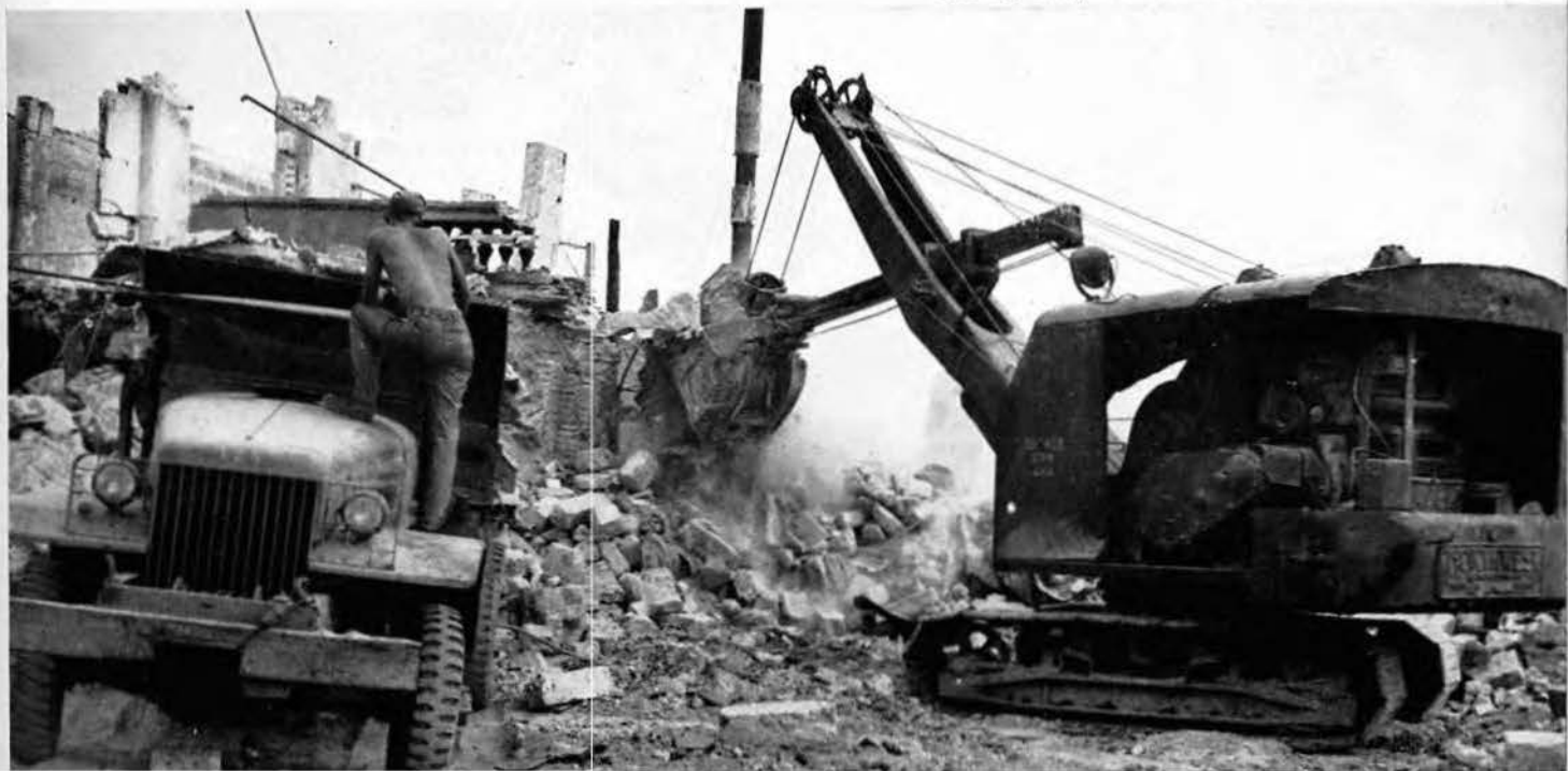
Clearing away the rubble for a construction site.
