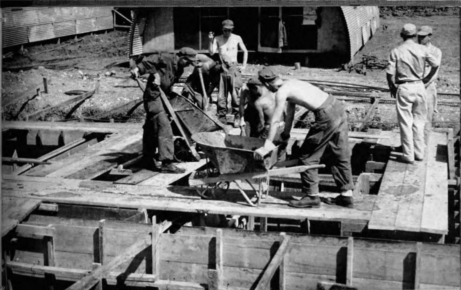
Pouring a concrete Septic Tank.
