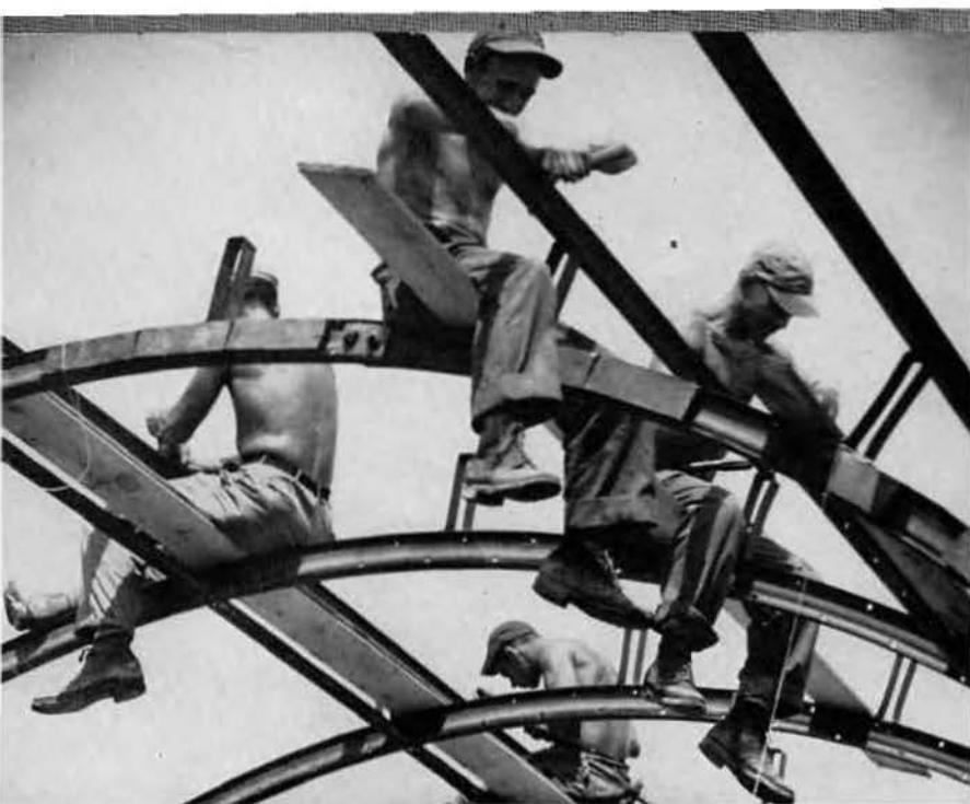
Securing the Purlins on a Quonset Hut.
