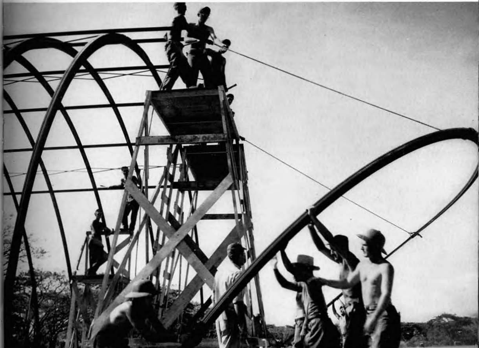
Raising an Arch Rib on a 40' x 100' Quonset Hut.
