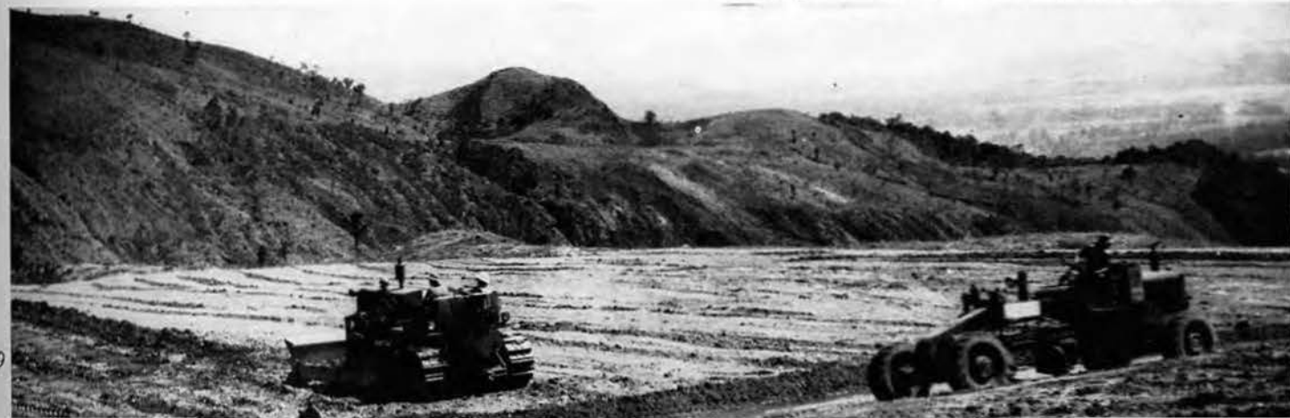
Grading on the Seventh Fleet Headquarters project.
