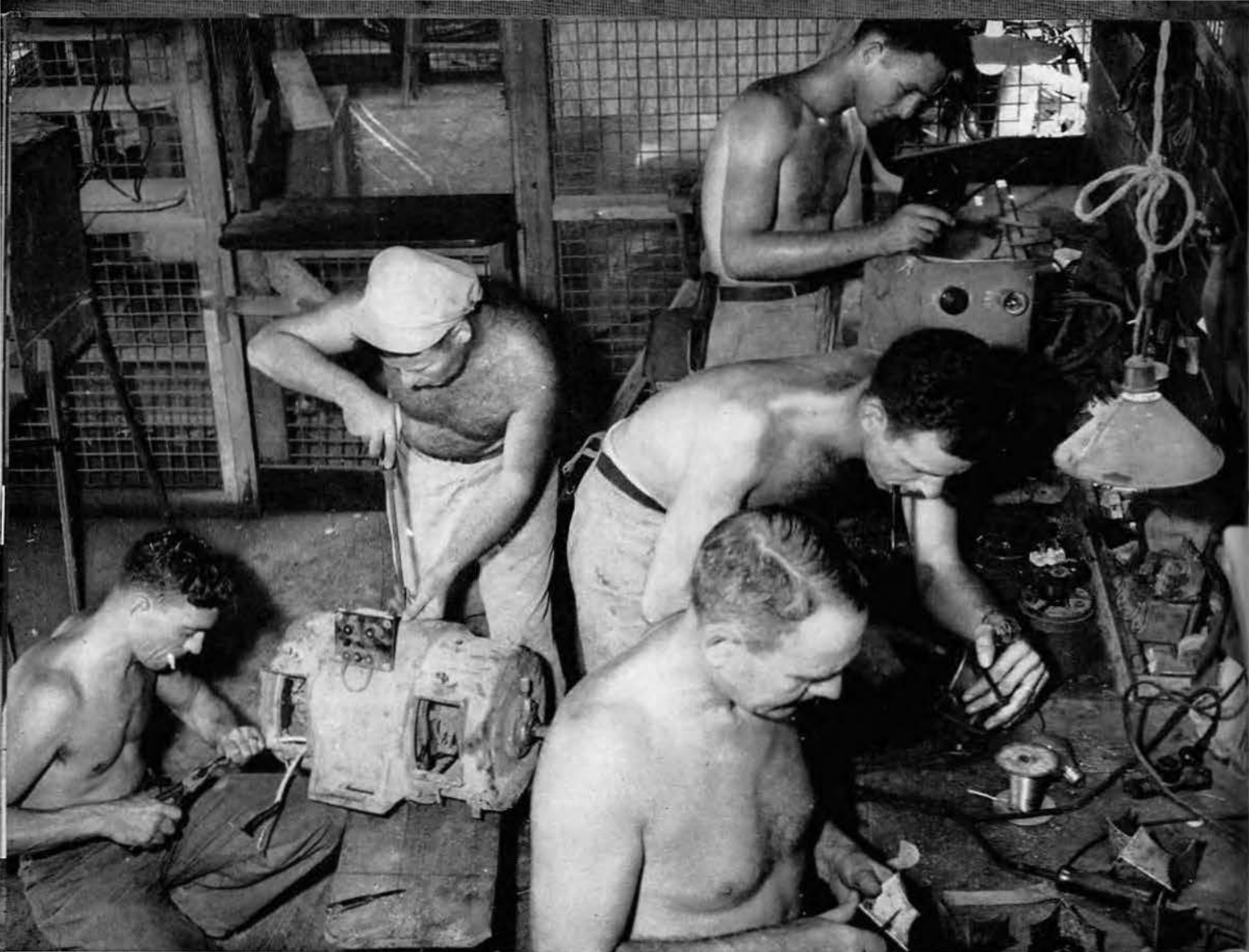
Men in the electrical shop tinker with 101 problems a day.
