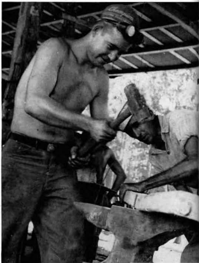
Seabee blacksmiths straighten bent tongue of carryall.
