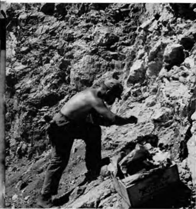
Placing charge for blast. Eugene "Boom Boom" Comtess attaching wires in series to blast loose gravel.
