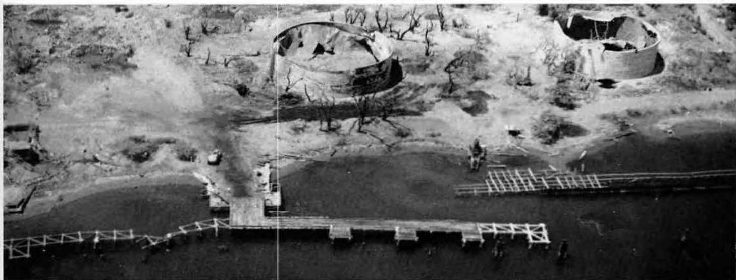
Wrecked docks and fuel tanks at Cavite.
