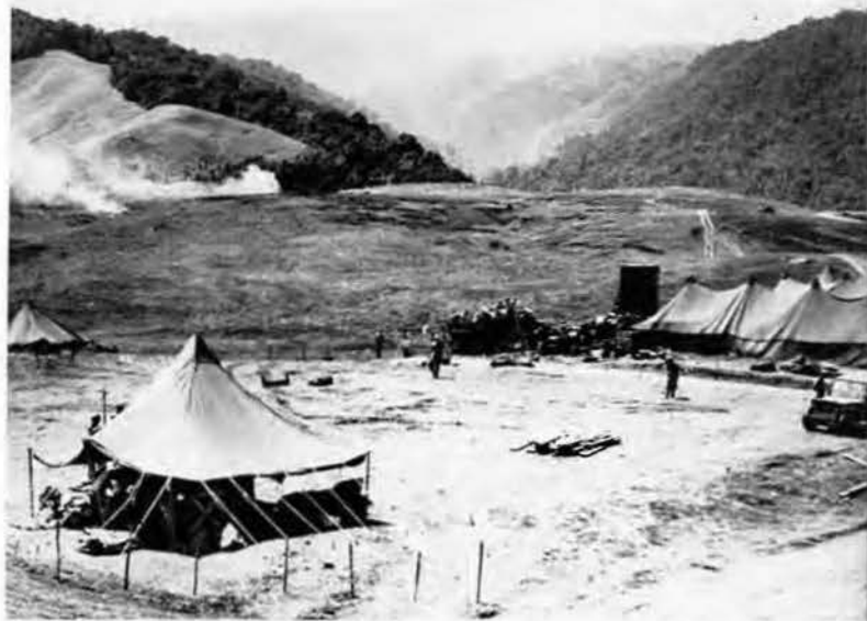
Laying out the galley.
