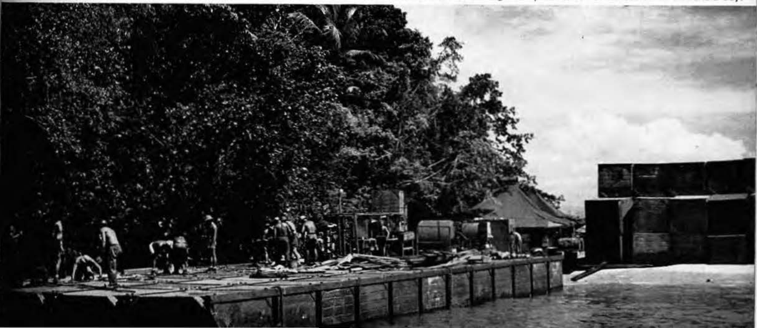
A completed pontoon barge ready to launch at Madeeran in Hollandia Bay.
