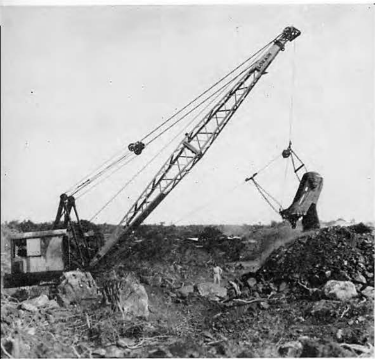
Ditching with Drag Line
