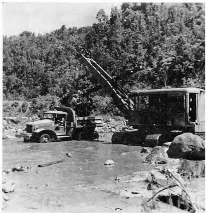
Loading gravel from river bed
