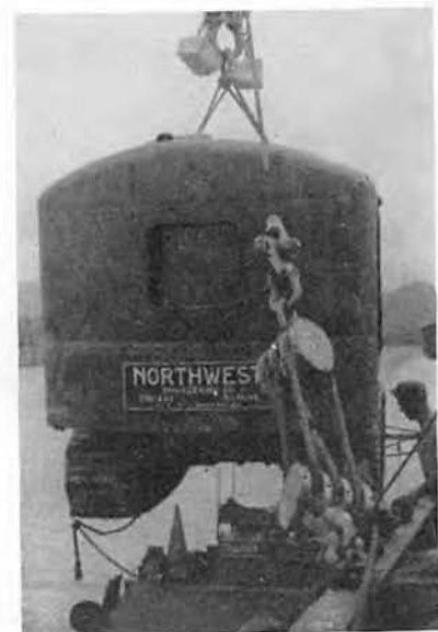
Unloading the big shovel at Hollandia
