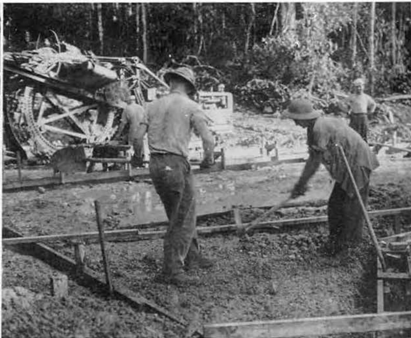
Laying the Chow Hall Foundation at Hollandia
