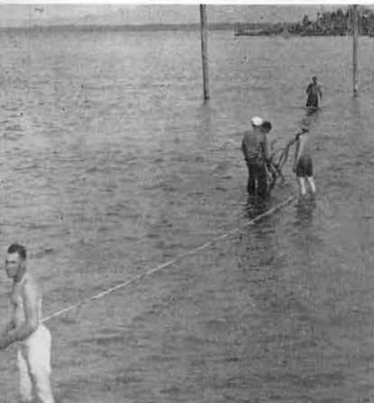
Laying submarine cable
