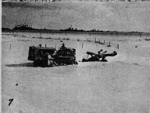
1. Pilot gives Casu 30 man instructions. 2. First fighter is serviced. 3. The airstrip grows. 4. Teresa Island parking area for airplanes. 5. Causeway to Teresa Island from Salome is started by Century Seabees. 6. Parking area nearly finished. 7. Bulldozer plows coral for causeway. 8. Parking area completed. 9. First planes parked on area.
