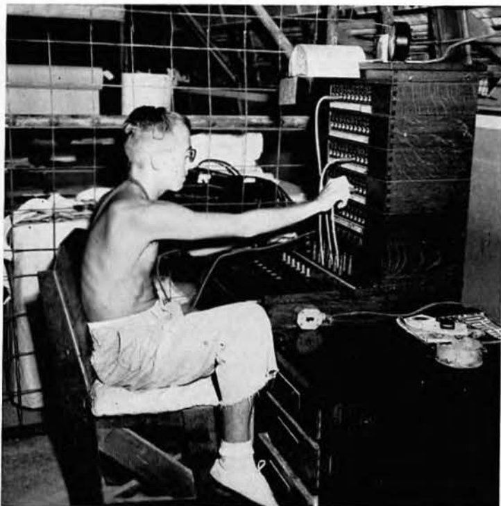
Telephone service—BuDocks Exchange.
