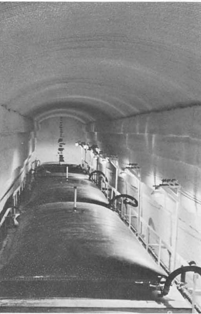
At Byrd Station, 10,000-gallon fuel bladders are coupled together in a side tunnel to feed DFA to the generators. Although Byrd is below the ice, some of the men must go outside to reach several of the scientific buildings. In Deep Freeze '66, to reduce the chance of their being lost, new poles were placed to support the lifelines, and the flags were set at shorter intervals.
