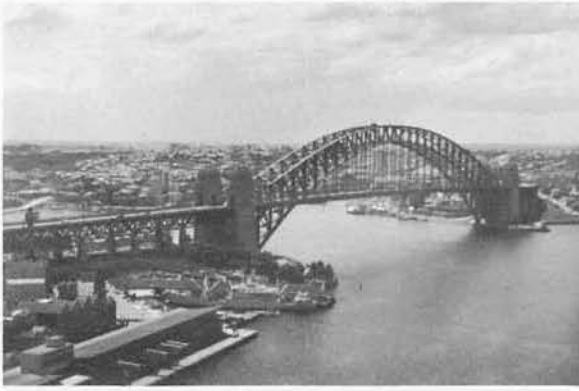
Sydney Harbor Bridge
