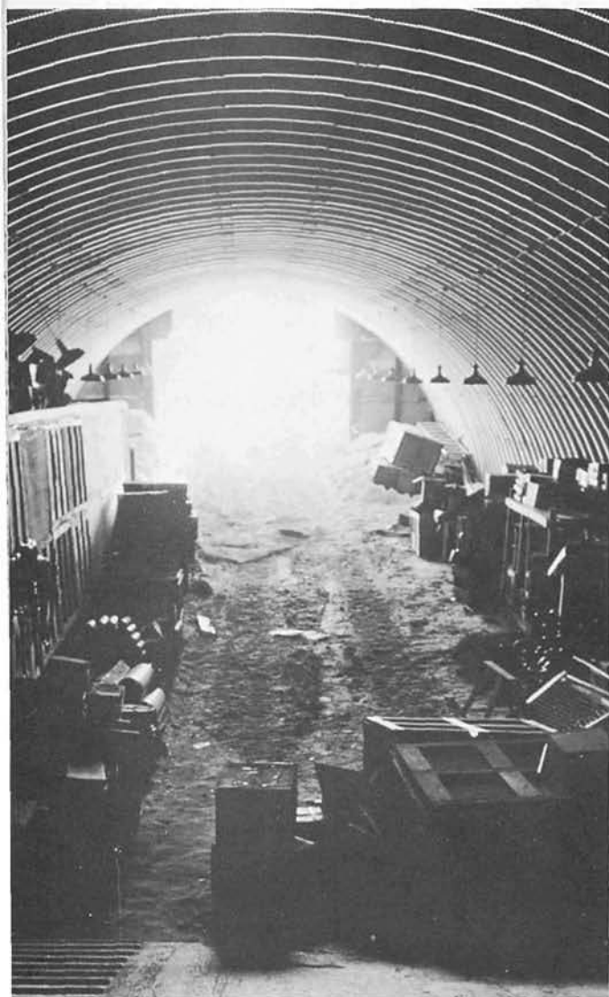
Above: Ramp for vehicles at the South Pole, showing the Wonder Arch that has made it possible to protect several stations far out on the ice from drifting snow.
