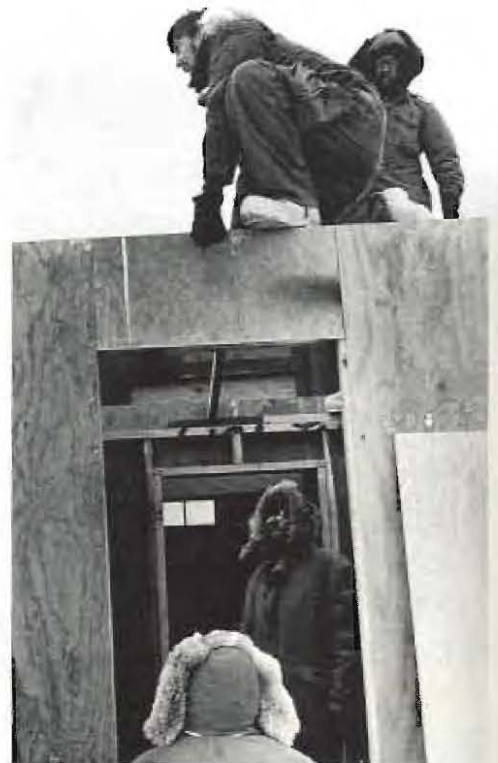
LTJG LEROY SAUERWINE DIRECTS activity (ABOVE) as Builder third class William Nixon and Builder first class Paul Renaud prepare to close the entrance to one of the Williams Field buildings.
