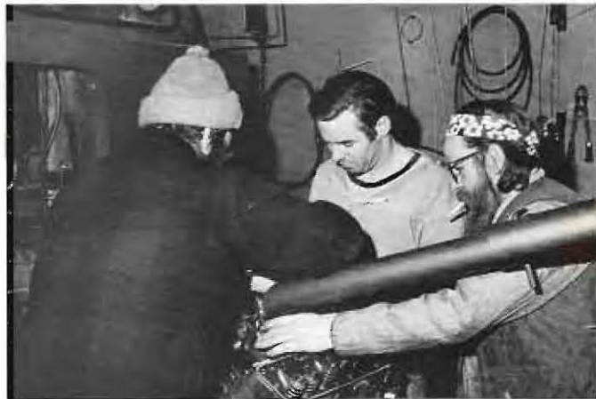
THE ELECTRONICS MONITOR, Hayden M. Mercer, Hospital Corpsman first class, is assisted by a member of Public Works, Equipment Operator second class Donald J. Hudlemeyer, in preparing (FAR LEFT) a spent core shipping cask for 30,000 curies of radioactive material. Meanwhile, (LEFT) Dudley Wells, Specialist 6th class, U.S. Army, double checks the pressure of the main turbine lube oil system at the nuclear power plant. The three Holmes and Narver employees, (BELOW) Jim Prill, Fred Dotterer, and Pat Arendt battle a bulky torque wrench as they conduct equipment maintenance.
