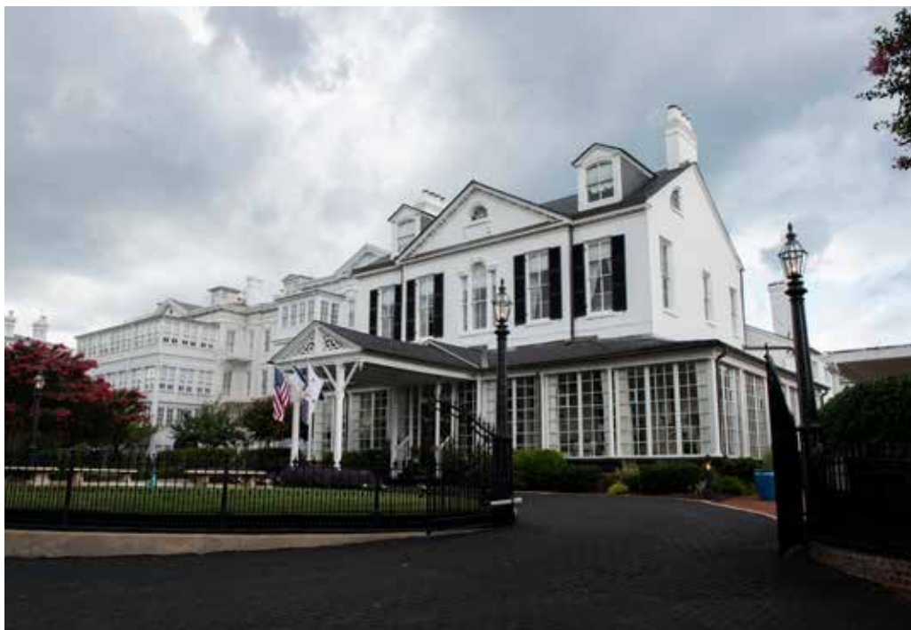
Tingey House exterior, southeast view. (U.S. Navy/200804-N-BB269-1161)
