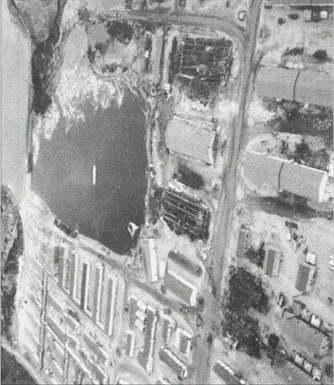
Damage to Ft. Mears caused by Japanese raid of 3 June
