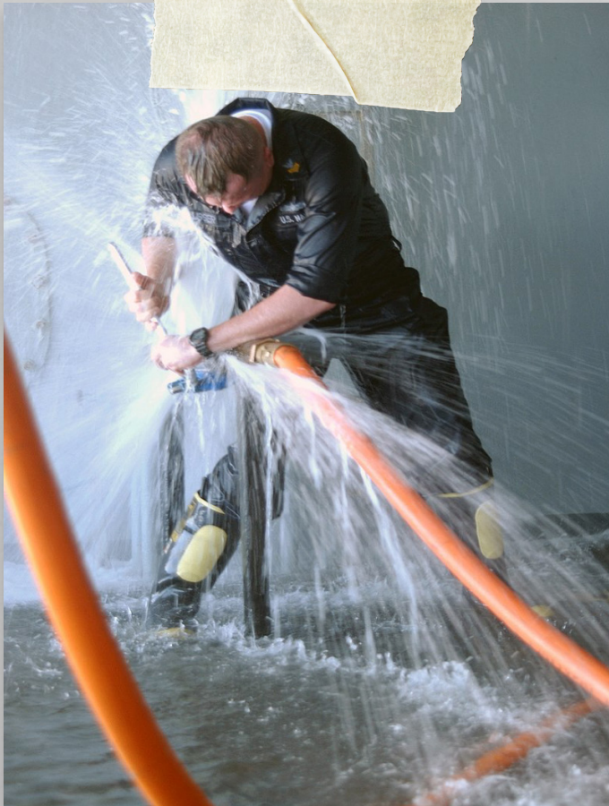
In this photo a U.S. Navy damage controlman practice pipe repair.
