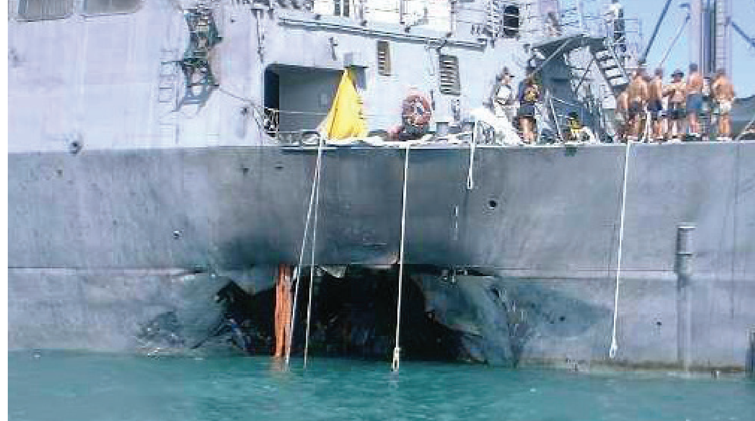
USS Cole's damage is shown clearly in this image. (Courtesy of James Parlier)
