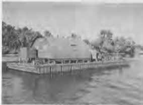
Fully equipped gate vessel.
