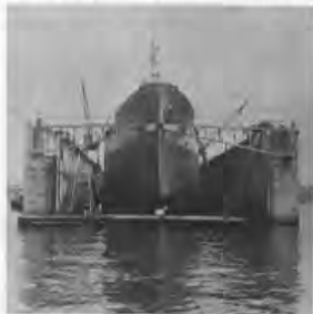
Floating pontoon drydock accommodating vessel.
