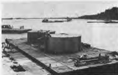
Seabees put finishing touches on fuel barge.
