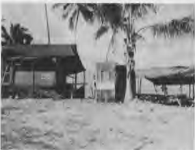
Good chow-wagons on the work also help morale
