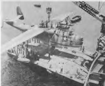
Seaplane being lowered to pontoon propulsion barge for repairs.
