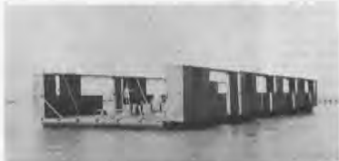
A typical floating pontoon drydock.
