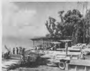
Advanced base construction uses lots of lumber.
