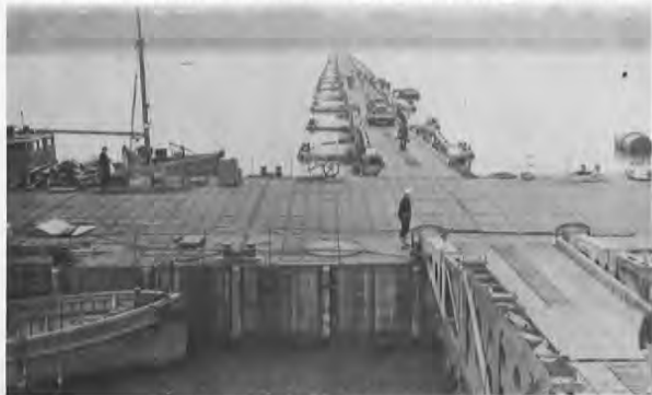
A spud pierhead and British built "Whale" bridges at Normandy
