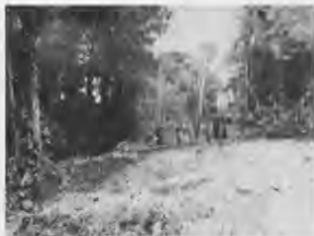
Roadwork must begin on D-day.
