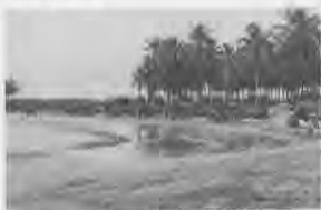
A completed taxi-way.
