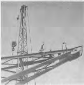
Ship repair requires heavy cranes.
