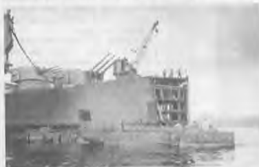
Cruiser with the damaged bow section removed.
