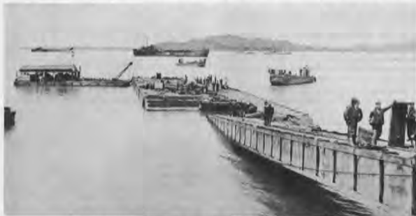
Pontoon pier construction is usually needed at an advanced base.
