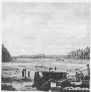
Seabees ready to begin final surfacing.
