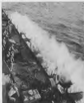
Seabees chop lashings and launch pontoon causeway.
