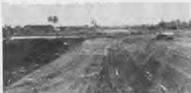
Surfacing material arrives at strip.
