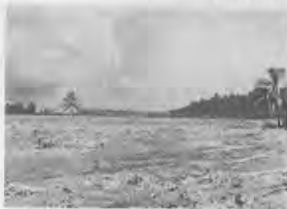
Fighter strip clearing nearing completion.
