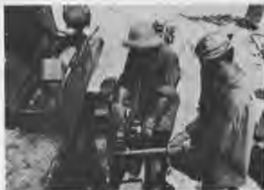
Seabee "know-how" can accomplish equipment repairs without the usual facilities.
