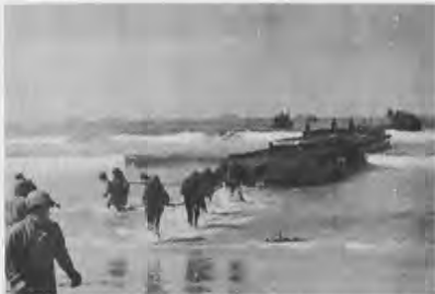
Seabees carrying anchors ashore to secure causeway to beach.
