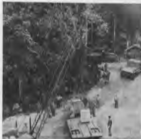
Cherry picker unloading cement clumps.
