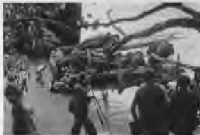
Temporary radar for base defense is landed on D-day.
