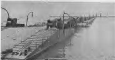
"Whale" bridges leading out to spud pierhead.
