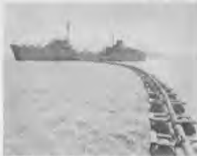
Seabees unloading oil via floating pipeline.
