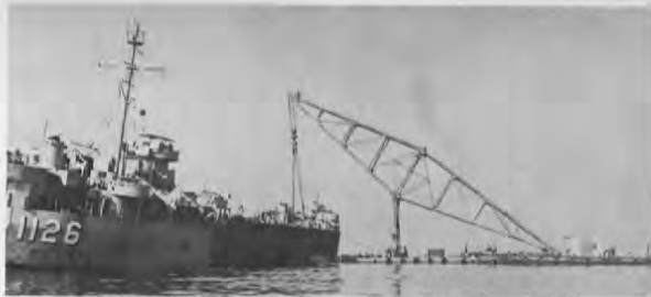
Pontoon causeway section being secured to LST.
