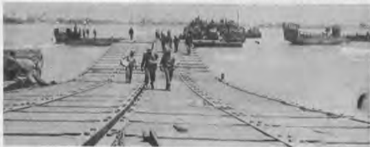
Rhino ferry comes alongside pontoon causeway to unload vehicles at Normandy.
