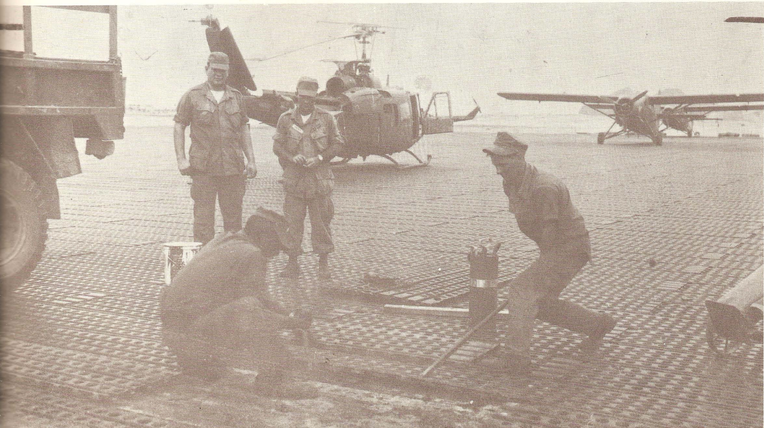
Repairing a runway
