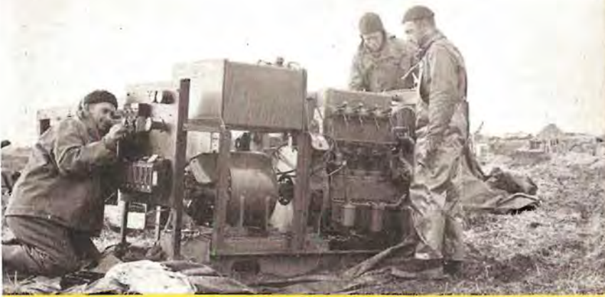
● On an Aleutian beach Seabees set up a Diesel Electric Generator as quickly as possible after landing in order to supply electric power.
