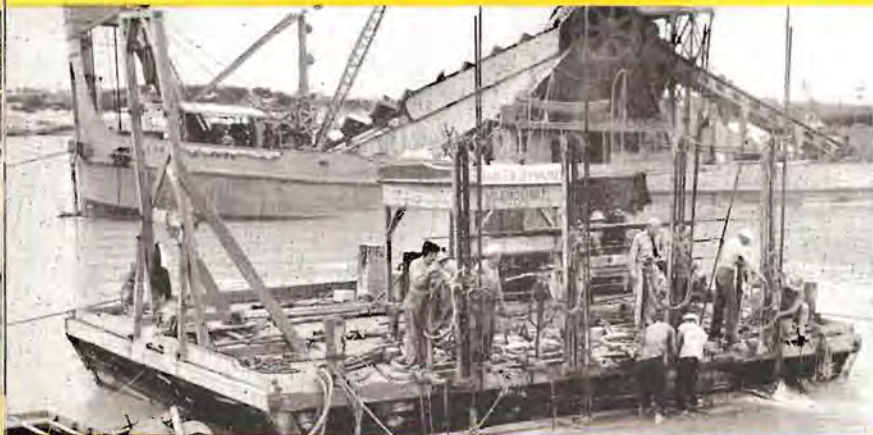
● Caribbean. Blasting huge coral growths to make way for the construction of a marginal wharf at this outlying base. Seabees on a dredge derrick drill before laying dynamite charges.
