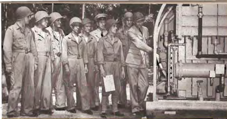
● As part of the technical training in the use of advance base gear, these Seabees are receiving instruction in the operation of a water purifying unit.
