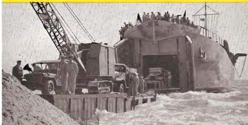
● As part of advanced training at Port Hueneme, Calif., Seabees receive intensive training in landing operations. Equipment is being unloaded over a pontoon causeway from the LST.
