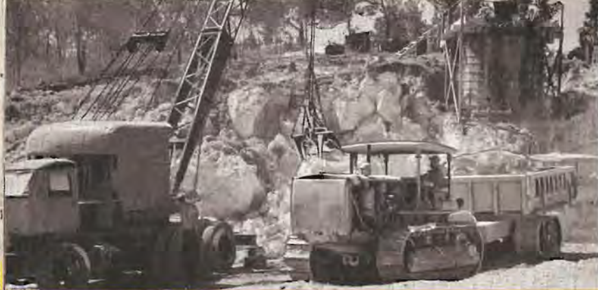
● Bermuda. Excavating coral rock which forms the basis of all roads on this island. The entire road system at this base was greatly improved by the Seabees.
