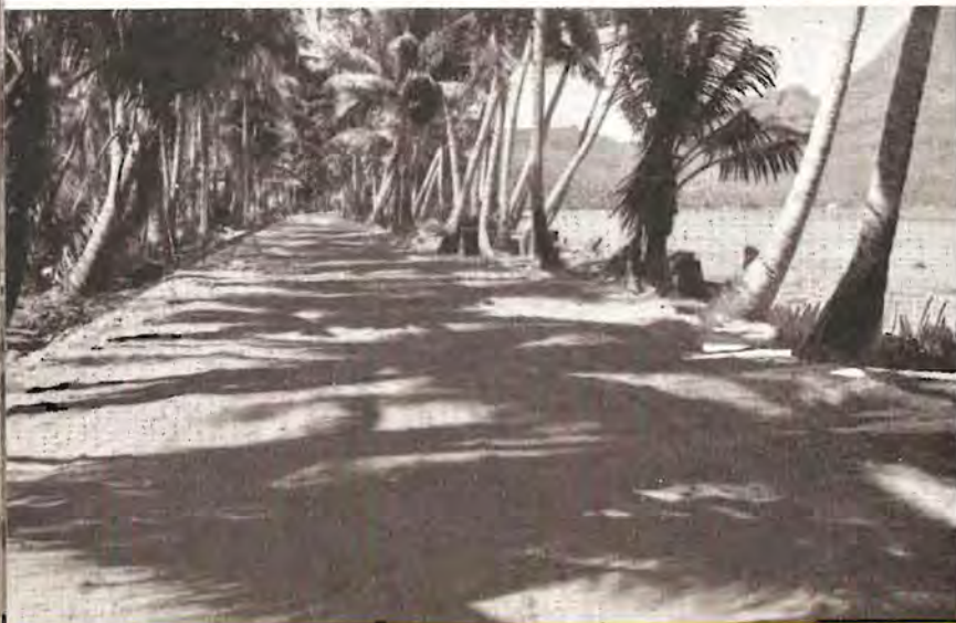
● Before and after. The upper picture shows the beginning of a roadway along the beach; and below, the park-like drive which appeared in a few days.
