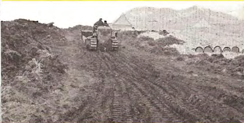
● Temporary road cut by bulldozers through the frozen tundra of an Aleutian beach. At this point it is far from a park boulevard but today it is firm and serviceable.
