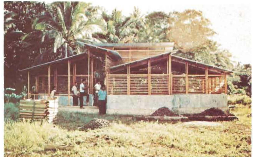
Supervised Micronesians in building Tol Island dispensary.
