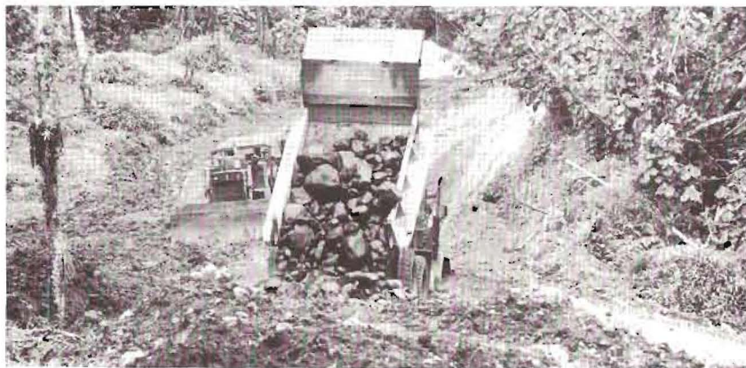
. . . and placed on road surfaces . . .
