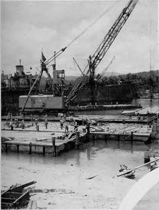
Assembling pontoon causeways for the Philippine landings
