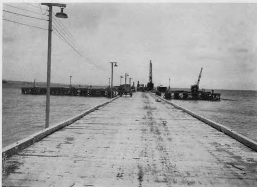
Timber dock constructed of Philippine mahogany
