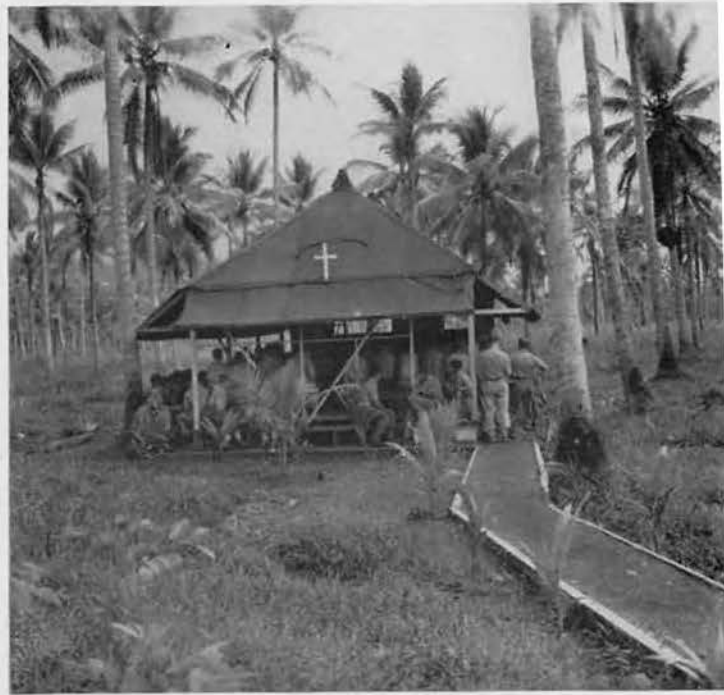
We aided the Aussies in building this small roadside chapel
