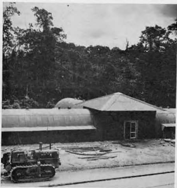
Naval Administration building
