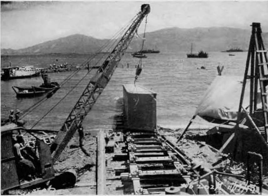
Launching a pontoon string
