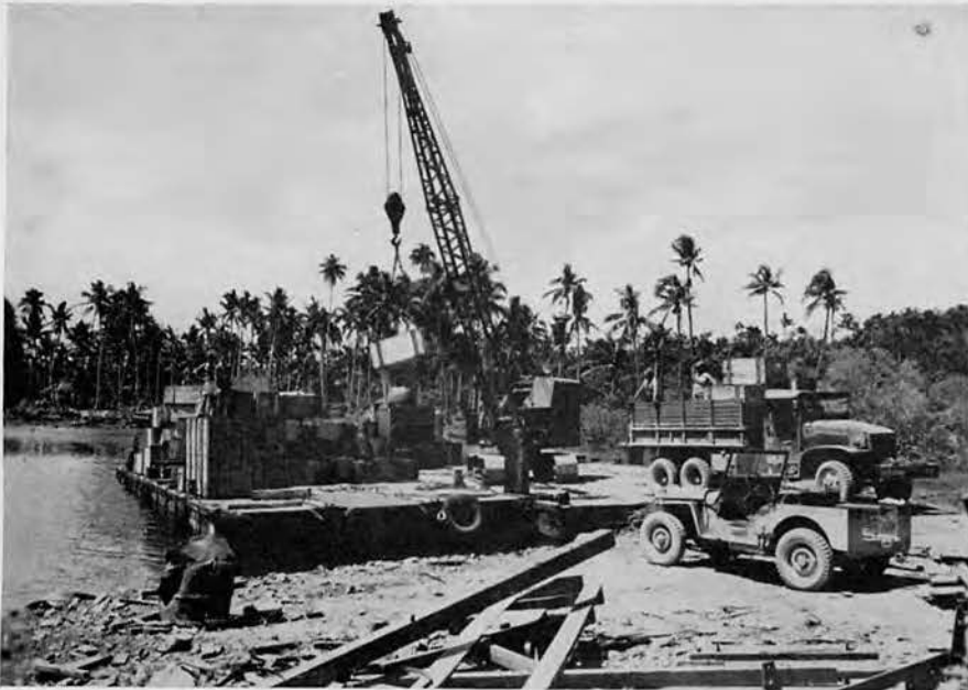
Top —Supply office and warehouse.
