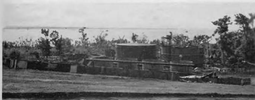
Water filtration plant under construction
