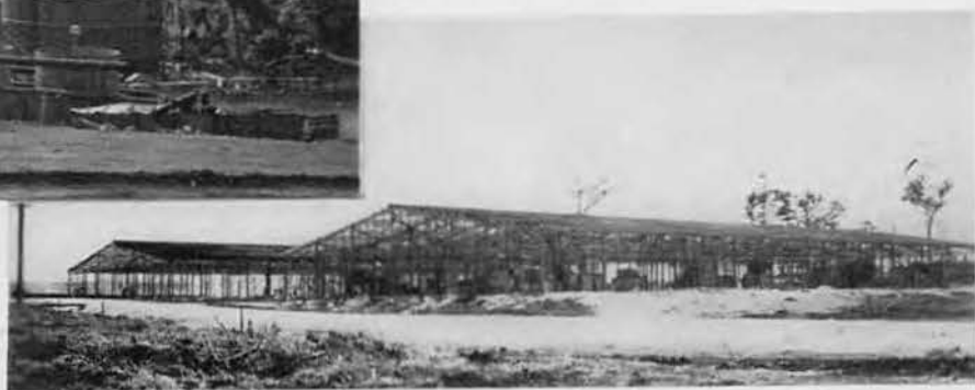
Frame warehouse under construction
