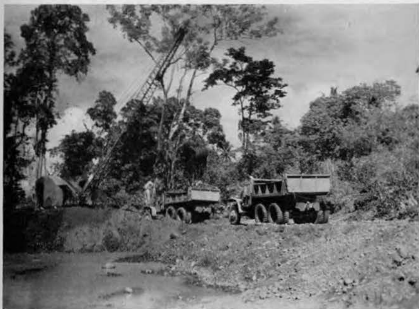
Loading gravel for highway fill
