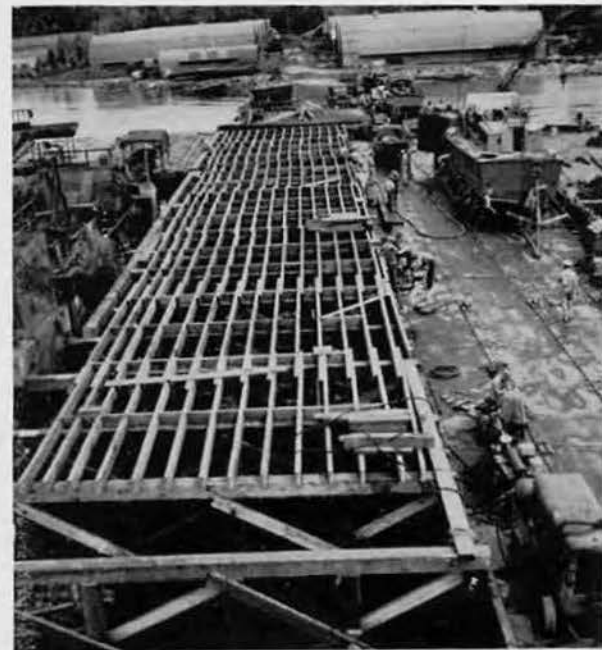
New Guinea repair dock
