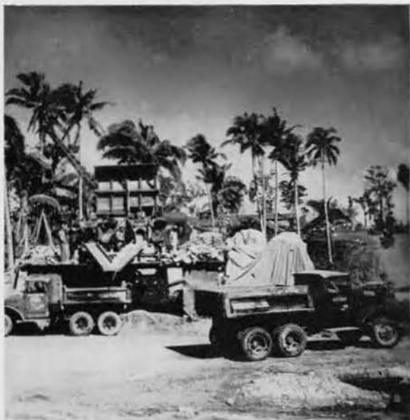
Philippine ready-mix concrete plant
