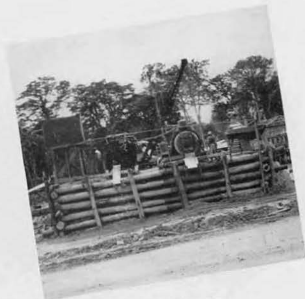
One of our New Guinea ready-mix plants
