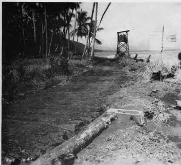
Corduroy road construction
