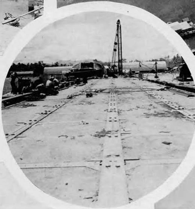
Temporary pontoon dock
