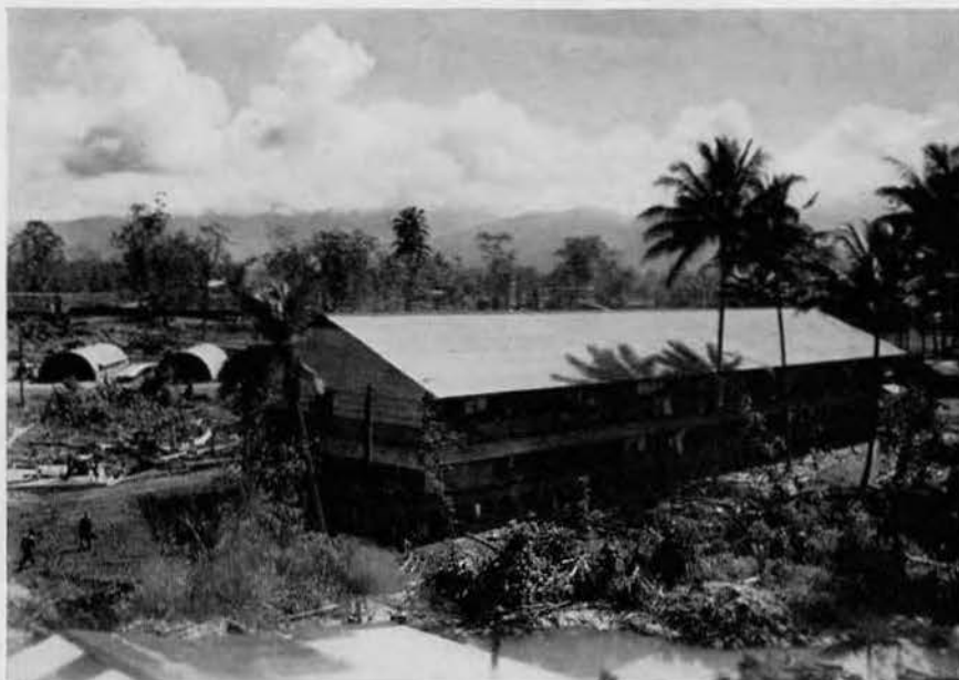
400-men barracks at a New Guinea base
