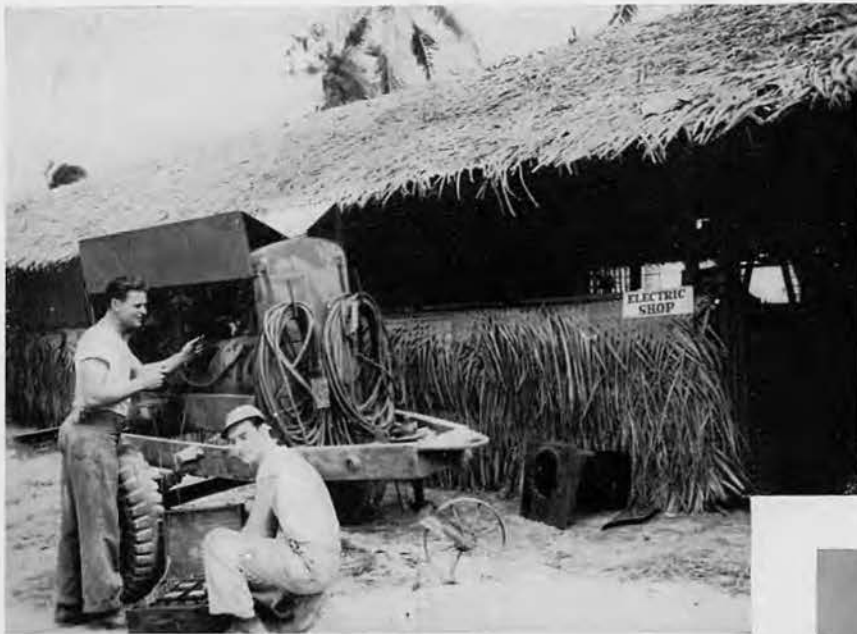
Left —Saleski and Shultis test a portable welding machine.
