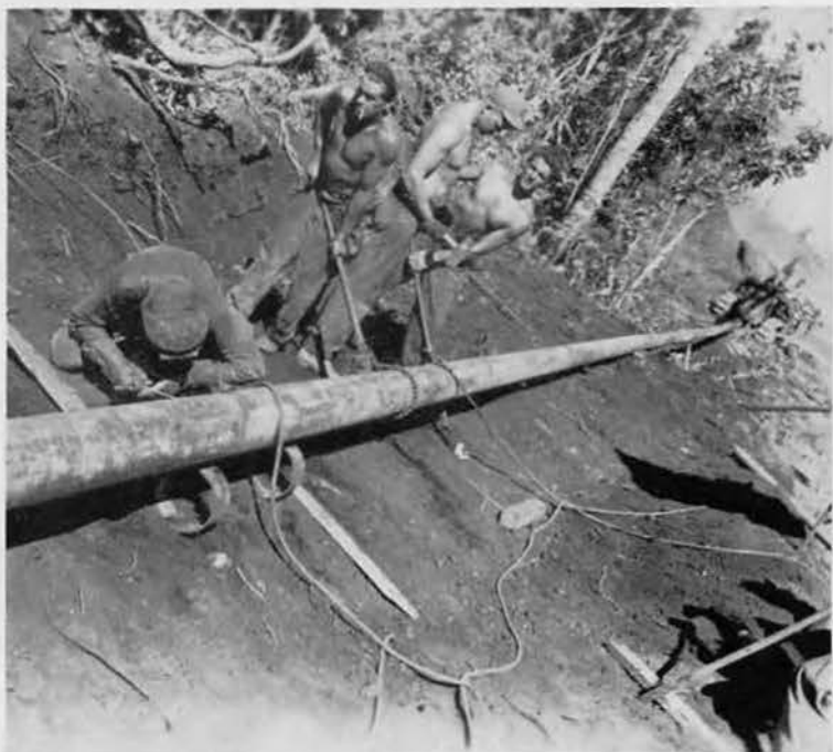
No frost worries on this pipe line job
