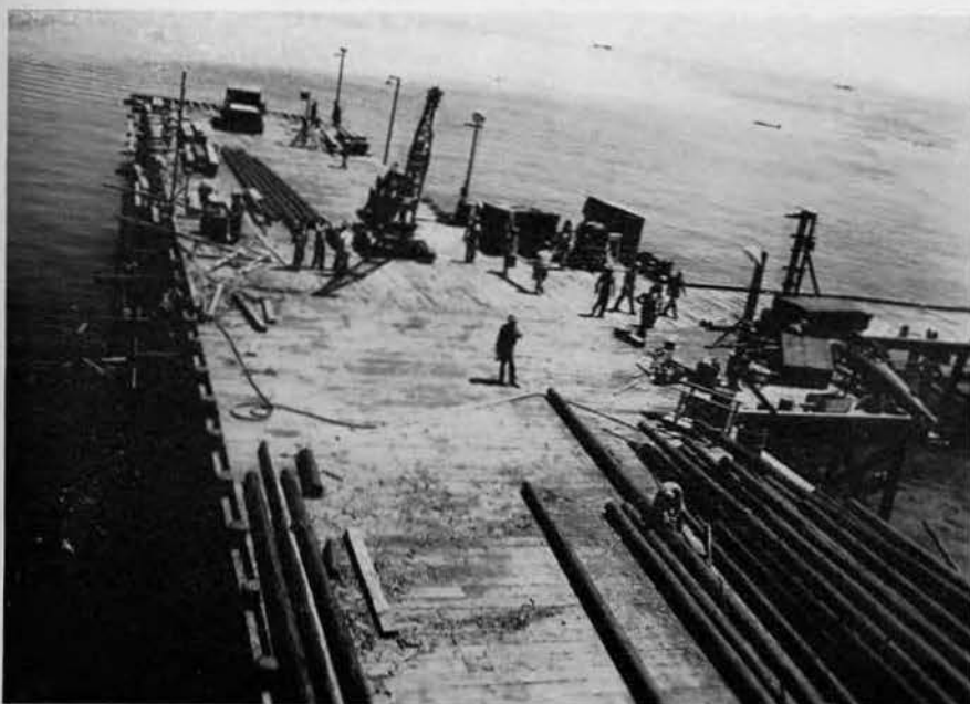
View of T-section of the above dock
