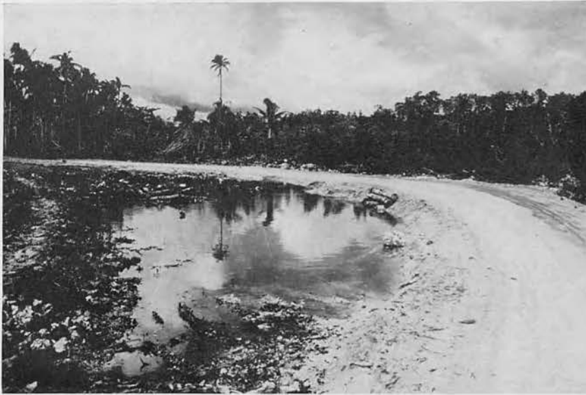
Two methods of crossing a swamp — native coral causeway on the left, a Seabee road on the right.
