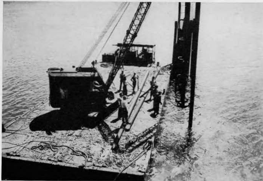
Floating pile driver
