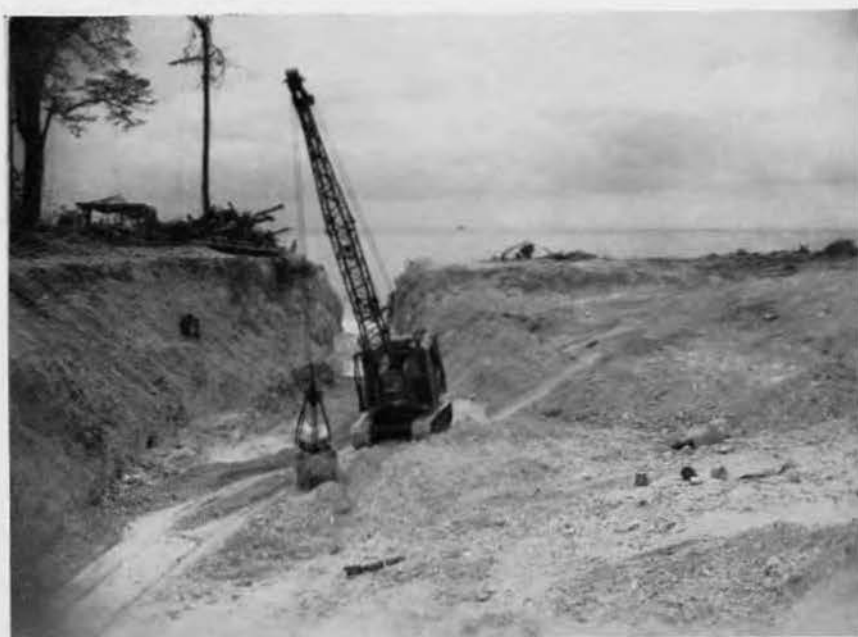
A dual operation—draining a malarial swamp while obtaining coral fill
