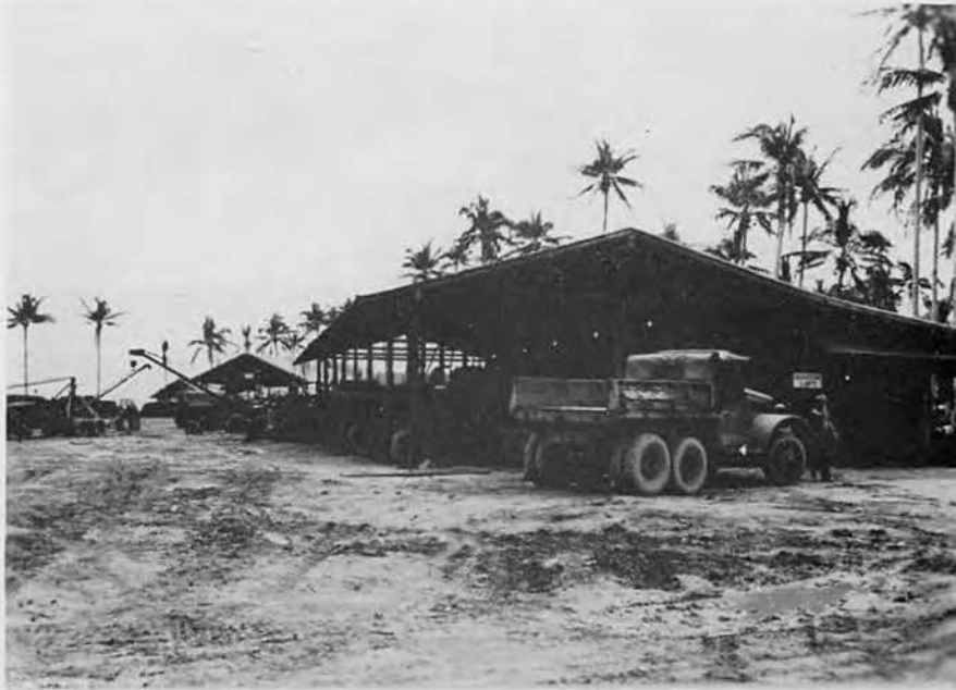
General view of equipment repair shops
