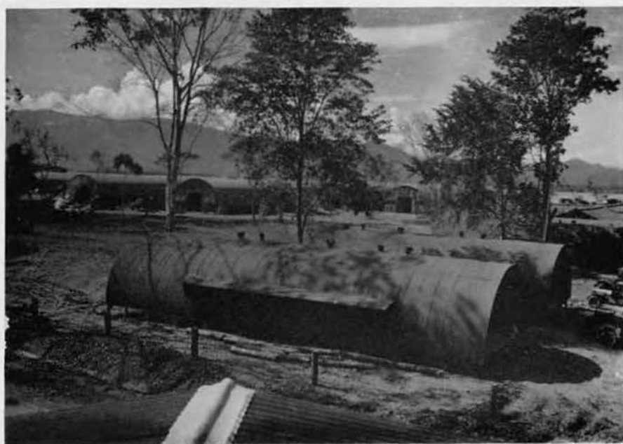
Officers' Quarters and Repair Shops
