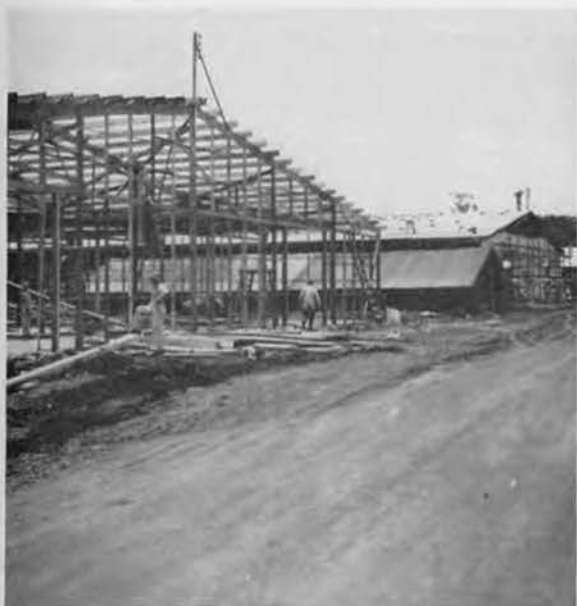
Frame warehouse under construction
