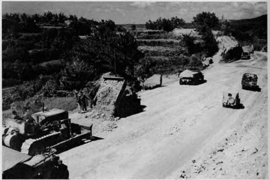
Single lane road is converted to a two-lane highway.
