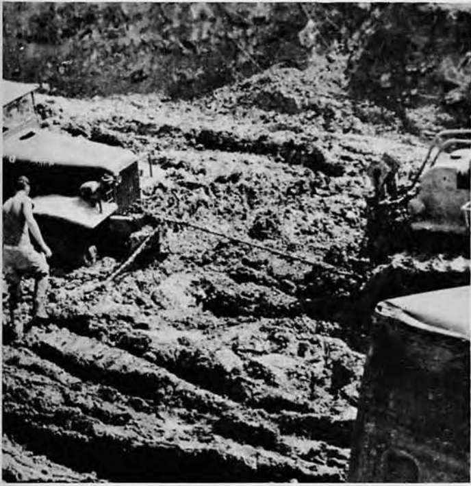
'Dozer deep in the mud extracts a Marine supply truck enroute to the front lines.
