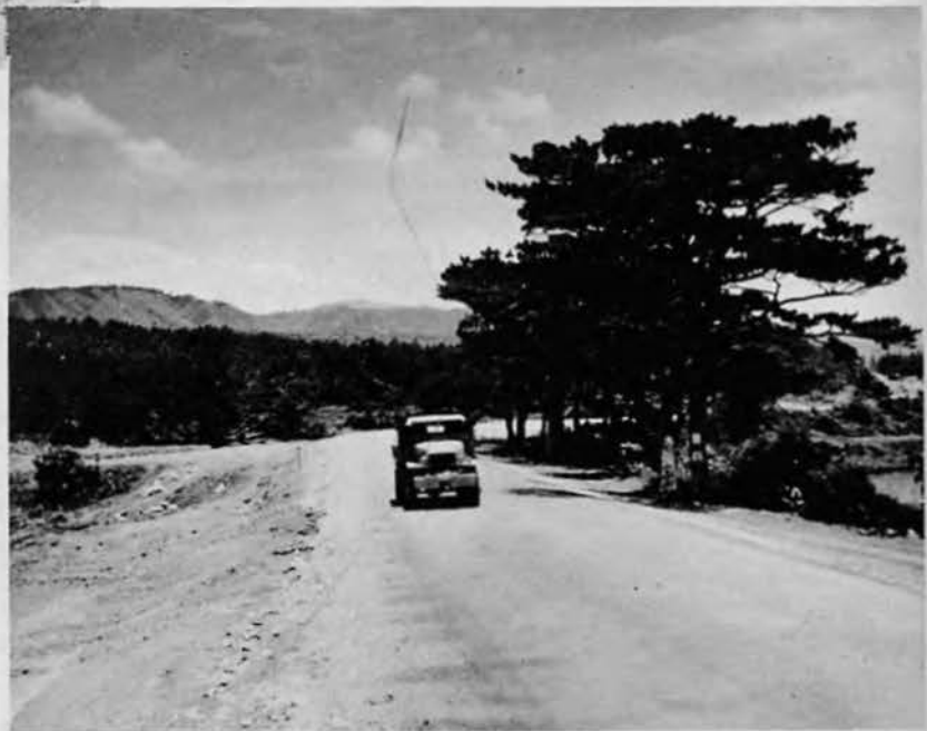
Here is the finished product. The super-highway as it approaches the village of Onna.
