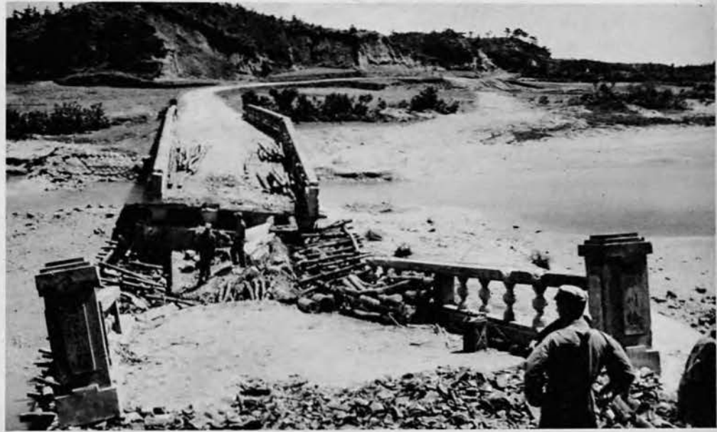
Bridge approach damaged by combat action at Ishikawa.
