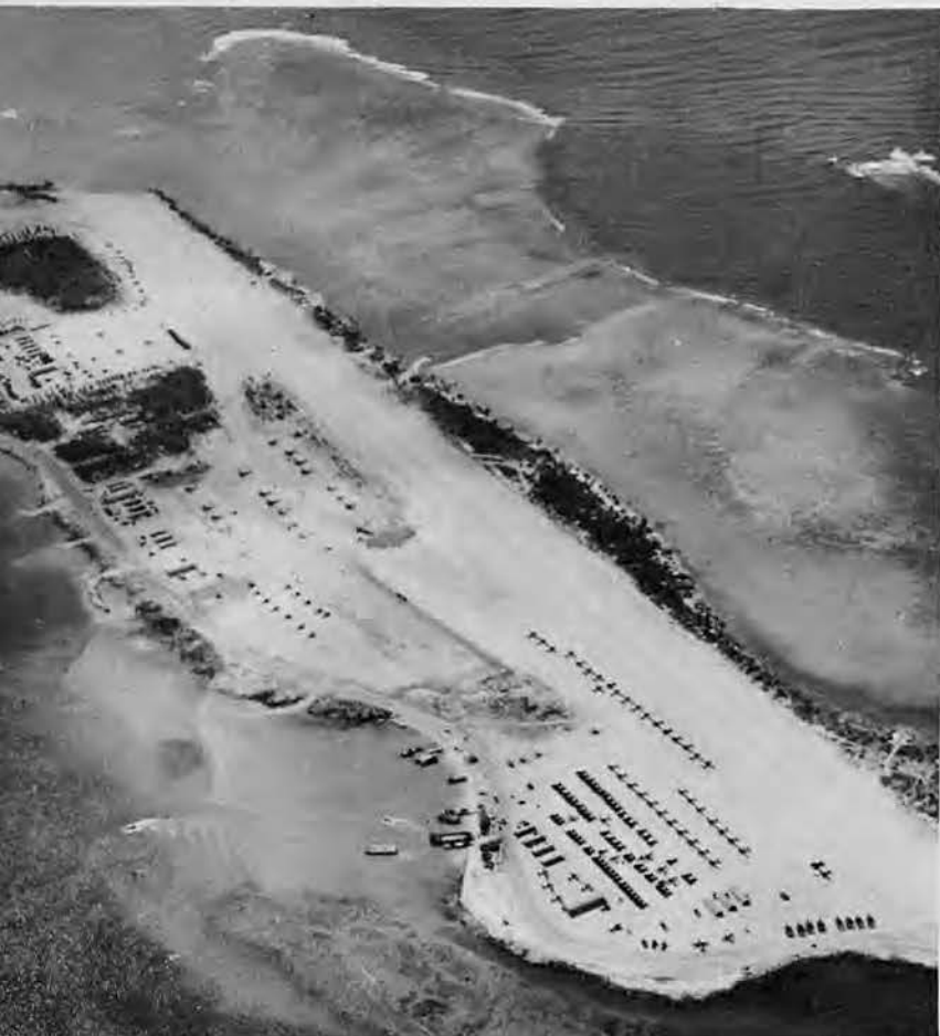
The 5500' air strip hewn out of the dense palm plantation and completed within thirty-five days.
