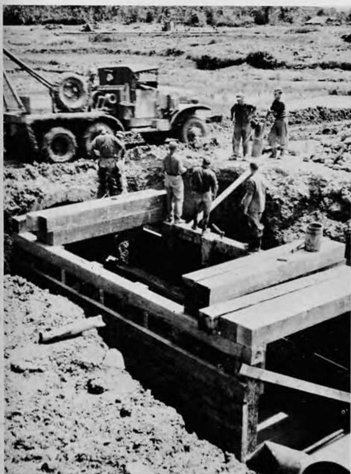
Heavy timber box culvert replaces inadequate Jap bridge.
