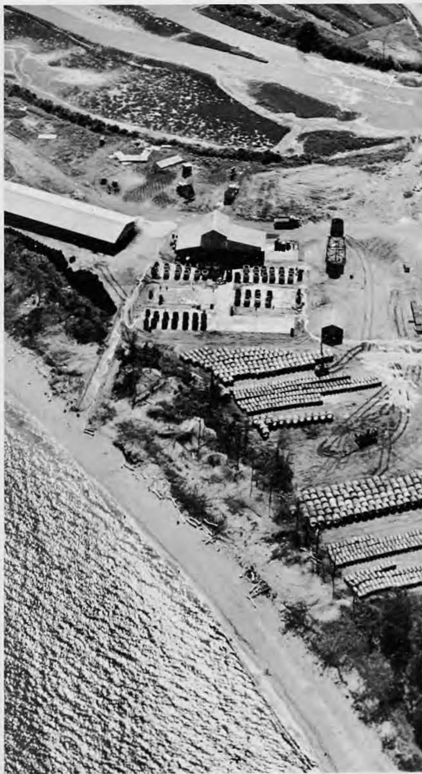
An aerial view of our concrete pipe plant and storage yard at Antuso.
