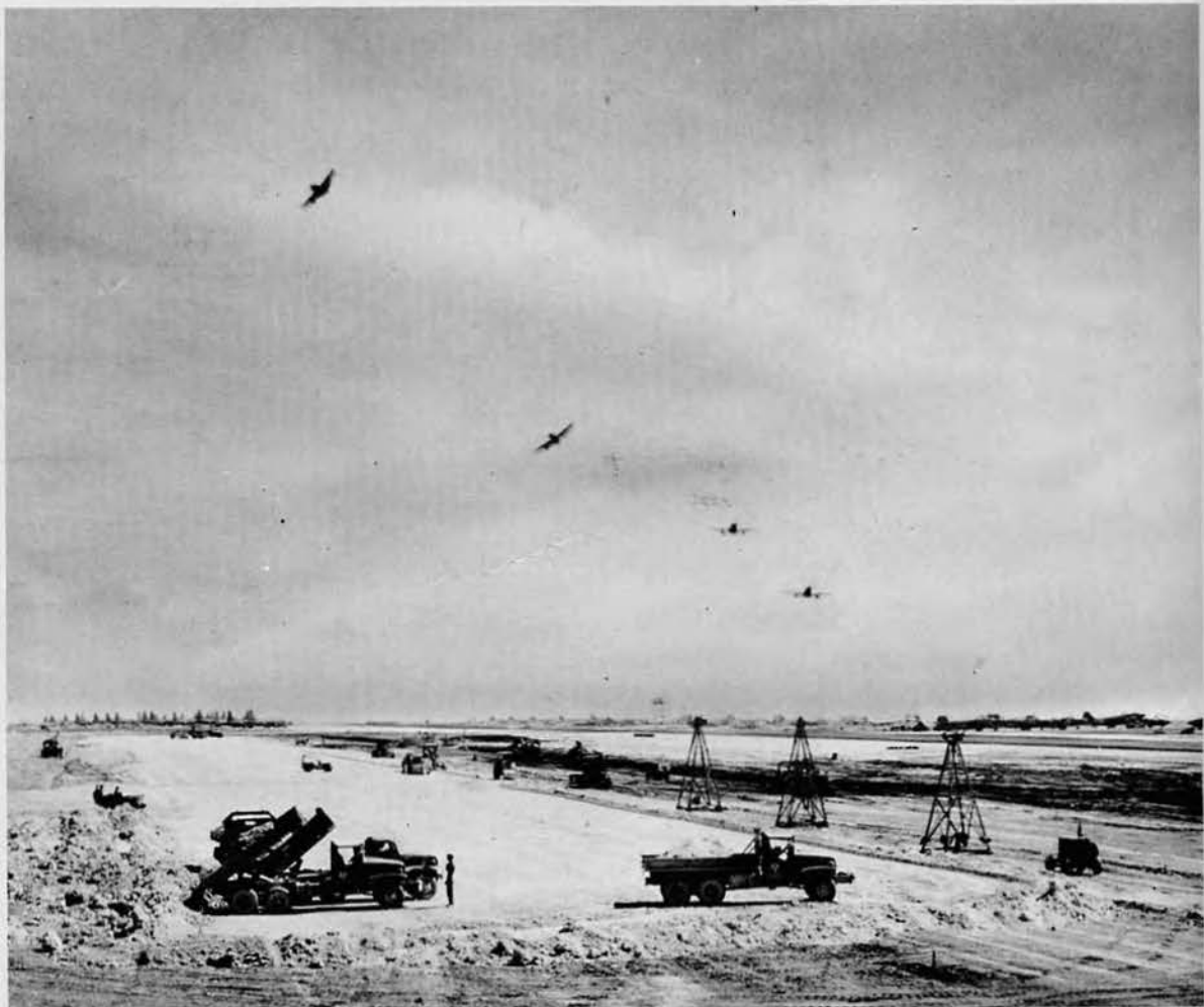
(Below) Four P-51 Mustangs zoom over the tops of our men, just returning from a bombing mission over Tokyo. We worked 24 hours a day to hasten the completion of the new field. Portable lights on towers furnished the lighting for the crews at night.
