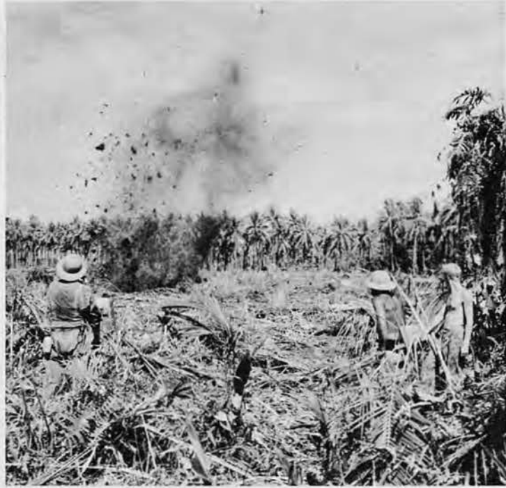
Blasting tree stumps with dynamite as project begins.
