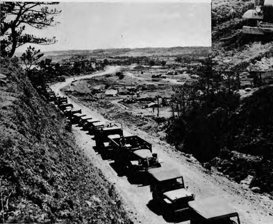
(Below) Results of exhausting efforts, the roads were packed down and traffic moved forward at a rapid pace.
