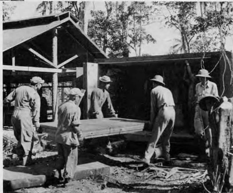
Paul E. Roll, CSF, and his men erect the immense "reefers" on native logs for support.
