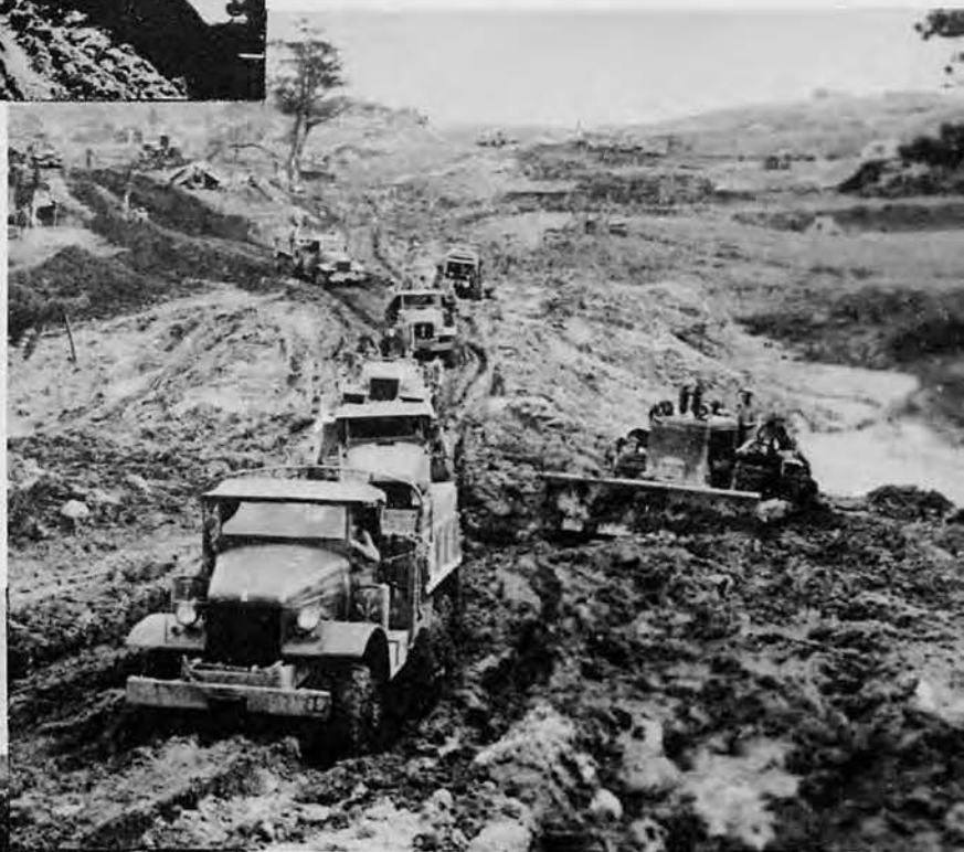
(Above) Supply train returning from nearby front lines, assisted thru impassable stretch of knee-deep mud by our big bulldozers. It was such conditions as shown that earned our Battalion the Navy Unit Citation during heavy artillery shelling.
