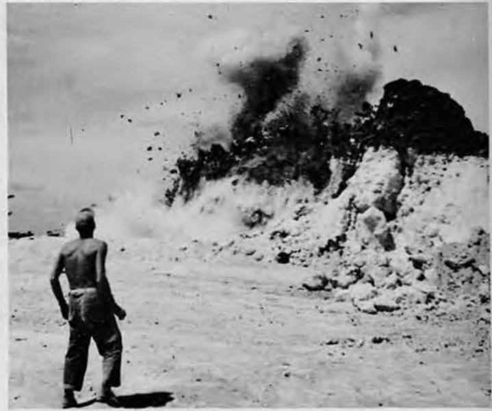
Blasting coral for road surfacing and compacting materials.
