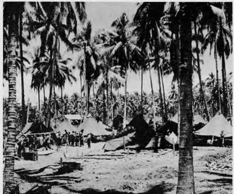
First construction camp in a palm grove situated at Torokina Point.
