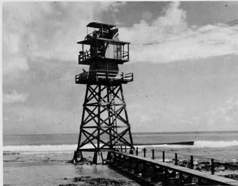
"Still another crew went to Ndrillo Island and constructed many things, one of which was this Harbor Control Tower."
