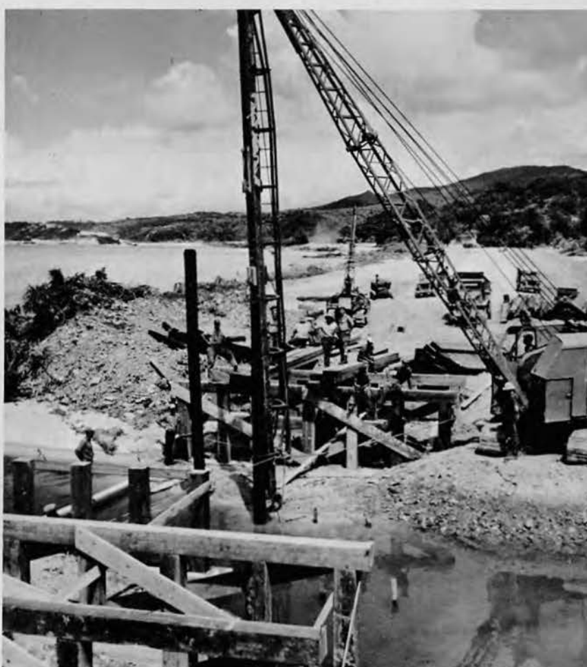
A new bridge eliminates blind curves.
