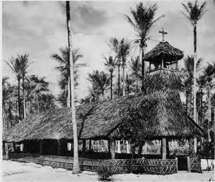
Grass thatched woven palm Chapel constructed by the Christian natives on Ndrillo Island.
