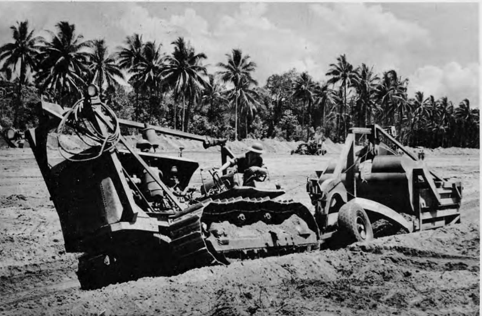
... 'til at last ... we installed the final drainage system, and kept the strip operating ...
