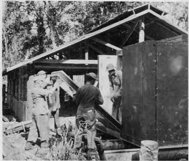
Refrigerator crew setting up "cold storage boxes" by sections.
