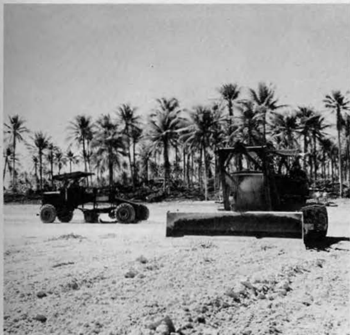
Another link toward the completion of the Strip on Pityilu Is.
