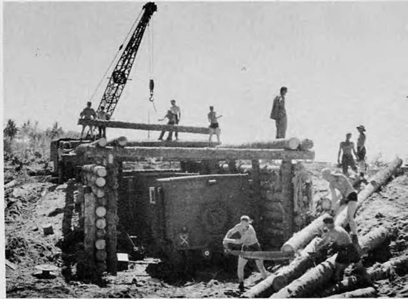
Underground Radar Station protected by heavy coco-logs.
