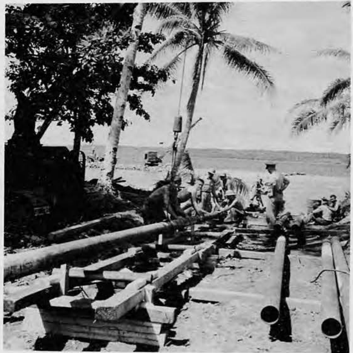
Preparing the long pipe-line . . . ship-to-shore lines for fuel.
