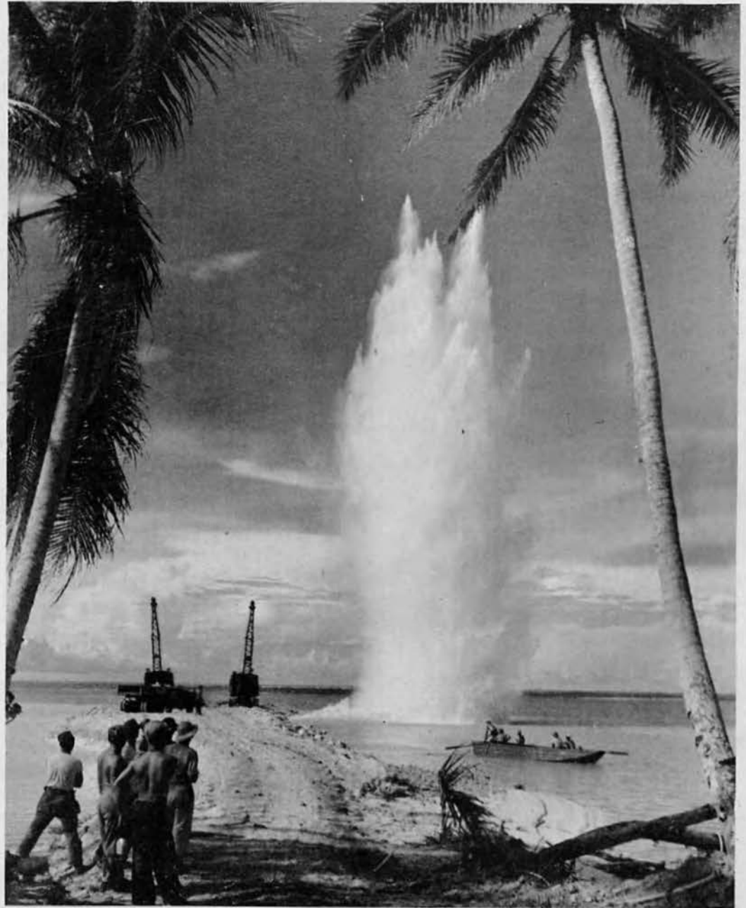
Tons of water surge majestically into tropical skies as coral reefs are blasted for air-field material.
