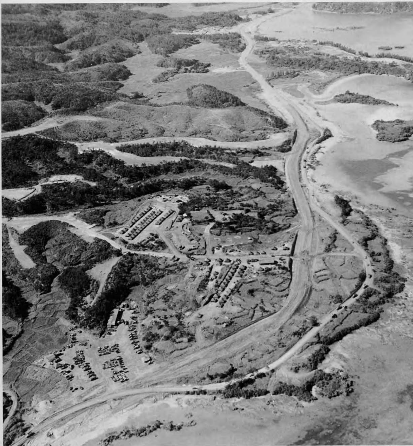
Aerial view of the new three lane highway showing the elimination of unnecessary curves which can also be seen winding along the shore line. In the background the scenic view of one section of Okinawa . . . untouched . . . unspoiled with its rural effect. Taken just north of Onna-by-the-shore.
