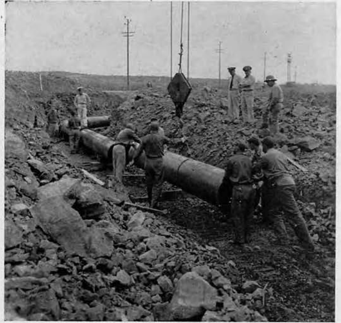
LAYING A SECTION
