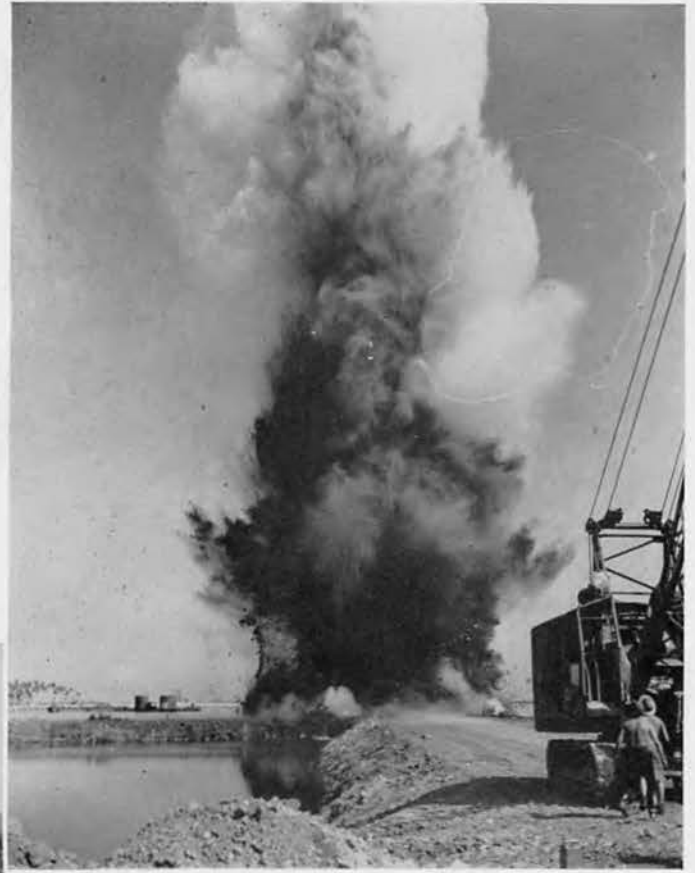
BLASTING APPROACH TO BOAT BASIN
