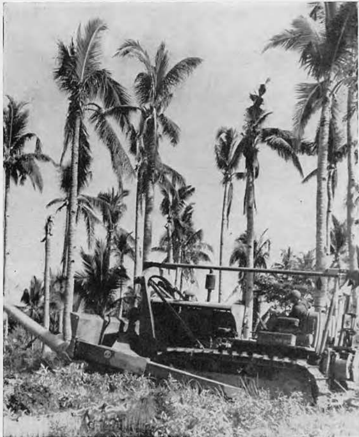
THE BULLDOZER TOOK OVER
