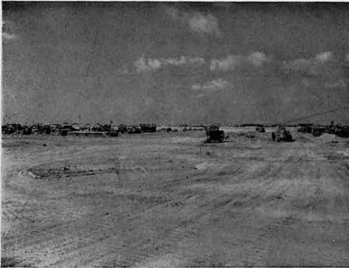
EXCAVATING FOR TAXIWAY
