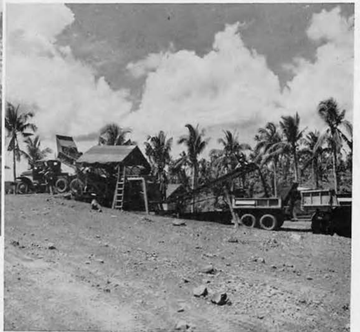
AGGREGATE FOR CONCRETE AND ROAD SURFACING
