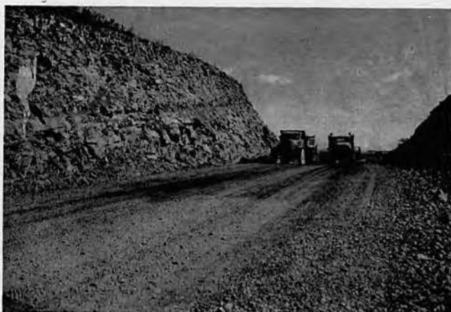
THE BIG CUT 13,000 YARDS, 4 TONS OF DYNAMITE
