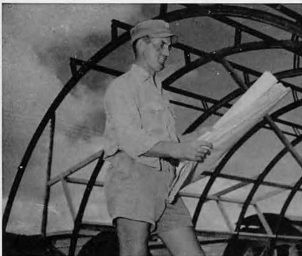
L. C. FROST, JR. Chief Carpenter, C.E.C.
