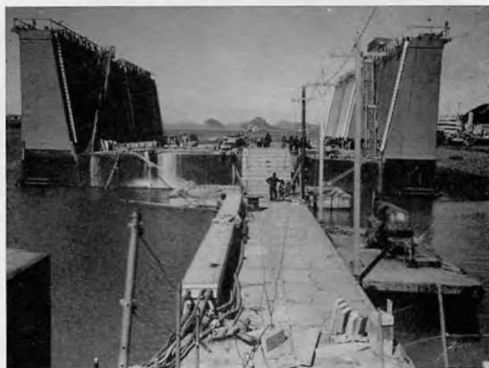
INSTALLING 7,000-TON DRY DOCK
