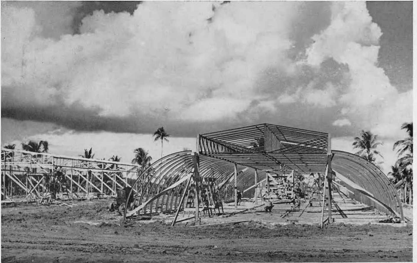
CENTRAL SHIP'S SERVICE AND POST OFFICE UNDER CONSTRUCTION
