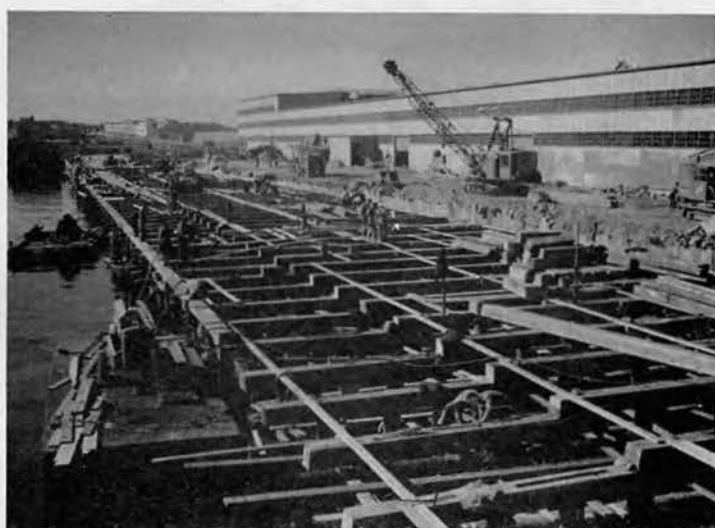
INSTALLING 7,000-TON DRY DOCK
