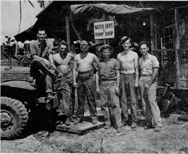
WATER AND PUMP PLANT CREW
