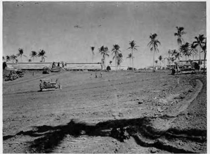
GRADING FOR OPEN AIR THEATER
