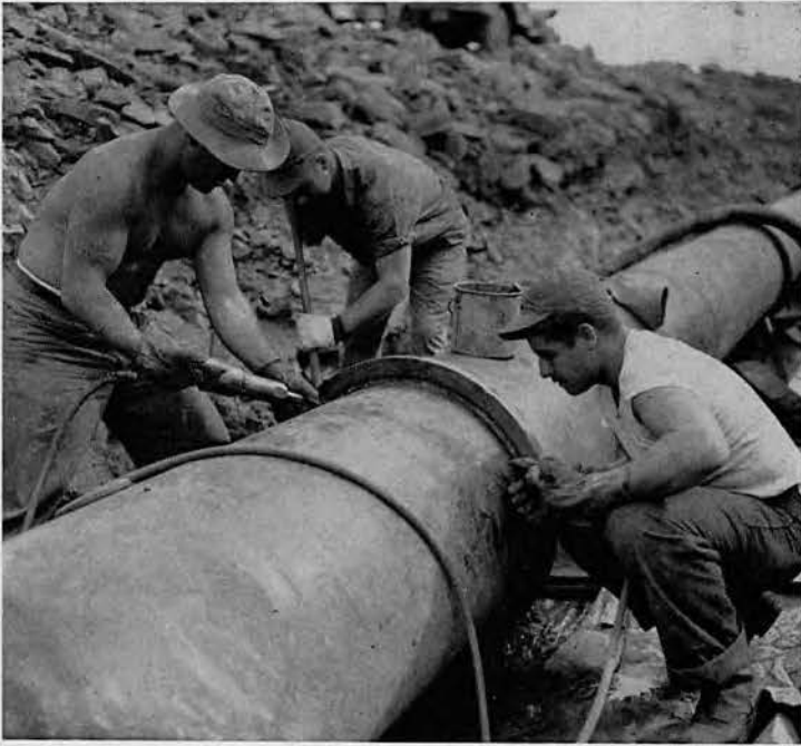
CAULKING A JOINT
