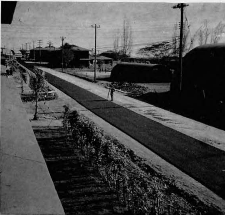
13,700 L'N FEET OF PAVING
