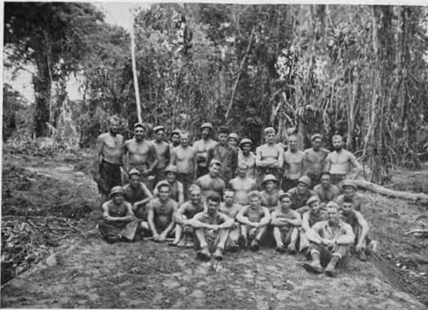
Construction party poses on completed bridge
