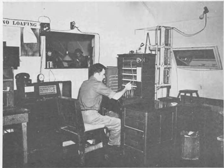
Communications office with Kaplan at the switchboard.
