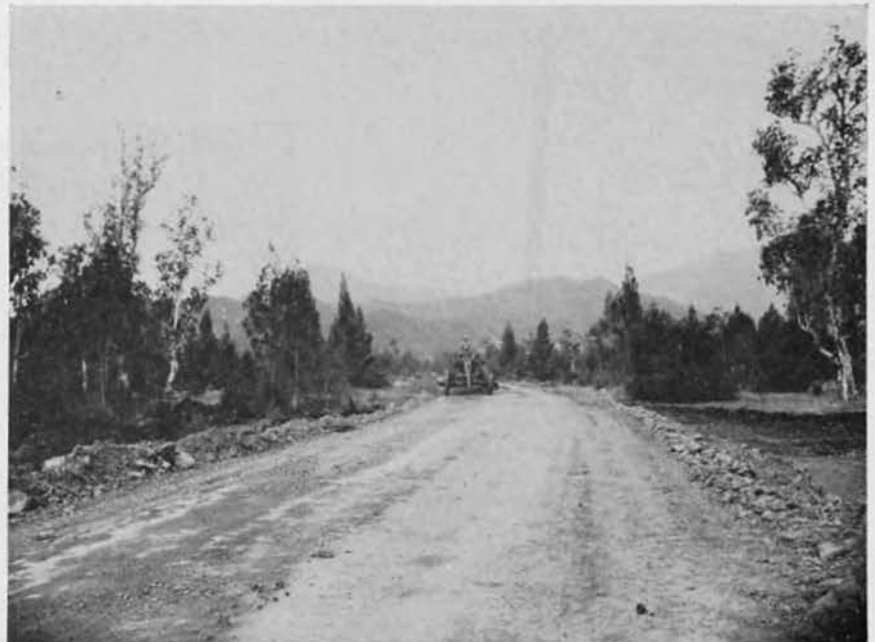
Road construction, Camp Kaiser.
