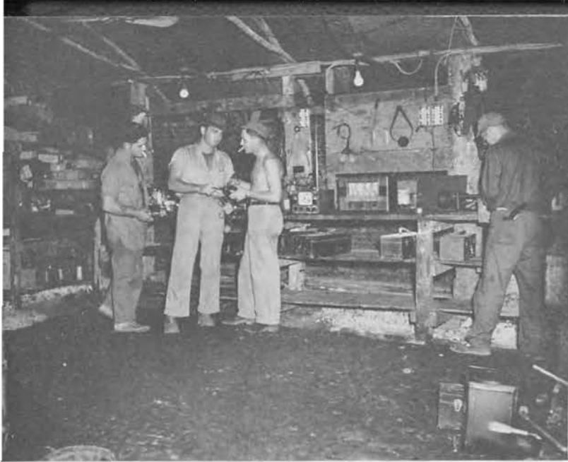
Electric Shop—Demonte, Chief Hill, Gass, Budd.
