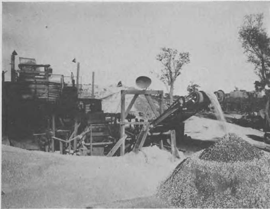
Below: Crusher in operation.
