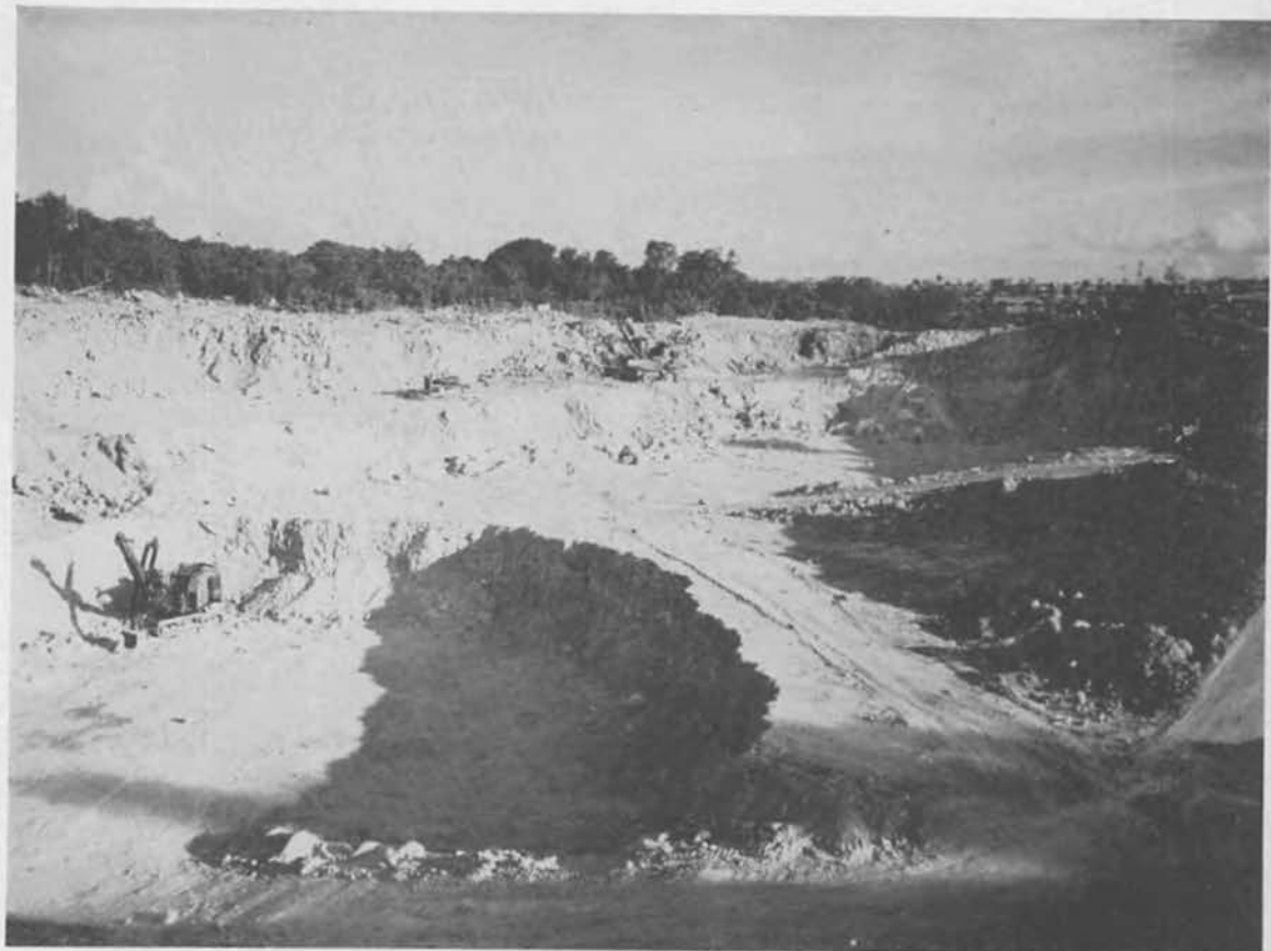
Three tier operation in Quarry.
