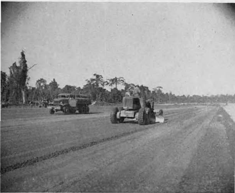
Grading on Fighter Strip.
