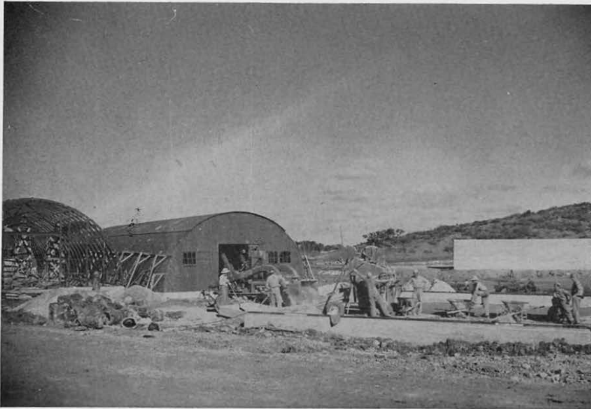
Construction scenes at Engineer Warehouse, Marine Corps, 1st Base Depot.
