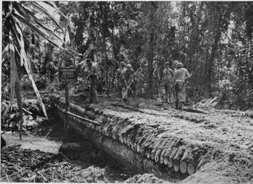
One of the first bridges nearing completion
