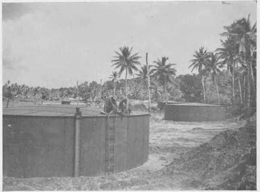
Tumon Bay tank farm. Two 10,000 bbl. and twenty 1,000 bbl. tanks with connecting lines were erected by the 53rd NCB. This was a part of the storage for AvGas for B-29's.
