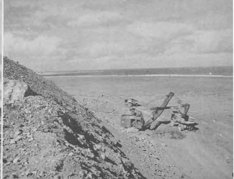
Shovel at work on the Seawall Cut.
