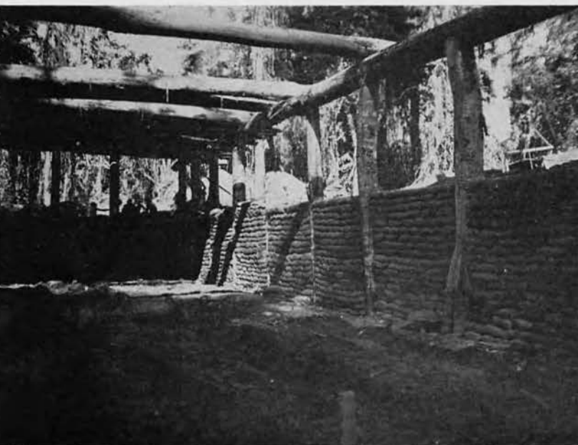
Air Warning Station under construction.
