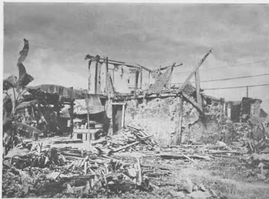
One of the early types of concrete houses in ruins.
