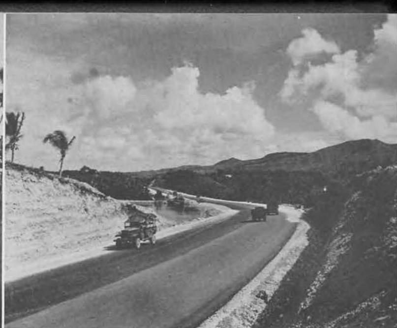
Completed portion on Marine Drive, 1st January 1945. This is a 44' pavement.
