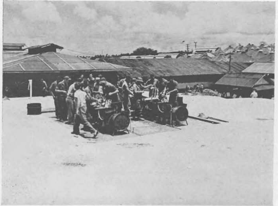
Mess gear wash stands.
