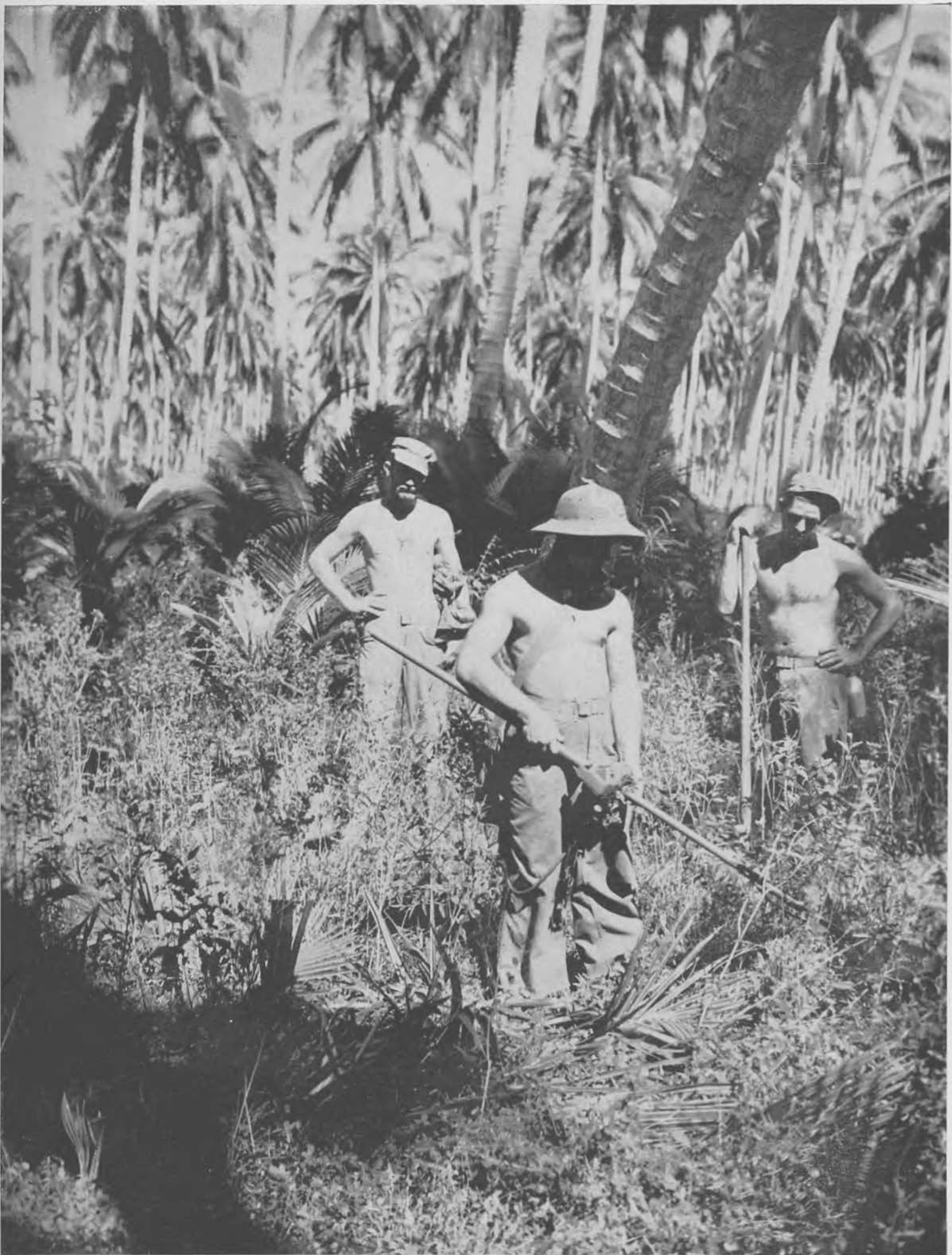
Mine detector being used on proposed road extension, Guadalcanal.
