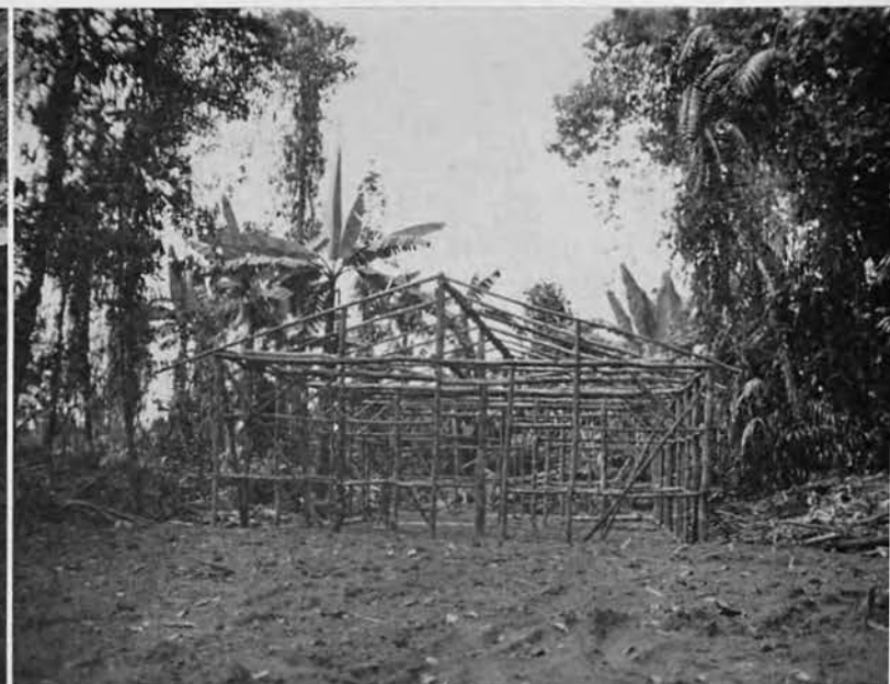
Typical framing to be covered with tarpaulins for operations building on fighter strip.
