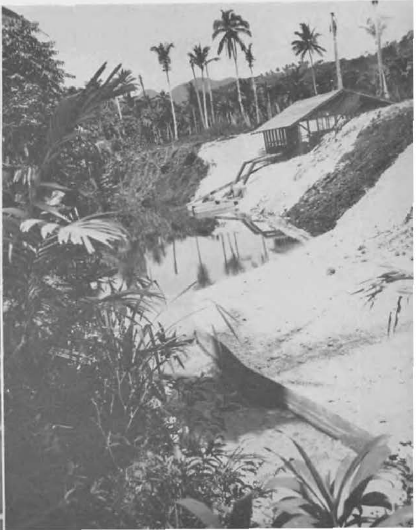
Almagosa water project. This work consisted of the construction of a small dam built with a concrete and sheet piling core; concrete spillway; a pumping station with two additional booster stations; and approximately three miles of 12-inch water main. This system added about 1,500,000 gallons per day to the island supply.
