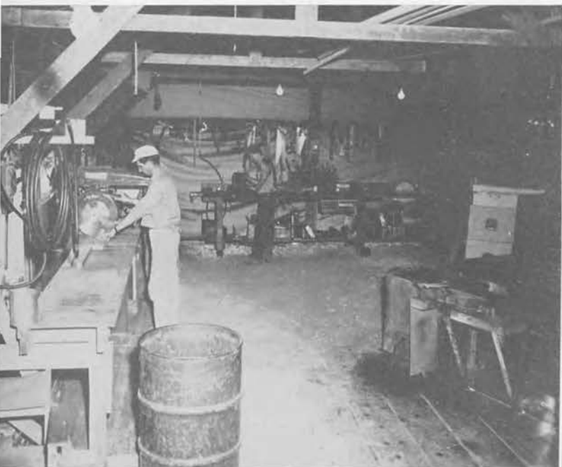
Carpenter Shop—Carpenter, CM1c; Bagette, CM1c; Robert Stout, CM2c.
