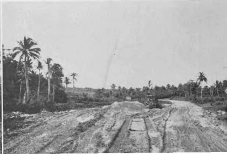
The fill for a road-bed is placed by crews of the 53rd NCB.
