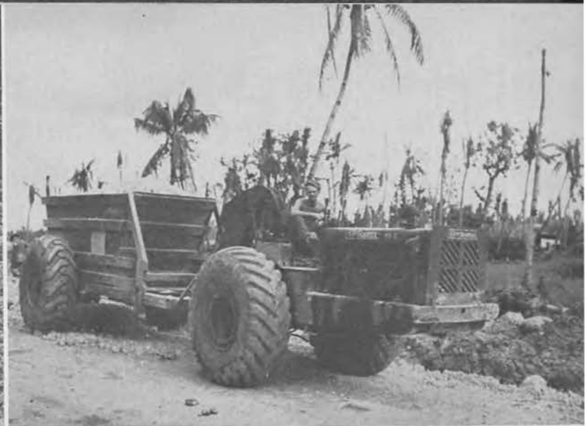
Spreading the coral base course on the Sumay-Piti Road Crocher at the controls of the tourne-trailer.
