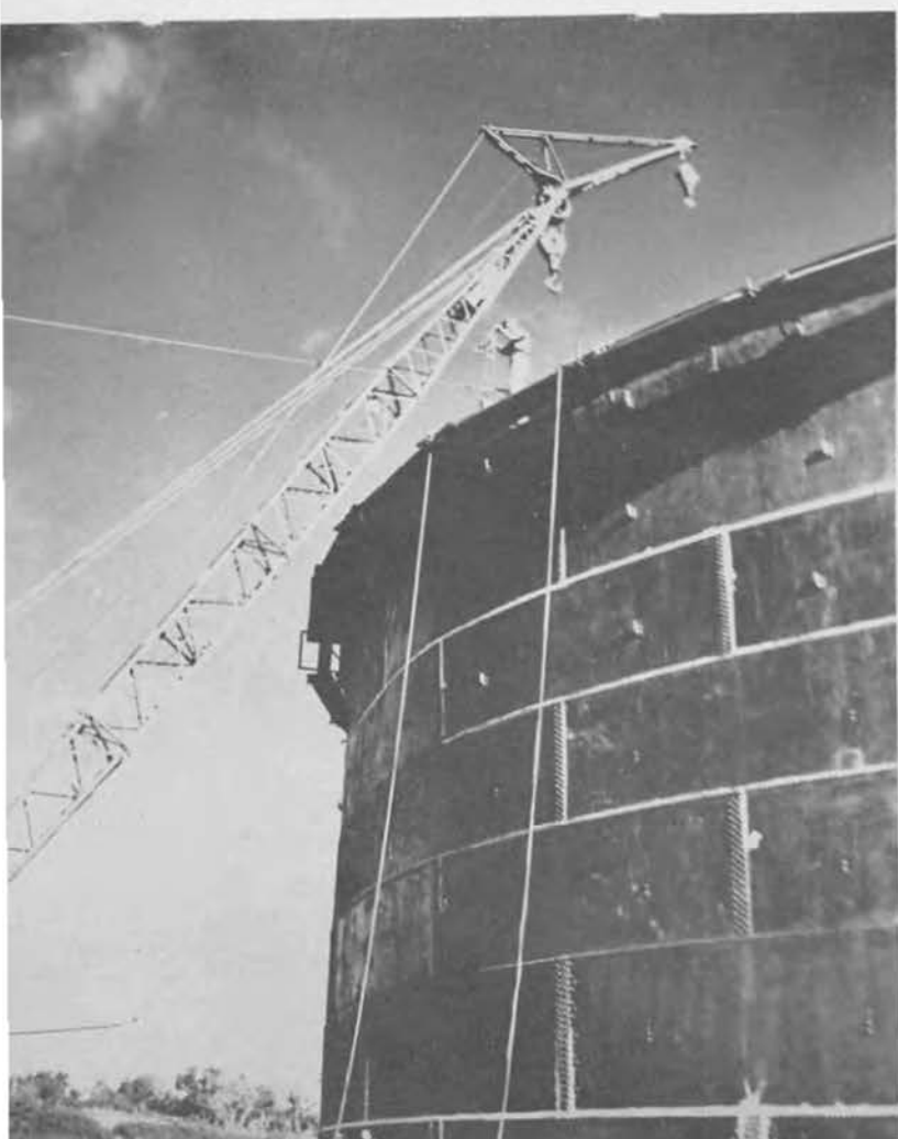
80,000 bbl. tank nearing completion.
