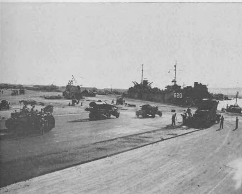
Paving a 100 foot strip at the docks.
