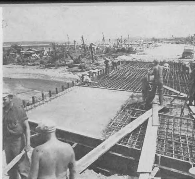
This structure over Anigua River near the Agana Cemetery is a reinforced concrete deck supported on wood piling. Note shattered palm trees in background.
