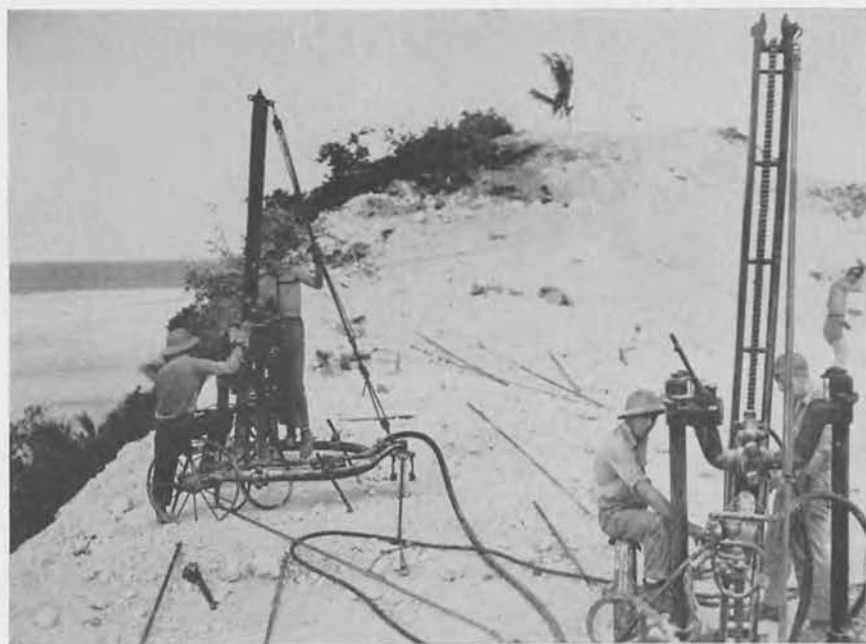
Wagon Drills in initial operations on the 115' Assan Point cut. Approximately 200,000 cu. yds. of excavation came from this site.
