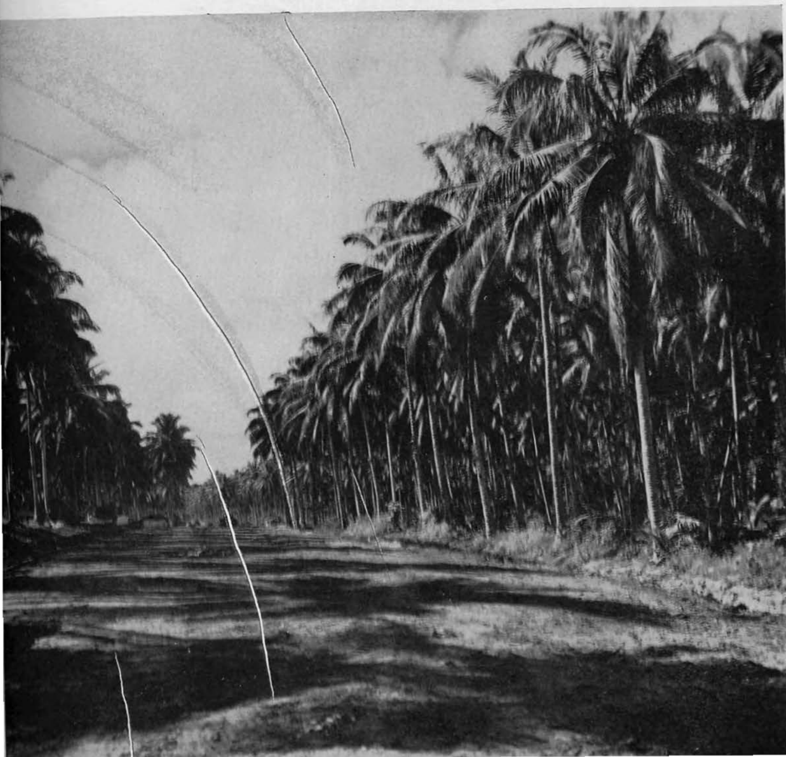
Completed section of road.
