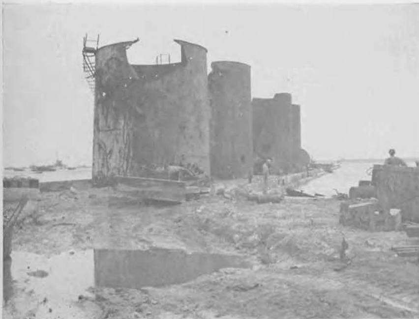
One of the first projects undertaken by the 53rd NCB: cutting down and removing steel (Pan American) gasoline storage tanks at Sumay docks.
