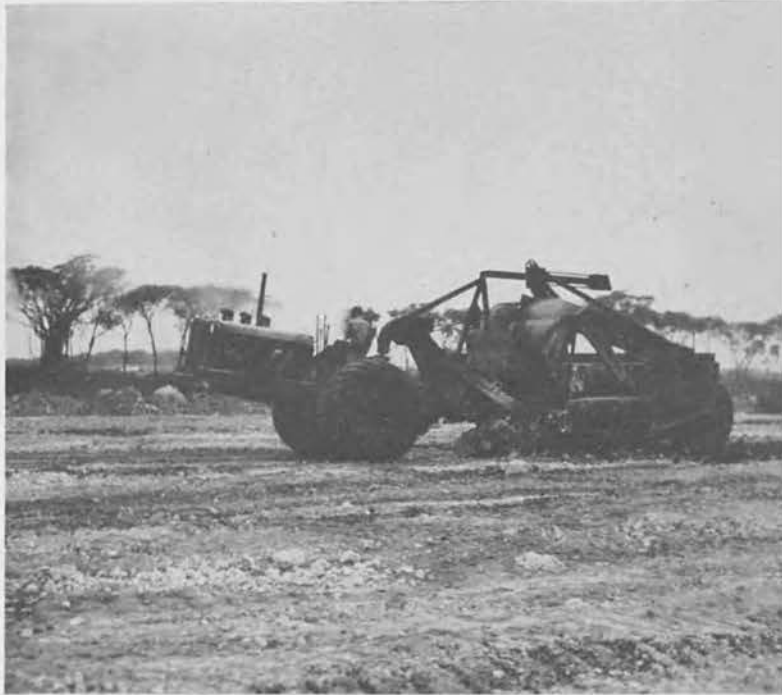
Right, Below: Finish surface grading at N. W. Field.
