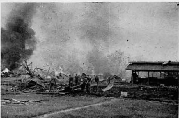
Clearing for central storage area.
