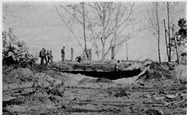
Fifteen-foot earth cover over Japanese communication installation. Note two-foot concrete slab.
