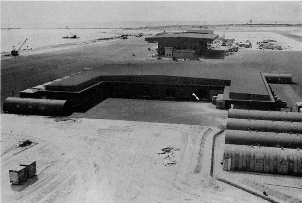
Mail and freight building, John Rodgers Airport, with the huge nose hangar in the background.
