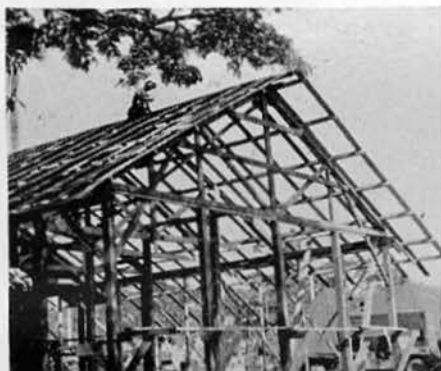
An old shed being converted into permanent galley.
