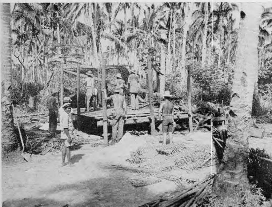
. . . clearing out the heavy growth . . .
