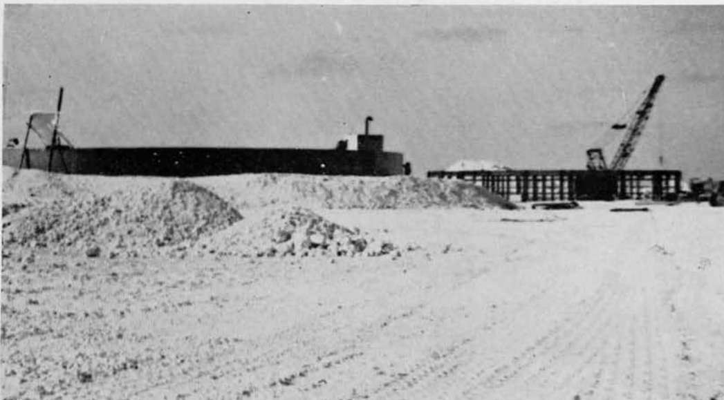
View of one of the completed tanks—second one under construction.
