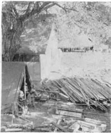
End of galley, plumbers' tent in left foreground.
