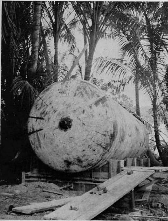
25,000-gallon gasoline storage tanks. Camouflage was no problem on this installation.
