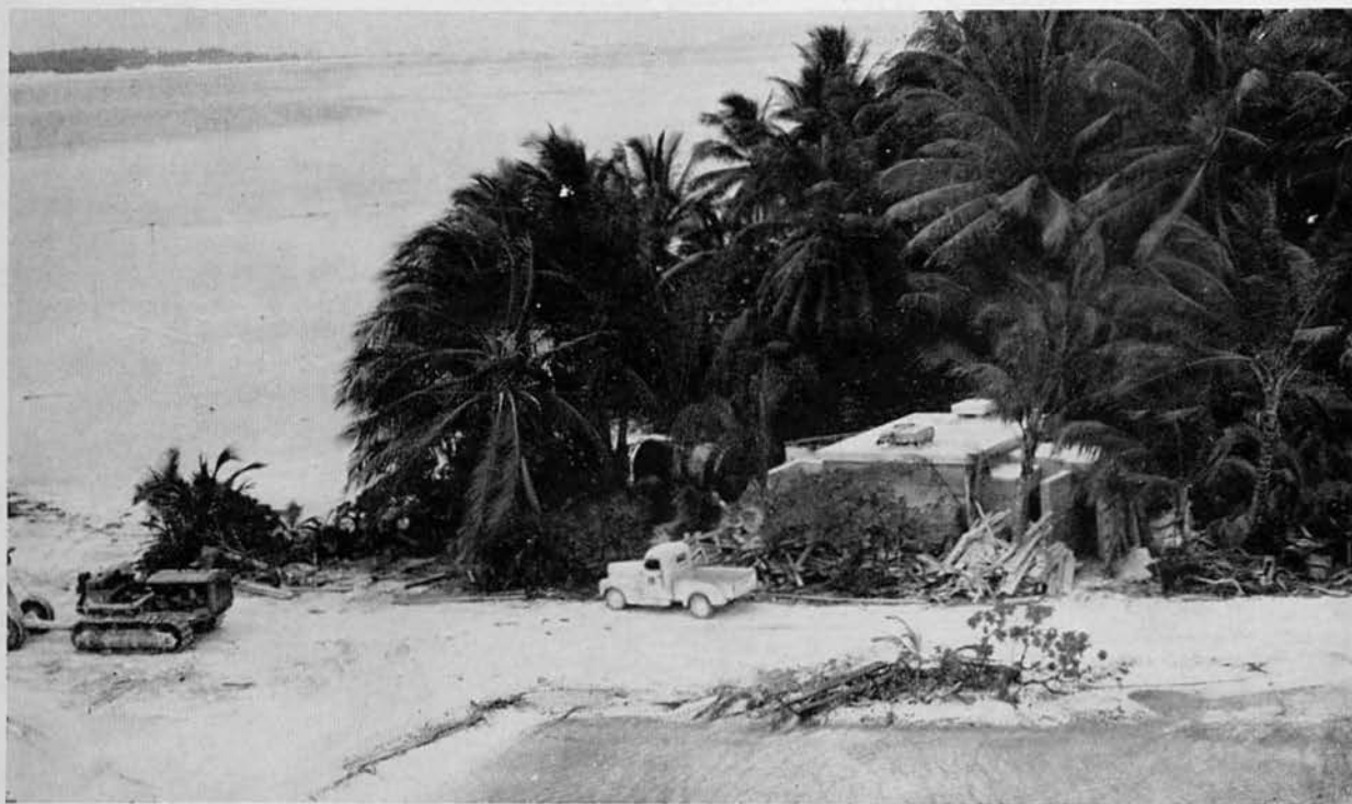
Power station, C.A.A. range.
