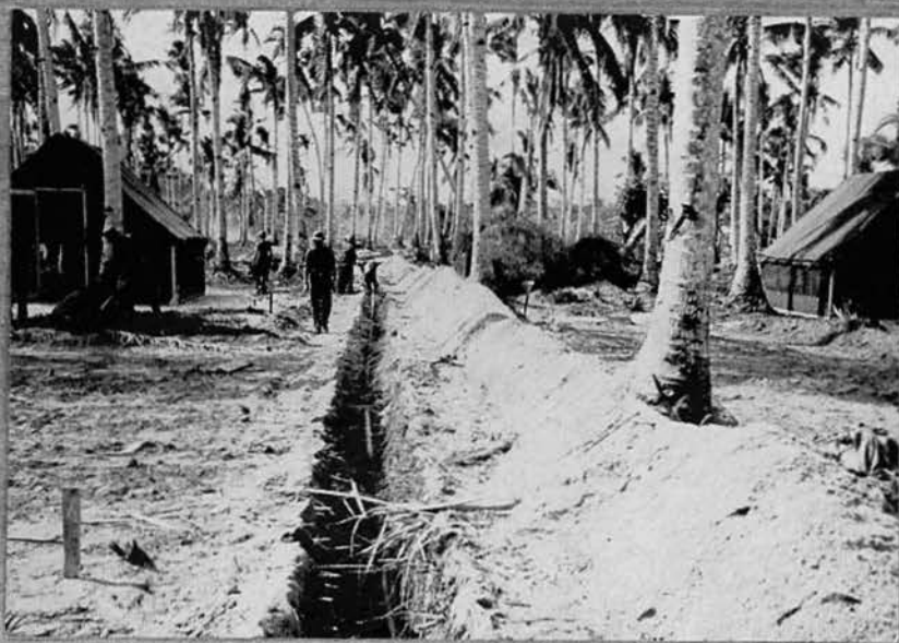
Laying water lines
