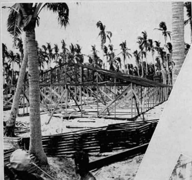
The galley is framed
