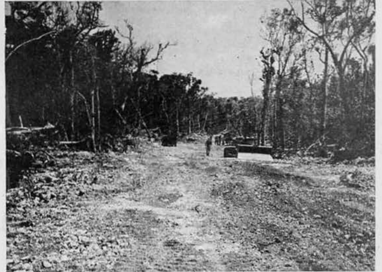
... Clearing road to the camp site ...
