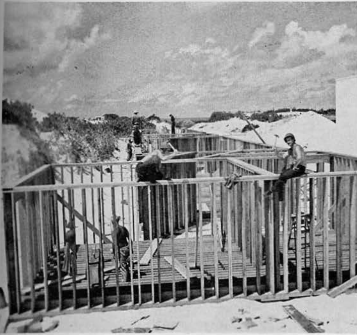
Underground hospital showing framing being raised (left) and roofing being applied just before receiving a ten-foot protective coating of sand (right).
