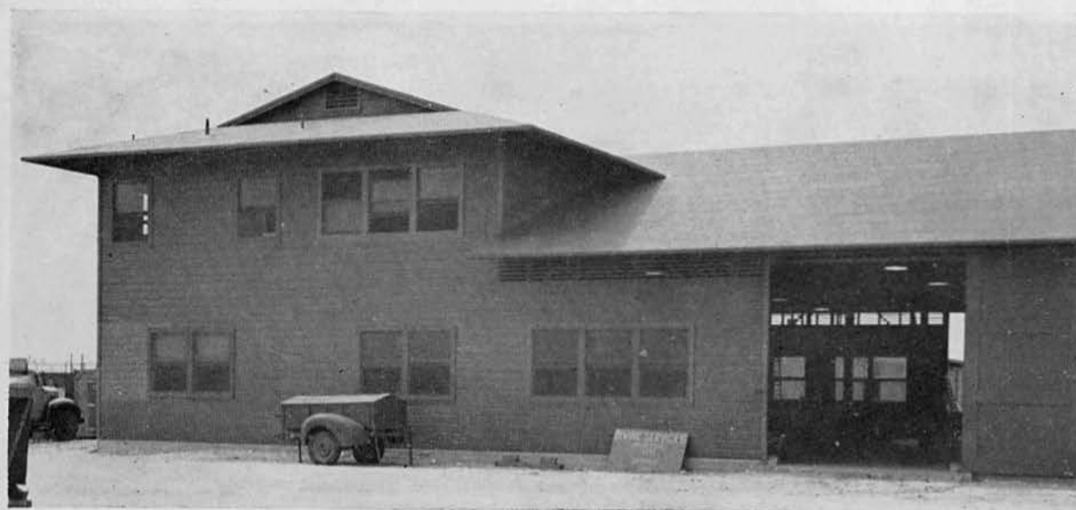
The Public Works Building—the "first structure" to be completed on the construction program. Until taken over by the air station, it was used by the Fifth for shops, disbursing office, warehouse, ship's service, chapel and band rehearsals.
