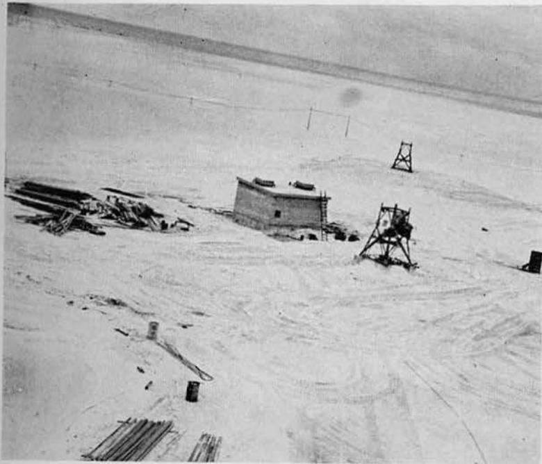
Transmitter station, C.A.A. radio range.
