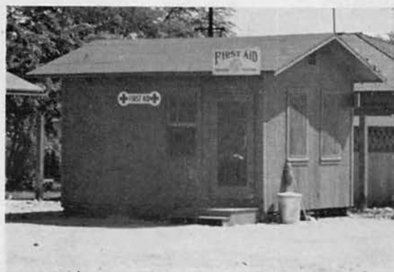
5 NCB Sick Bay. This was the "first building" to appear on the job. It was formerly an old contractor's shack, was remodeled, towed in on skids, and opened for business on the "first day" of operations.
