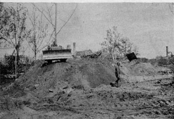
CLEARING FOR HOSPITAL AREA
