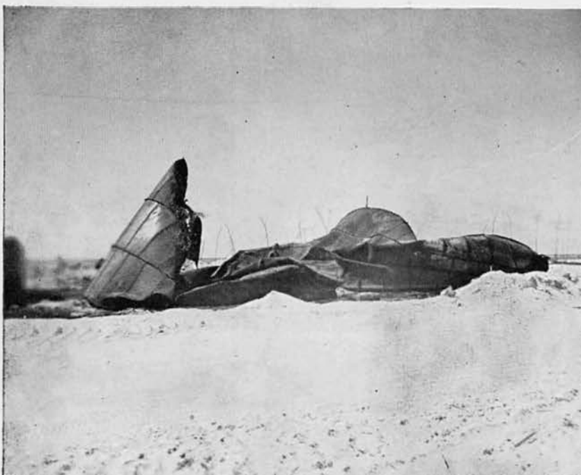
Scenes of destruction left behind after the Battle of Midway. This wreckage and debris had to be removed and new facilities constructed. Top: Hospital; Bottom: Fuel storage tanks destroyed by bomb and shell fire.
