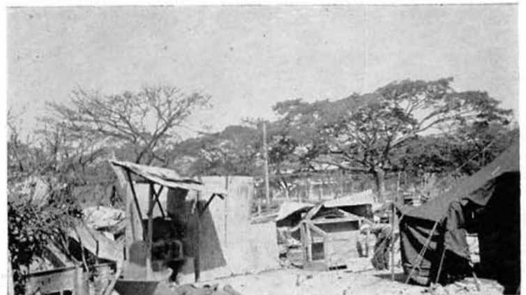
Storage tent near wrecked installations.
