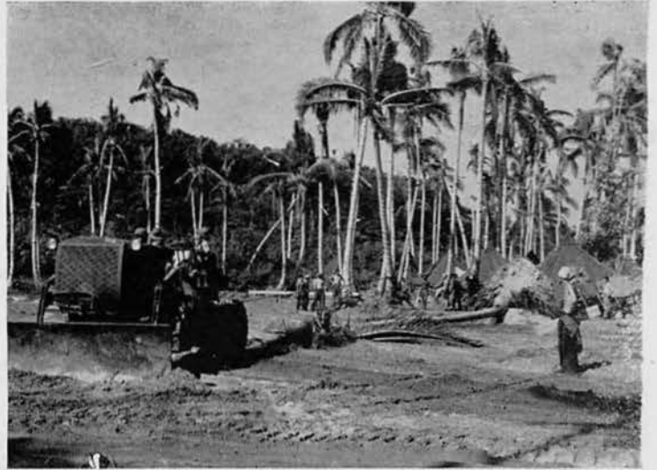
... Bulldozers clear the way ...
