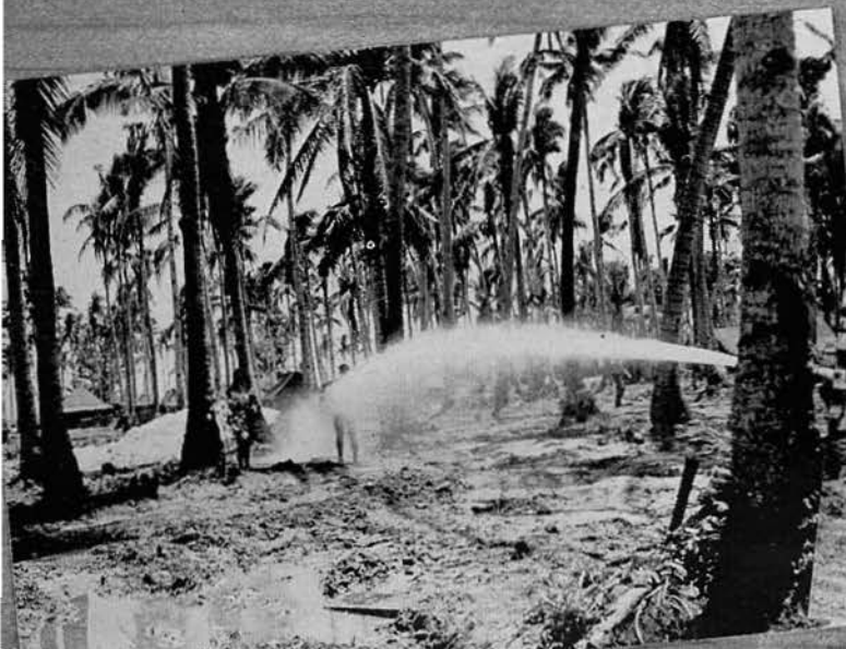
Testing well for volume
