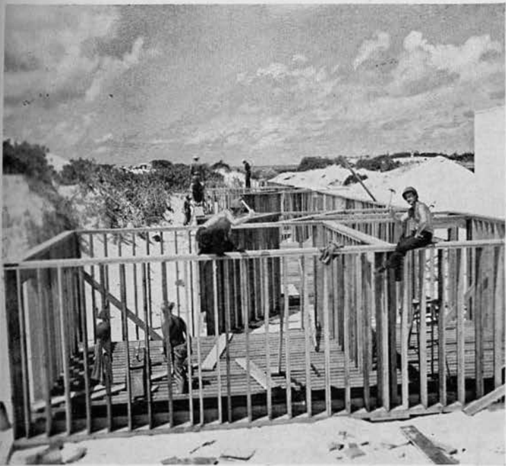
Underground hospital showing framing being raised (left) and roofing being applied just before receiving a ten-foot protective coating of sand (right).
