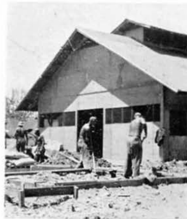
Putting finishing touches on permanent galley.
