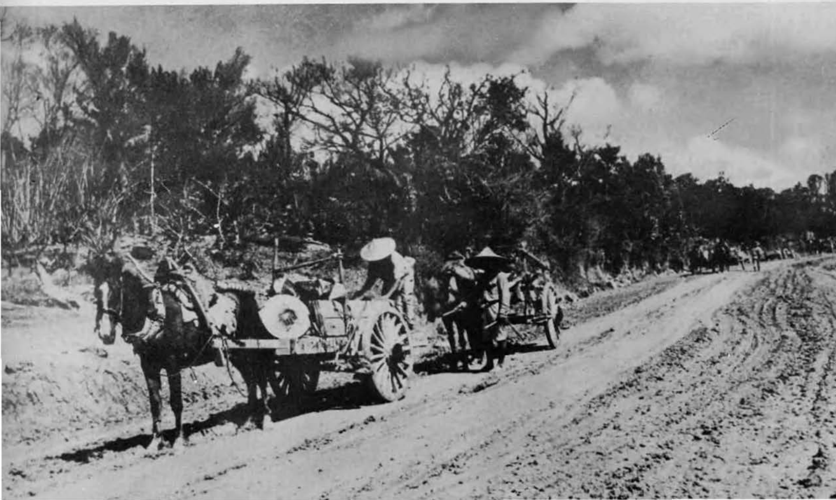
HIGHWAY No. 13 BEFORE OUR CONSTRUCTION WORK BEGAN
