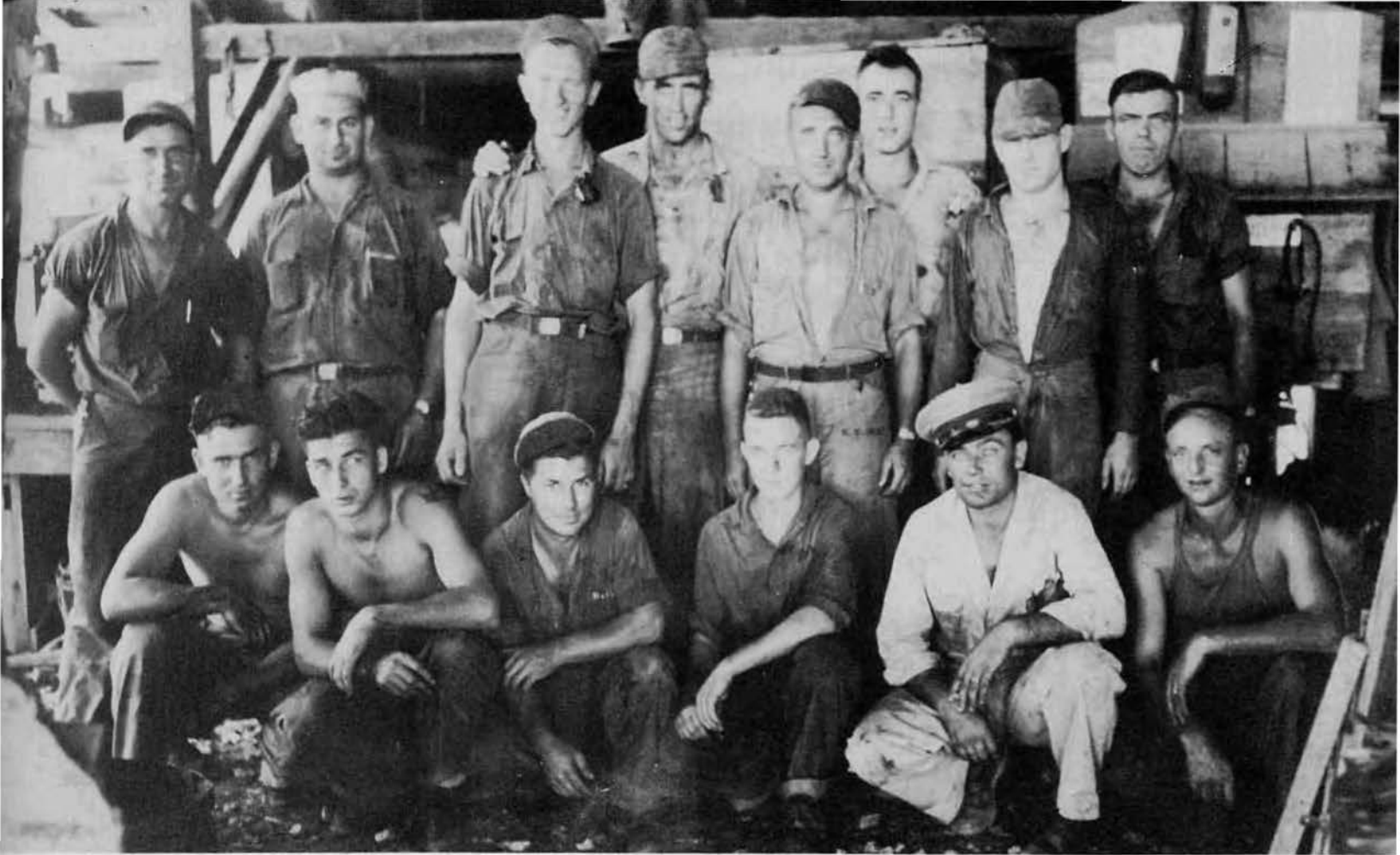
MORE "CAT" REPAIRMEN
