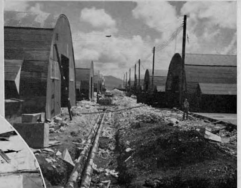
cluded approximately 40 buildings with complete facilities for the overhaul of aircraft, including air, steam, water, electric and sewer.
