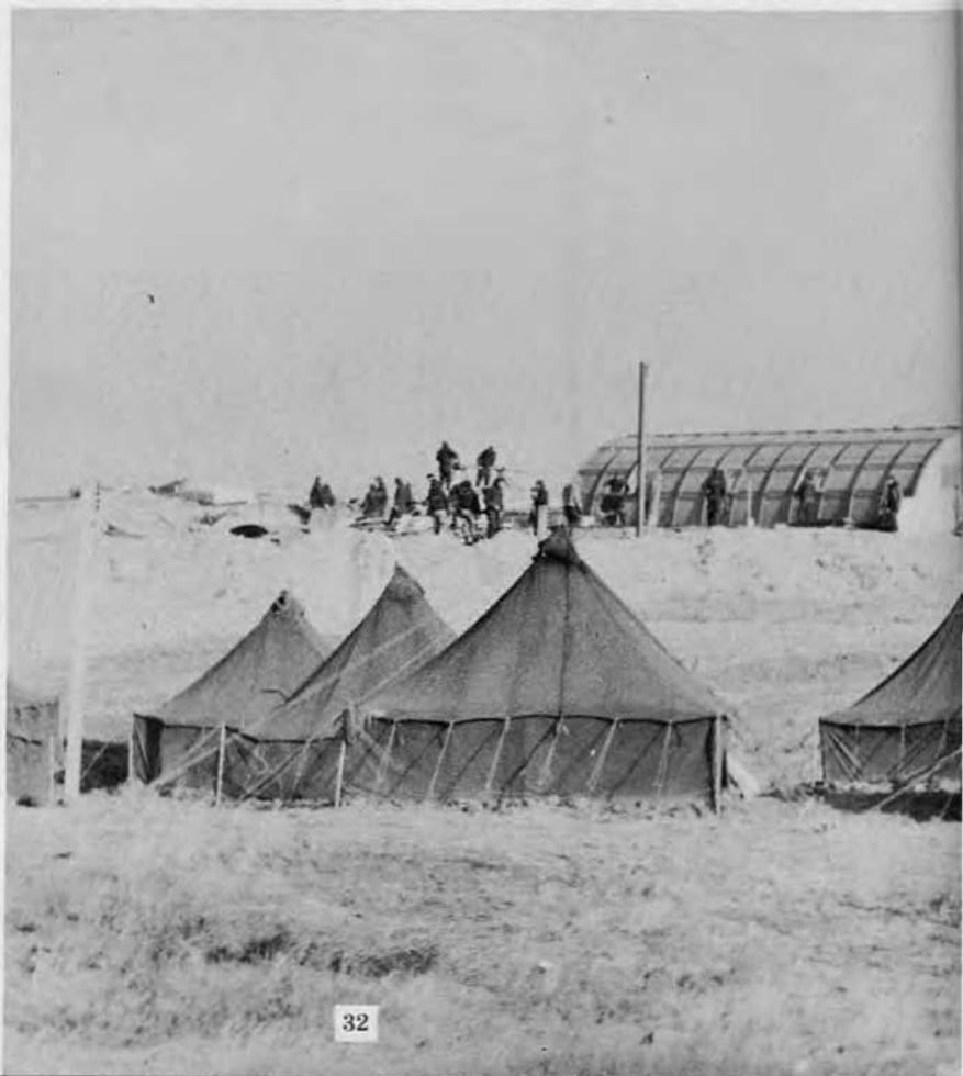
Permanent camp in the background with the Seabee tents in front
