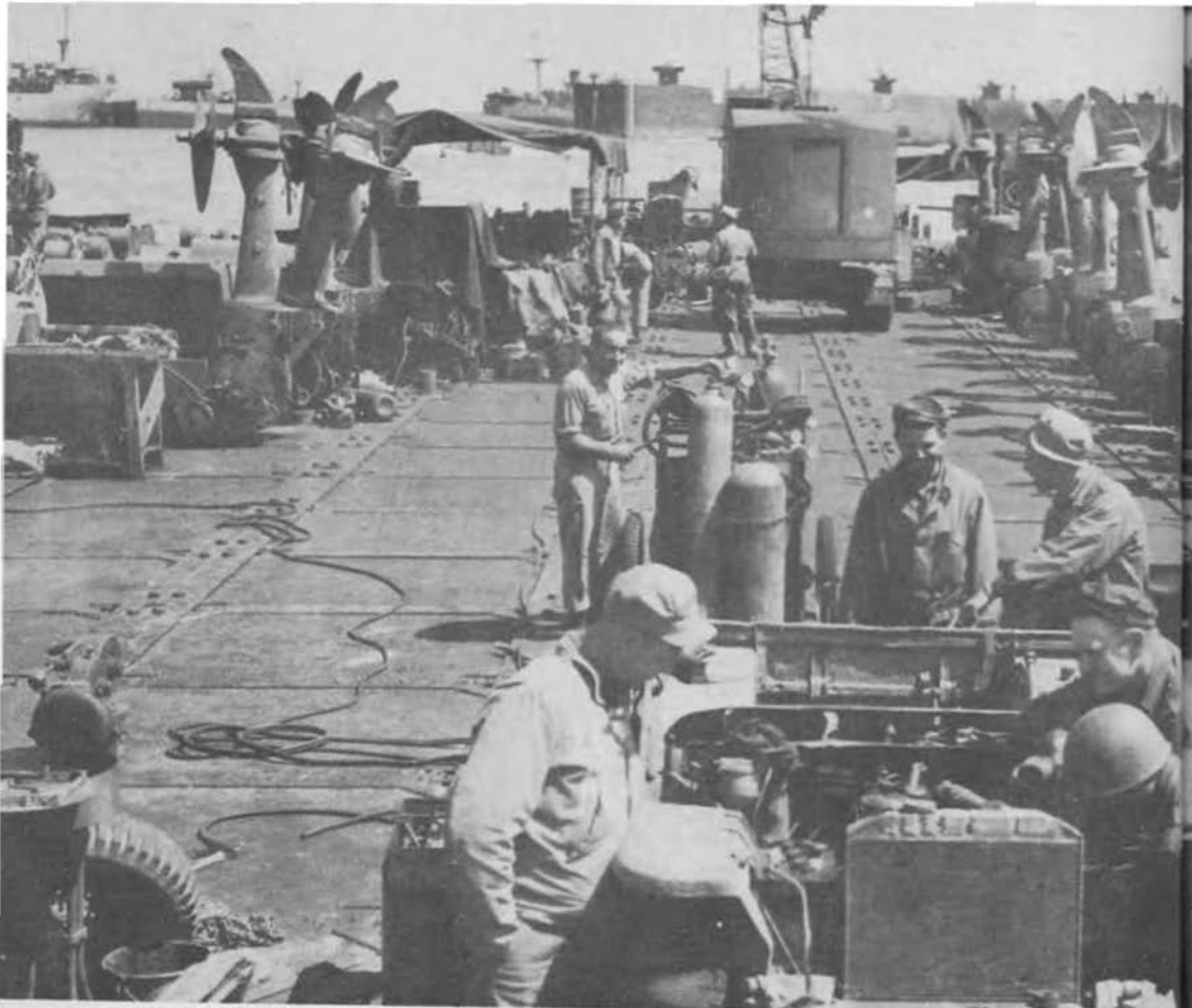
Many of the Supplies were kept on the repair barge deck.
