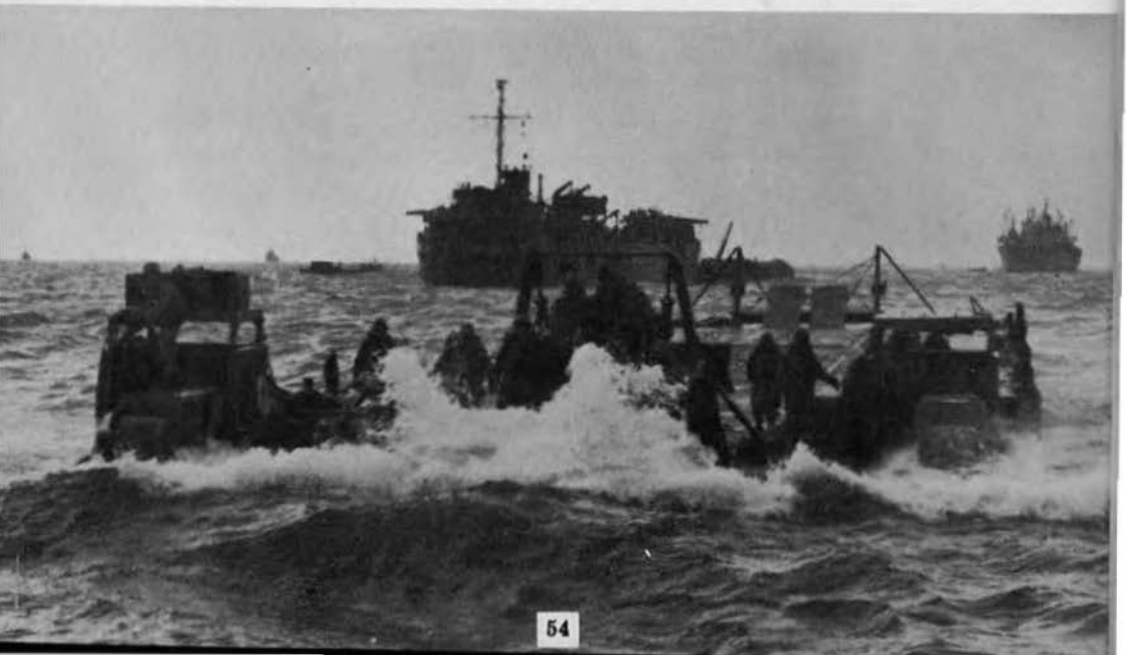
The repair barge was towed from England to maintain operation of the Rhino-ferry
