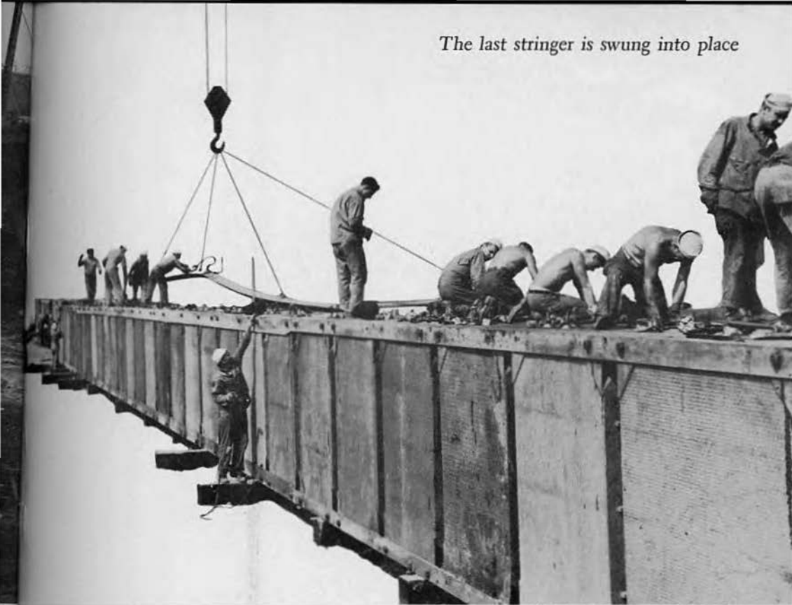
Strings nearing completion
