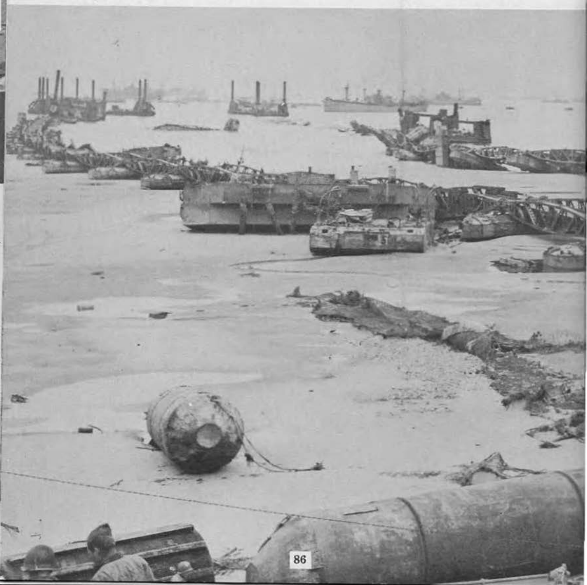
This bridge used to transfer supplies from ship to shore was demolished by the storm June 20
