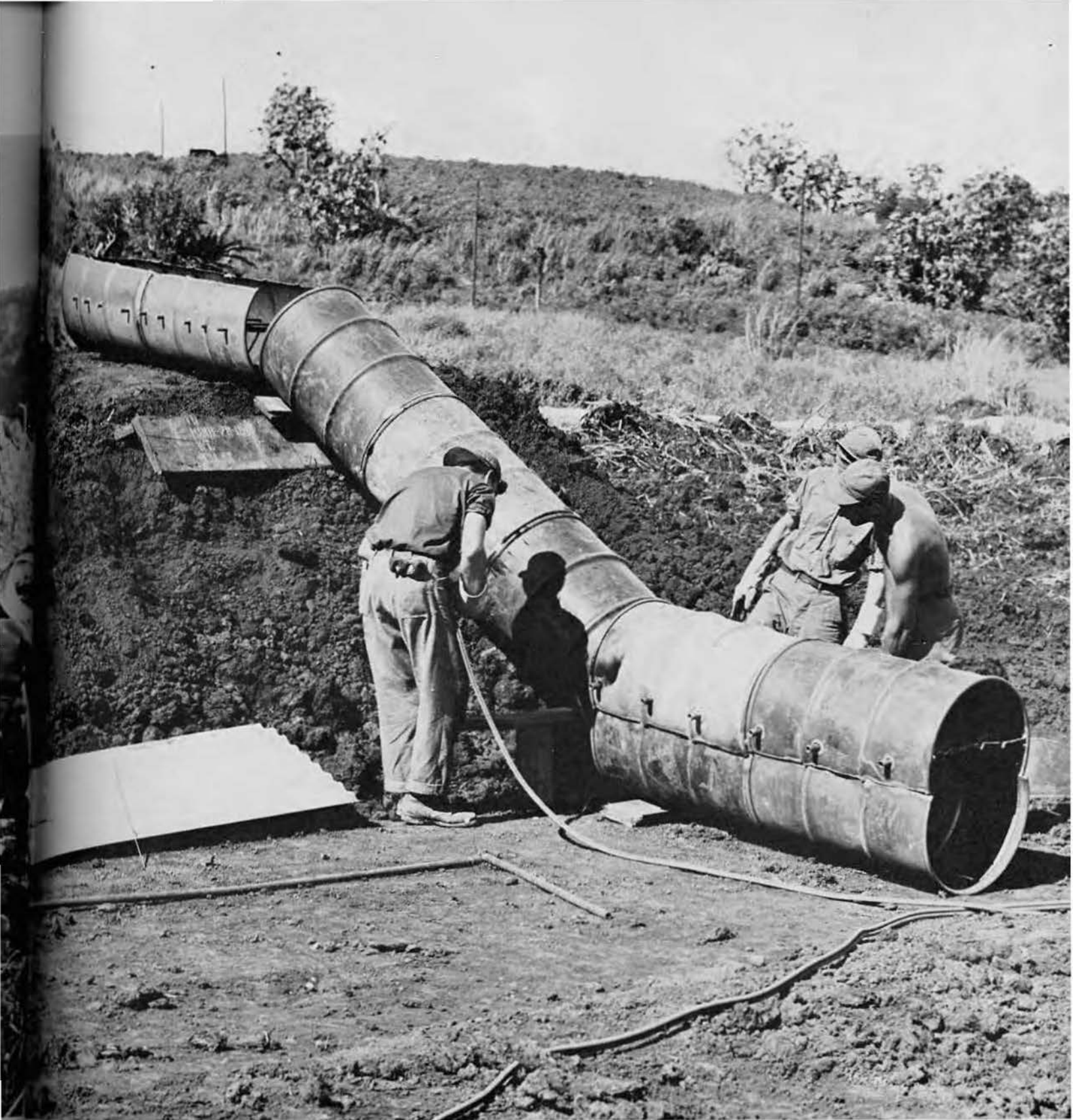
Health precautions demanded an immediate means of refuse disposal . . . our homemade incinerator was ready within three days after landing.
