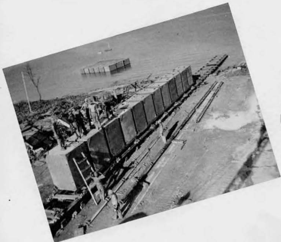
This war's No. 1 invention . . . the much publicized pontoon . . . we used them to construct a floating dock.
