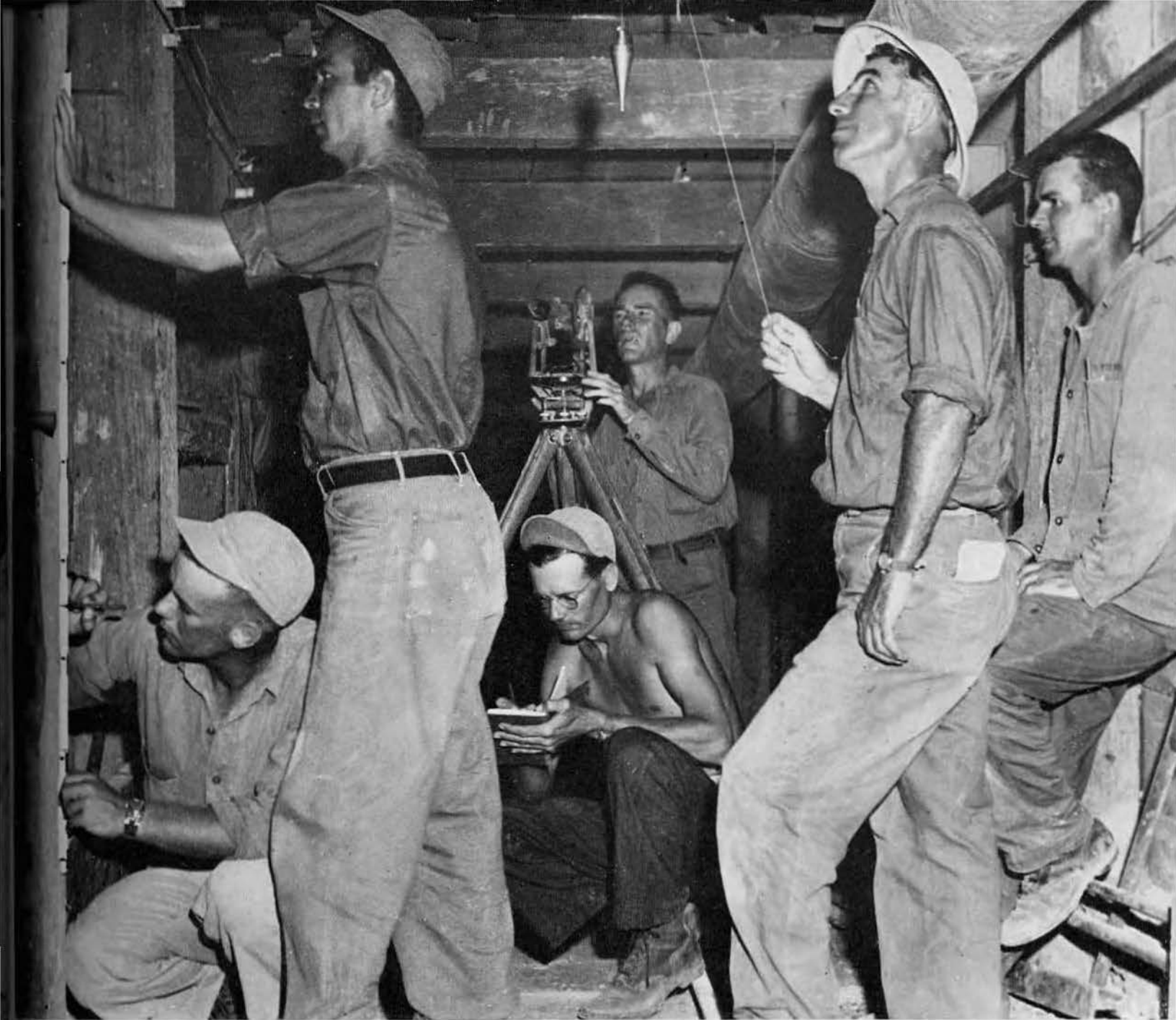
Infinite safety precautions had to be taken in shoring up the tunnel . . . we had to survey the job once in a while to check slope and direction.
