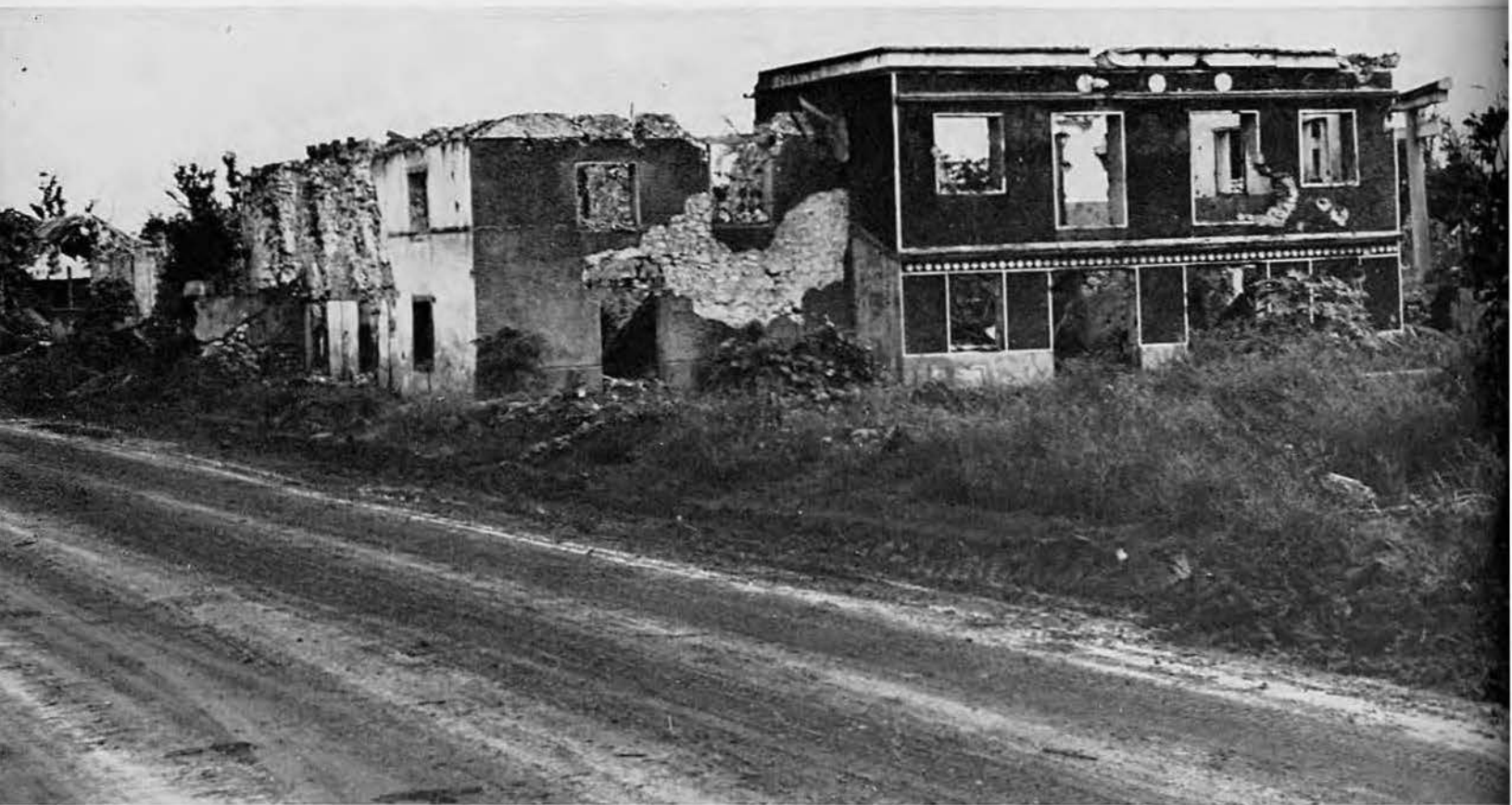
The most modern of the buildings were constructed of brick veneer over a coral cement base.
