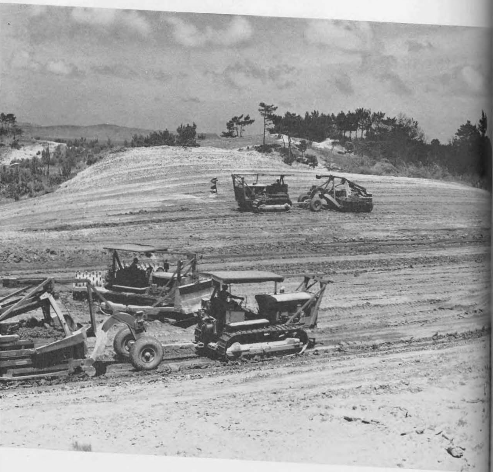
Building roads over the soft, rolling terrain of Okinawa was an easy task after having to hack them out of the hard coral rock of Saipan.
