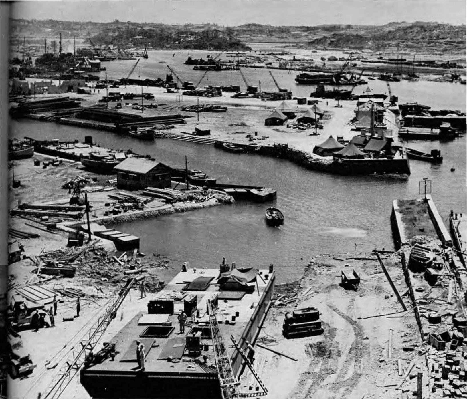
Less than a month after the city had been destroyed, wreckage and rubble had been leveled and channels had been dredged. In place of the buildings of city-fortress Naha, huge American cranes worked ceaselessly in the new Port of Naha.
