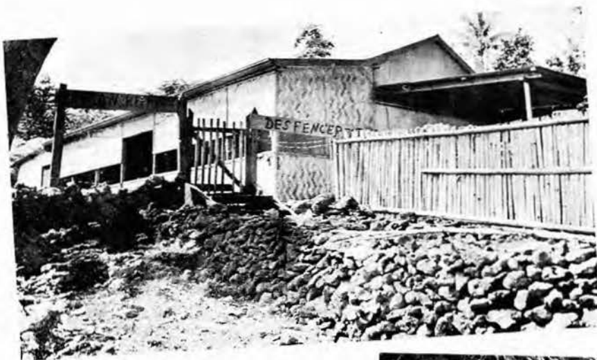
"MAN KEEP OUT", SIGN POSTED AT APPROACH TO INTERIOR VILLAGE
