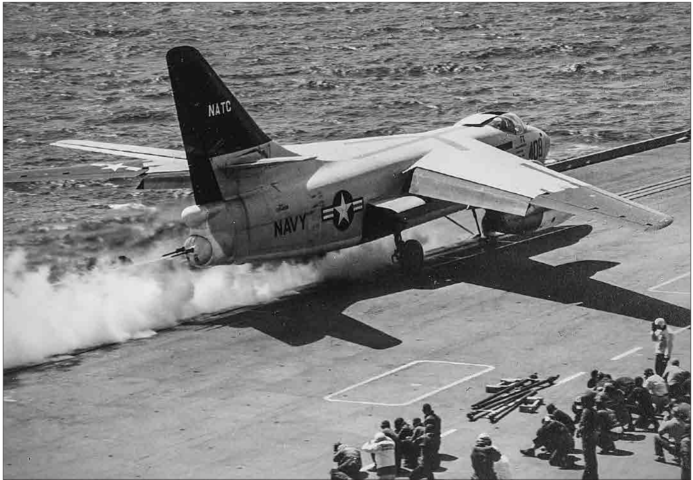
One of two A3D-1 Skywarriors, BuNo 135408, used for Naval Air Test Center carrier suitability trials in June 1956 is launched from Forrestal (CVA 59).
