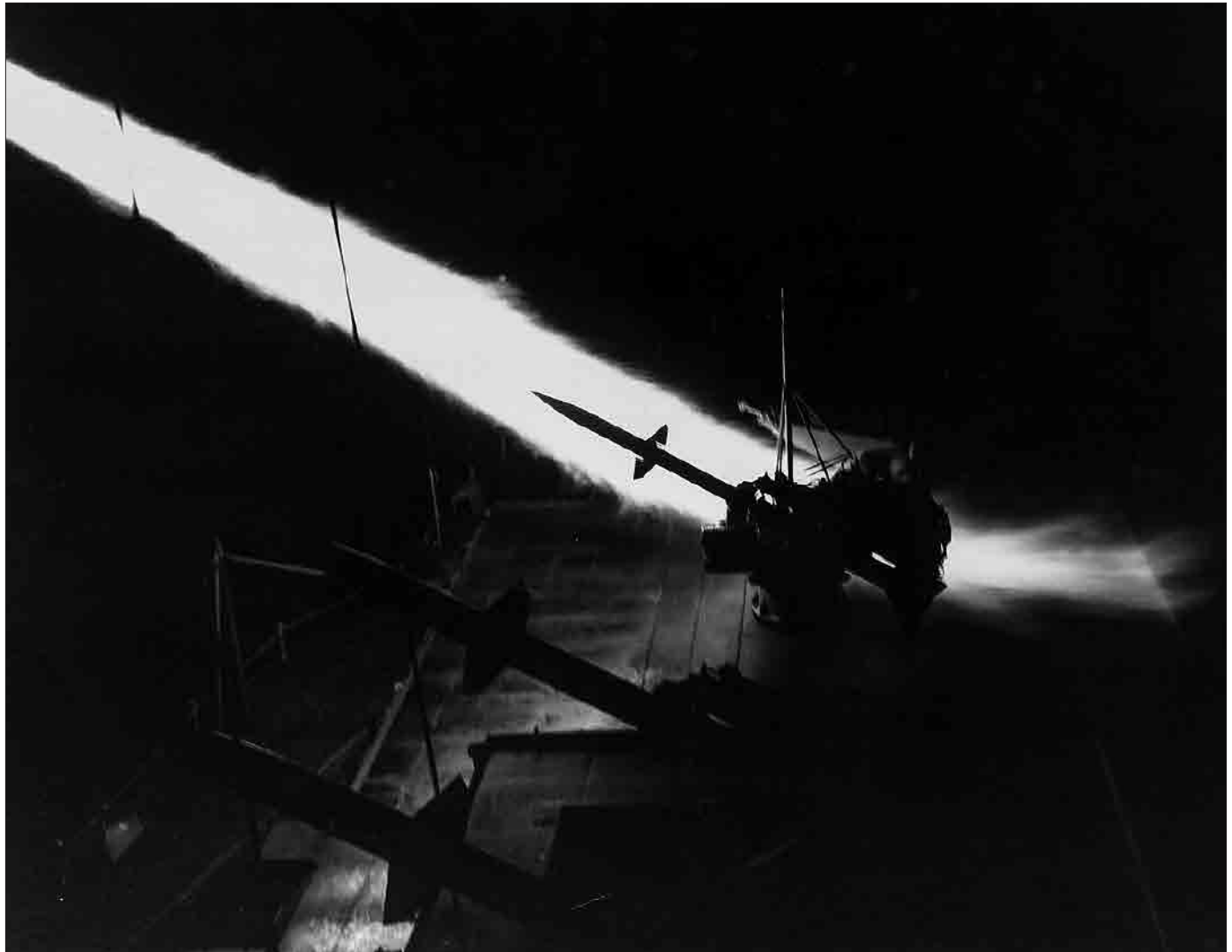
Converted battleship Mississippi (AG 128) first launched a SAM-N-7 Terrier surface-to-air missile during tests in January 1953. This is a later night launch.
