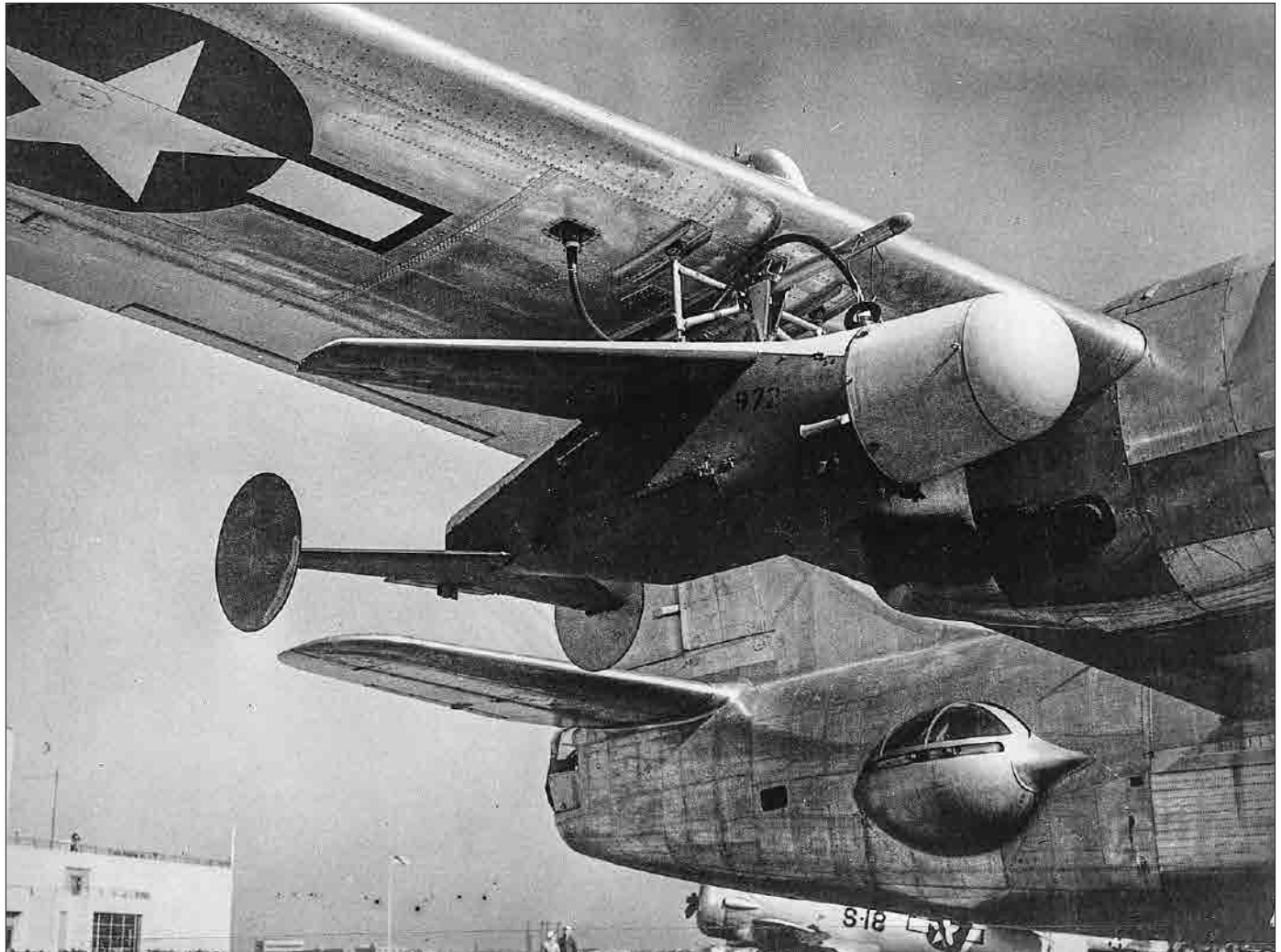
A Bat radar-guided glide bomb is mounted under the wing of a PB4Y-2 Privateer. The weapon carried an internal 1,000-pound bomb.
