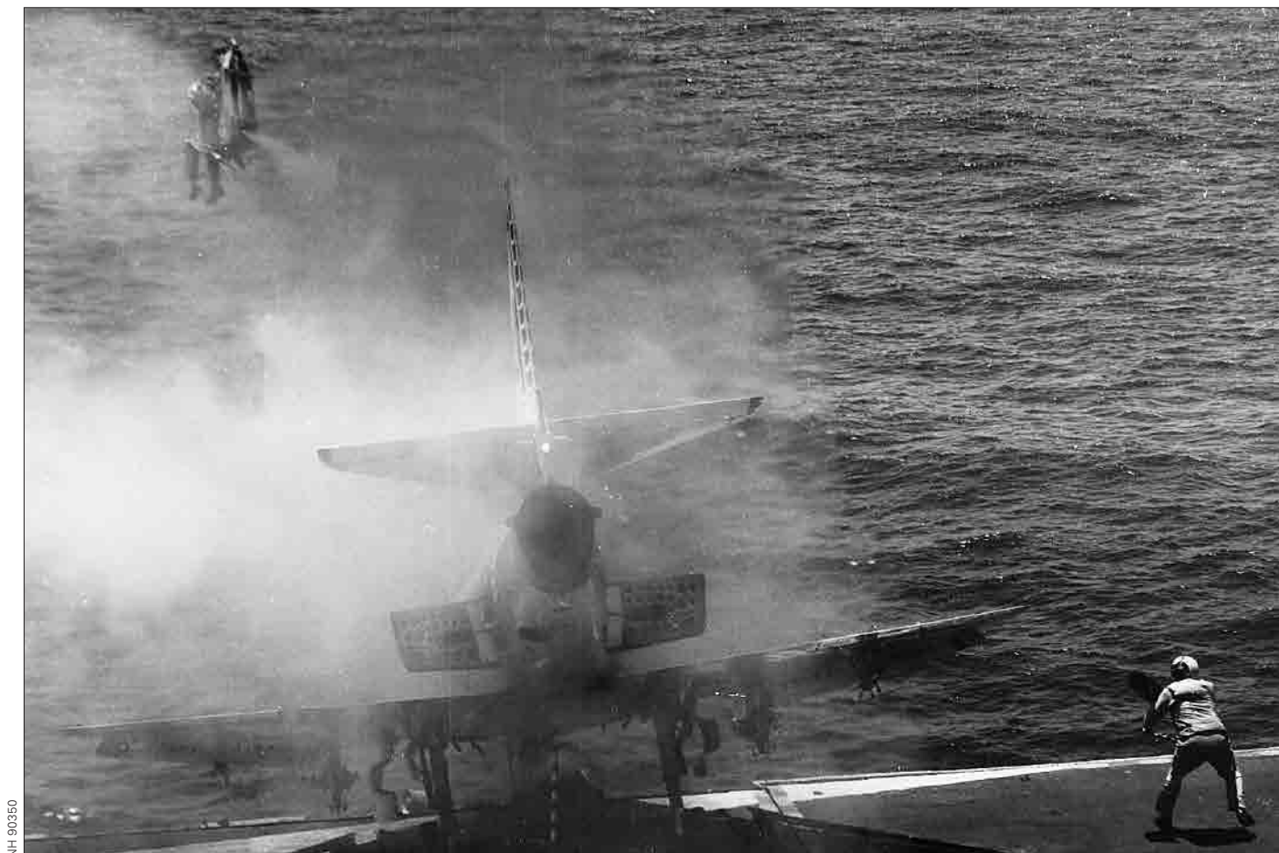
Lt. j.g. William Belden safely ejects from A-4E Skyhawk, BuNo 150117, as it rolls into Shangri-La's (CVS 38) port catwalk after suffering a brake failure following recovery, 2 July 1970. The A-4E was assigned to VA-152 of Carrier Air Wing 8.
