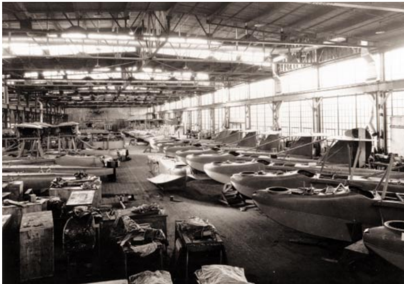
HS-1s under construction.
