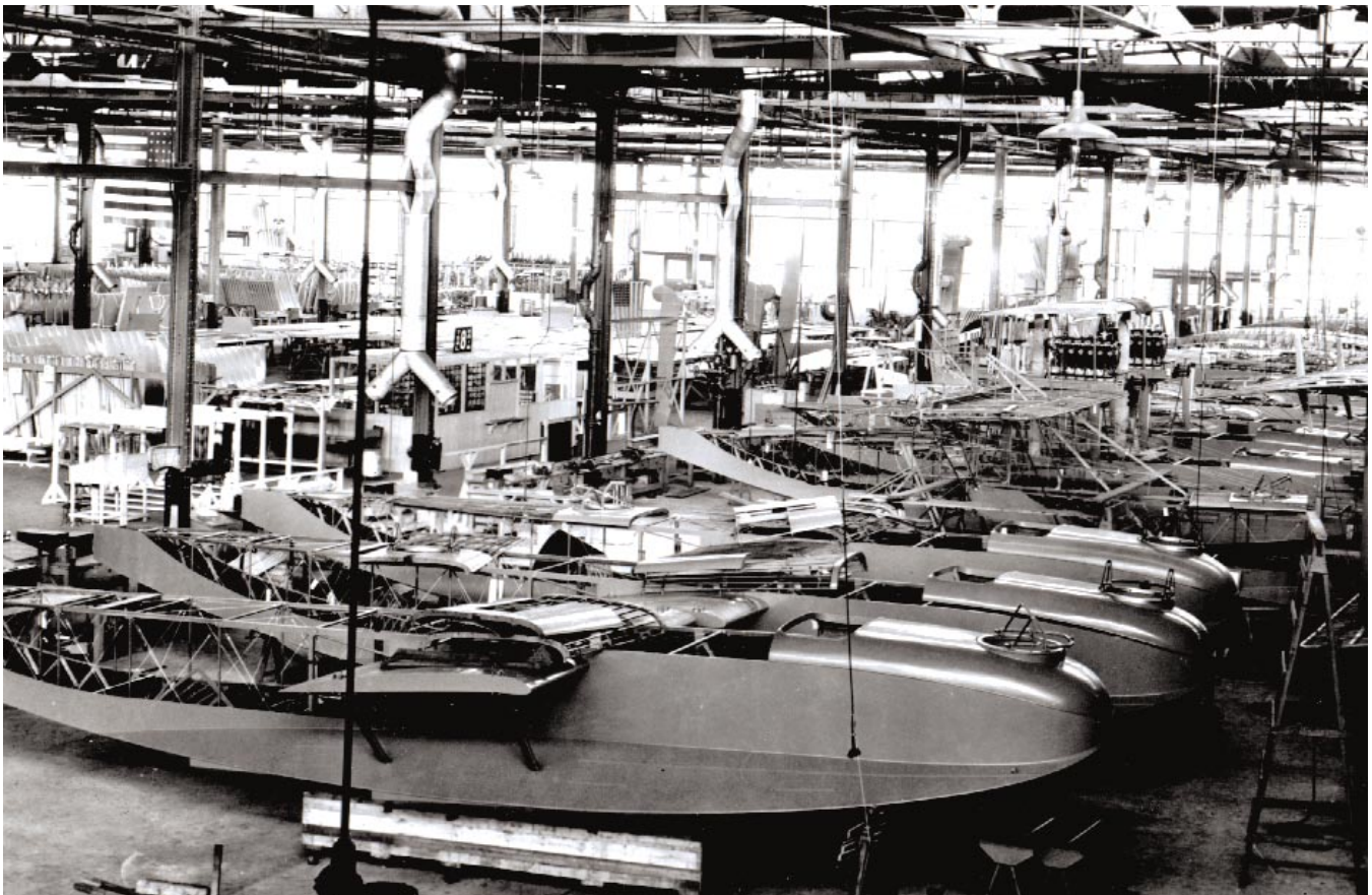
F-5Ls on the assembly line.
