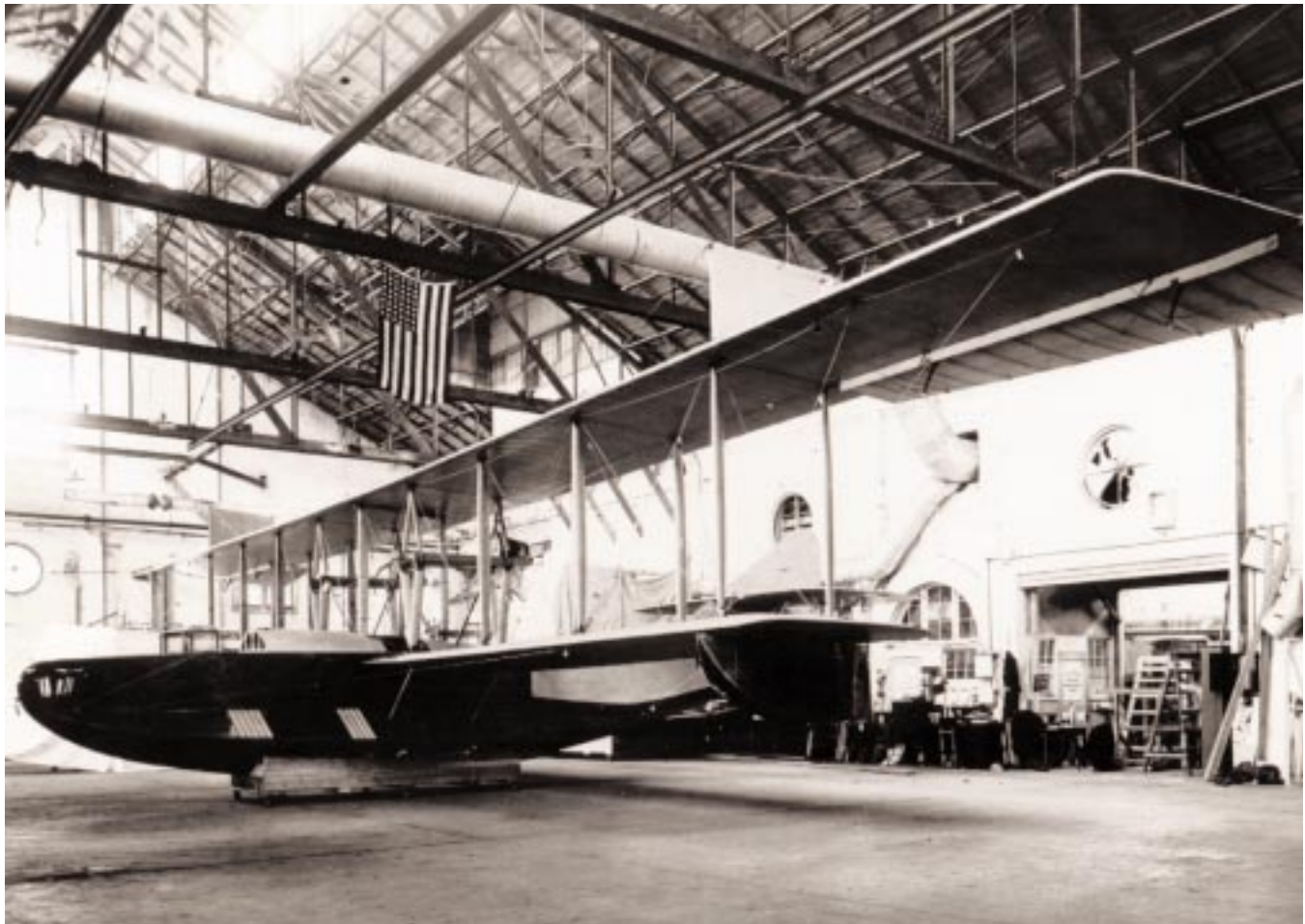
An H-16 under construction at Curtiss Aeroplane and Motor Corporation.
