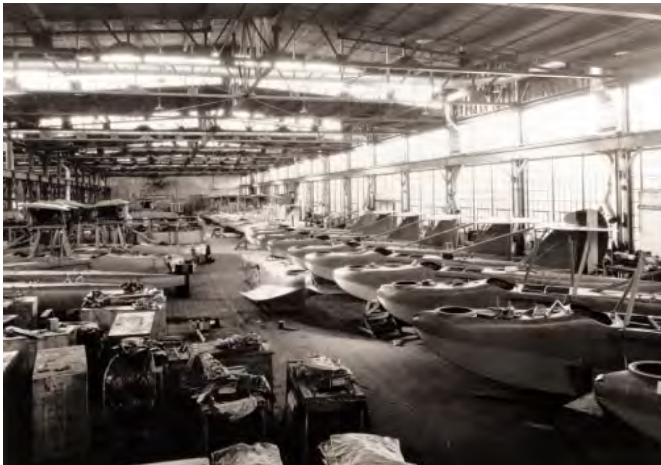
HS-1s under construction.
