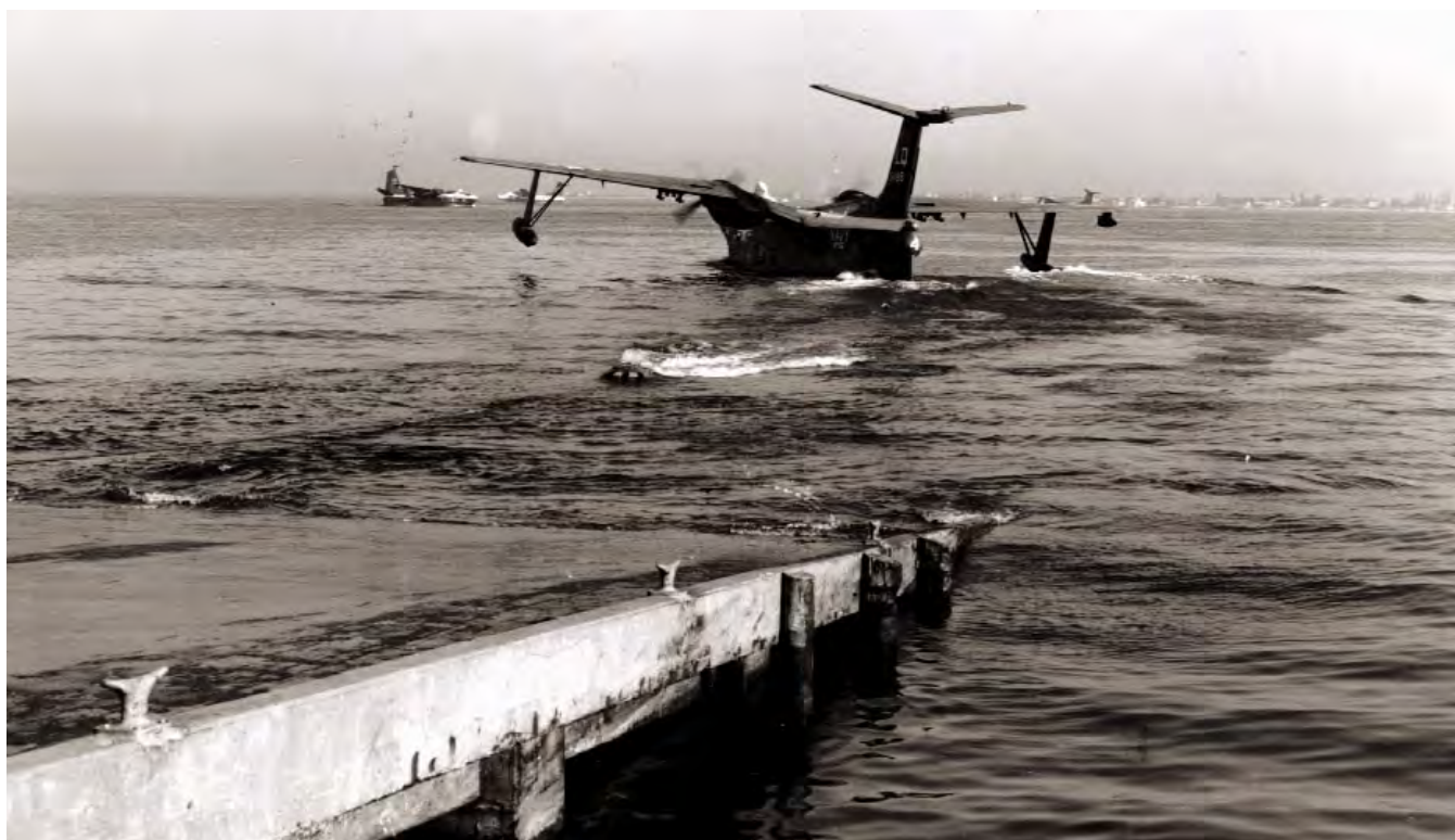
A squadron P5M just after launching from the boat ramp.
