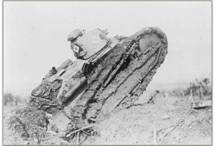
Tank forging through a trench
