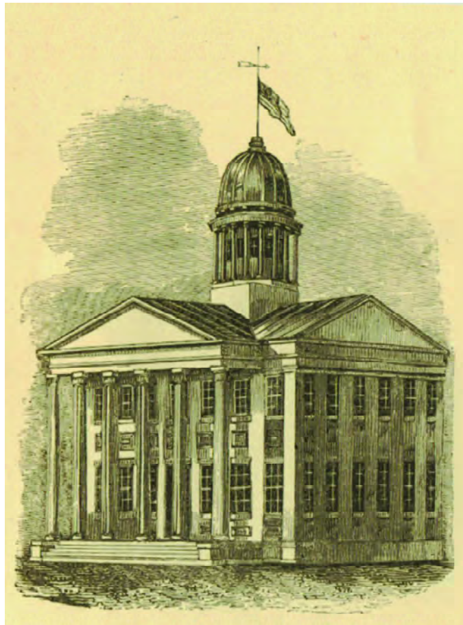
The brand new Norfolk City Hall served as the home for the regional Federal district court for several years and was the site of the trial of the William G. Lewis and her crew. Christened in 1850 as the "worshipful court for the City of Norfolk," the building is now a memorial and museum to General Douglas MacArthur. (1853 engraving from William G. Forrest's Historical and Descriptive Sketches of Norfolk and Vicinity)
