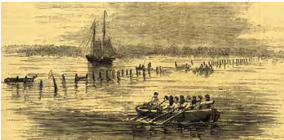
To prepare for a possible Federal assault on Roanoke Island, Lynch had wooden poles staked across Croatan Sound between the north end of the island and the mainland. (London Illustrated Newspaper engraving)
