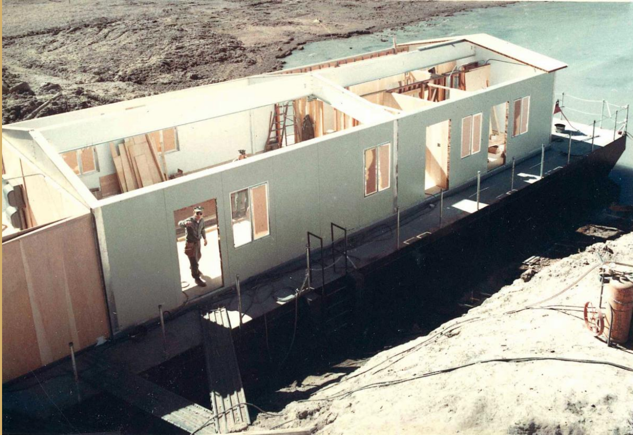
Seabee Team 7412 members constructing prefabricated building on AMMI pontoon, 1972.
