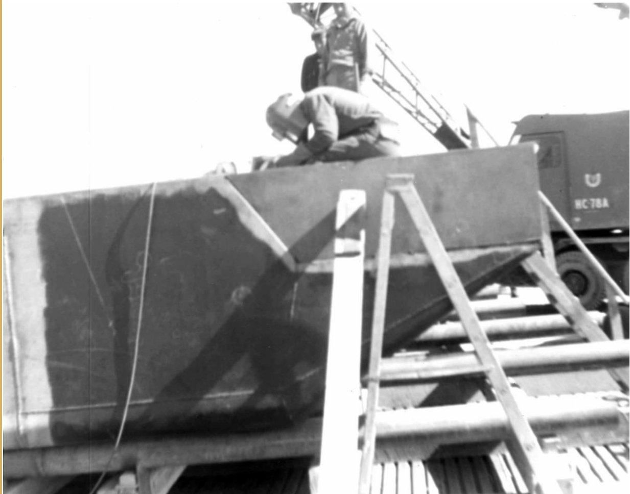
AMMI Pontoon Repair
