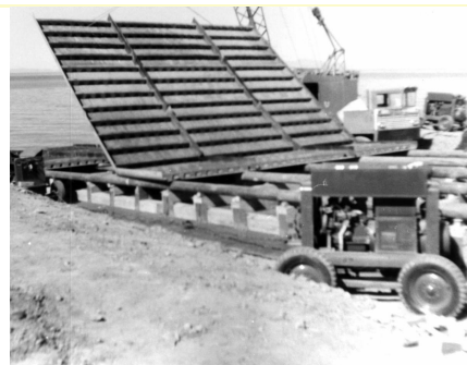
Placing base for AMMI pontoon onto ramp, June 1972
