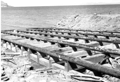
Matting and launching ramp rails, Puerto Chaguaya, June 1972
