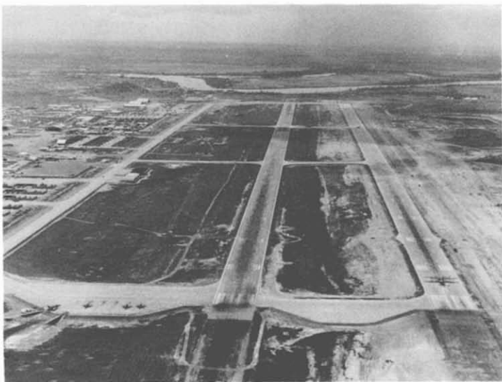
12. Bien Hoa Airfield. Located about 15 miles northeast of Saigon. Bien Hoa was the only military airfield in Vietnam prior to 1965. A 10,000' concrete runway and taxiway was built by RMK in 1963. A parallel 10,000' concrete runway was added in 1967.
