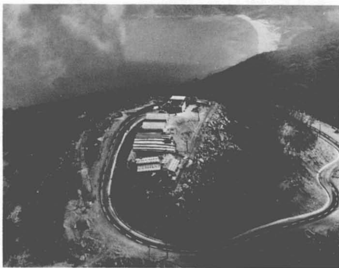
56. ACTOVRAD Site—Da Nang. Among the final projects built by RMK-BRJ was a series of ACTOVRAD (radar) sites strung along high points of the South Vietnam coast and the peaks of nearby islands. This site is atop Monkey Mountain.
