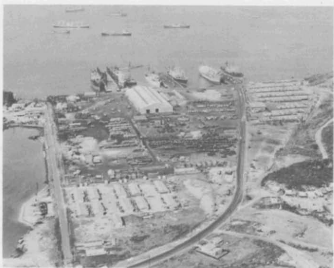
2. Observation Point (Da Nang) Port Facility—September 1969. Complete and fully operational. Note the DeLong mobile pier on the left, and the containerization storage/staging area to the right.
