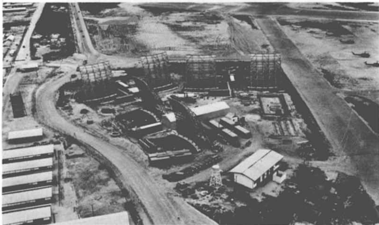
60. Communications Facility—Nha Trang. In June 1965, RMK began construction of antenna foundations and support buildings for this communications facility at Nha Trang; in July, construction was begun on barracks and messing facilities for U.S. Special Forces. The foundations were completed in July 1965; the cantonment, in January 1966. The electronic phases of the installation were accomplished by Page Communications. Nha Trang was a terminal for voice submarine cable from the Philippines, and a link in a tropospheric scatter radio system.
