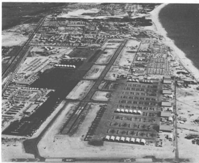
15. Marble Mountain Air Facility (MMAF)—Da Nang. This was a light plane and helicopter airfield. The original runway was 2,000 feet, built of Pierced Steel Plank (PSP). The PSP was subsequently replaced with an asphaltic-concrete wearing surface. The parking aprons were of PSP and measured 135,000 and 45,000 SY each.
