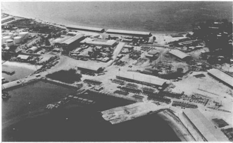
59. Fabrication Yard—Poro Point. Poro Point is located 180 miles north of Manila, on the west coast of Luzon, Philippines. An assembly-line type of operation was employed throughout the length of the Yard. Prefabricated pier and bridge units were fabricated on these assembly lines and railway wheel trucks were used to transport the completed units to the load-out pier, where they were placed on barges for transport to Vietnam. The jacket-templates made at Poro Point were used to build the marine terminal facilities at Newport and the bridges at Da Nang and Cam Ranh Bay.
