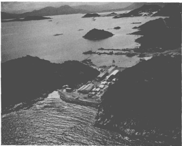
26. MARKET TIME Facility—Cam Ranh Complex. "Market Time" is a coastal patrol operation. There were 6 such installations along the South Vietnam coastline, all relatively self-sufficient. They consisted basically of repair and maintenance shops, floating drydocks, pontoon piers, crane pads, POL storage, utilities, and roads. This is the Market Time site at Cam Ranh Bay.
