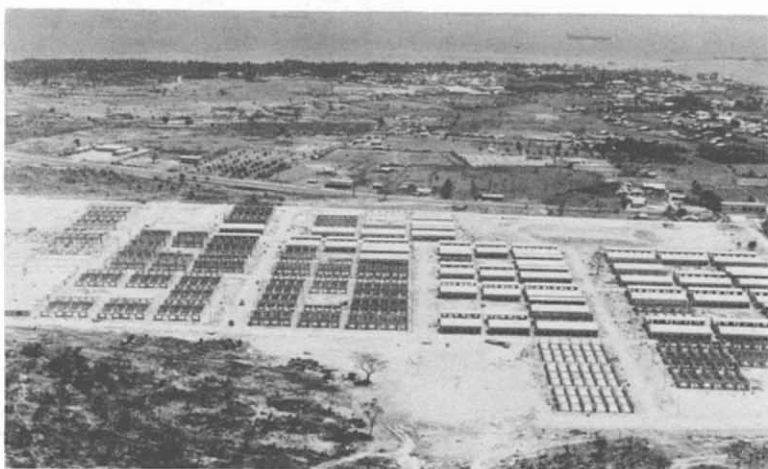
28. USAID Housing at Cam Ranh Complex. Construction of Community Housing at Cam Ranh Bay for Vietnamese tenants. Included in the Project were an Administrative Building, Fire Station, Elementary School, and Market Building; also, sewage collection and treatment, water supply and distribution, and power distribution.
