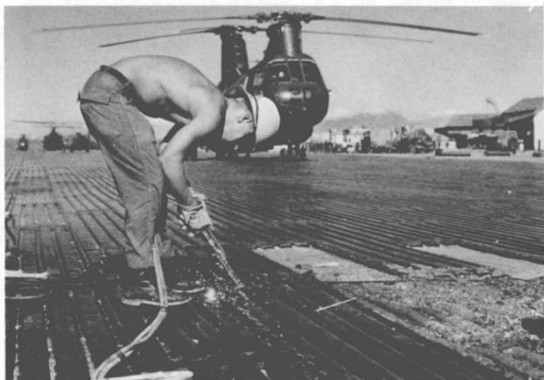
71. M8A1 Parking Apron Repairs—Dong Ha. Seabees of NMCB-11 repair and relay a type M8A1 steel matting of a parking apron which was damaged by enemy mortar fire.
