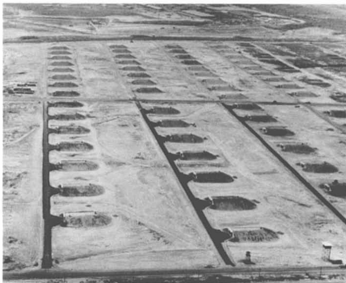
31. Ammo Storage Facility at Long Binh. These massive earth-covered concrete and steel Stradley ammunition bunkers were among the final projects completed by RMK-BRJ.
