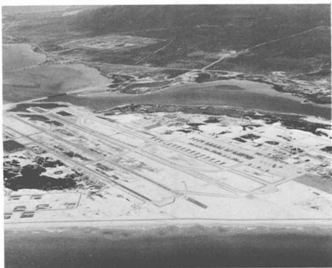
22. Cam Ranh Airfield—Completed. The 17-mile Cam Ranh Peninsula is characterized by rolling sand dunes. The original 10,000' interim (expeditionary) runway/taxiway was constructed of AM-2 (aluminum matting), shown in the left half of the airfield in the photo. A parallel permanent 10,000' concrete runway/taxiway was then added to complete the basic airfield.
