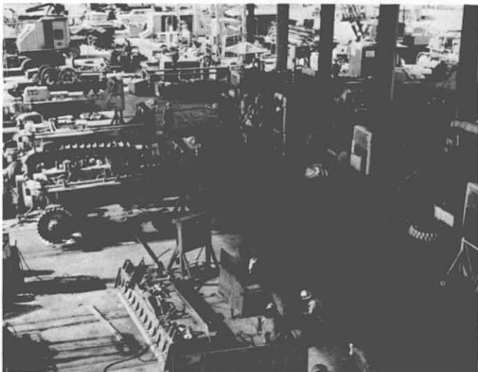
40. Contractor Equipment Repair Shop. In 1964, RMK built the following shops: Carpenter, combination Mechanics and Welding, Electrical, and Plumbing. Millwork, mechanical repairs (as shown in the photo)—for all construction sites throughout the Delta—were accomplished at these shops.
