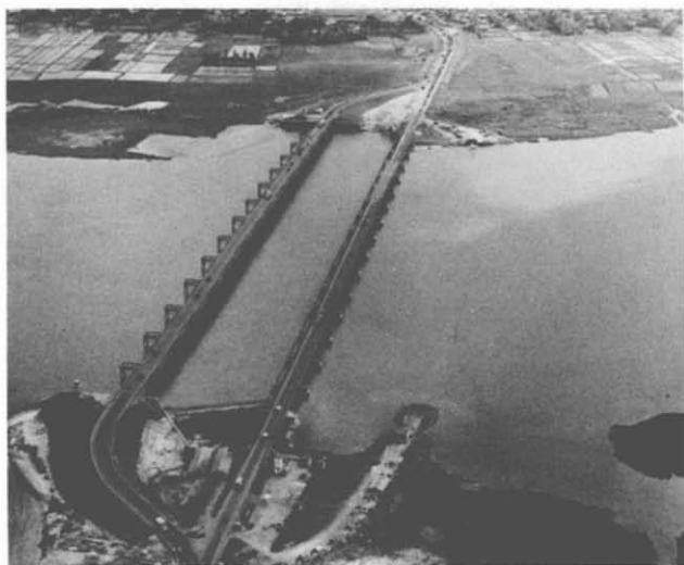
51. New Da Nang Bridge. A second Da Nang Bridge was authorized in June 1966, to be built adjacent to the existing bridge which separated Da Nang East from Da Nang West. The new bridge (left, in photo) was designed for multiple parallel bridge spans, each having a 24' roadway. Only one span was installed; the second span was to be added in the future, if needed. Total length was 1,680 feet between abutments, with 13 piers in the river. The bridge elements were prefabricated at Poro Point, Philippines. Work on the abutments and piers began in September 1967 and the bridge was completed and in use within 10 months.
