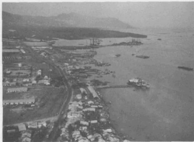
6. Vung Tau Waterfront. In early 1966, Vung Tau was the waiting point for vessels awaiting availability of deep-draft berthing space upstream at Saigon. The DeLong mobile pier (upper-middle of photo), subsequently built, is a 2-berth finger pier extending from an earth causeway. In the center of the photo, 3 tankers are tied up to a POL pier.
