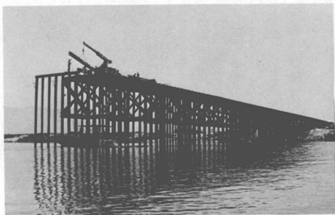
84. View of "Liberty Bridge." This 2,040' timber bridge is the longest ever built by the Seabees. It is also the longest timber bridge in Vietnam.
