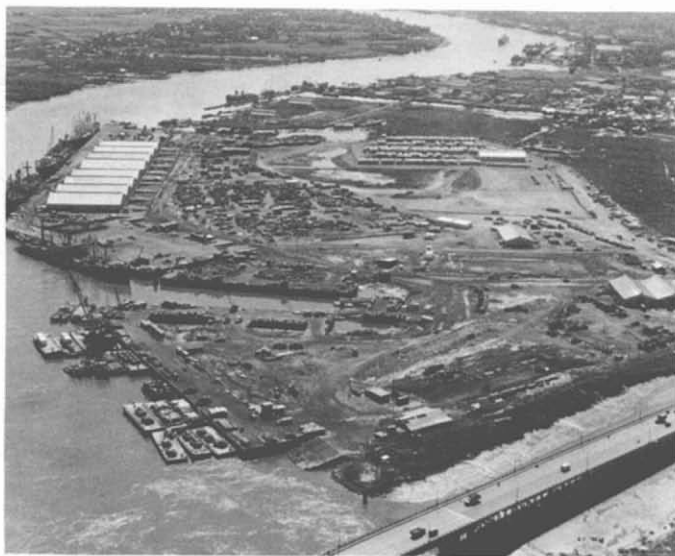
19. Newport (Saigon)—Completed. The 100-acre Newport project required 2,000,000 CY of fill. It took a total of 4,050 steel piles (a combined length of 107 miles); 35 miles of structural steel was used. The 760,000 SF staging deck required a pour of 18,000 CY of concrete. Total construction time was 15 months. Newport can accommodate, simultaneously, 4 ocean-going vessels, 2 fleet-size LSTs, 7 barges, and 2 LCMs. The estimated cargo handling capability is 150,000 tons per month. Newport was "turned over" to the Army First Logistical Command on 10 July 1967.
