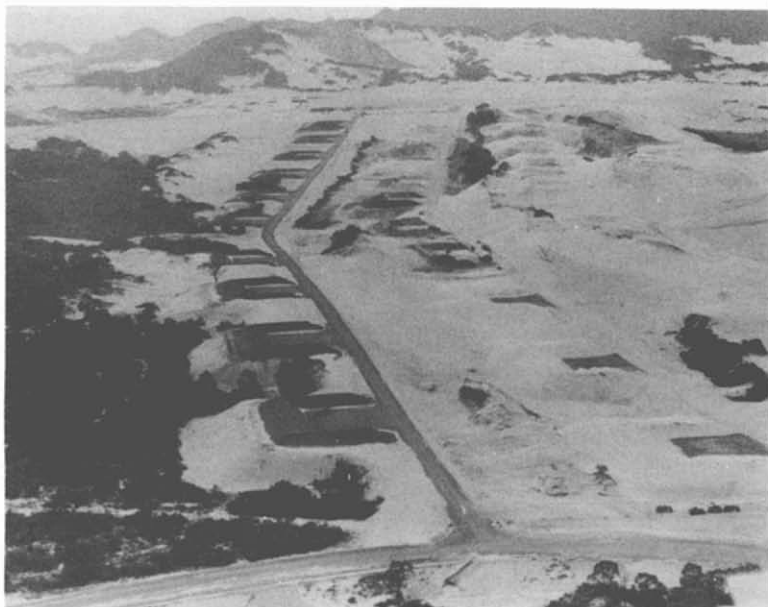
27. U.S. Army Ammo Supply Point at Cam Ranh Complex. The problem of construction in a sand dune environment is obvious here. Both the open and revetted hardstands measure 50' \times 128' \times 8' . The revetments go around 3 sides and are 12' high.
