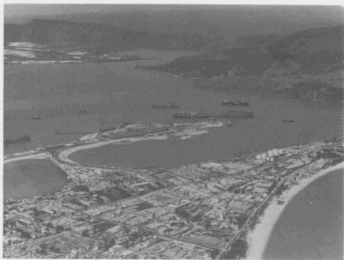
4. Qui Nhon Harbor. The man-made deep-draft facility at center of photo called for dredging an entrance channel and turning basin and depositing the fill on a Japanese constructed rock breakwater. The fill formed a 30-acre staging area. The T-shaped pier is composed of four joined mobile DeLong units.
