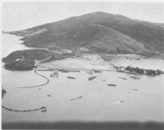
1. Observation Point (Da Nang) Port Facility—July 1966. Work involved dredging an entrance channel and turning basin to a depth of 39 feet; the bulk of the dredged material was used to fill a 45 acre tidal swamp, thereby creating a staging area for off-loaded supplies. A 2,000 sheet piling bulkhead (seawall) was built. Two jacket-type piers were to be installed. Each pier is 90' \times 600' . These piers were prefabricated at Poro Point, Philippines, by RMK-BRJ and shipped by barge to Da Nang. The abutment for a third pier, a mobile DeLong type, was also in the job.
