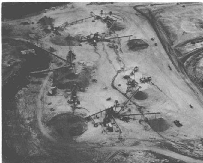
37. University Quarry—Saigon. This site derived its name from the fact that it was near the future Saigon University. In February 1966, a few months after its opening, the quarry had a 250 tons-per-hour crushing plant in operation, making rock for use throughout the greater Saigon area. In November 1966, a 400 ton-per-hour crusher was added and aggregate production jumped to an average of 6,500 tons per day. In January 1967, a hot-mix asphalt and concrete batch plant were set up. The new diversity of products led to the imposing new site title: "Saigon University Materials Products Company" or, for short: SUMPCO.
