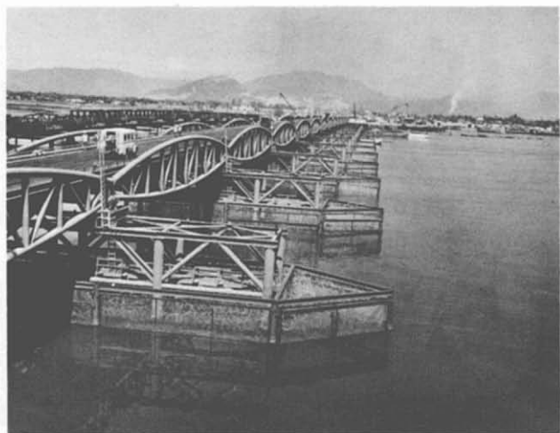
52. New Da Nang Bridge Detail. Bridge pier protection was undertaken as a deterrent to enemy attempts (by frogmen and floating charges) to destroy or damage the structure. Pier protection included pier lighting and approach lighting; steel bracing to pier structure for added support; and framing, chain link panels, and loosely-placed concertina wire.
