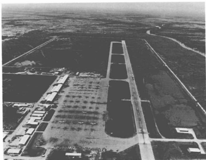
14. Binh Thuy Airfield. Located about 100 miles southwest of Saigon. This is a 6,000' asphaltic-concrete runway; it was built in August-October 1964. The asphaltic-concrete parking apron is 165,000 SY.
