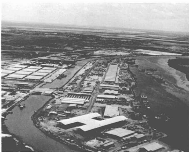
41. Saigon Island Depot (RMK-BRJ). This is Thu Duc Island—one of RMK-BRJ's 3 such depots in South Vietnam. Originally marsh land, this GVN-owned island required filling and stabilizing of 590,000 SY of area, and the hauling of 1,200,000 CY of sub-base material, and 240,000 CY of rock for surfacing the area. The Thu Duc Depot included major repair shops, warehouses, open storage areas, and marine construction facilities.
