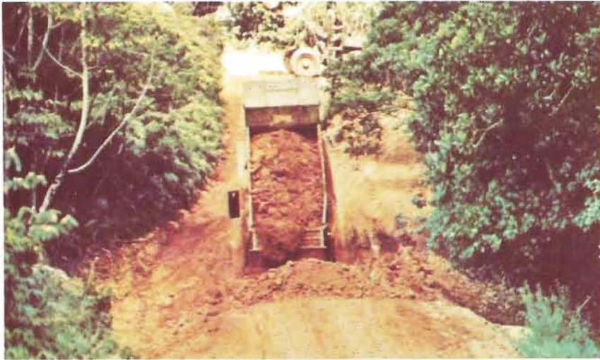
Yap's road building program is important . . .
