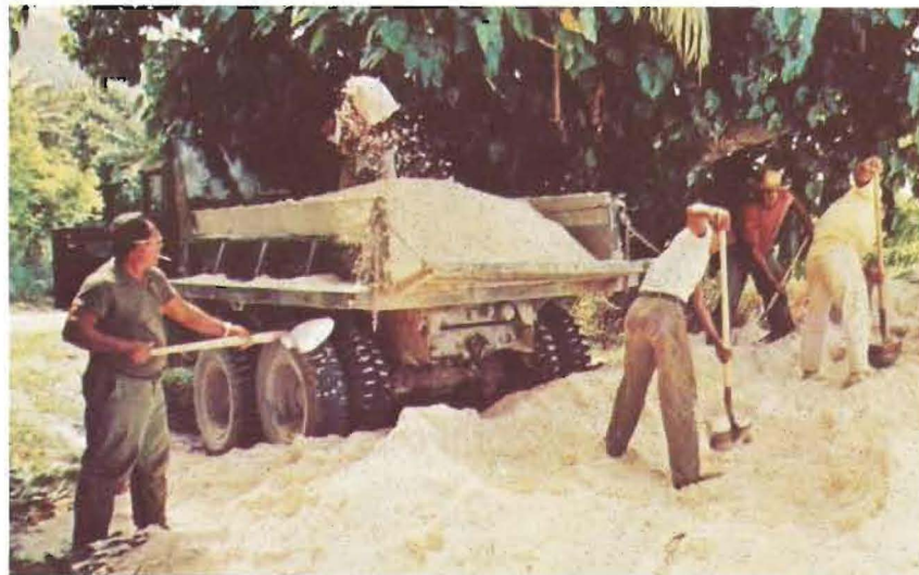
Local coral is used for road work.
