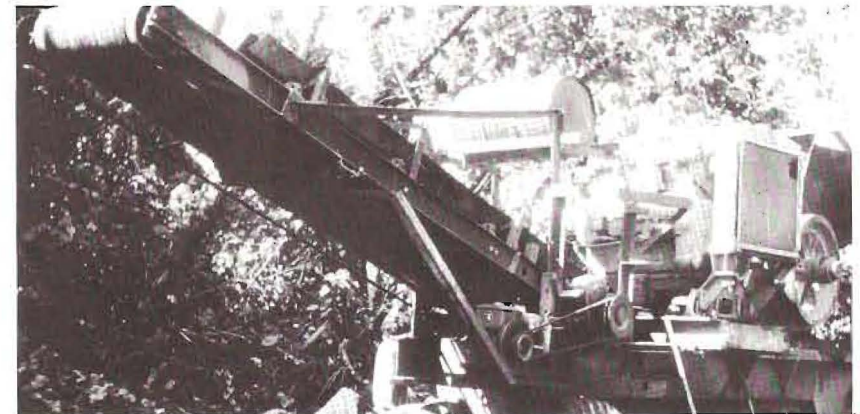
. . . to this Seabee-repaired crusher . . .
