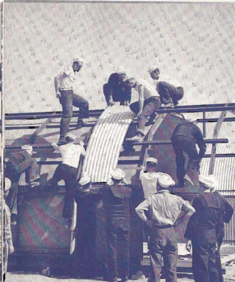
At a Virginia training center, Seabees learn how to build the famous Quonset huts in which they will live overseas.
