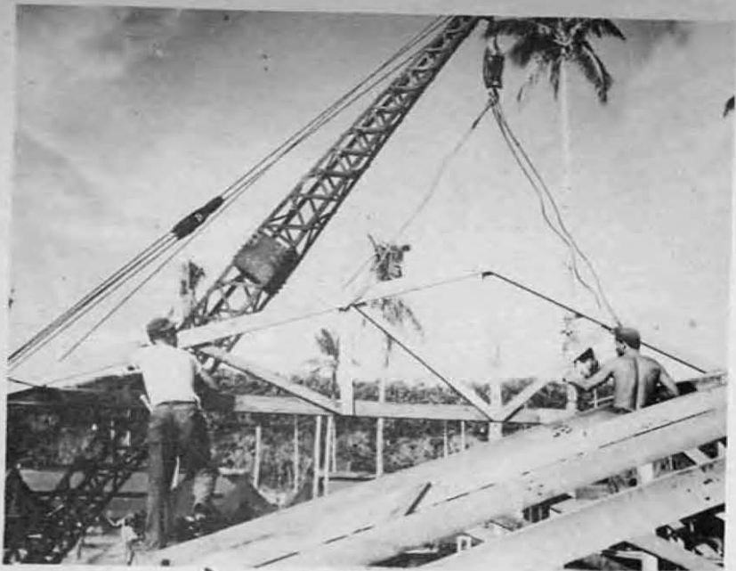
Cross Beam Placing Early Reefer
