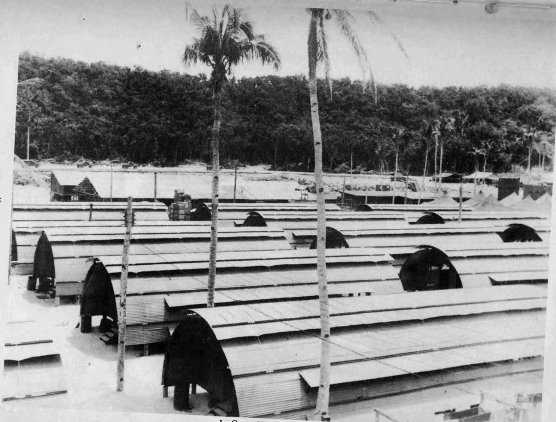
As' Camp Nears Completion
