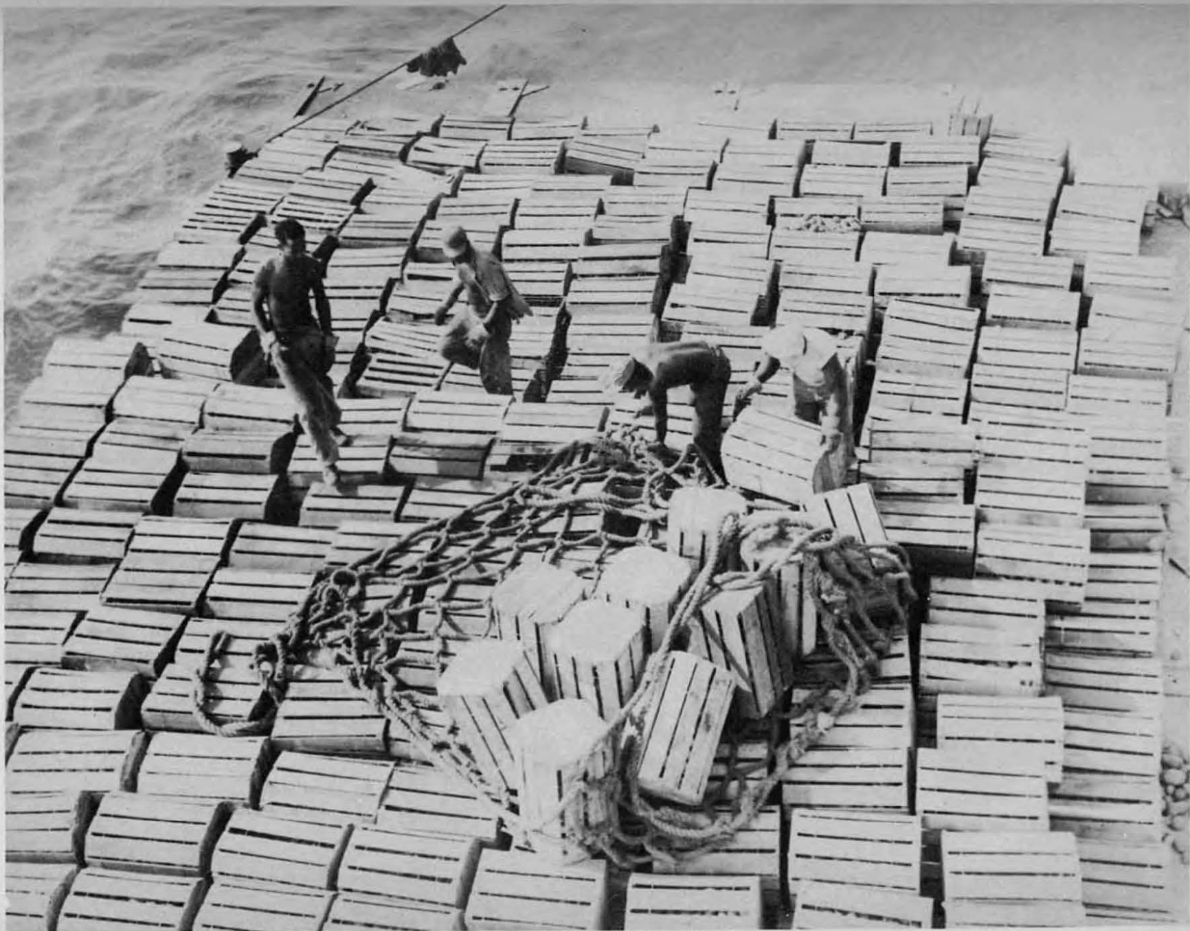
Barge Load of Spuds
