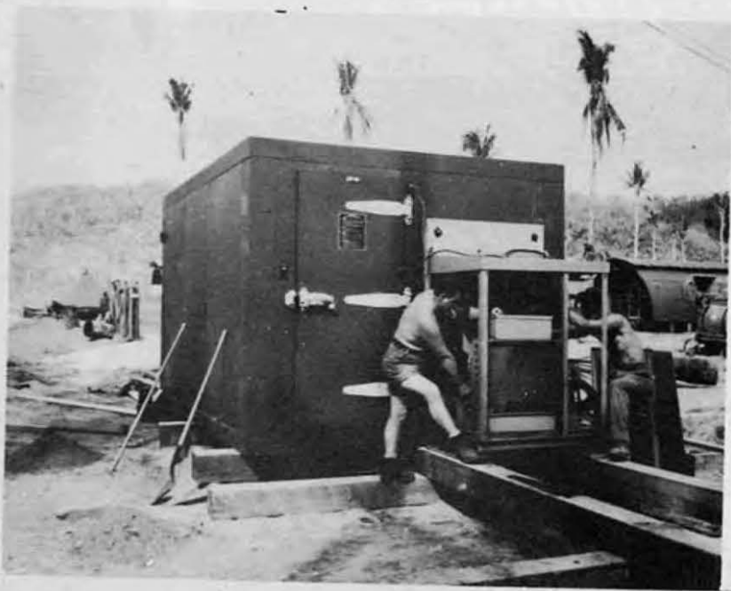
Cross Beam Placing Early Reefer
