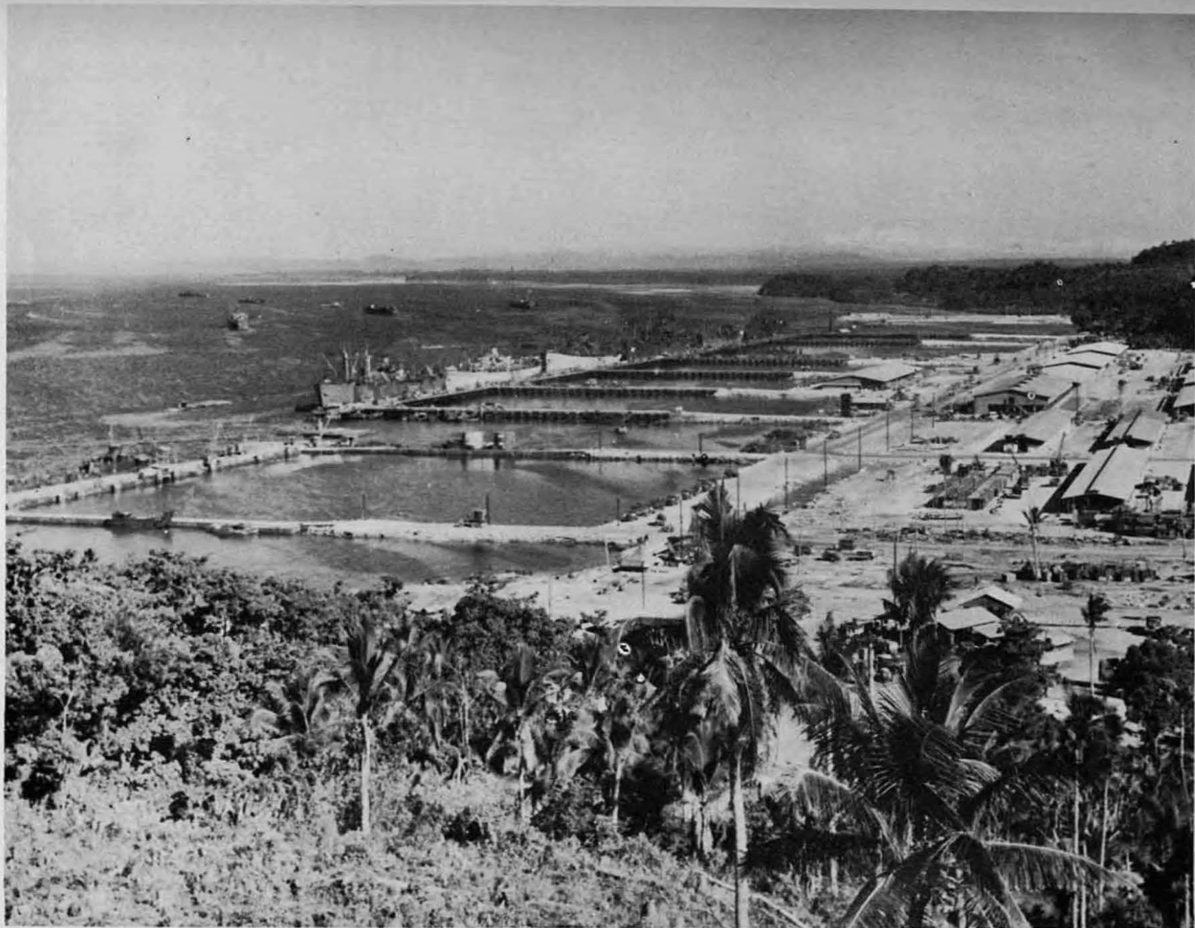
View of Calicoan Docks and Anchorage
