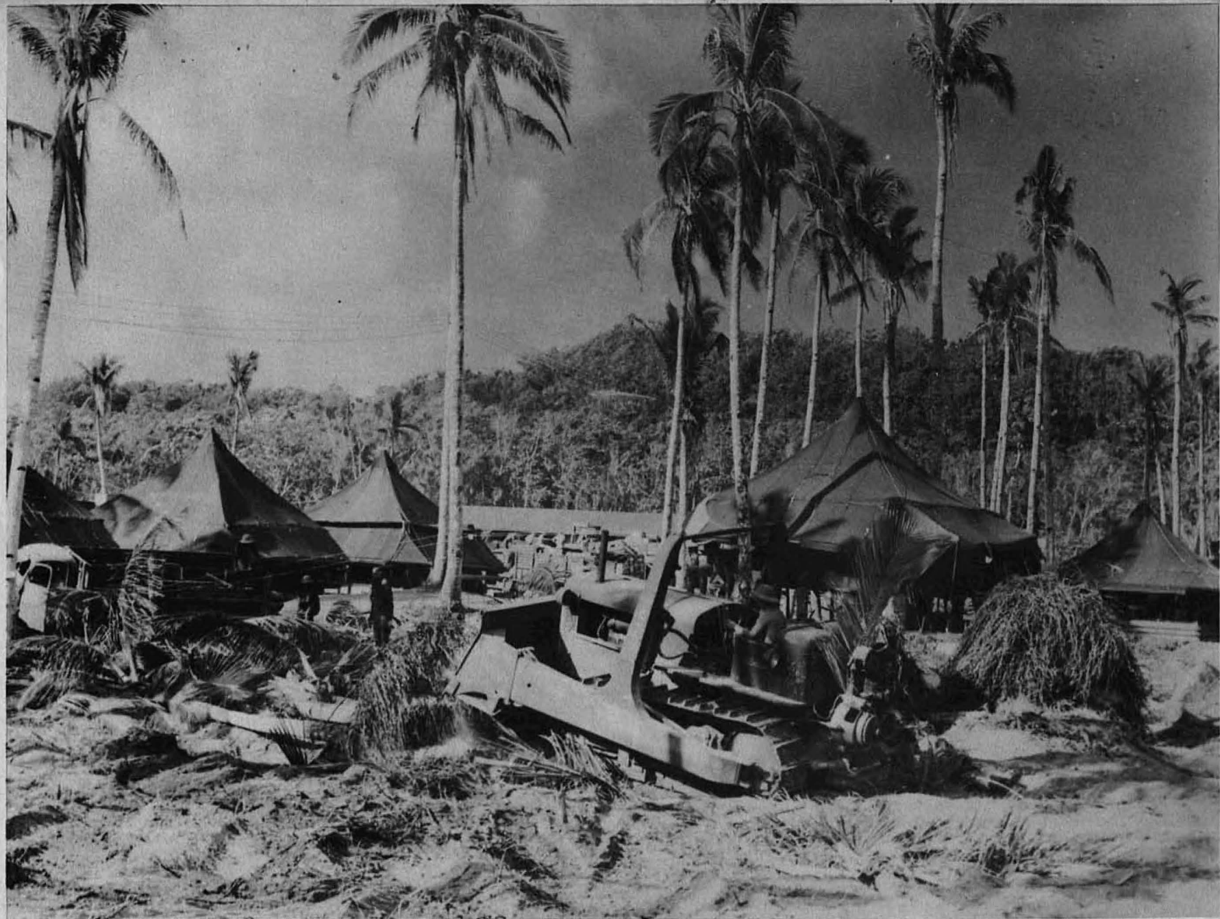
Clearing the Way
