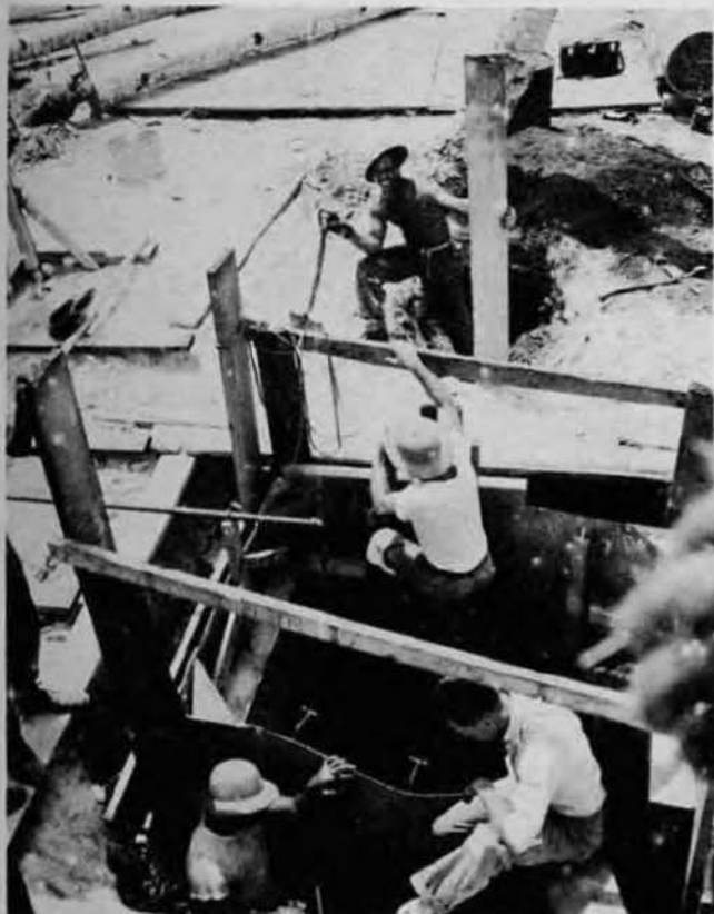
Drilling Water Well
