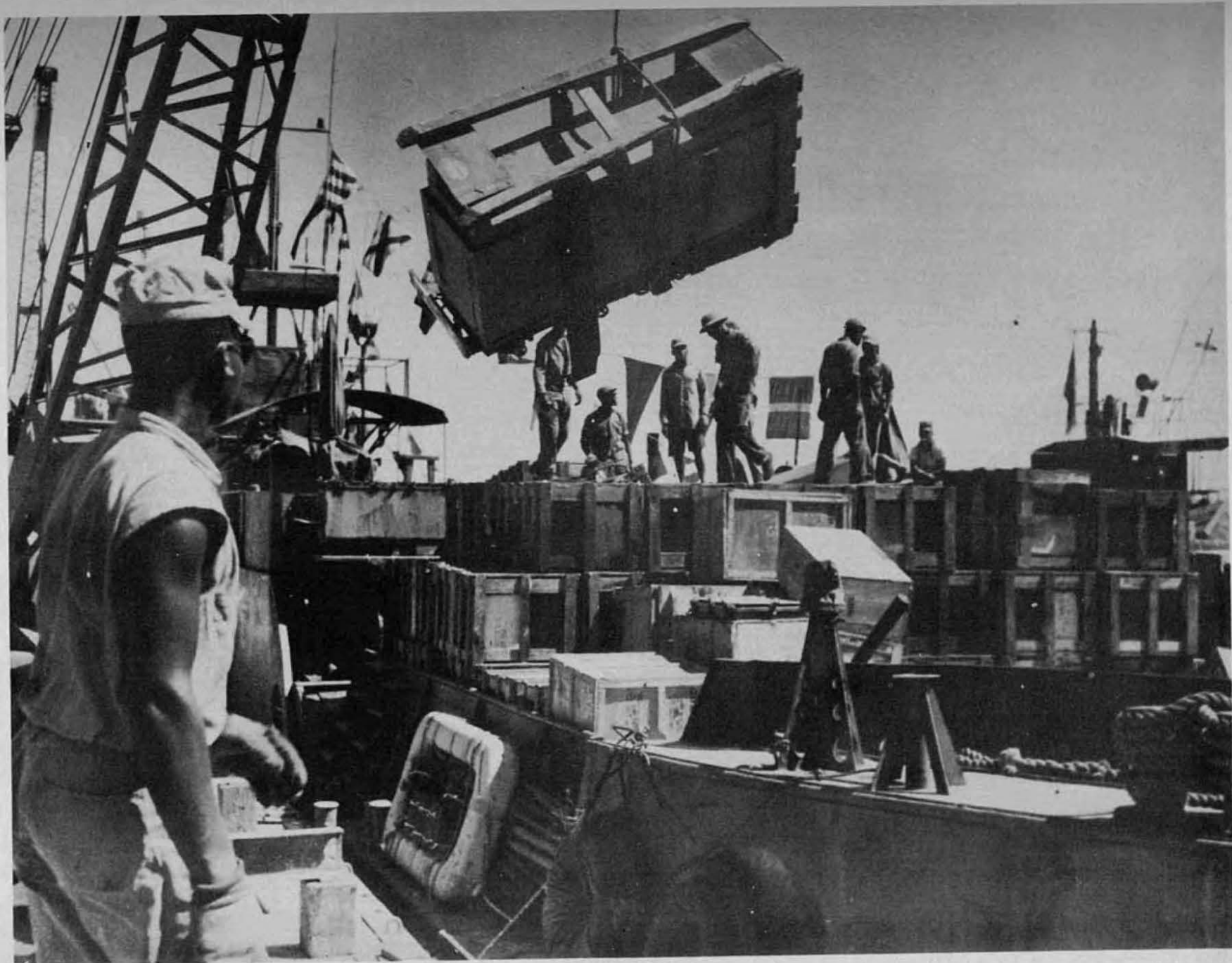
Close-Up of LCT Discharging
