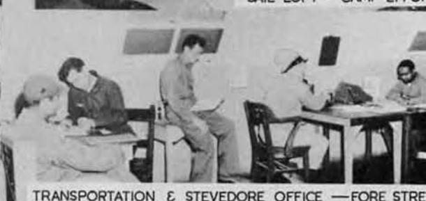
TRANSPORTATION & STEVEDORE OFFICE — FORE STREET
