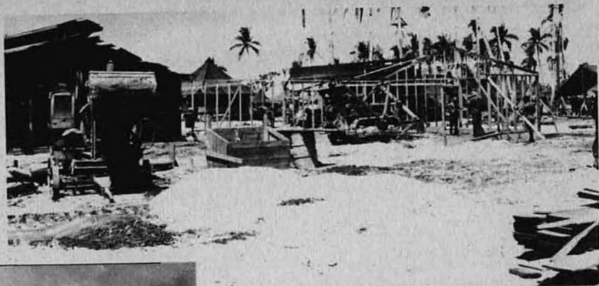
Carpenters at Work
