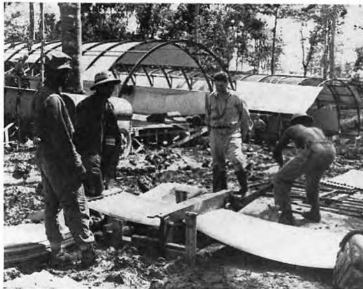
QUONSET HUT CONSTRUCTION
