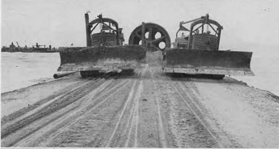
UNLOADING CABLE FOR 125-TON CRAWLER
