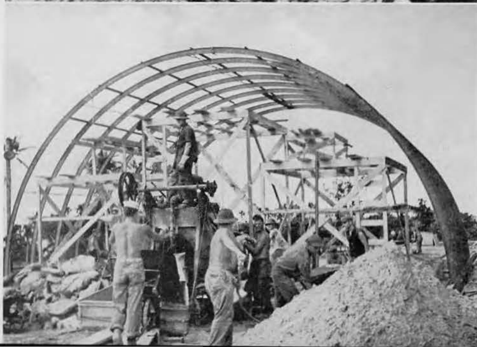
POURING CONCRETE FOR CHOW HALL
