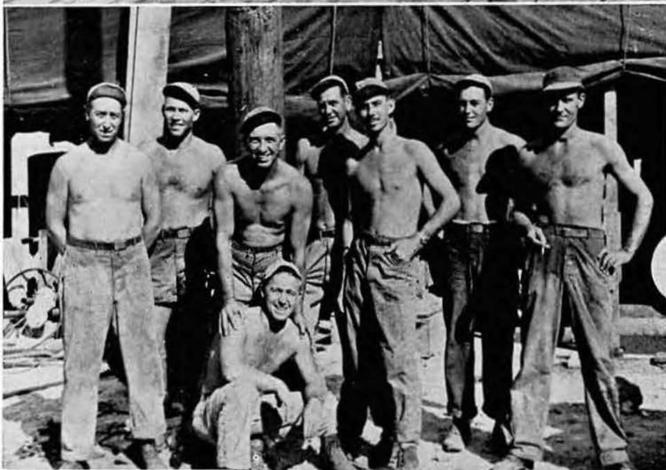
96TH ELECTRICIANS AT SHIP REPAIR BASE
