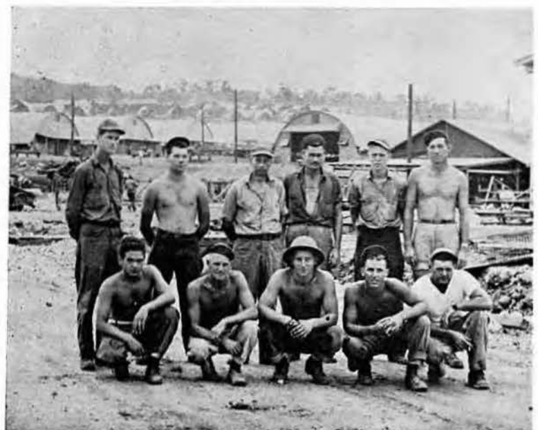
CEMENT FINISHING CREW
