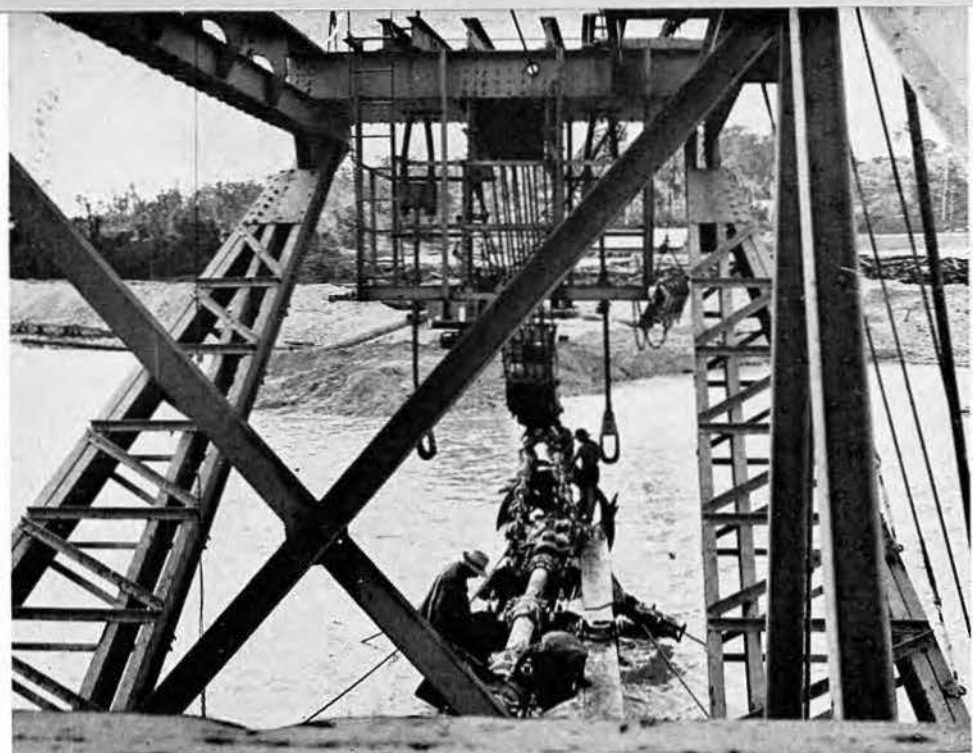
DREDGE SUCTION AND CUTTER HEAD
