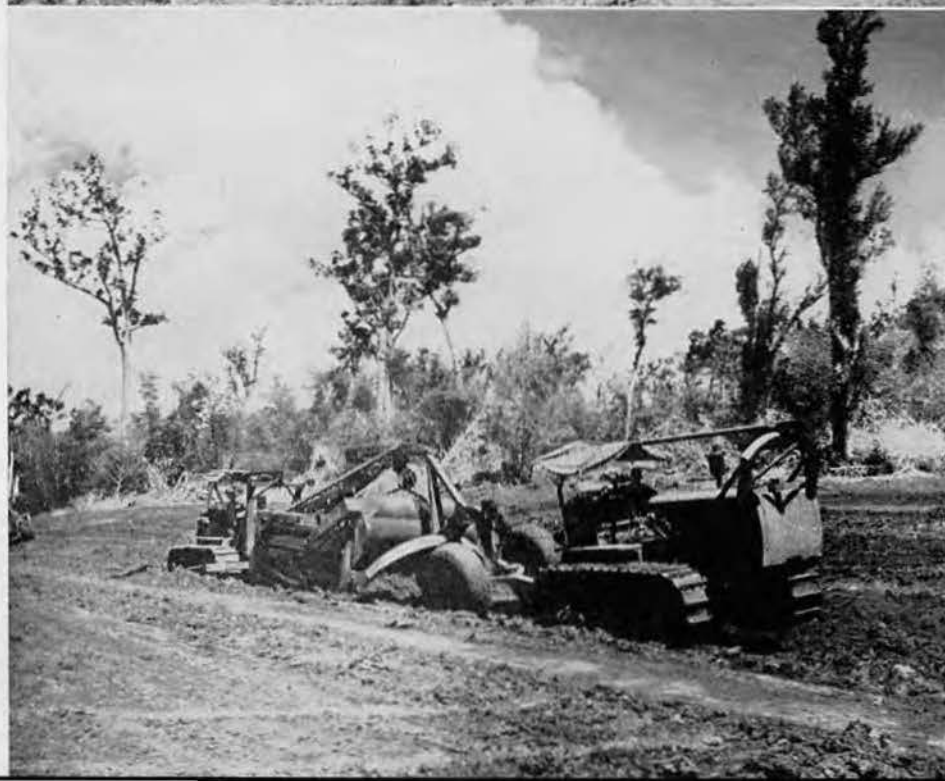
D-8 WITH SCRAPER GRADING COMPOSITE
