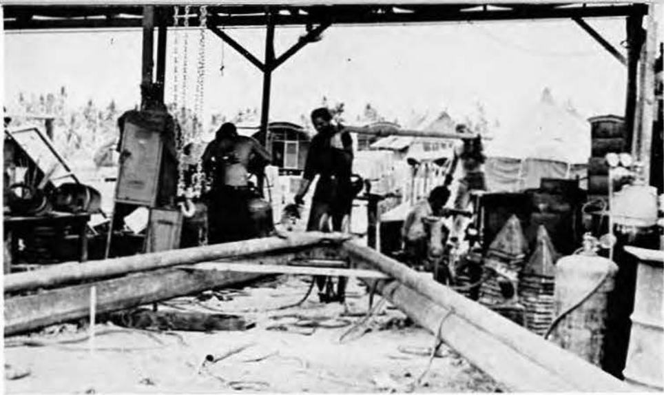
WELDING SHOP FABRICATING BARGE 'A' FRAME
