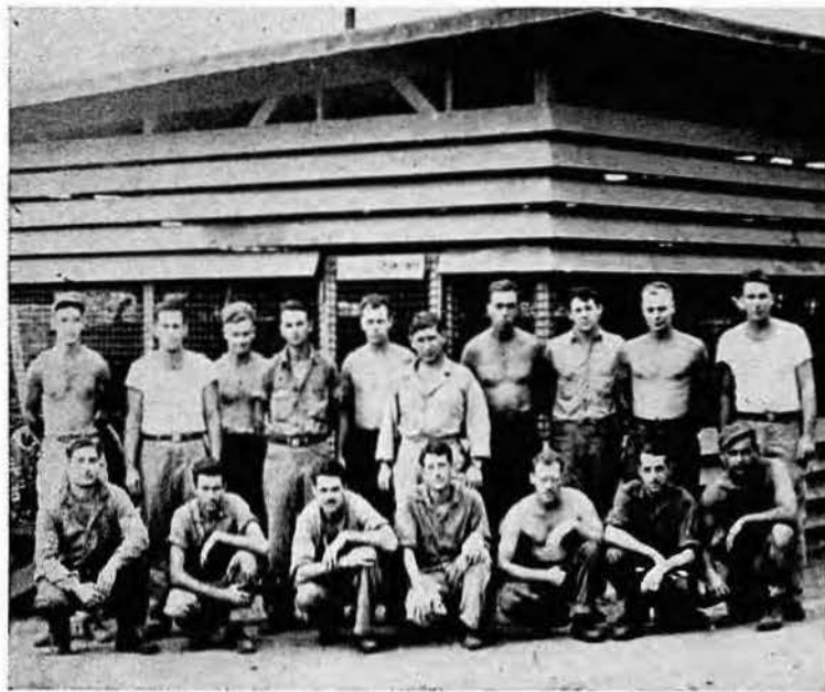
CHIEF WALKER'S ELECTRICAL CREW
