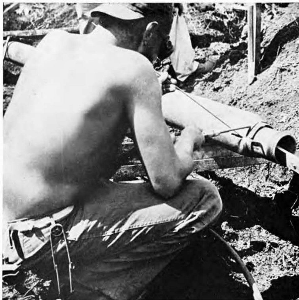
WATER LINE WELDER
