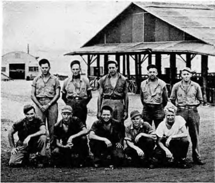
CHIEF CLINI AND CARPENTER CREW
