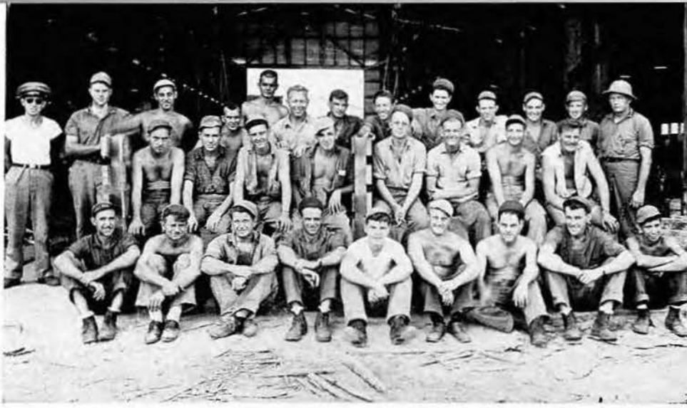
ELECTRICAL CREW WORKING AT S.R.B.
