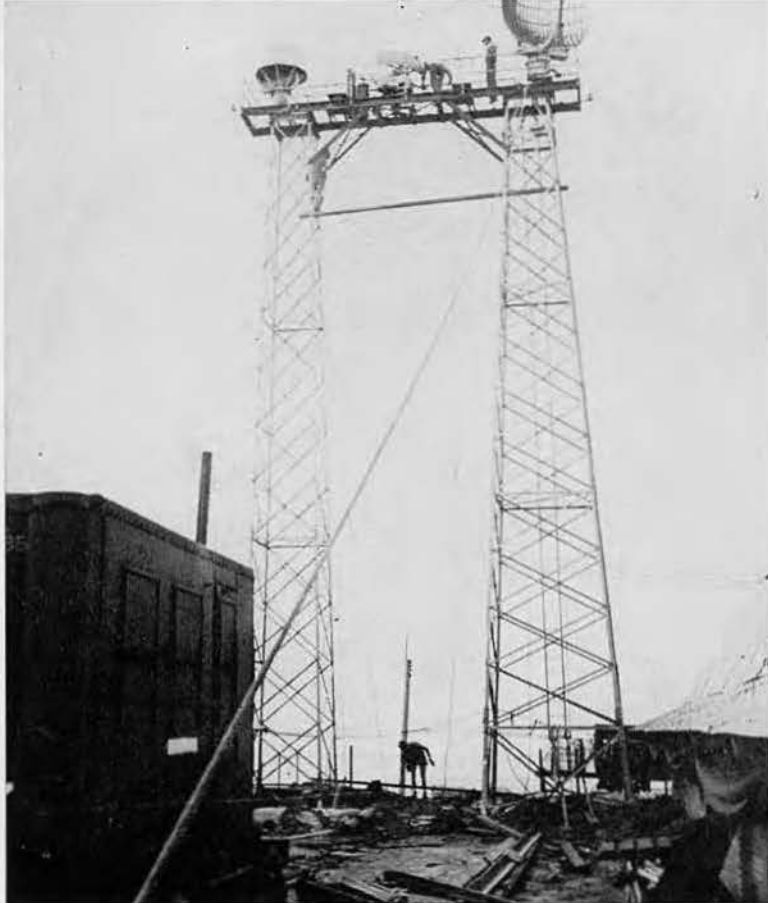
A RADAR TOWER GOES UP
