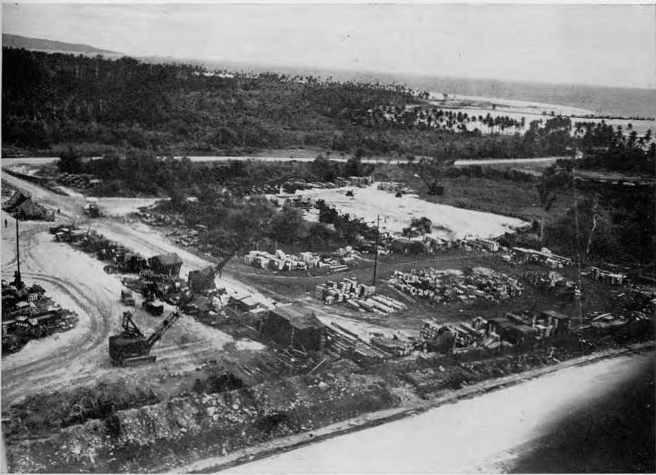
96TH STORAGE YARD AND MECHANICAL REPAIR AREA
