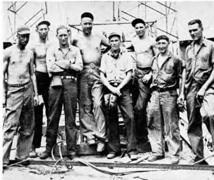
TOWER ERECTION CREW
