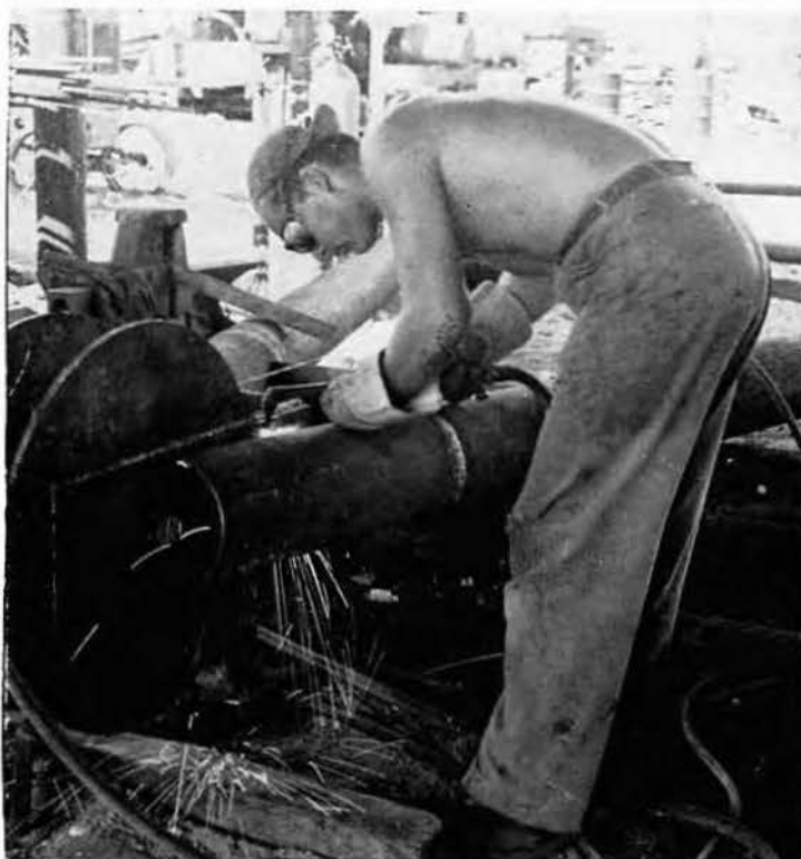
WELDER WORKING ON BARGE FRAME
