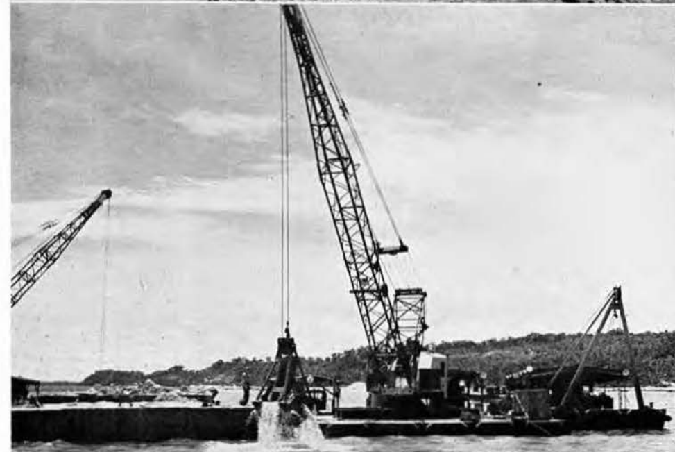
96TH-BUILT CLAMSHELL CRANE DREDGE IN OPERATION OFF CALICOAN
