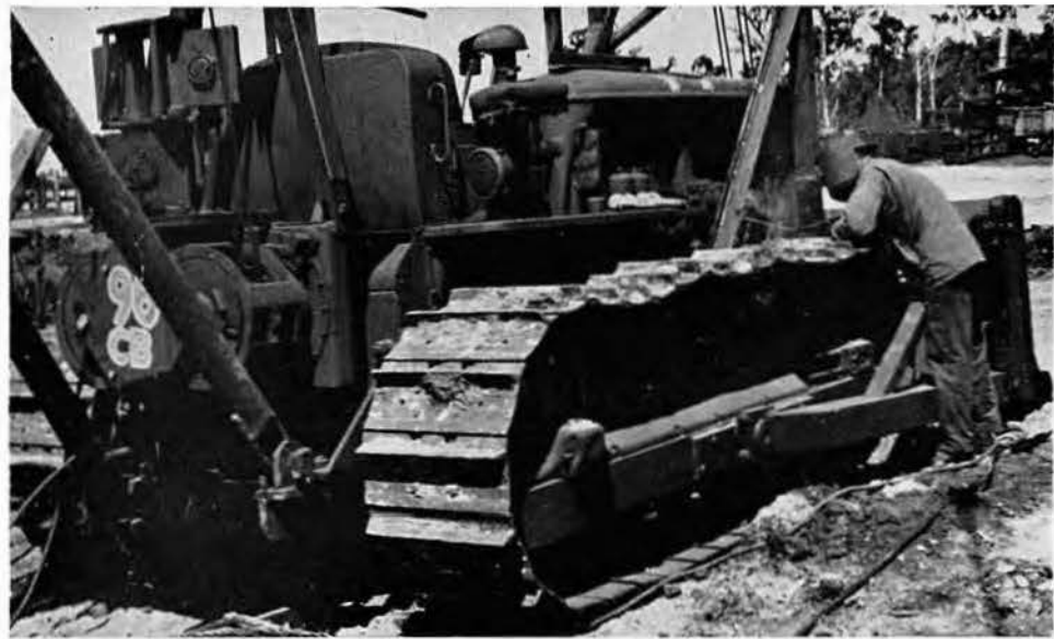
WELDING ON A D-7
