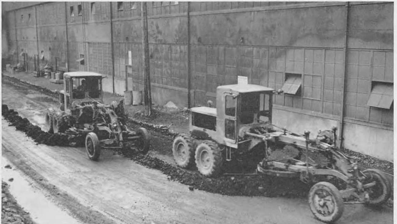
The Roads and Runway department kept the roads in excellent condition. Motor Patrols were worked constantly because of rain and snow.
