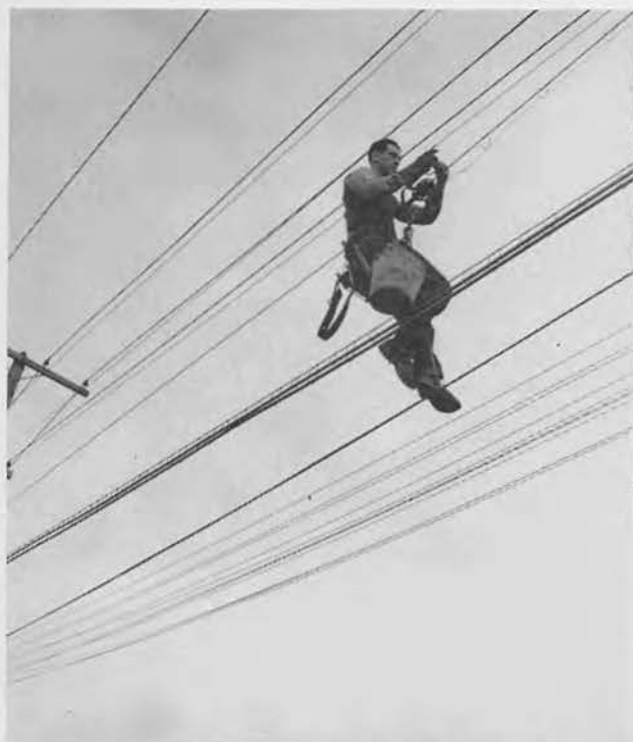
Ringin strand preparatory to pulling cable.
